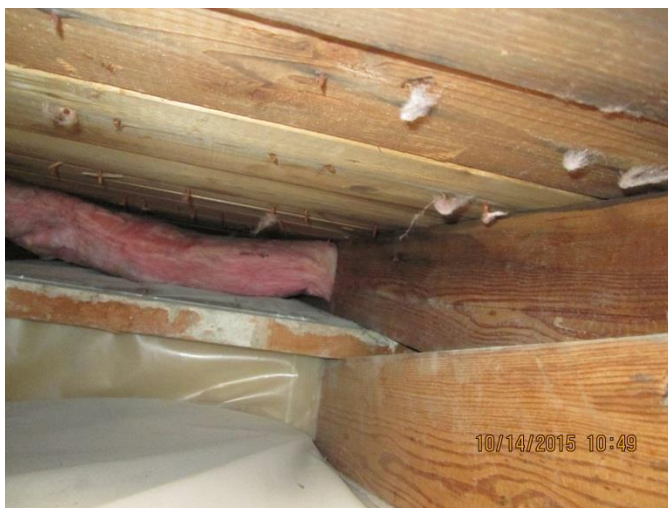
Figure 3: Close-up View of Roof Rafter (Upper Beam) and Outrigger Rafter (Lower Beam)
