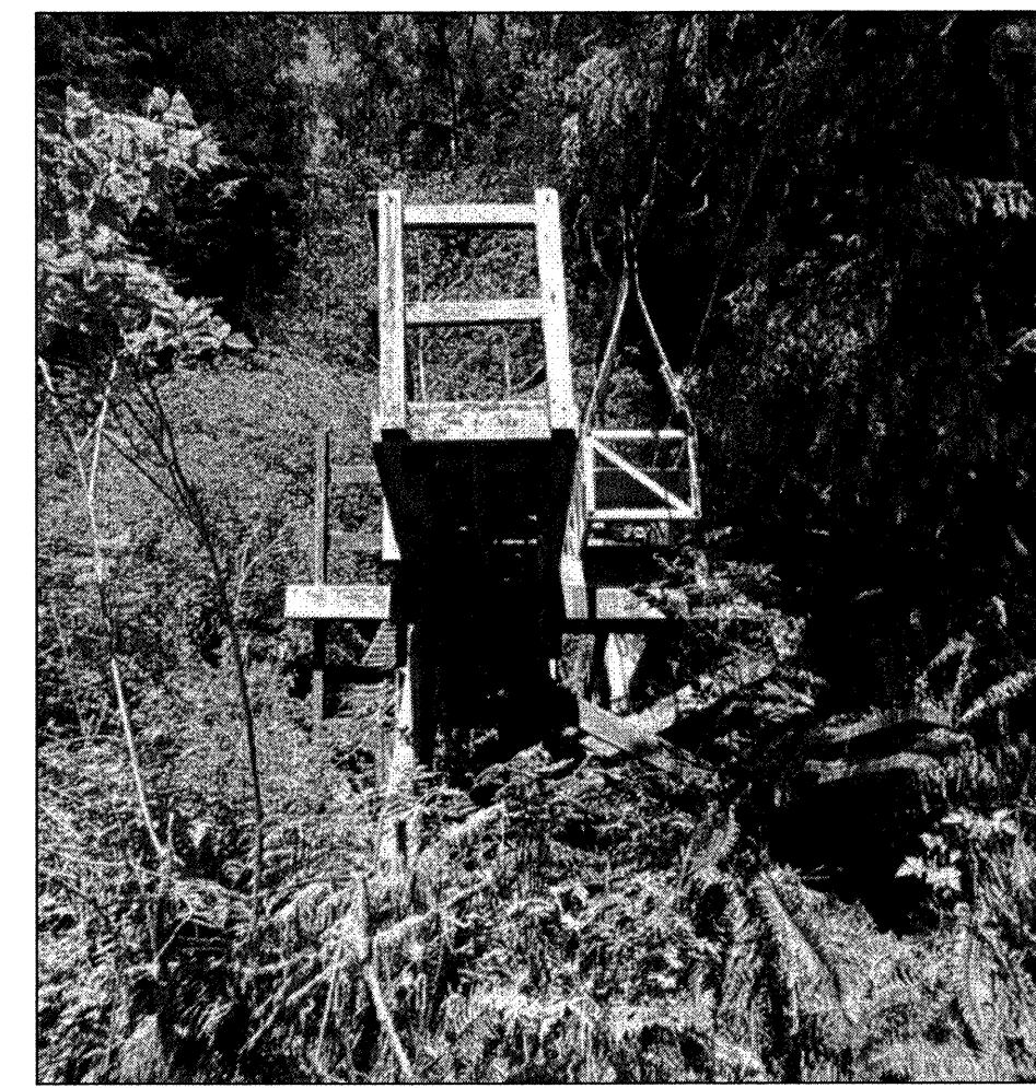
EXISTING WEST TOWER
