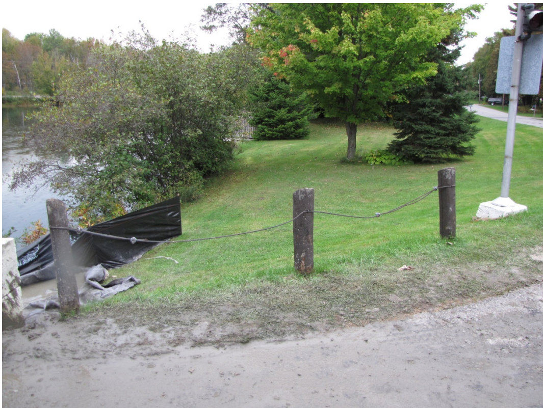
Photo F34: The two end posts of the north-east guide rail are rotten.
