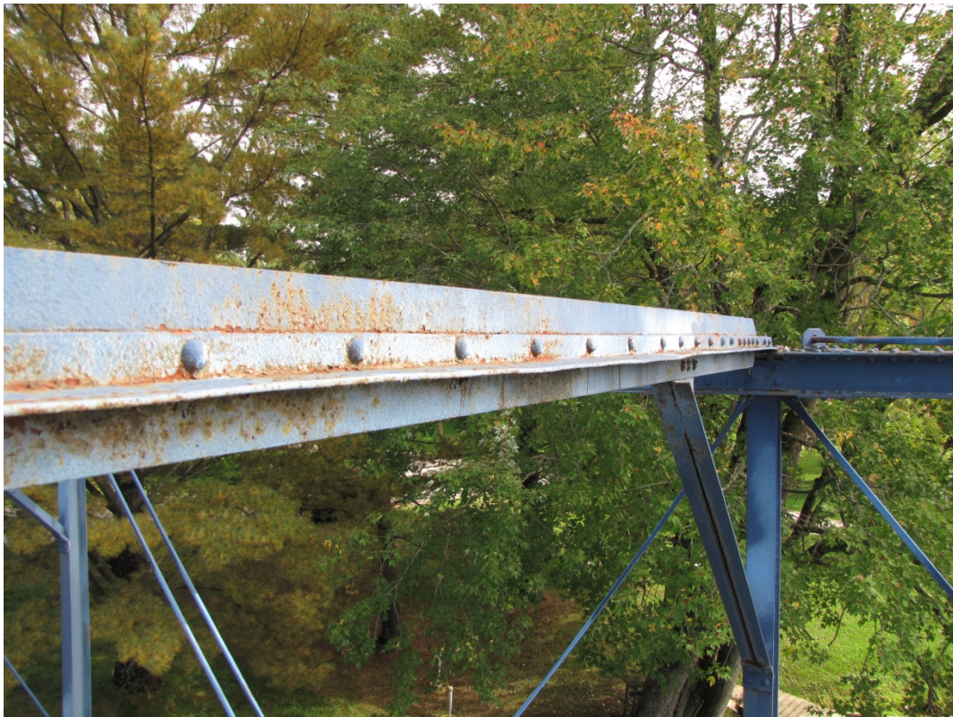
Photo F13: West horizontal flange of the lateral bracing member 4S-4N is deformed along its length.
