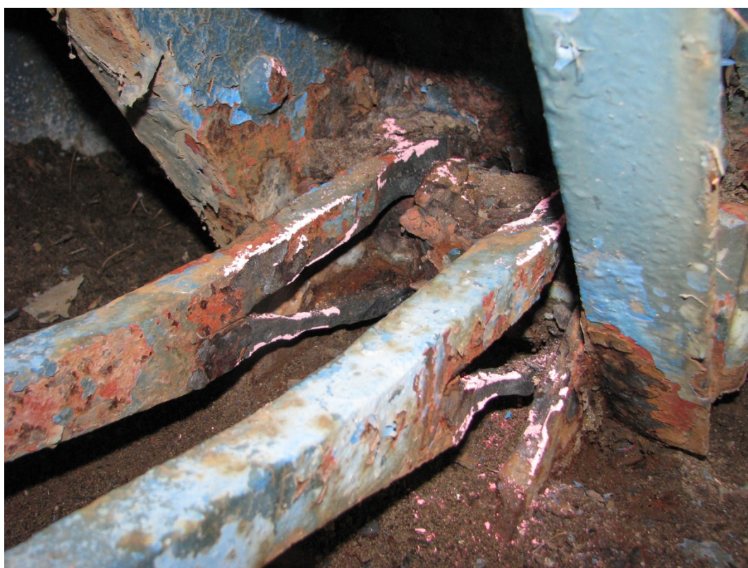
Photo F20: Very severe section loss in the south bottom chord I-bars at the east end of bridge.
