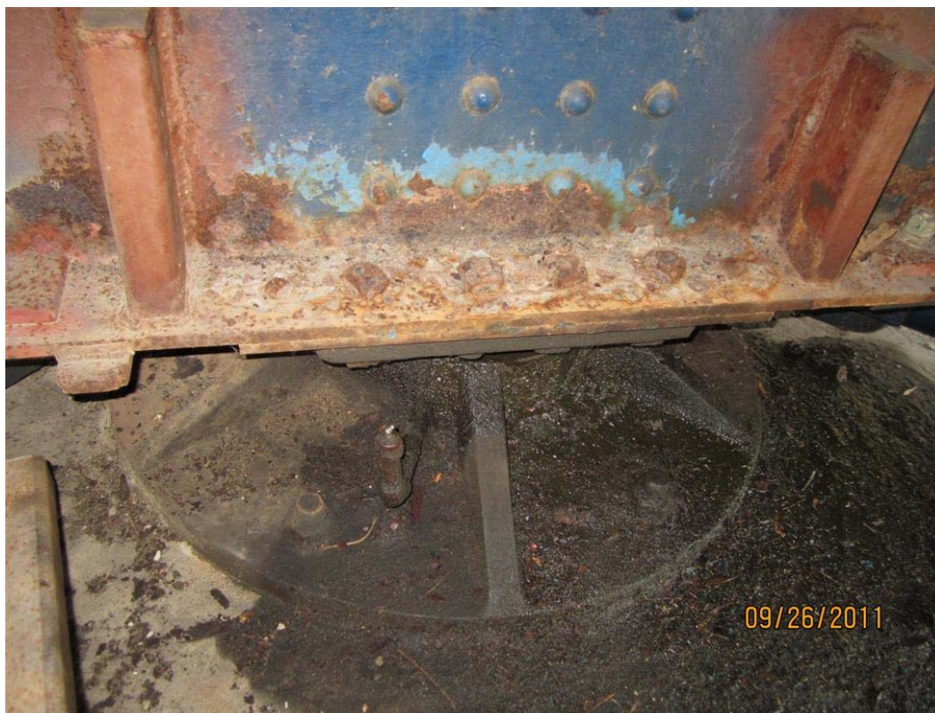
Photo M1: The center pivot top plate mounting bolts exhibit moderate corrosion with moderate section loss.
