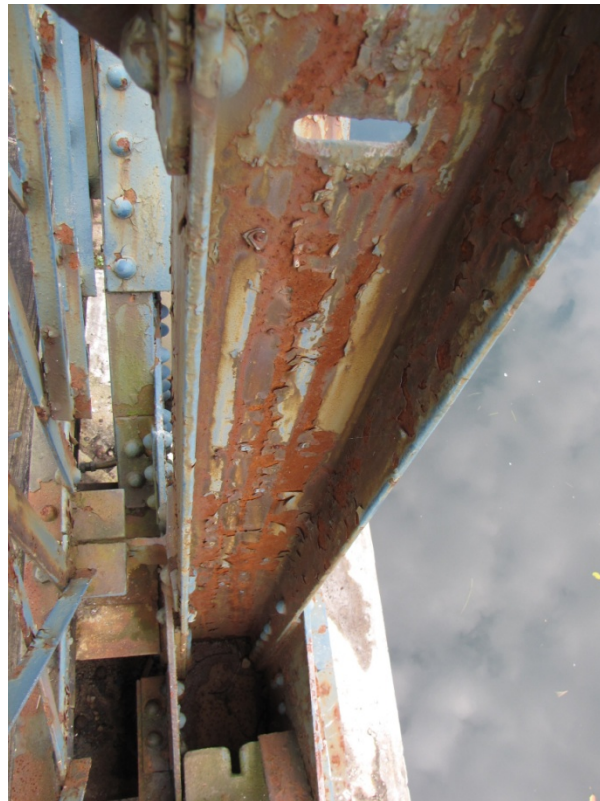
Photo S36: West side of V5S with extensive coating loss.
