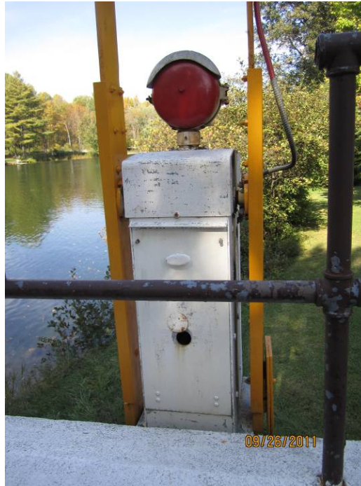
Photo E15: Typical Traffic Gate. Note the gong is provided on top of the gate enclosure to provide audible warning for the traveling public. Also note the cutout for the hand crank mechanism.
