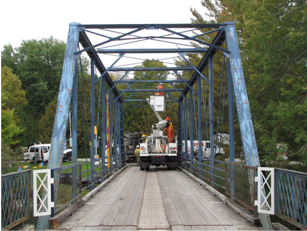
Photo F3: Looking east. Note the typical condition of the coating on the end top chord members.
