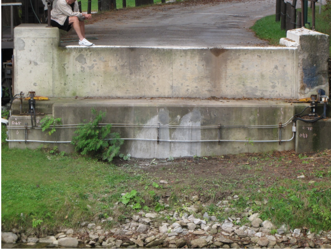
Photo S19: The west abutment is in good condition. Note the minor erosion of the embankment.
