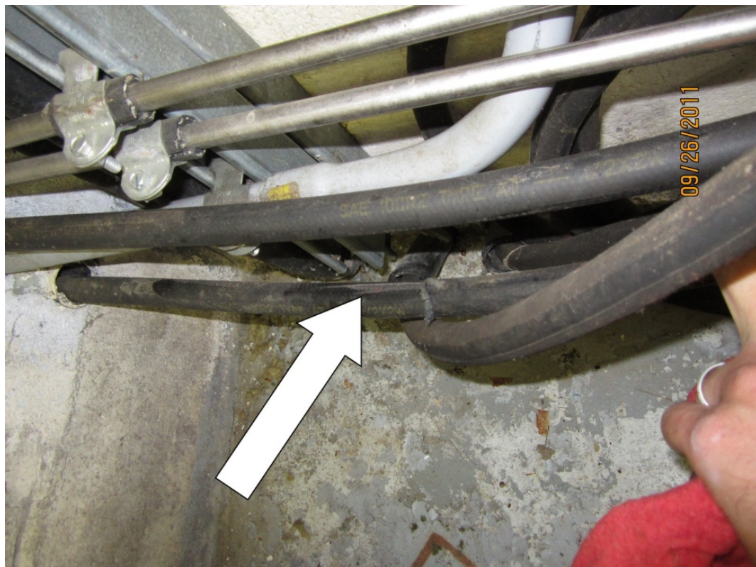
Photo M16: HPU. One hose is abraded at a location near the hose exit from the operator's house.
