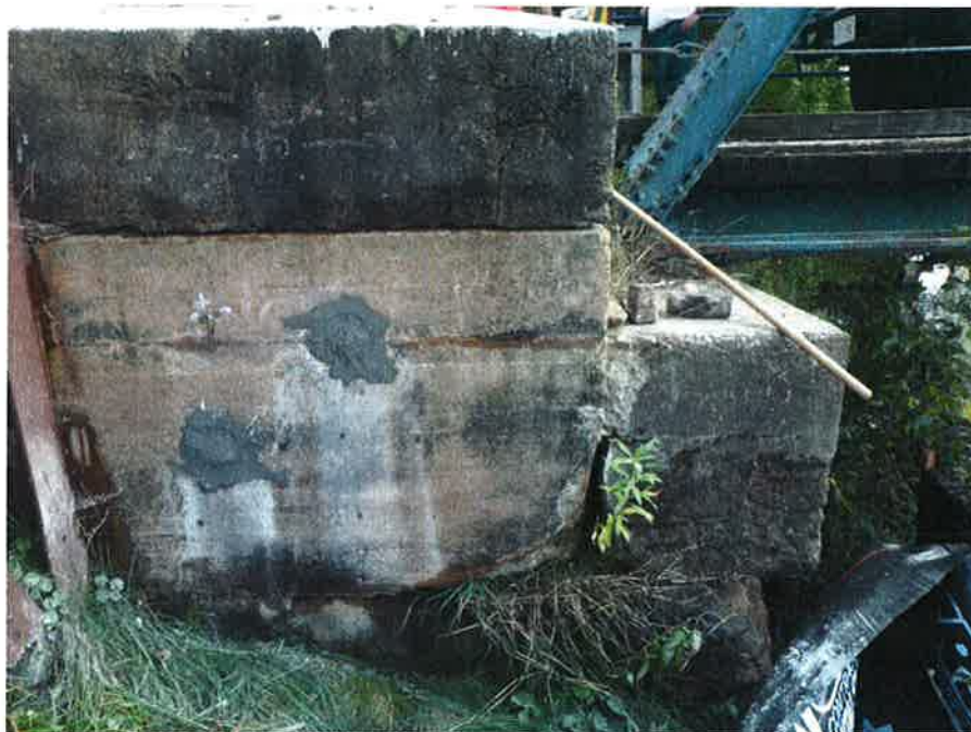
Figure 4-6 Overview of northeast wingwall with locations of cores C5 (upper) and C6 (lower).
