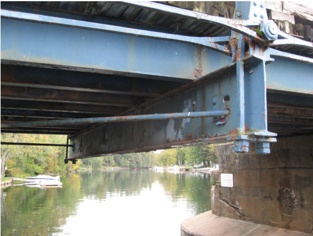
Photo F22: Typical condition of the lower truss connections and floor beams.
