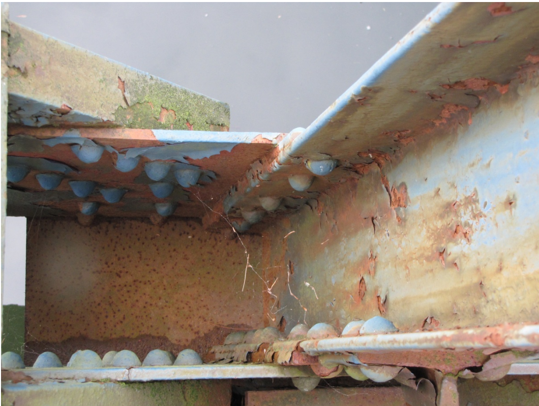
Photo S34: Typical condition of the coating system and truss members at the lower connections.
