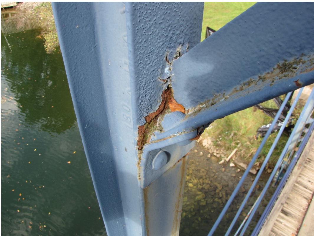
Photo F14: V5N – typical localized section loss of the interior flange of the vertical members at the connection to the vertical bracing.
