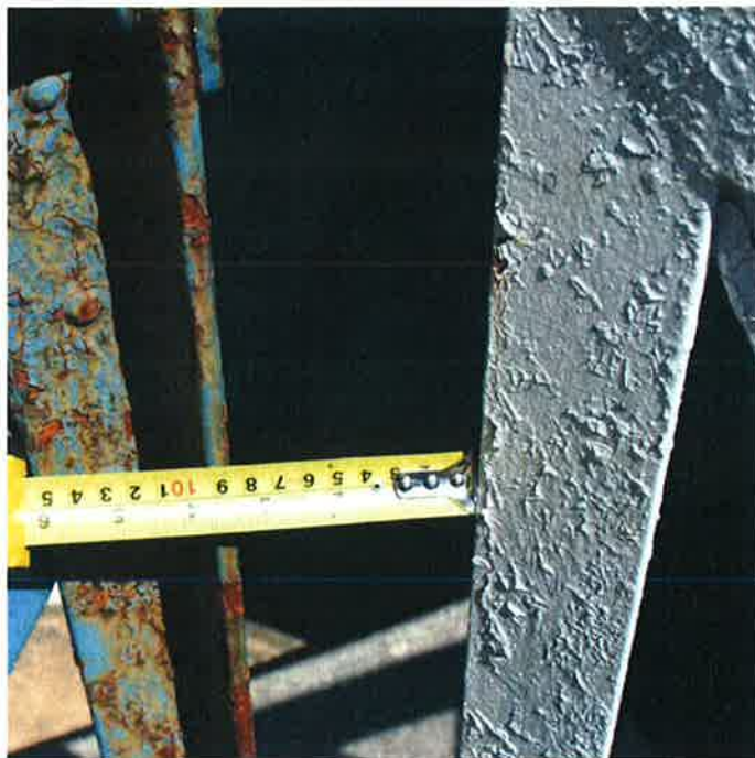
Picture 1: The space between the guardrails of the swing bridge and fixed bridge on the north side; the space was reported to be wider in the past.
