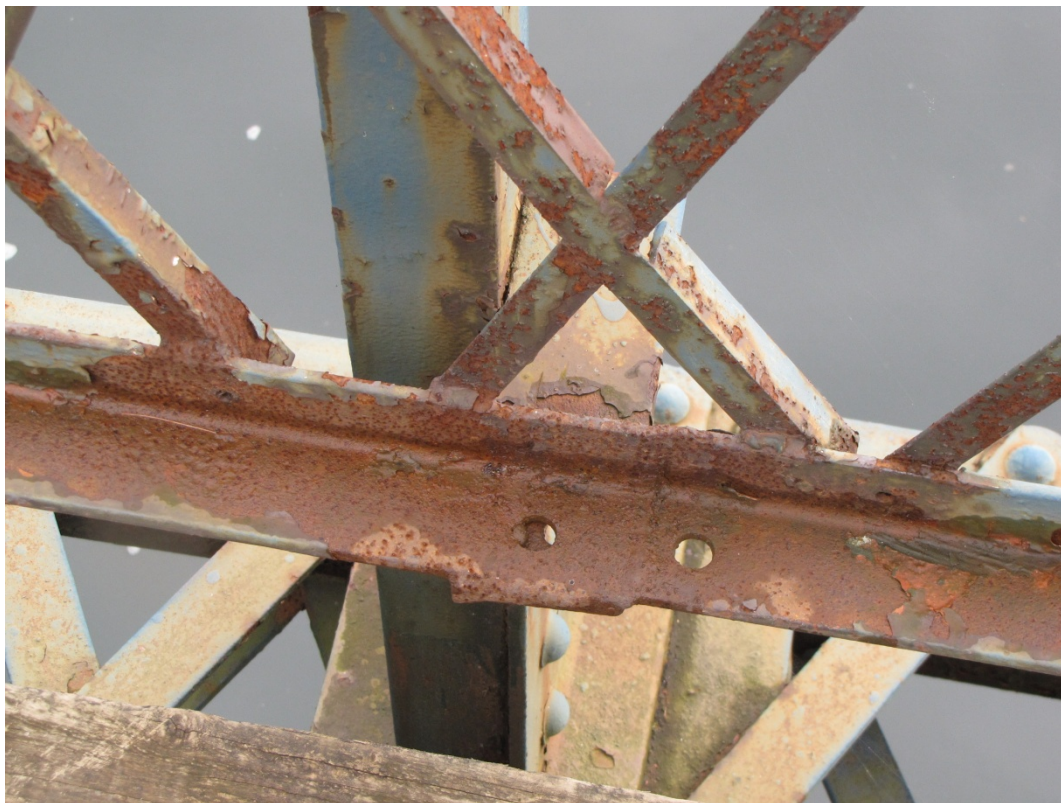
Photo S45: Missing bolt in bottom south rail between FB8 and FB9.
