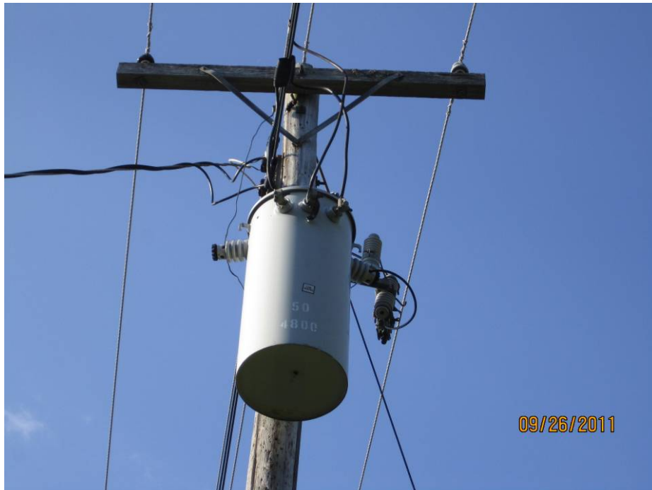
Photo E1: Existing oil filled pole mounted transformer providing 120/240V, single phase service for the bridge operating system. Note the lightning and fused cutouts used to protect the transformer installation.
