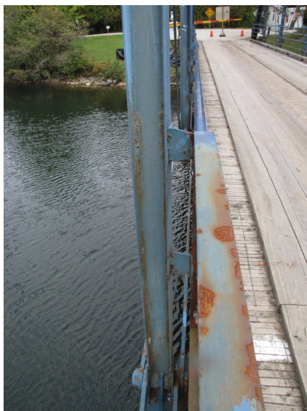
Photo F16: V1N is twisted about its longitudinal axis.
