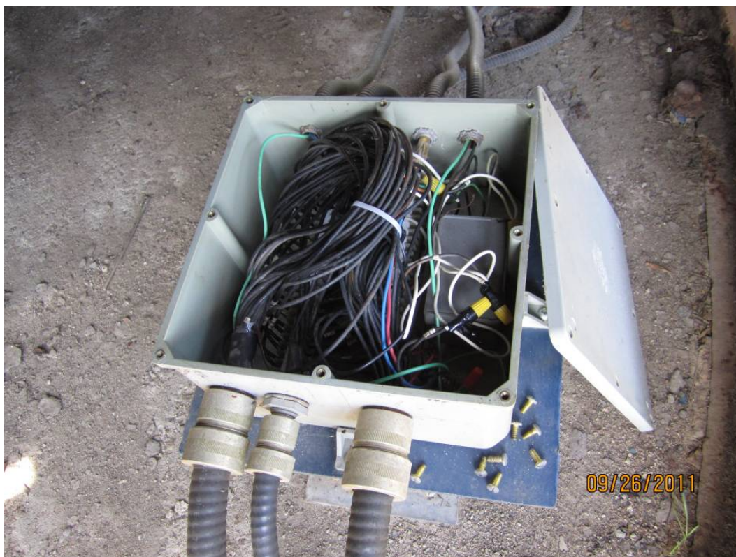
Photo E19: Center Pier Submarine Cable Junction Box. Note the poor installation of the wires.
