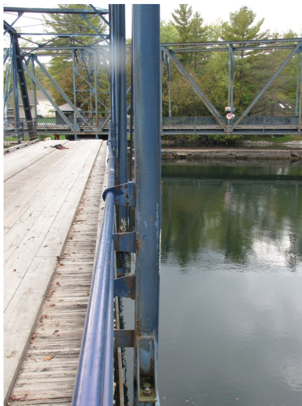
Photo F15: V6N is bent at the base.
