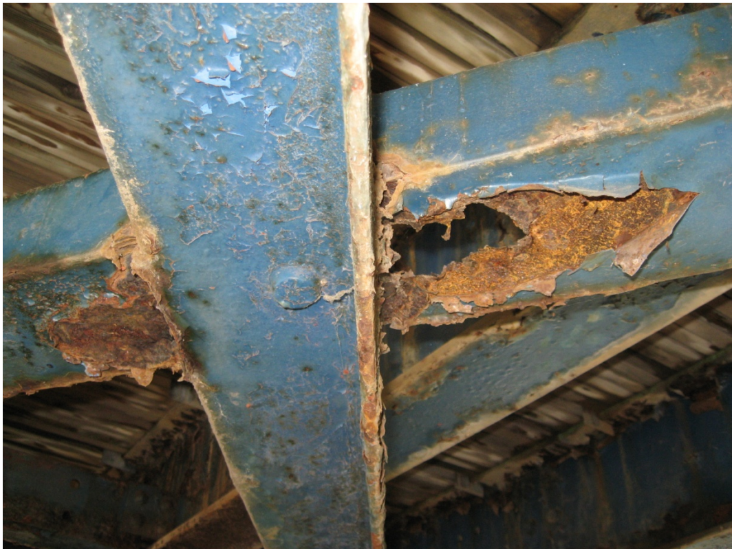
Photo S32: Bracing member 5S-6N has a long perforation in the horizontal leg.
