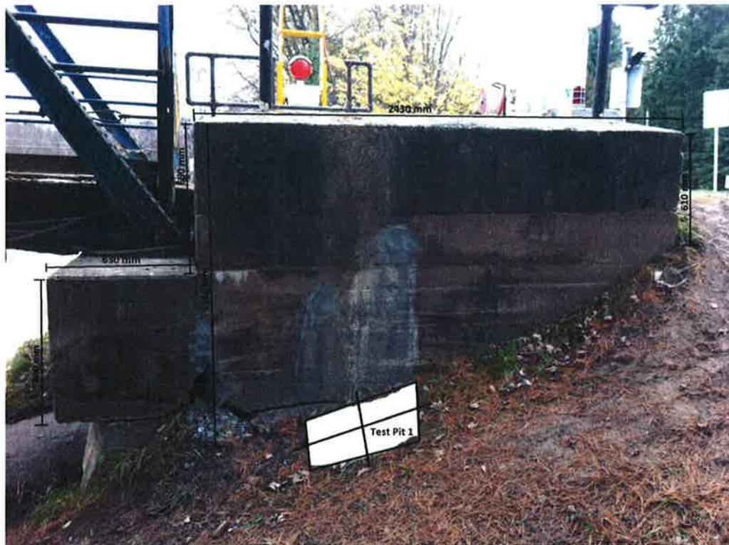
No.4: Test pit location at south side of south wing wall at east abutment and approximate measurements, looking north.
