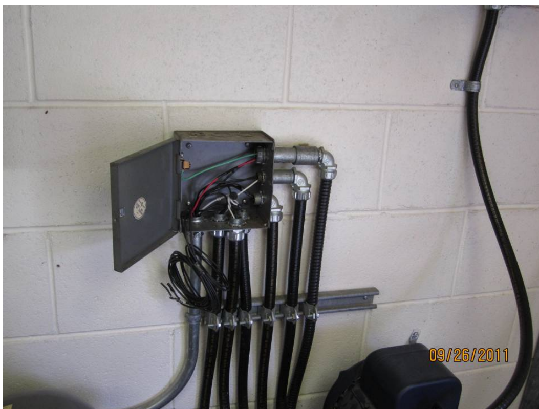
Photo E20: Typical Junction Box. Note the spare or unused wires are not properly terminated.
