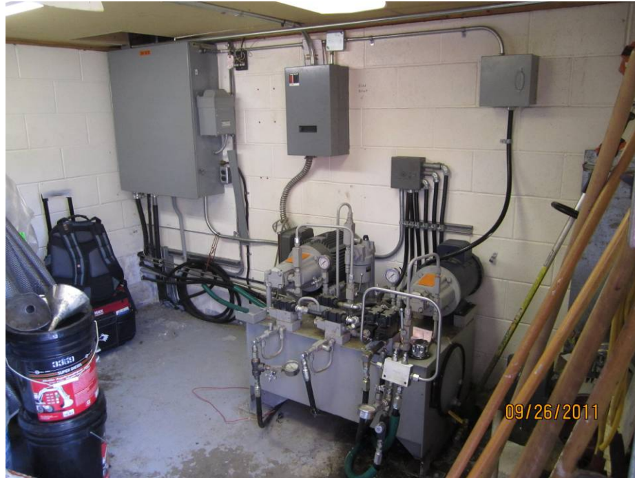
Photo E3: The swing span hydraulic pump motor, end lift / locking pin hydraulic pump motor, and solenoid valve system was replaced as part of the 1991/1992 rehabilitation and, as can be seen, is in good operational condition having been well installed and housed in the protected area of the bridge control building.
