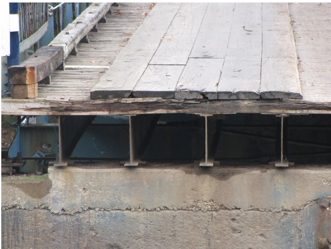
Photo F24: West end of the fixed span. Note the deteriorated timber deck member.
