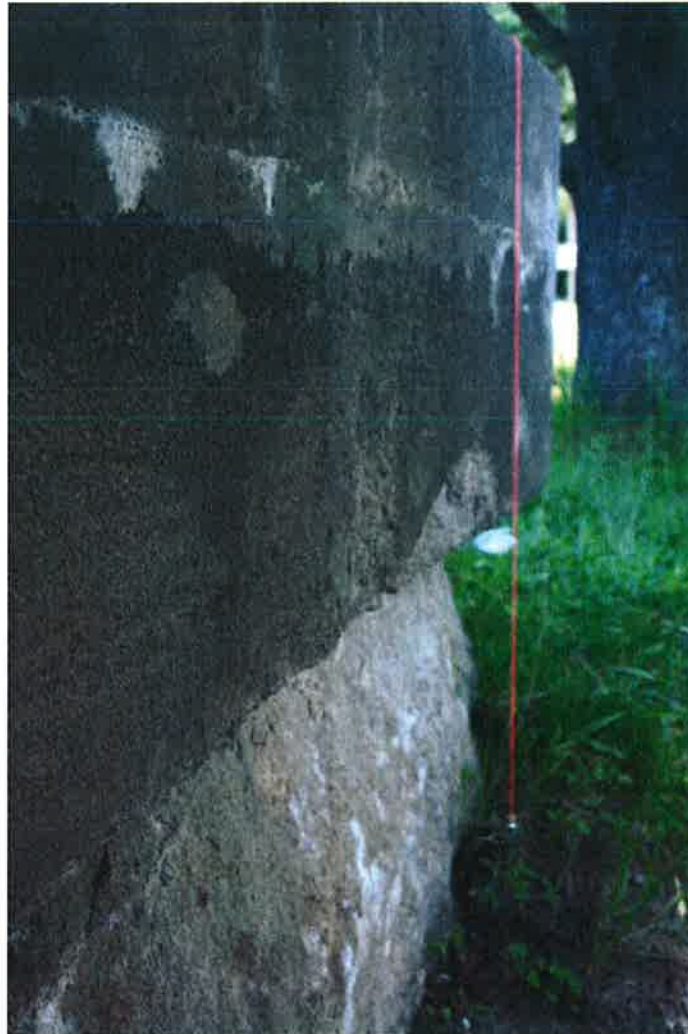
Picture 3: Note the tilting of the abutment wall and the severe concrete spalling at the lower portion of the abutment wall; a horizontal linear crack through the middle of the entire wall appears to be a construction joint.
