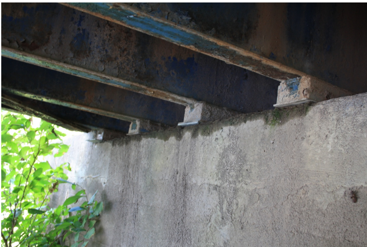
Photo F31: Stringer bearings at east end of bridge.
