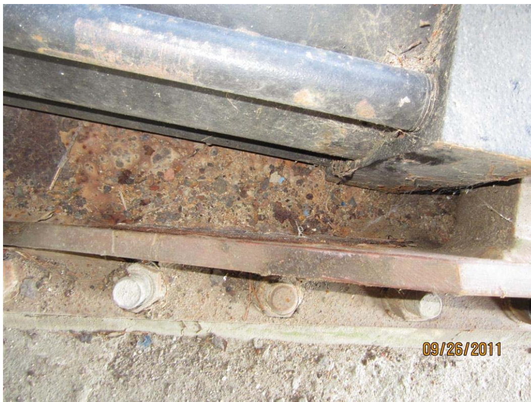
Photo M21: The blind end clevis and bracket for the span drive cylinder collects debris and exhibits light corrosion.
