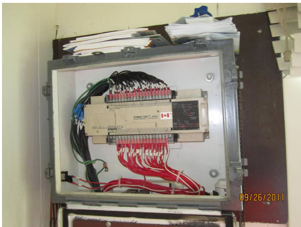
Photo E6: PLC Controller in the wall mounted enclosure. Note the PLC controller is obsolete.
