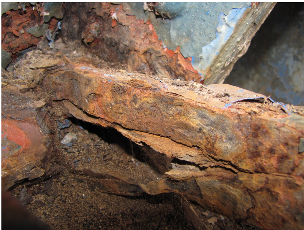
Photo F19: North bottom chord I-bar at east end of bridge has lost more than 90% of its lower cross-section.
