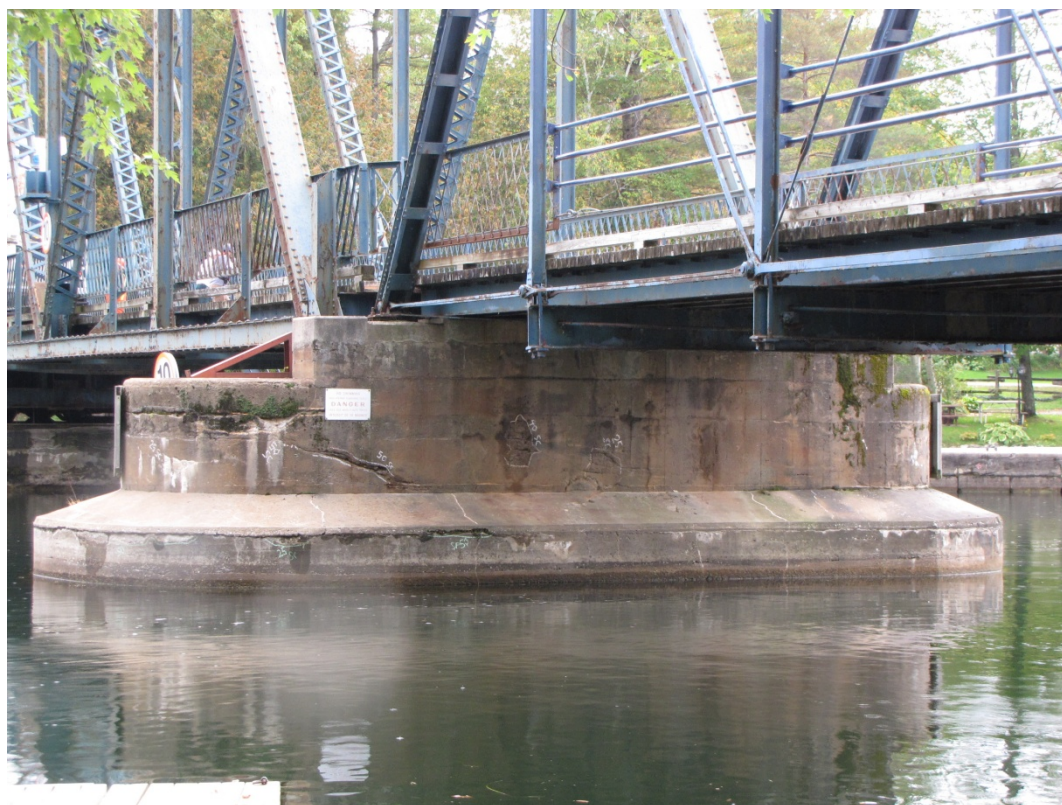
Photo F10: East face of the pier – numerous cracks, spalls and areas of disintegration noted.
