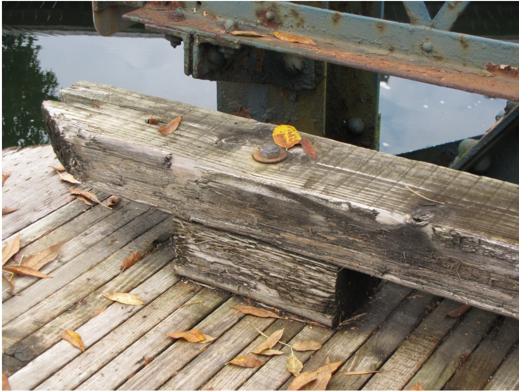
Photo S43: West end of north curb. The curb is loose and is starting to split from the west end.
