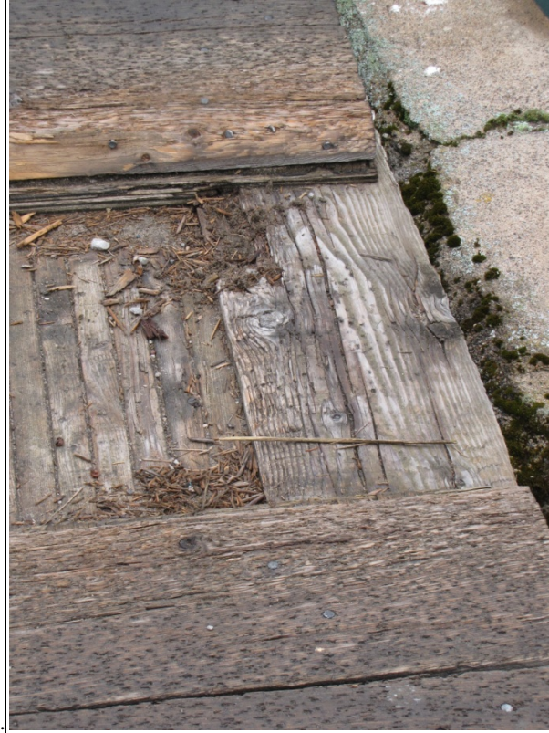
Photo S41: East end of central exposed section of deck. The end deck member is rotten and splitting. The plywood shims beneath the wearing surface members are also rotten.
