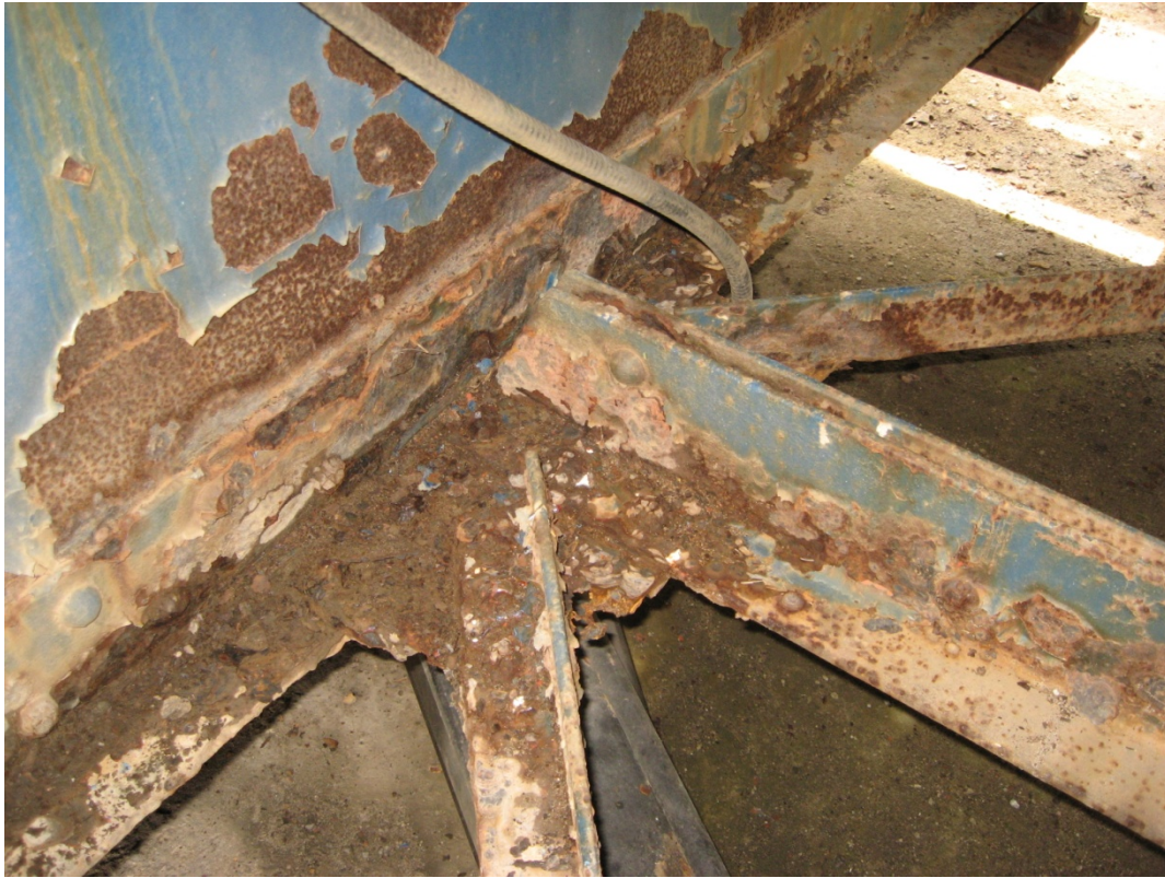
Photo S37: The steel members in the central pivot area typically have severe section loss, including perforations in gusset plates.
