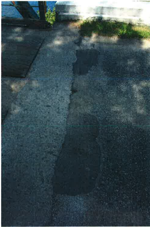
Picture 5: Note the voids/gaps developed behind the abutment wall (i.e. patched area).
