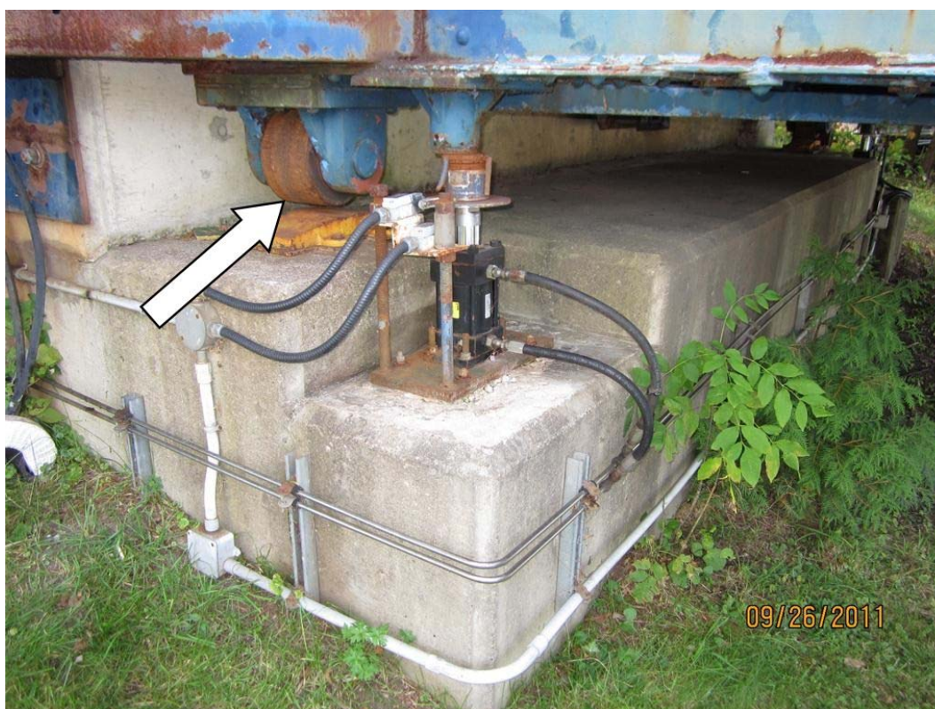
Photo M8: The west end castors are no longer utilized to support the swing span. The end lift cylinder body, base plates, and anchor bolts exhibit light corrosion.
