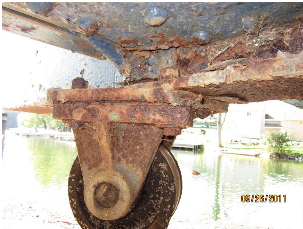
Photo M6: The balance wheel assembly and mounting bolts exhibit moderate corrosion and light section loss.
