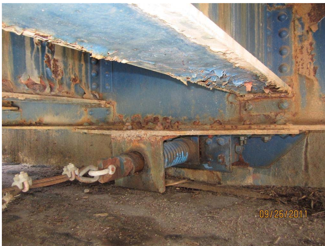
Photo M12: General view of the east locking pin.
