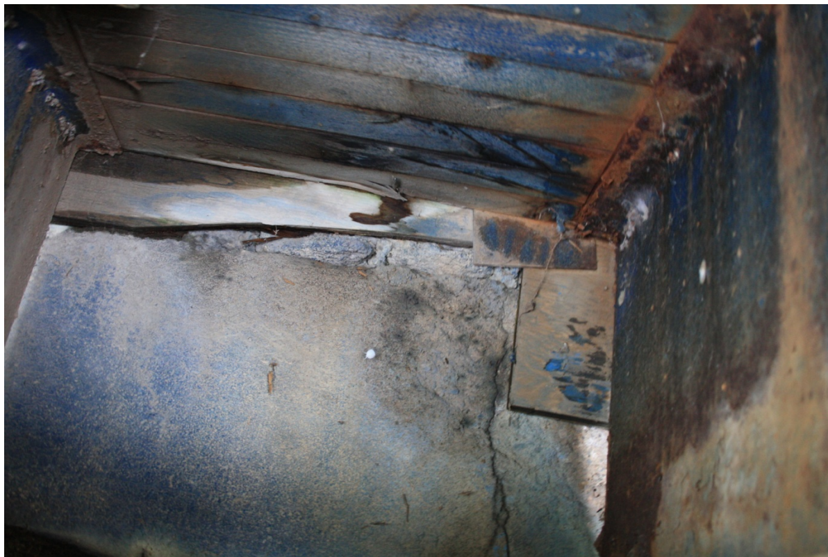
Photo F9: The east ballast wall has several vertical cracks.
