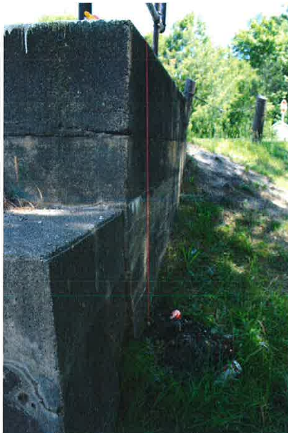
Picture 4: Note the tilting of the southeast wing wall; the linear crack at the ground surface level appears to be a construction joint.
