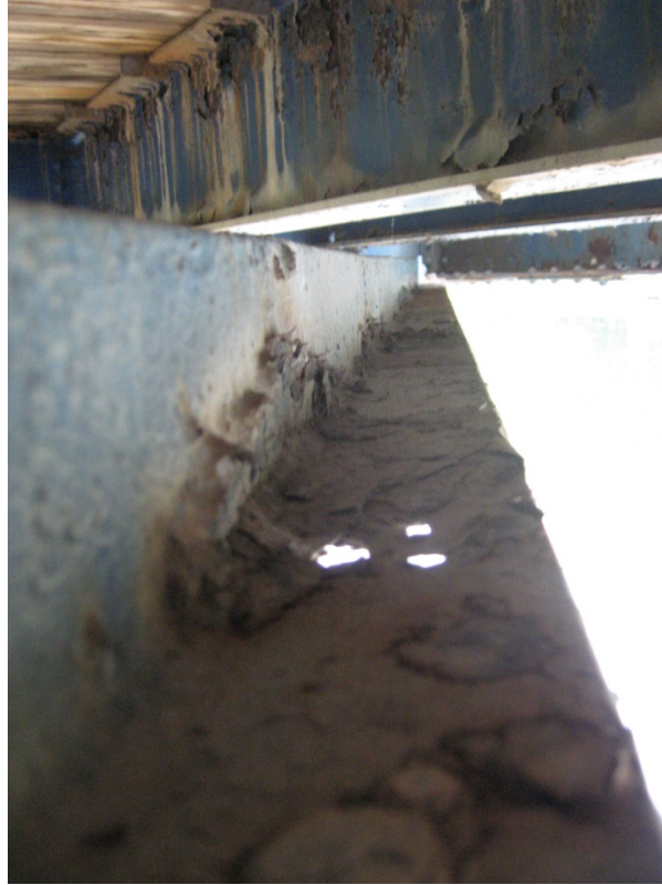
Photo S31: The south-east section of bracing member 6N-7S has severe pitting and three small perforations.
