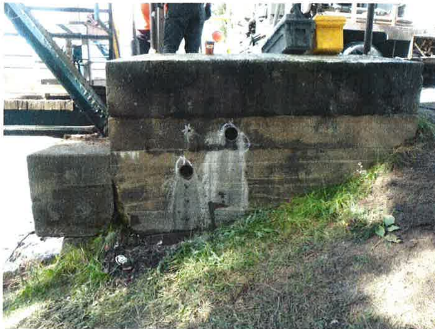
Figure 4-4 Overview of southeast wingwall facing north. Note the location of cores C3 (lower) and C4 (upper).
