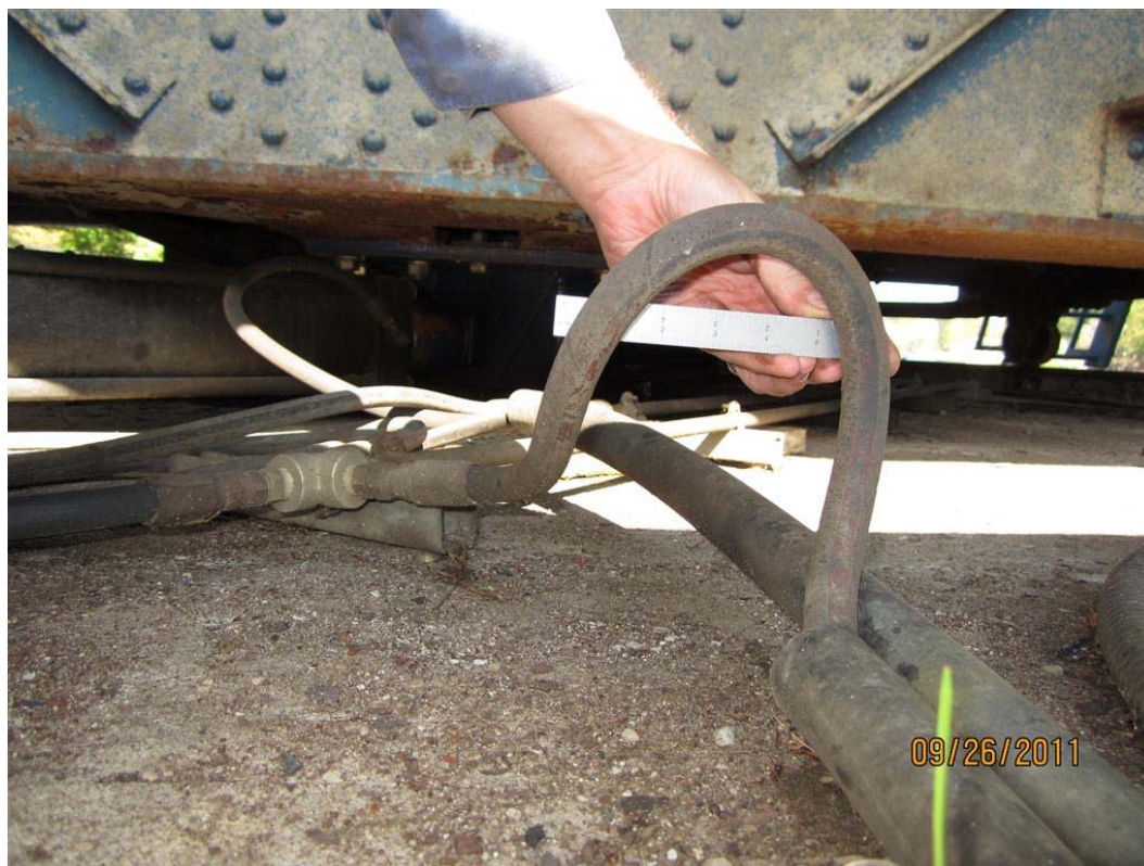
Photo M19: The blind end flexible hose connecting the HPU to the piping at the pier exhibits a severe bend radius (less than 120 mm radius).
