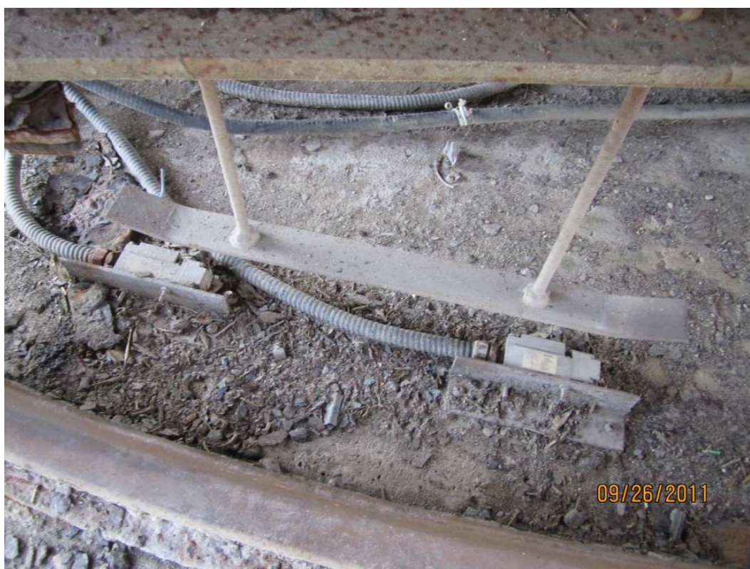
Photo E12: Typical Bridge Drive System Control Limit Switches. Note the debris on and around the limit switches.
