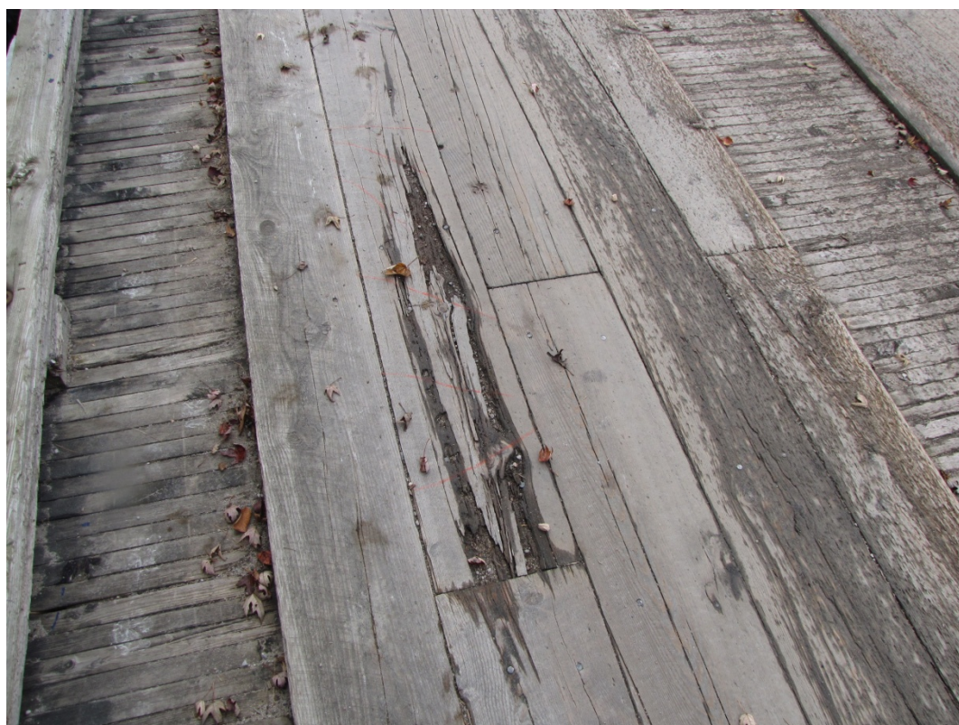
Photo F26: Typical area of rotting and checking in the timber wearing surface.
