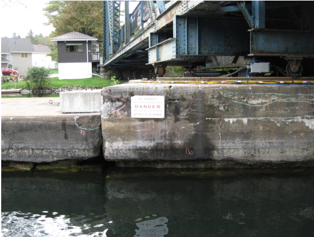
Photo S17: South-east corner of the central swing pier. Very severe erosion of the walls at the waterline.
