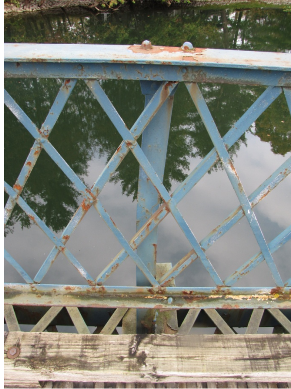
Photo S47: The north railing post between FB3 and FB4 is bent.
