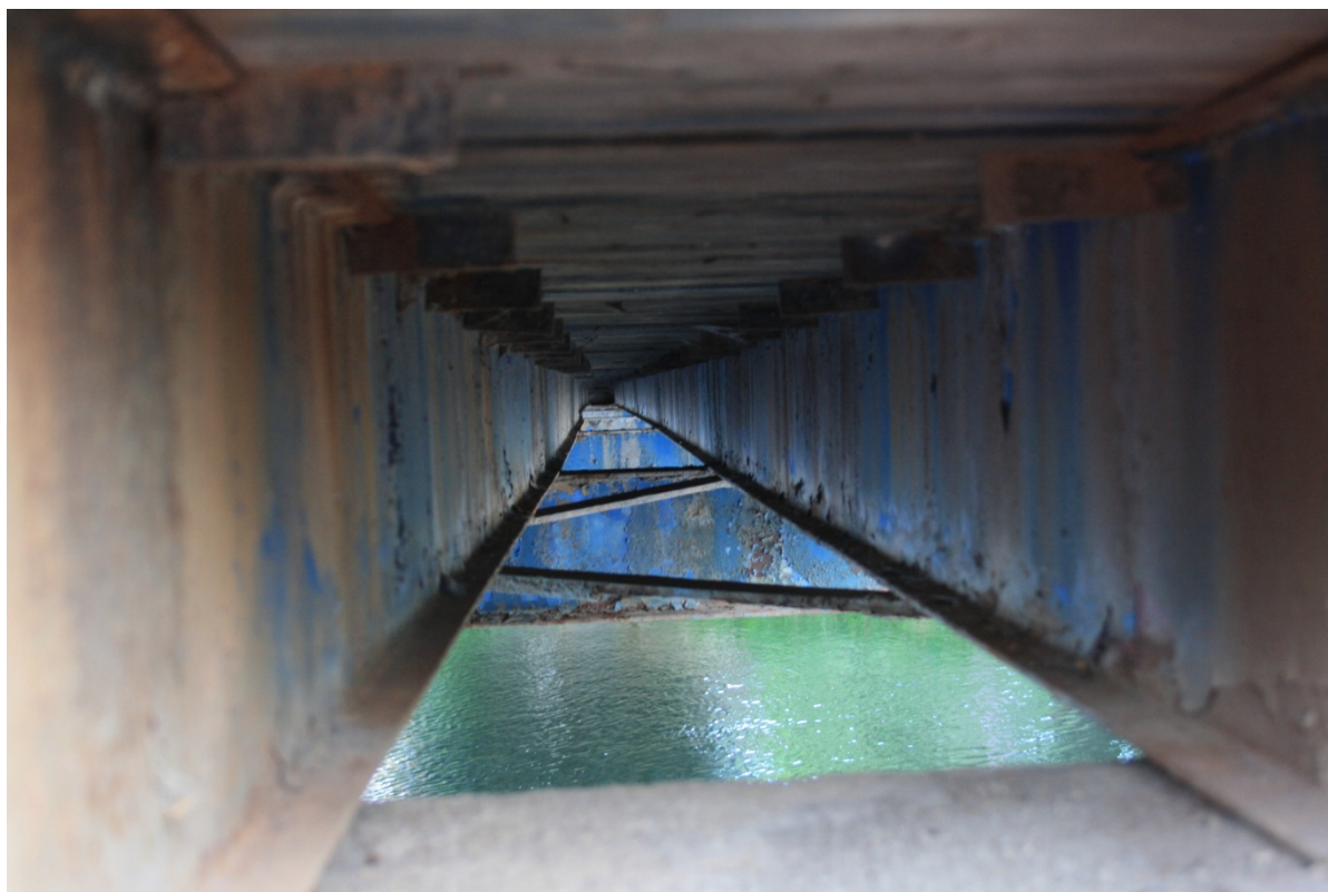
Photo F25: Looking east along the stringers. Some stringer out-of-straightness observed.
