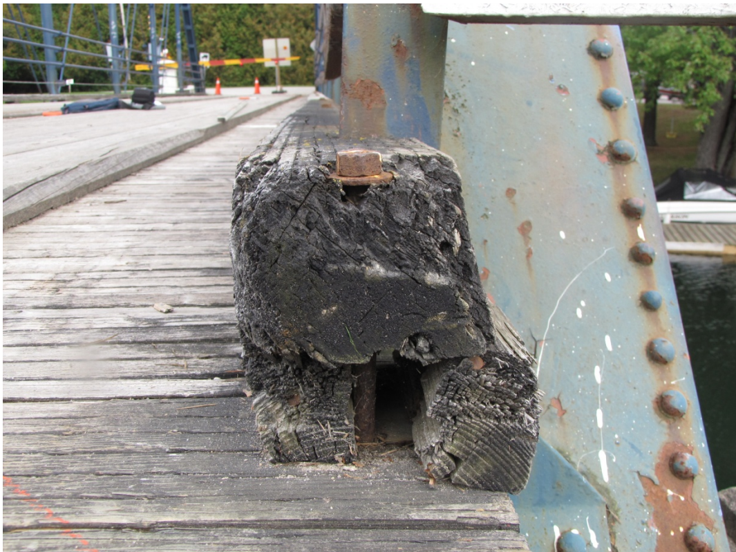
Photo F28: The block beneath the west end of the south curb has split into two pieces.
