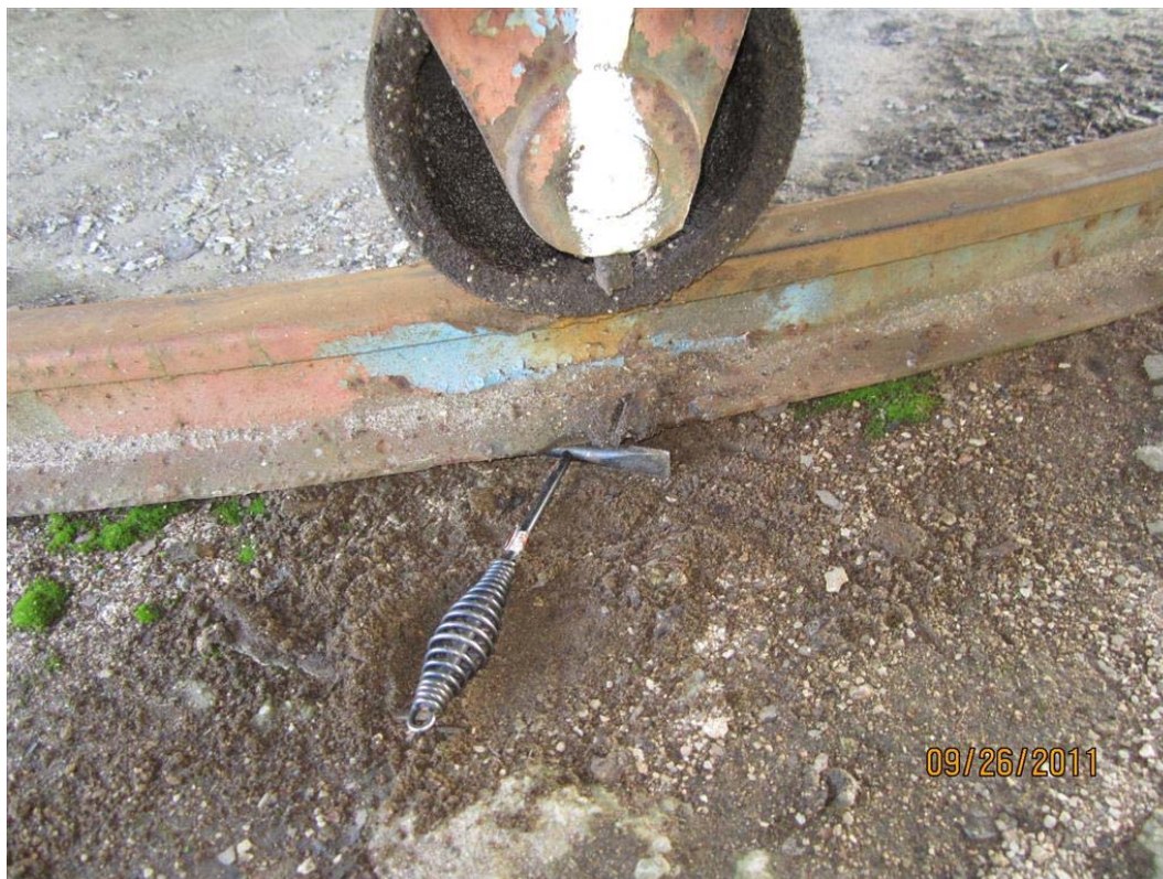
Photo M5: The rail support pier is undermined along a significant portion of the rail.
