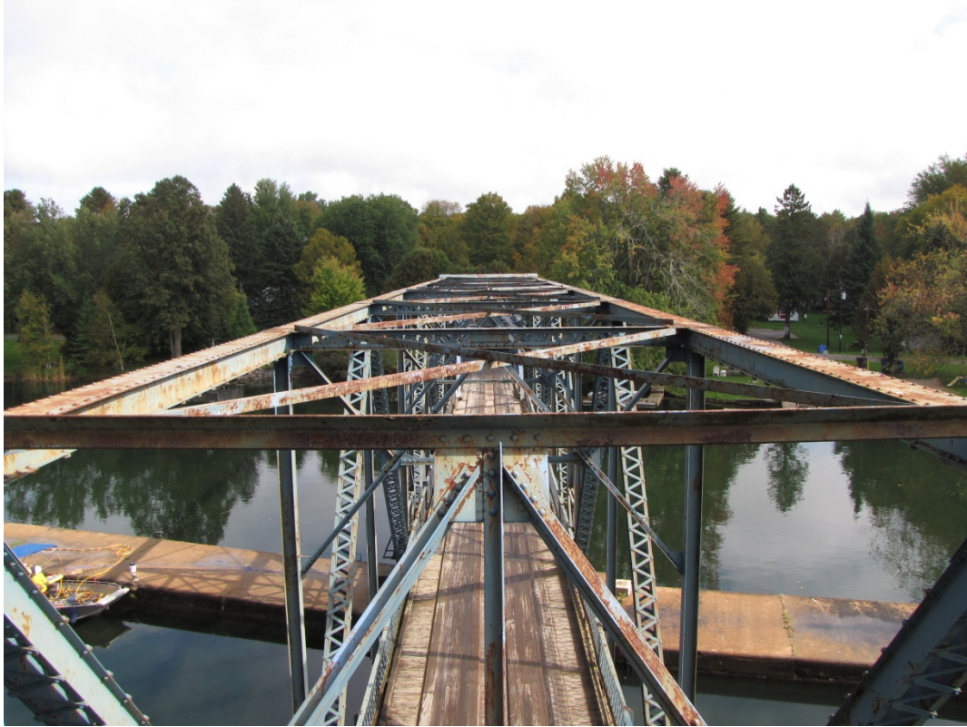
Photo S21: Looking east. The truss and bracing members typically have extensive areas of coating failure and light corrosion.
