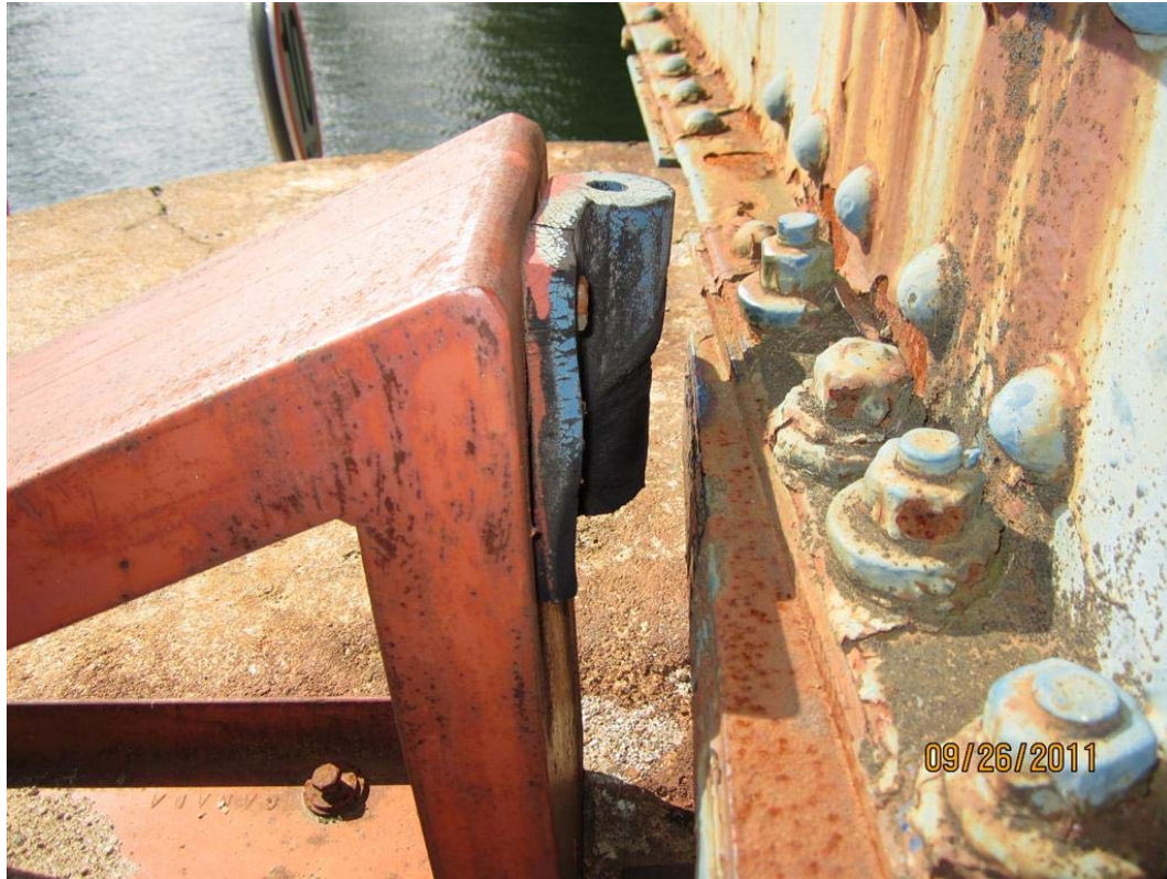
Photo M13: The east end of travel stop is installed with an energy absorbing pad that is in poor condition.
