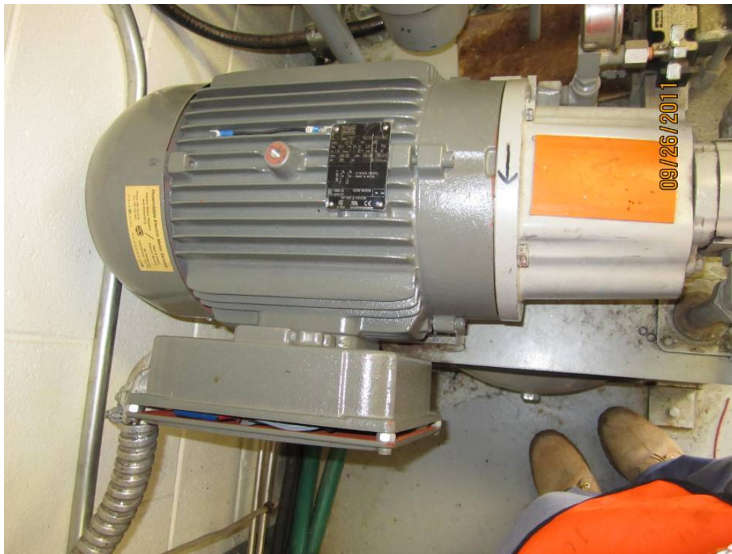
Photo E4: Swing Span Hydraulic Pump Motor. Note the gap in the motor power junction box.
