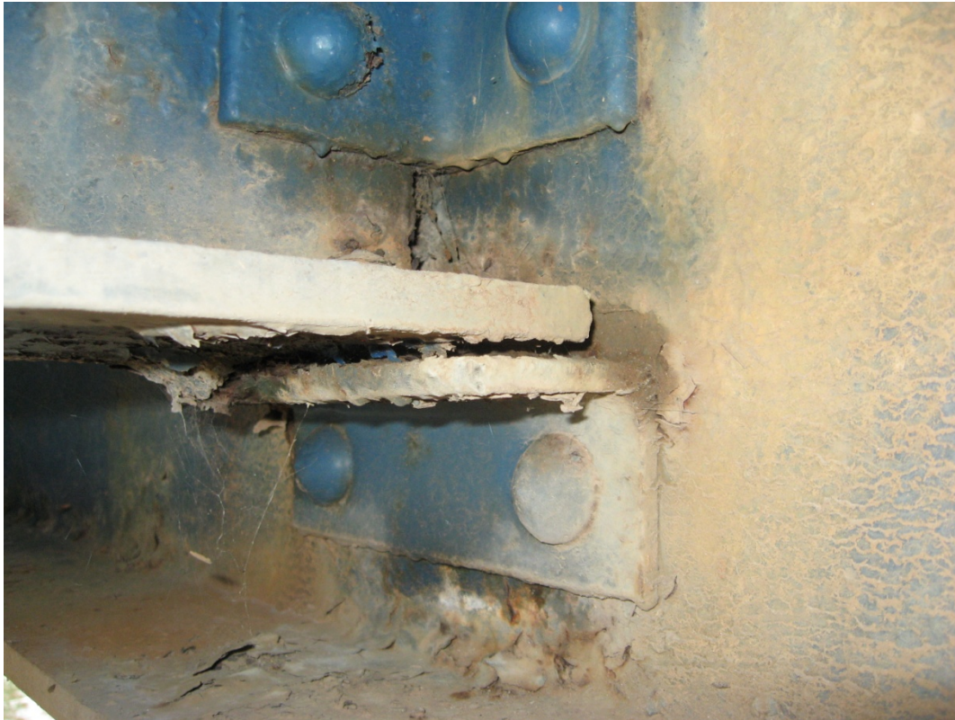
Photo S29: Typical gap between the supporting angle and the stringer bottom flange.
