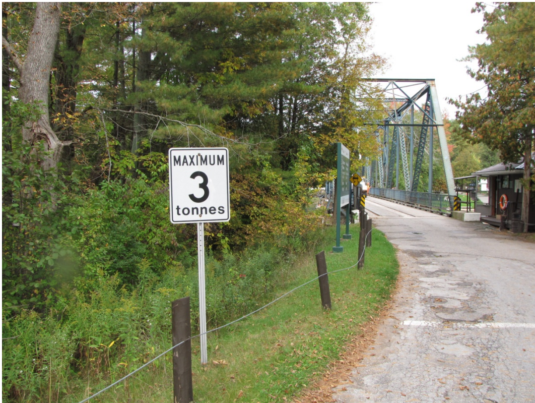
Photo S48: The steel cable in the north-west approach guide rail has tension loss.
