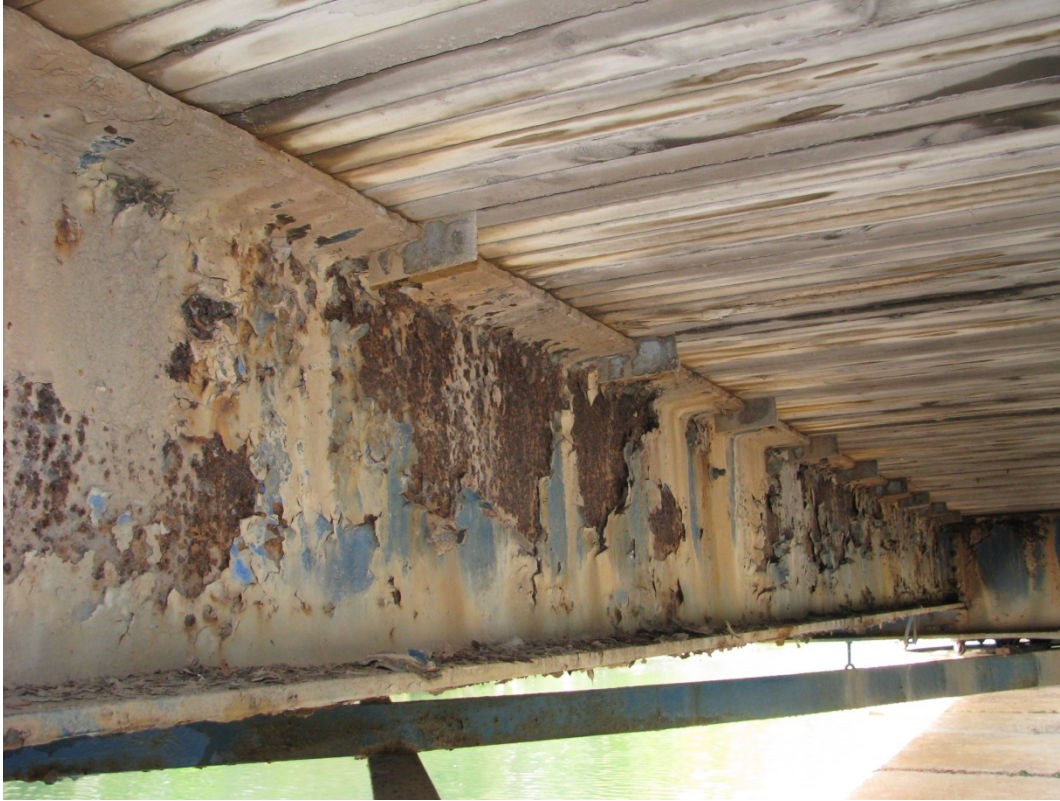
Photo S27: South side of stringer S0-3 between F0 and FB1. Typical condition of stringers with coating loss and light to medium corrosion.
