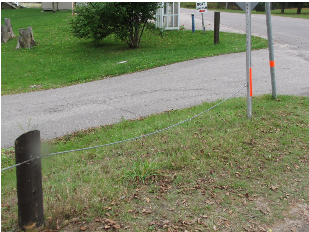
Photo S50: The west end of the steel cable of the south-west guiderail is attached to a road sign post.
