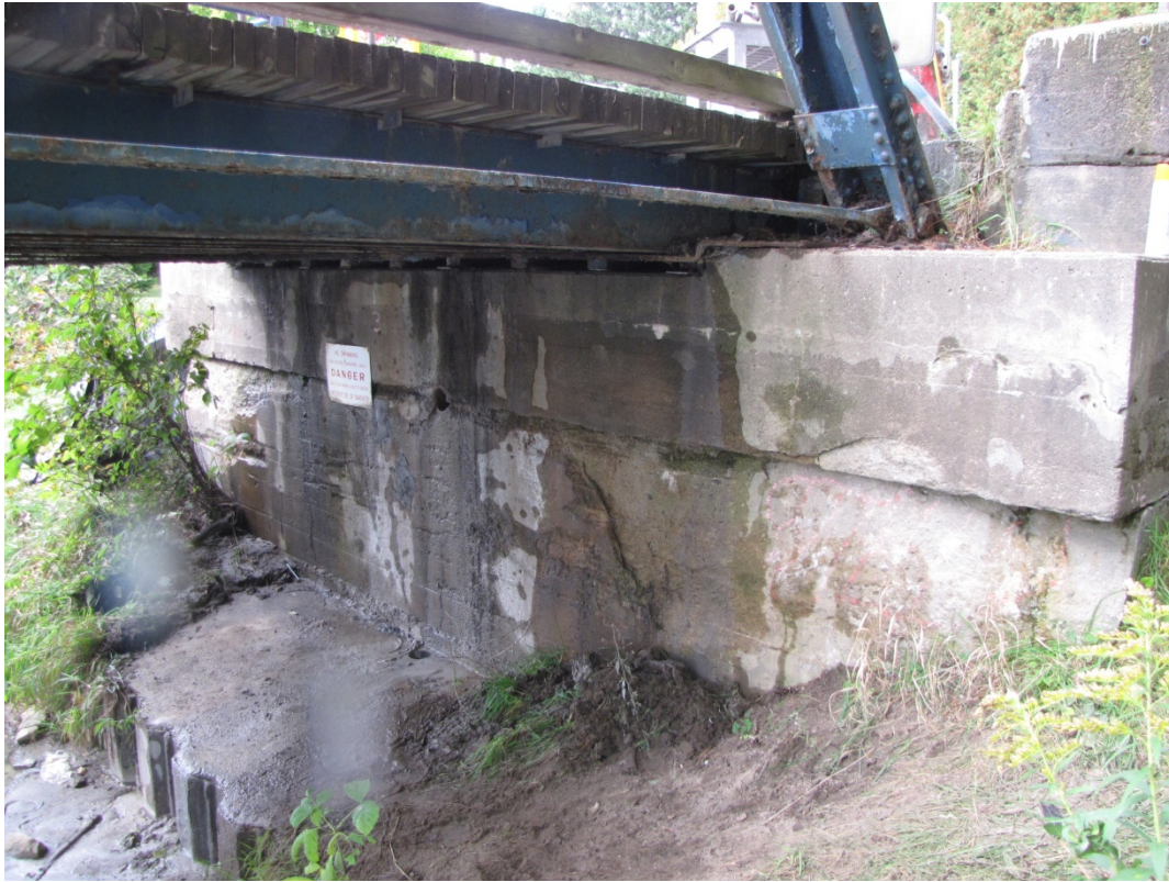
Photo F7: East abutment exhibits large areas of spalling and severe scaling. The wall is leaning to the west.
