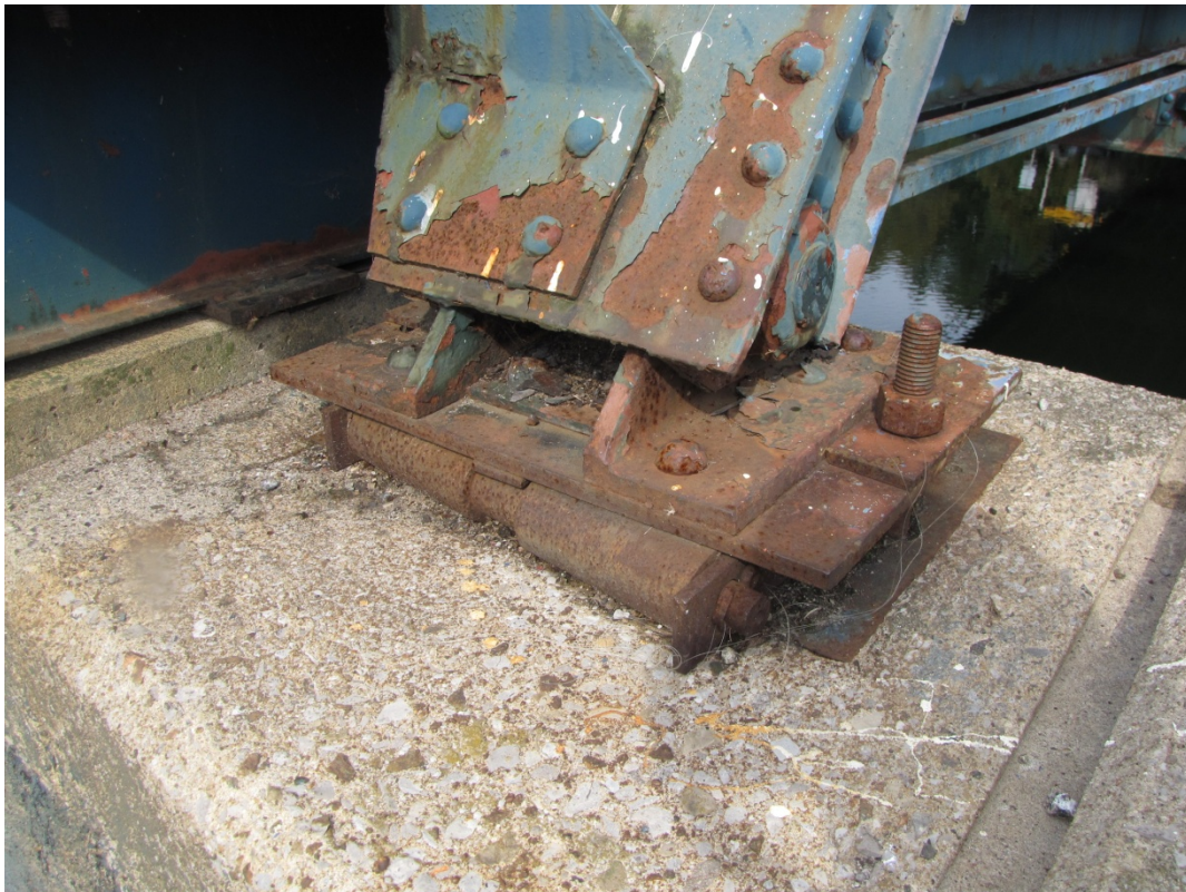
Photo F29: South-west bearing – the roller has twisted diagonally and is partially off the steel bearing plate.
