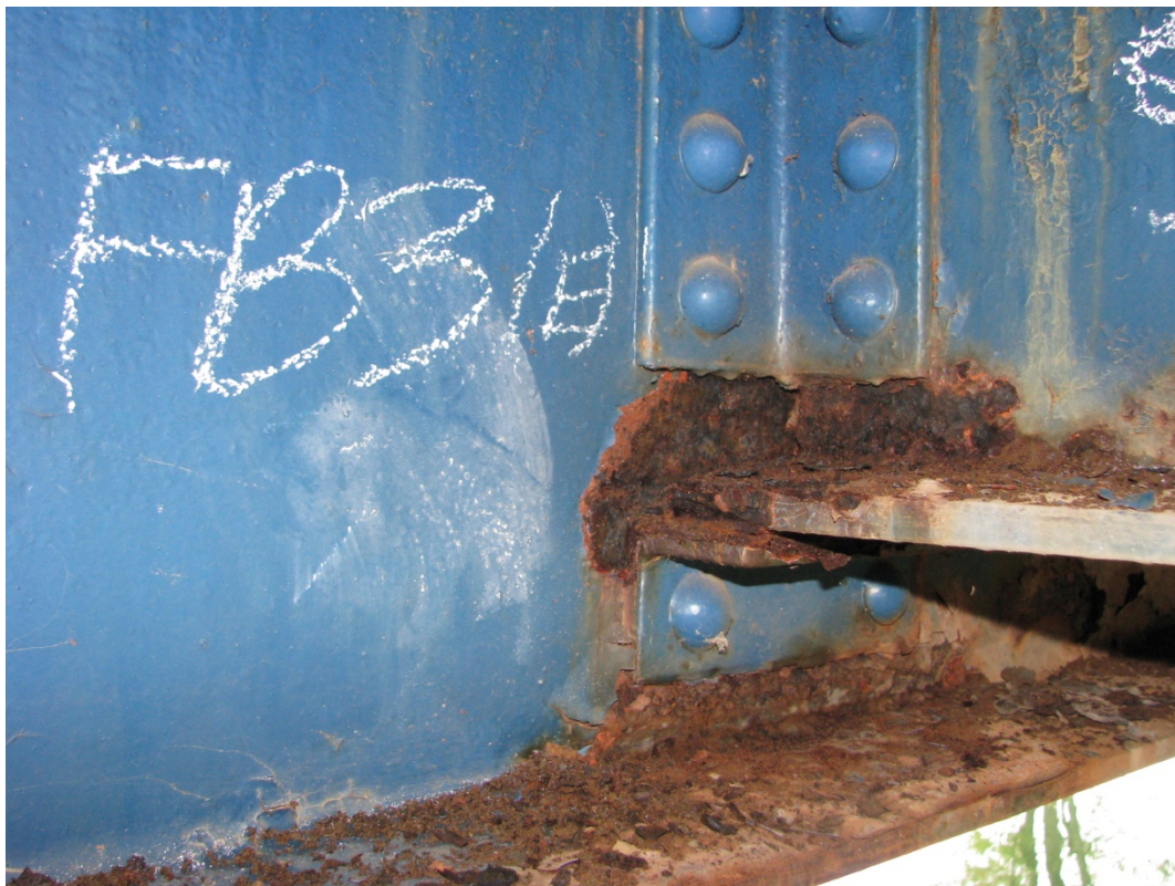
Photo S30: The east side of the web of FB3 has severe localized section loss at the connection with stringer S3-2.
