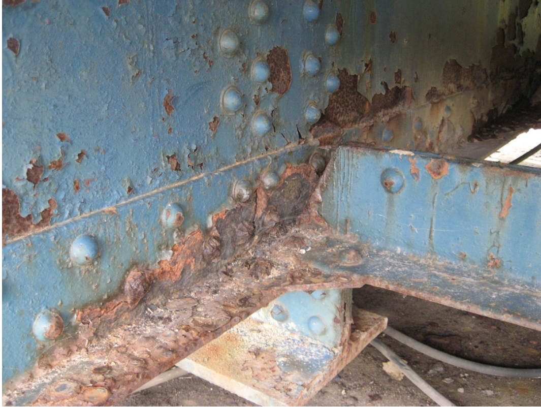
Photo S39: Typical severe section loss of pivot girder bottom flange.
