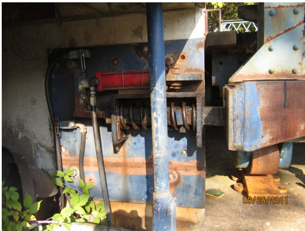
Photo E11: West Locking Pin. Note the corrosion on the mounting plate.
