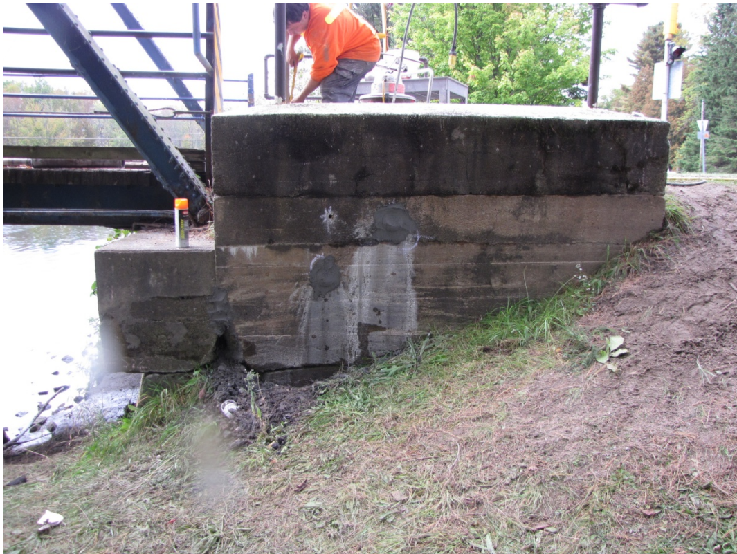
Photo F6: The south-east wingwall has wide gaps at the construction joints plus areas of spalling and disintegration. The wall is leaning to the south.
