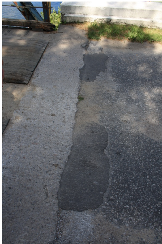
Photo F8: Asphalt patch repairs in the east approach.
