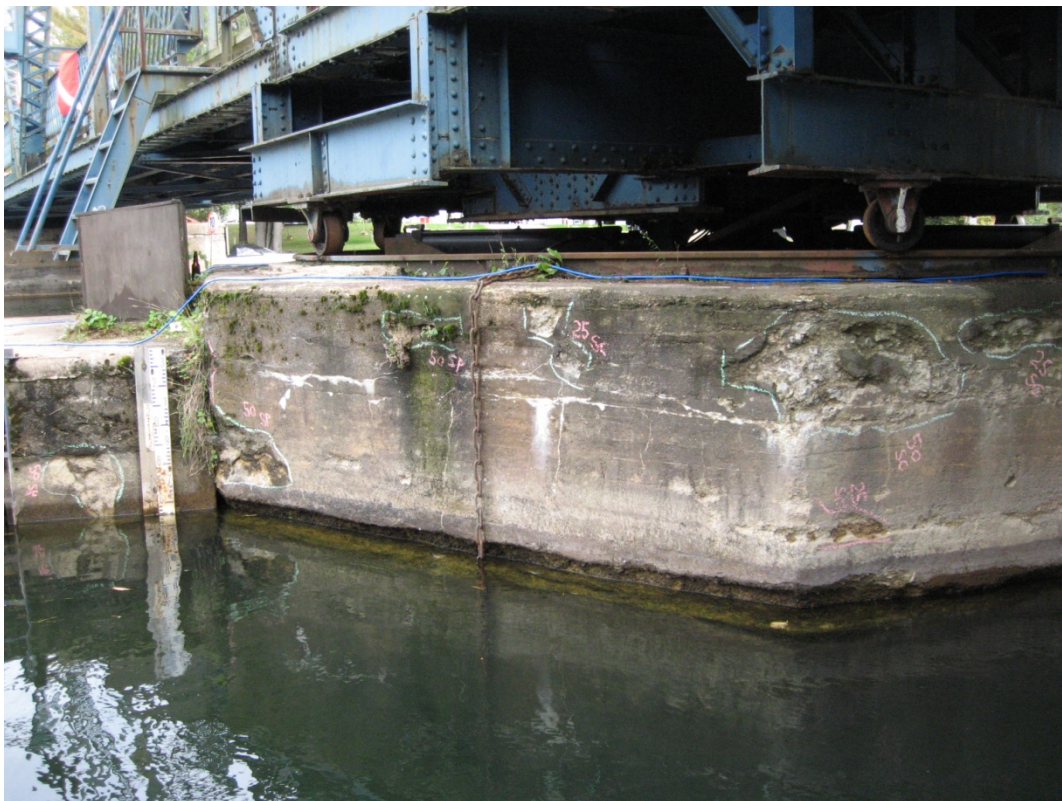
Photo S18: North-west corner of the central swing pier. Very severe erosion of the walls at the waterline, and several large areas of disintegration.
