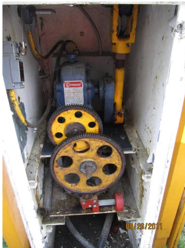
Photo E16: Typical Traffic Gate Equipment. Note the gate is provided with raised and lowered limit switch but no hand crank limit or door switches are provided.
