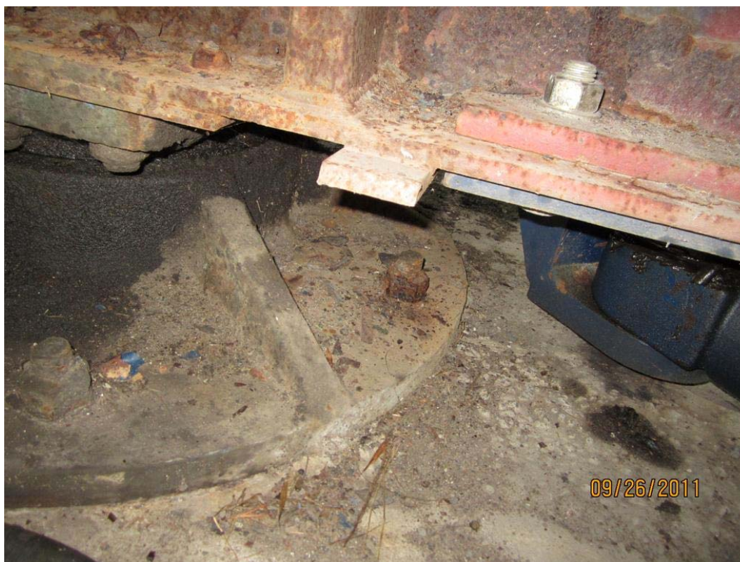
Photo M2: One of six anchor bolts exhibits corrosion and light section loss.
