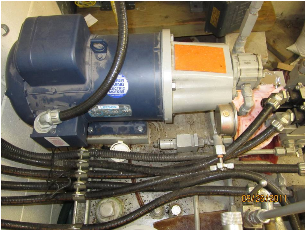
Photo E9: End Lift / Locking Pin Hydraulic Pump Motor. Note the as new condition of the motor.
