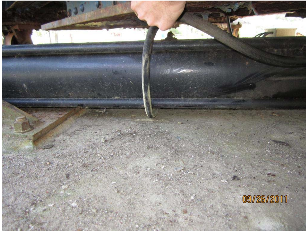
Photo M17: The flexible hoses that connect the span drive cylinders to the hard piping are abraded.
