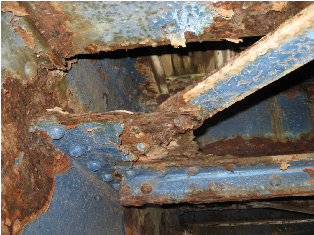
Photo S38: The steel members in the central pivot area typically have severe section loss, including perforations in gusset plates.
