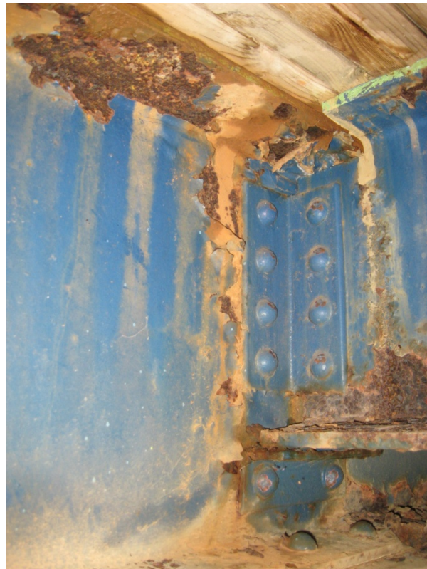
Photo S28: Typical light to medium corrosion of floor beams and stringers at floor system connections.
