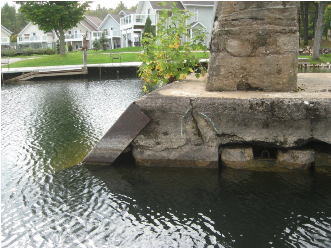
Photo S14: South-east corner of the rest pier. Typical wide cracks and large spalled areas in the concrete cap and blocks. Note the void beneath the steel plates.
