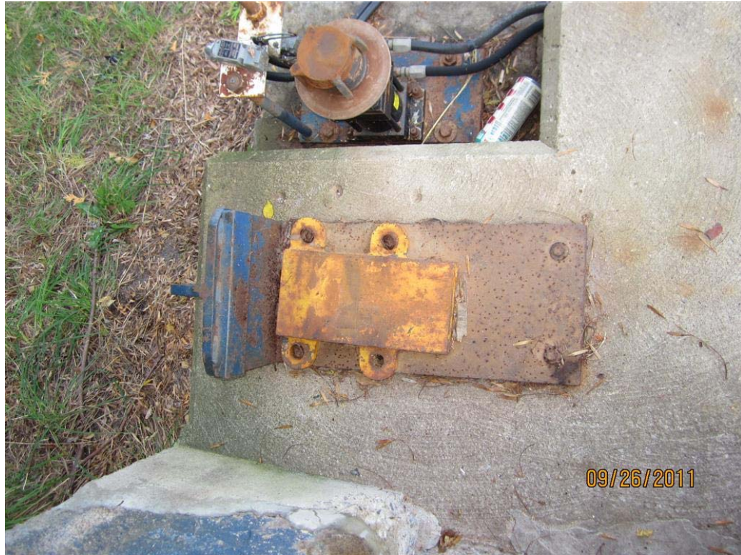
Photo M15: West end of travel stop. The rest plate anchor bolt heads are cut off and do not secure the rest plate to the pier.
