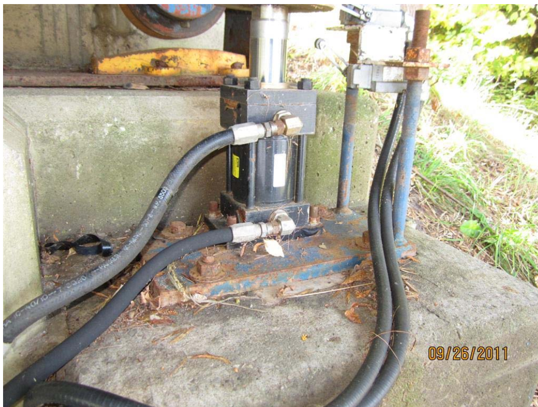
Photo M9: North End Lift. The base plate anchor bolts are not properly tightened.
