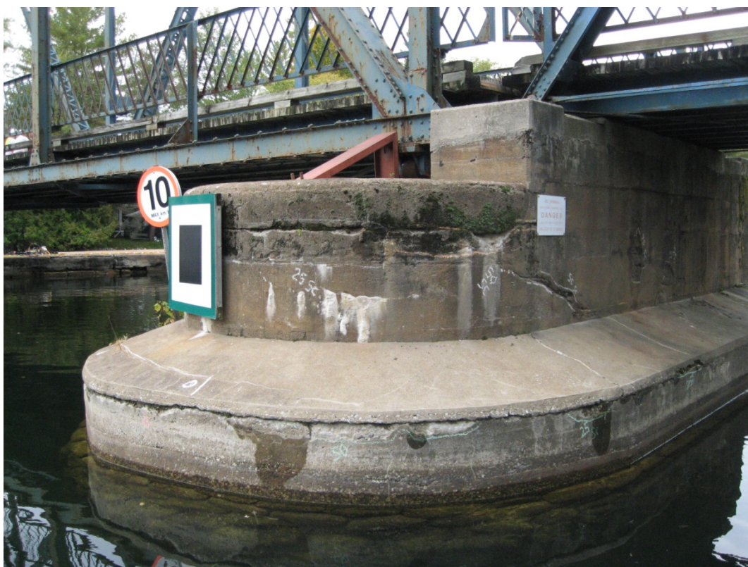
Photo F11: Typical very wide cracks, efflorescence and spalls in the south end of the pier.
