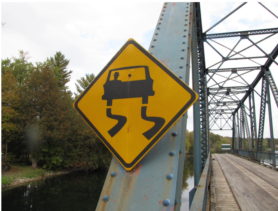
Photo S51: The sign on the west end of the north truss is missing a bolt.
