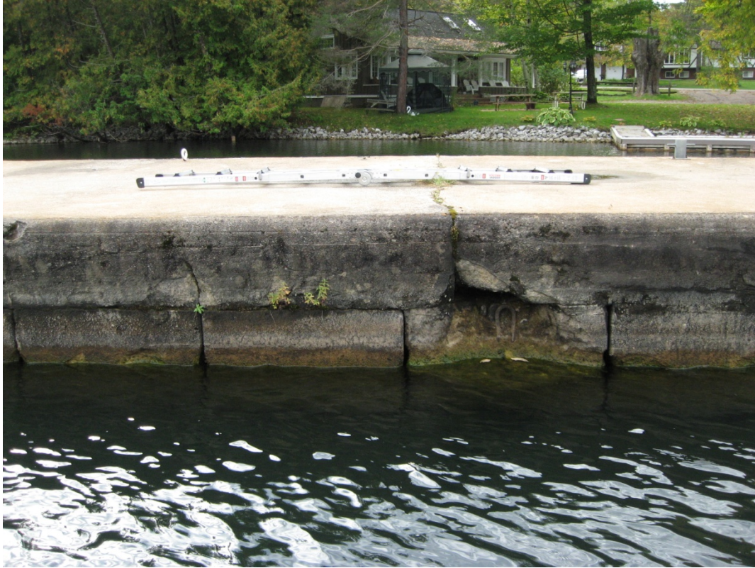
Photo S13: East side of the south section of the rest pier. Typical wide cracks and large spalled areas in the concrete cap and blocks.
