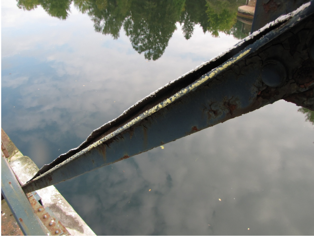
Photo S35: The top layers of steel of the bottom section of vertical bracing between V4S and V5S have delaminated.
