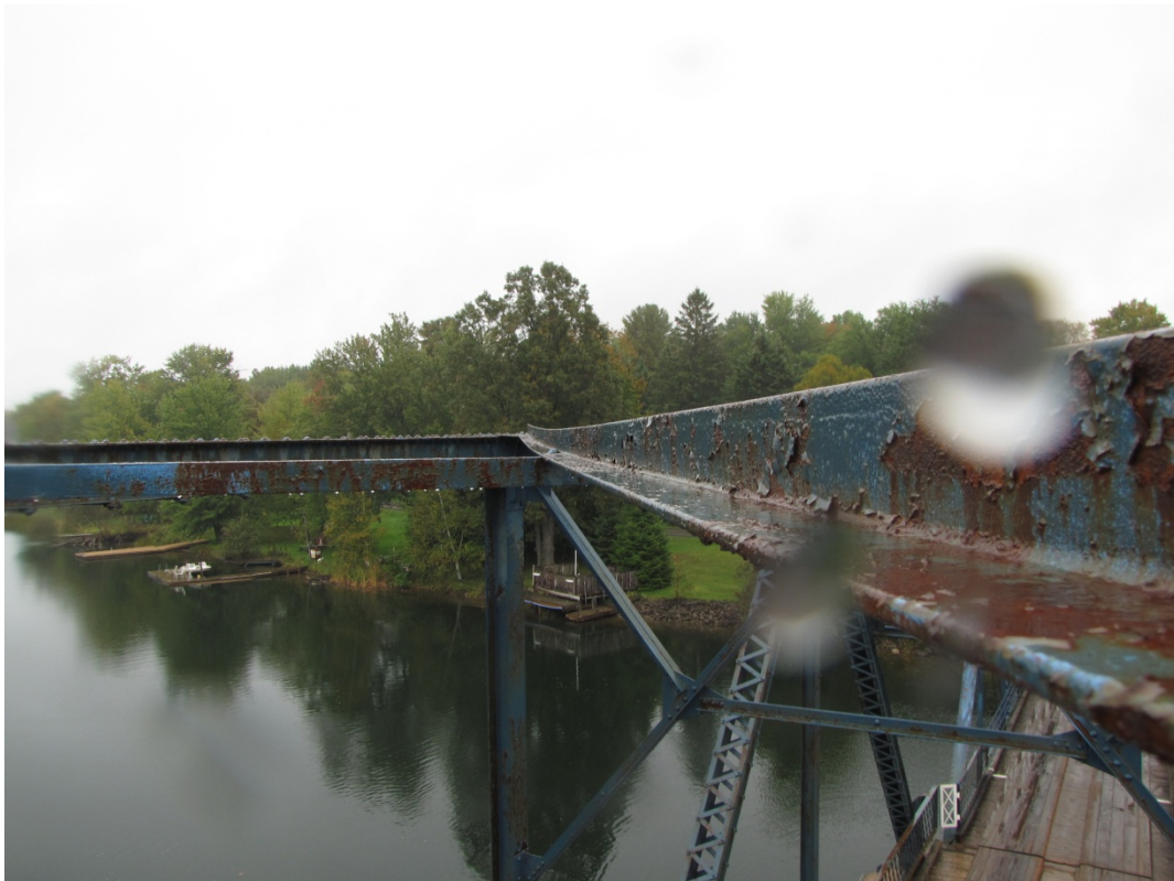
Photo S24: The upper lateral bracing members are typically bent.
