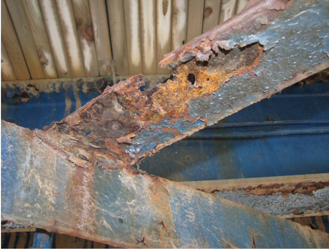
Photo S33: Very severe section loss and 75 mm x 50 mm perforation in bracing member 2N-3S.
