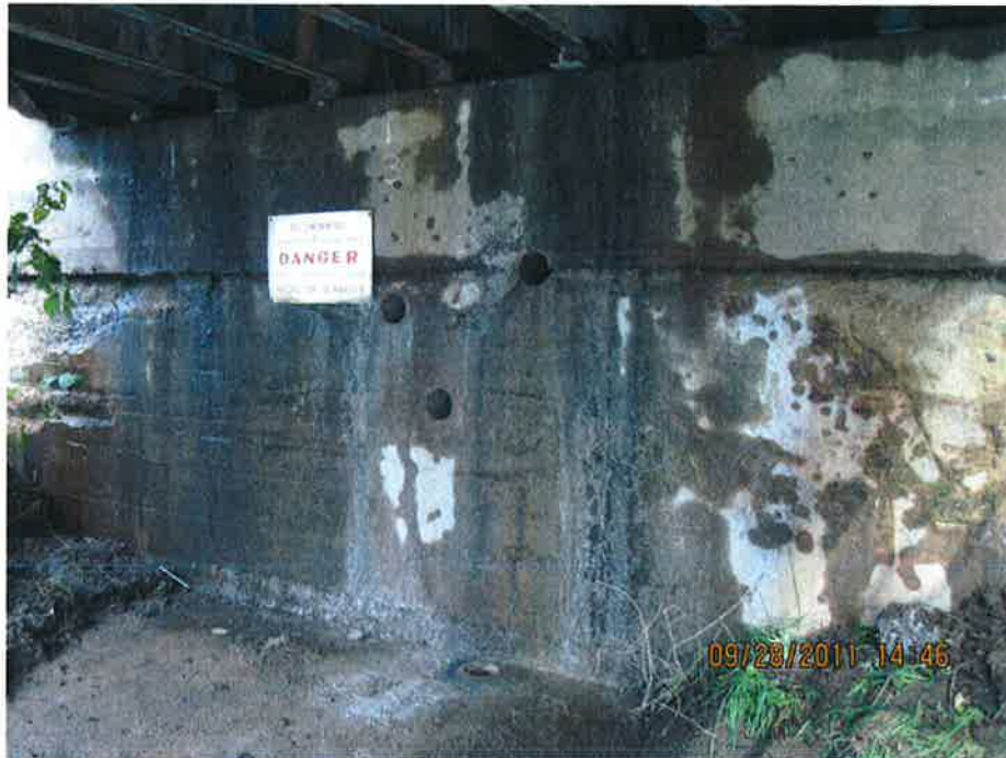
No.7: The north abutment concrete wall under the bridge; the linear crack appears to be the construction joint.
