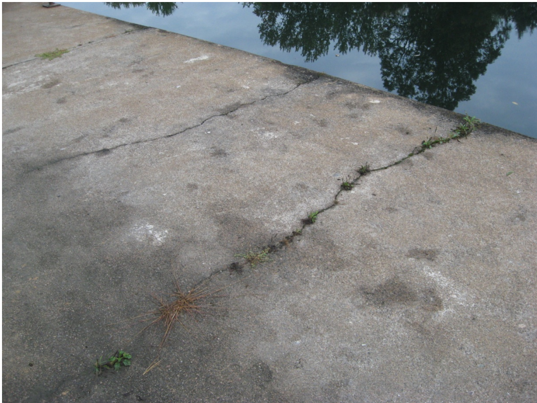
Photo S12: Typical wide transverse cracks in the top of the rest pier concrete cap.
