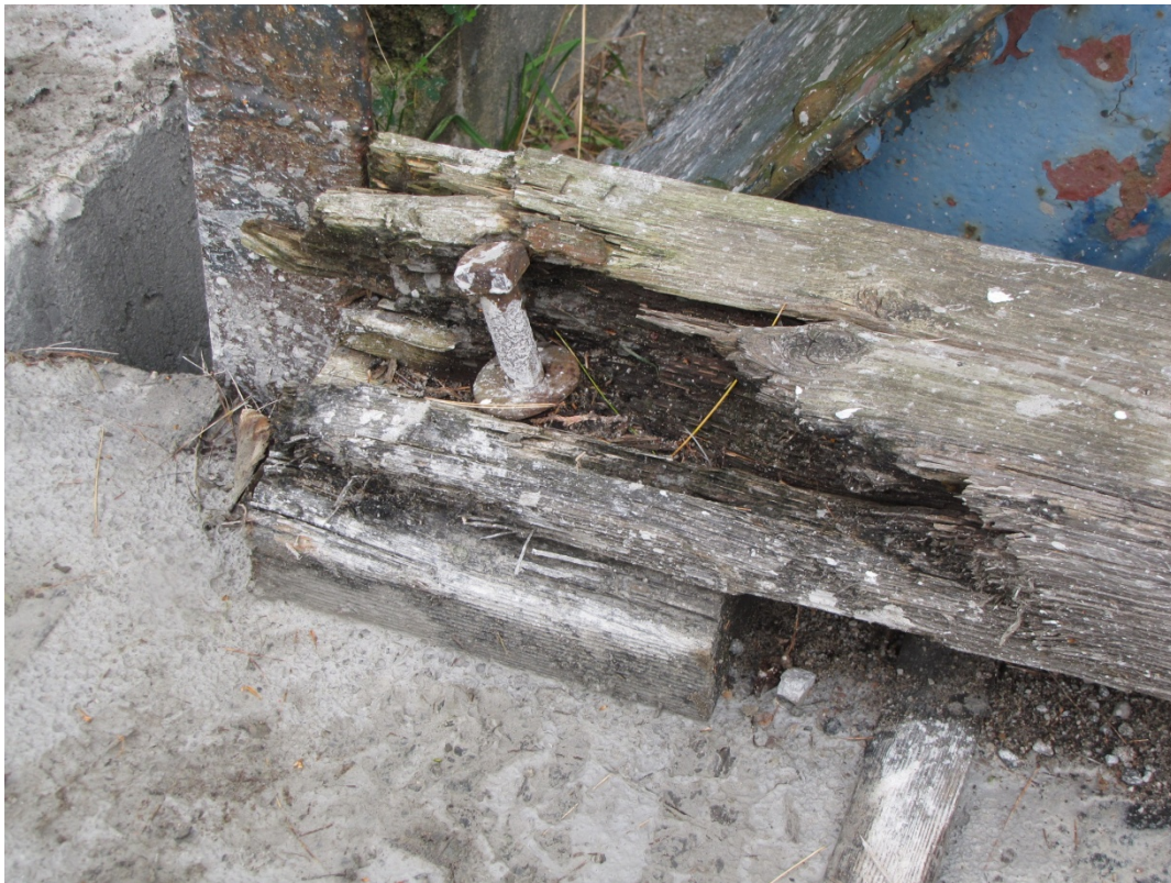
Photo F27: Severe rotting of the east end of the south curb.
