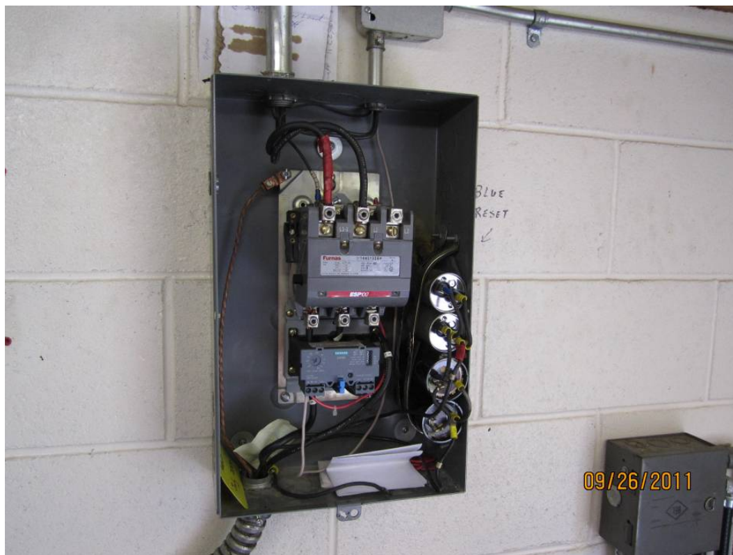
Photo E5: Swing Span Hydraulic Pump Motor Starter. Note the as new condition of the starter (Replaced in 2009).
