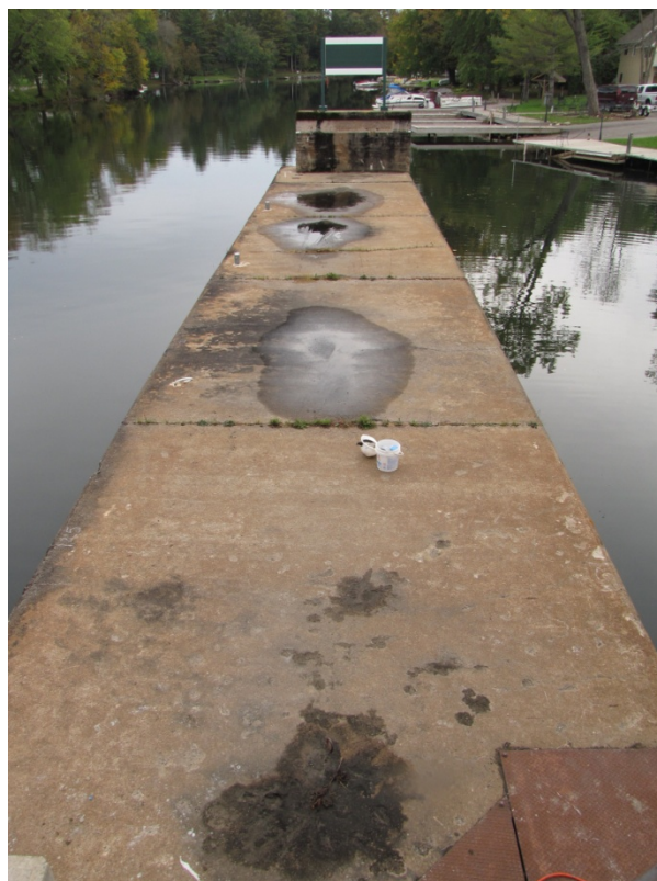
Photo S10: Top of the south section of the rest pier. Note the areas of ponding water.
