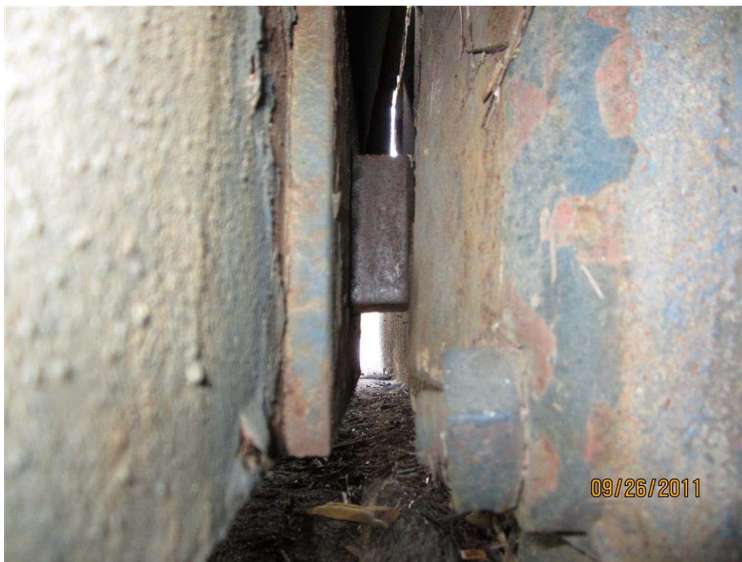
Photo M11: The east centering lock pin does not travel far enough to engage the receiver.
