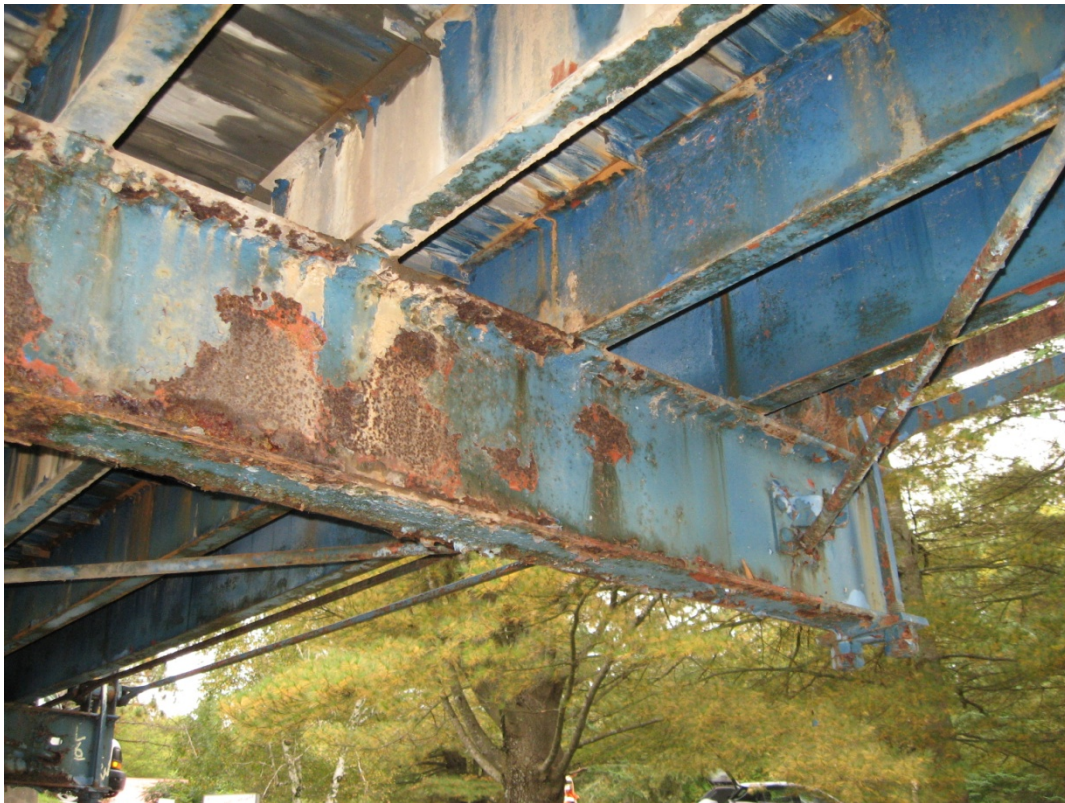
Photo F23: Typical condition of the floor beams, stringers and bottom lateral bracing.
