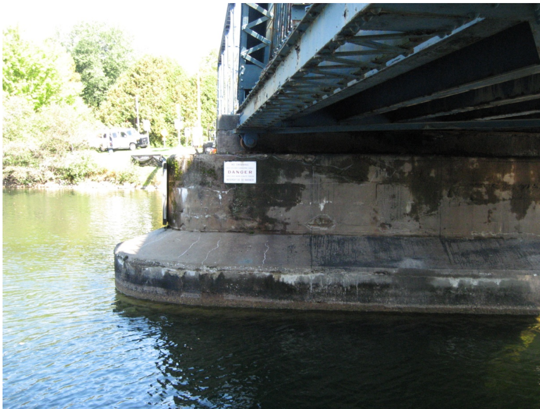
Photo S7: East pier. Note the typical cracks with efflorescence and areas of spalling and disintegration.
