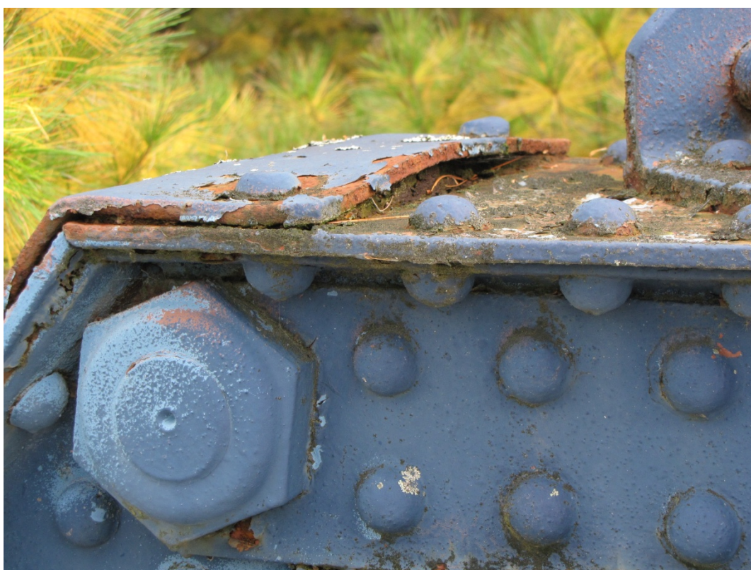
Photo F12: Severe rust jacking of the top chord cover plate at U6S.
