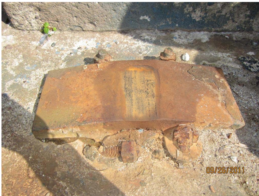
Photo M7: Northeast End Castor Rest Plate. Slight movement was noted between both end rest plates and the pier. One of the four north rest plate anchor bolts is bent. Also note the heavy wear on the rest plate due to contact with the roller.
