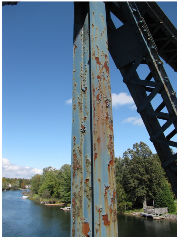
Photo S22: V6N – typical condition of vertical truss members with extensive areas of coating failure and light corrosion.
