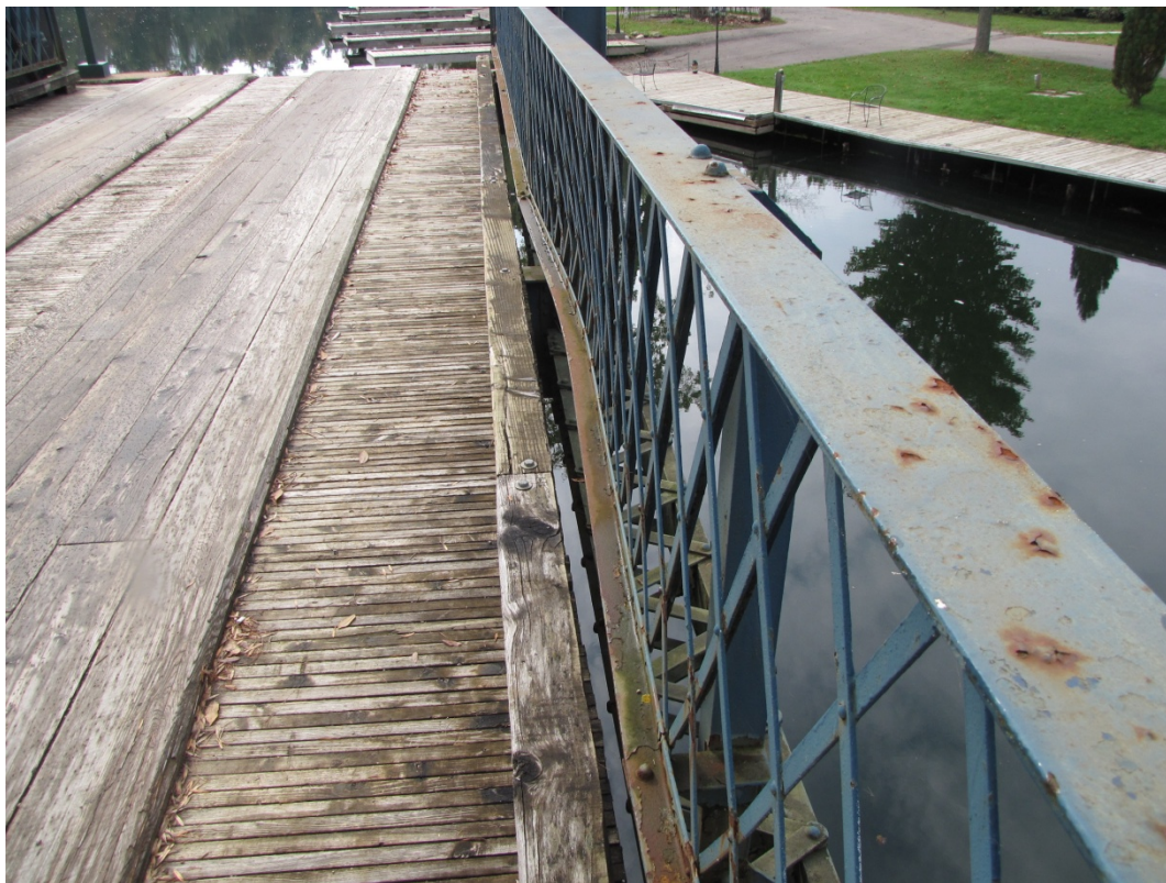
Photo S46: Impact damage to bottom rail on north railing between FB1 and FB2.
