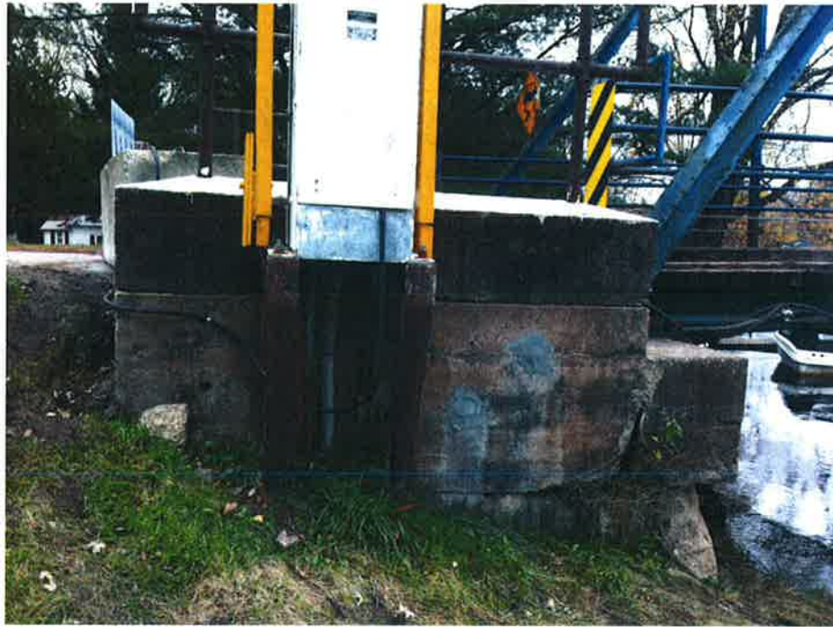
No.5: North wing wall of east abutment, looking south; the linear cracks appear to be construction joints.
