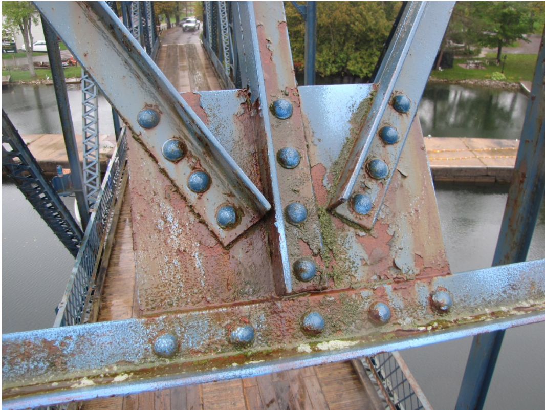
Photo S23: The east portal frame members exhibit the typical coating loss and light corrosion. Note the water collecting in the bottom member.
