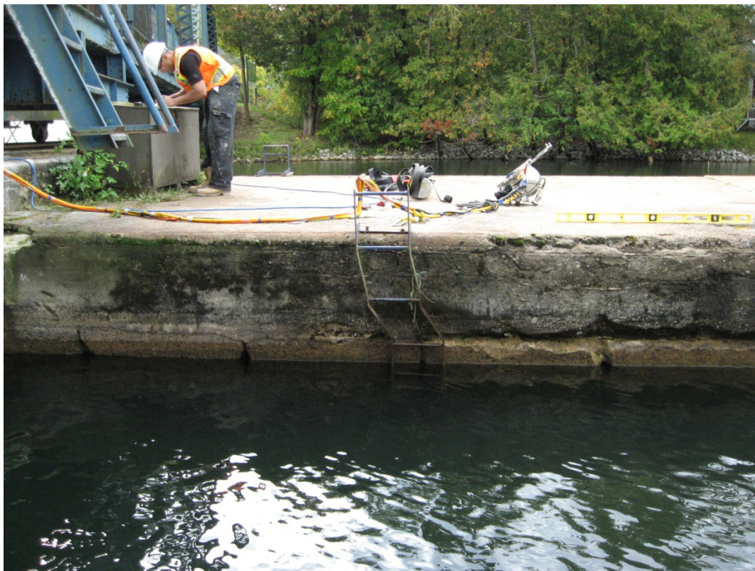
Photo S15: The ladder on the east side of the north section of the rest pier is bent in the downstream direction.
