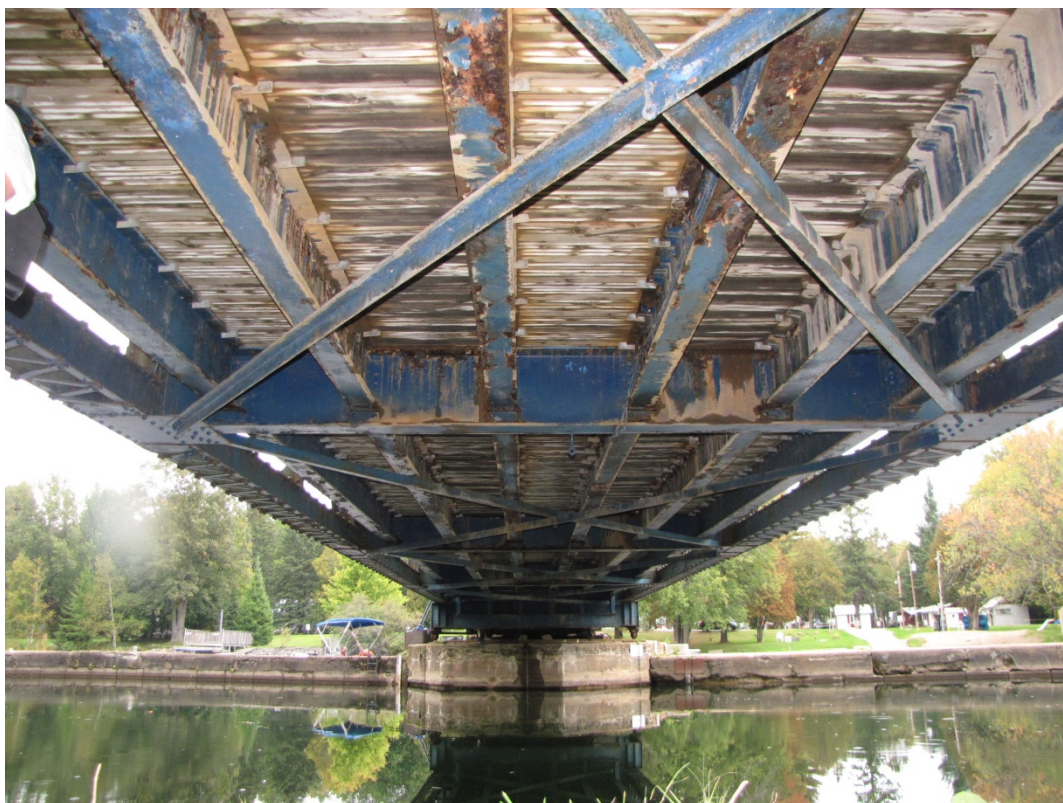
Photo S26: Looking east from the west embankment. Note the typical condition of the floor system and deck members.
