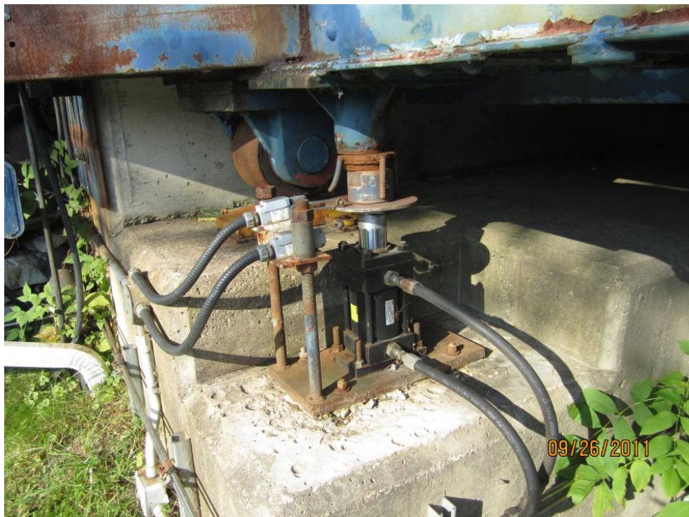
Photo E8: Bridge End Lift System. Note the corrosion on the limit switch support.
