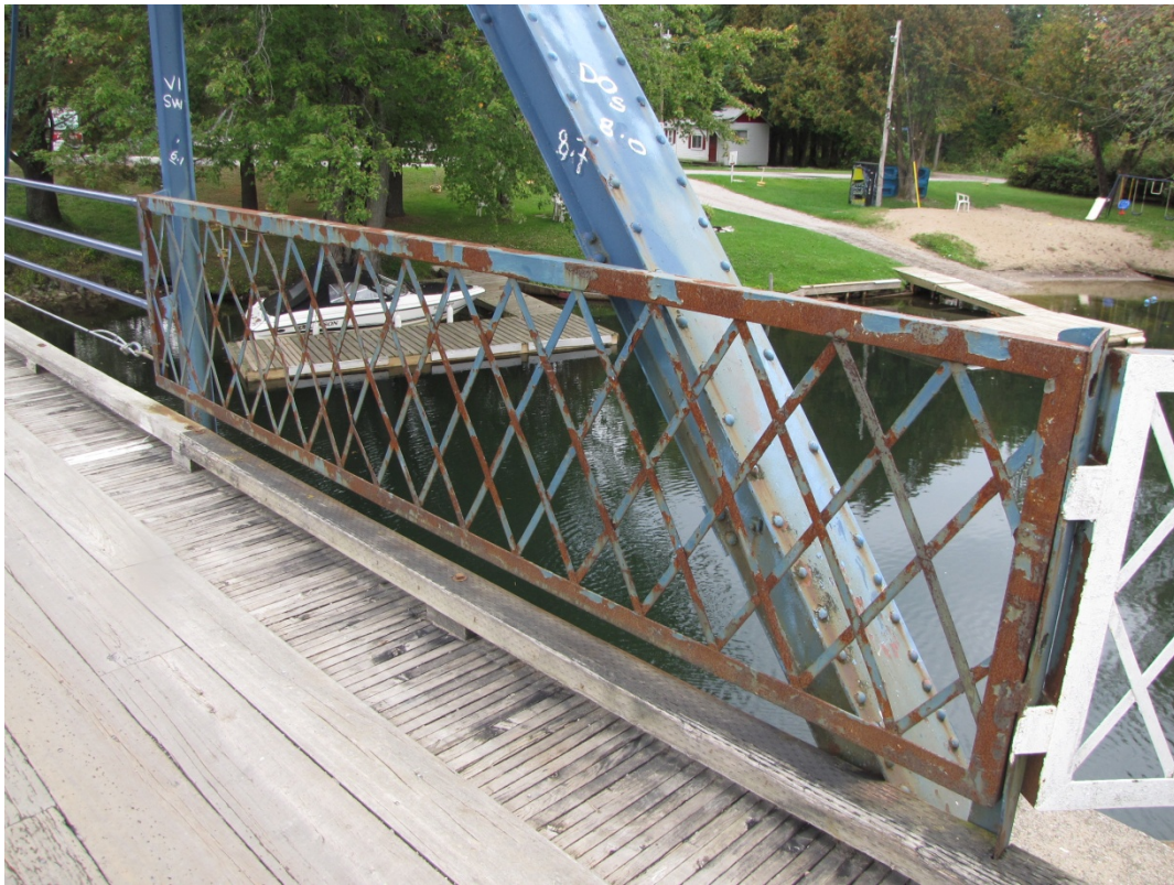
Photo F33: Typical extensive coating failure and light corrosion on the decorative railing panels
