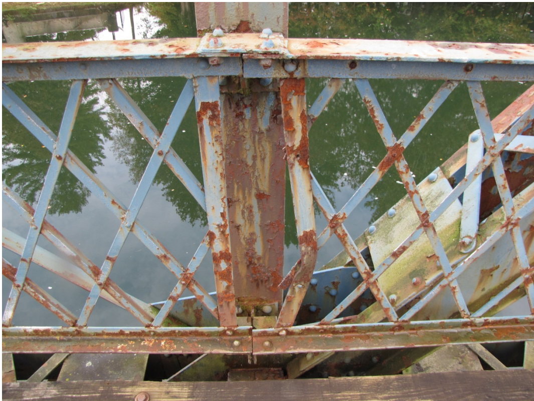
Photo S44: North railing at FB5. Impact damage to end baluster and lattice. The bolt in the lower connection is loose. Note typical coating system condition.
