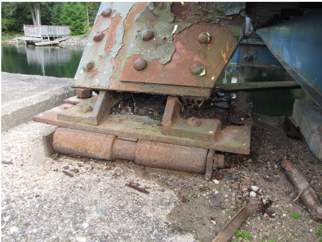
Photo F30: North-west bearing – the roller is no longer on the steel bearing plate.
