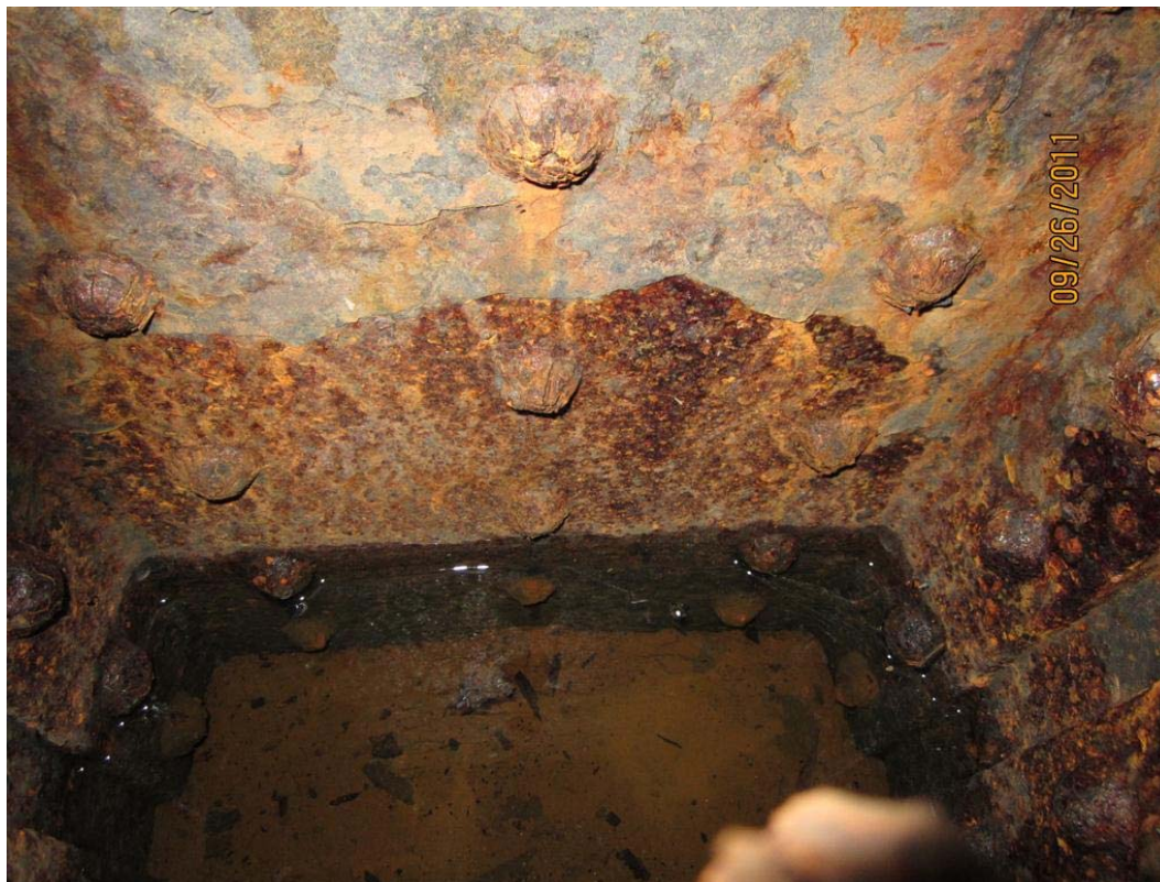
Photo M3: The interior of the pivot girder collects debris and standing water.
