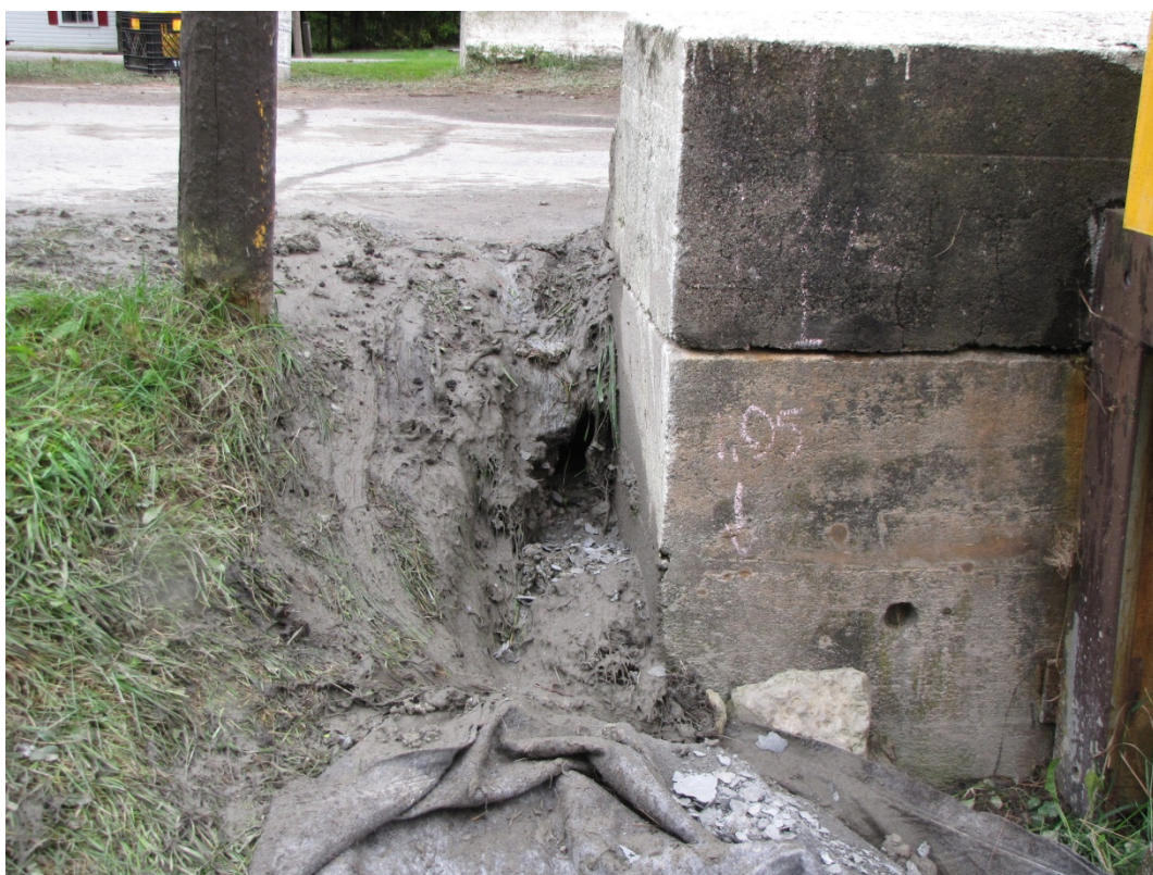
Photo F32: Erosion of the north-east embankment material around the guiderail post.
