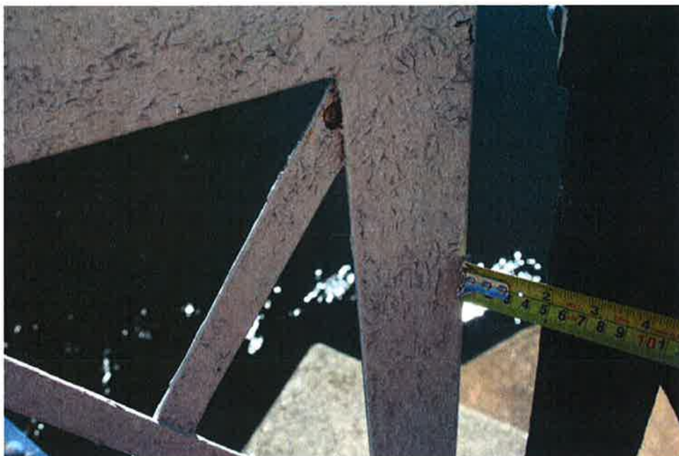
Picture 2: The space between guardrails of the swing bridge and fixed bridge on the south side; the space used to be much wider and was approximately the same as the space on the north side. It is now about 30 mm less than the space on the north side.
