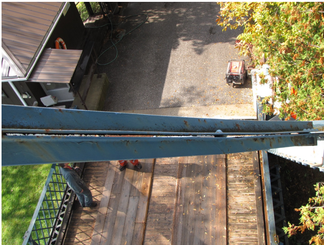
Photo S25: The north diagonal member in the west portal frame is bent.
