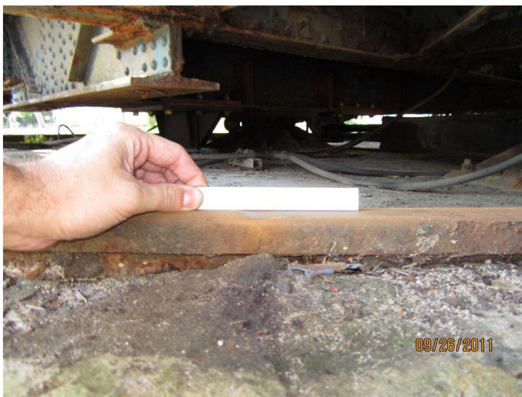
Photo M4: There is an impression on top of the rail from the wheel as a result of carrying live load.
