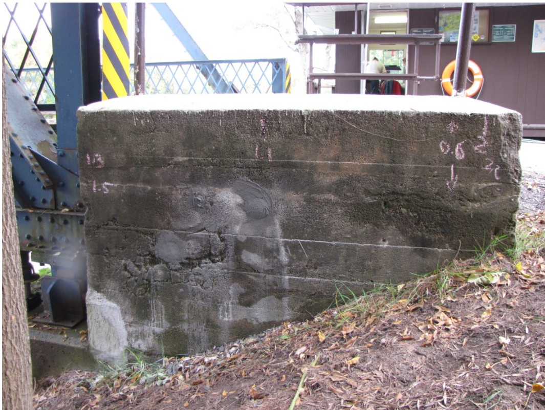
Photo S20: The north-west wingwall exhibits areas of honeycombing and scaling.
