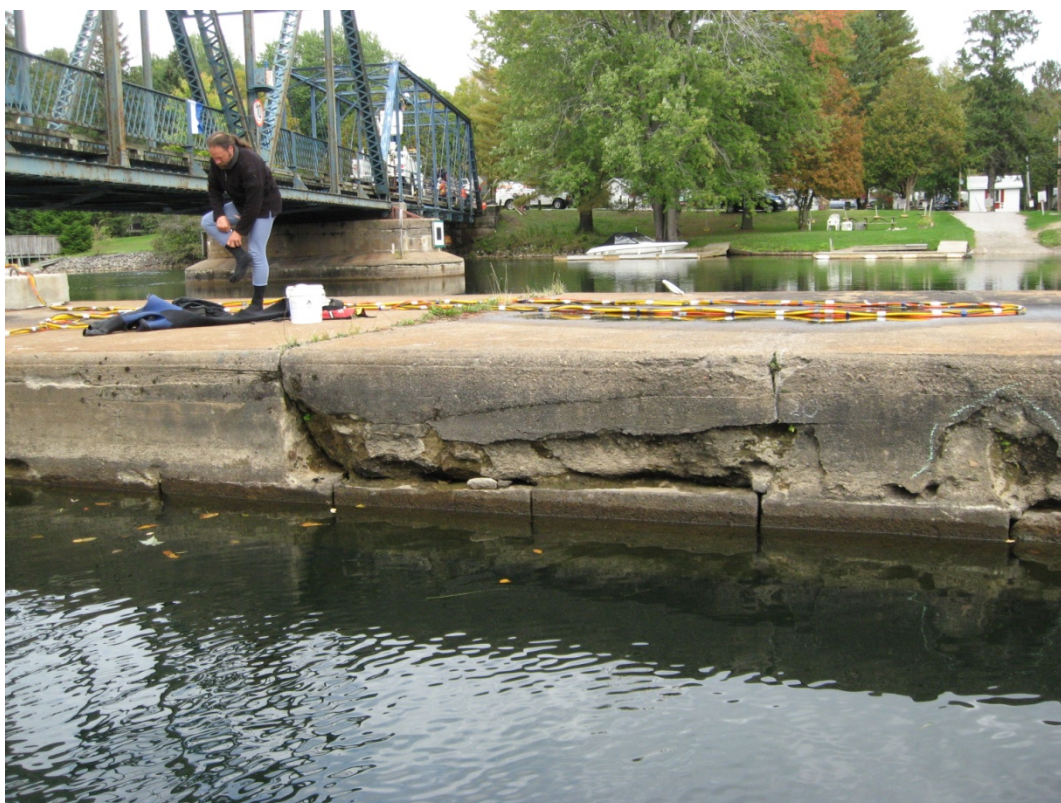
Photo S16: Large spalled section in the concrete cap on the west side of the south section of the rest pier.
