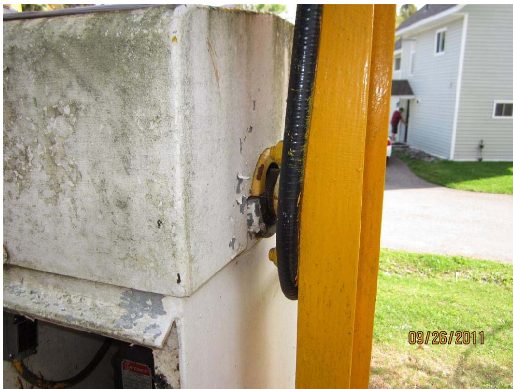
Photo M23: West Traffic Gate. The gate arm bearings are in poor condition and appear heavily worn.
