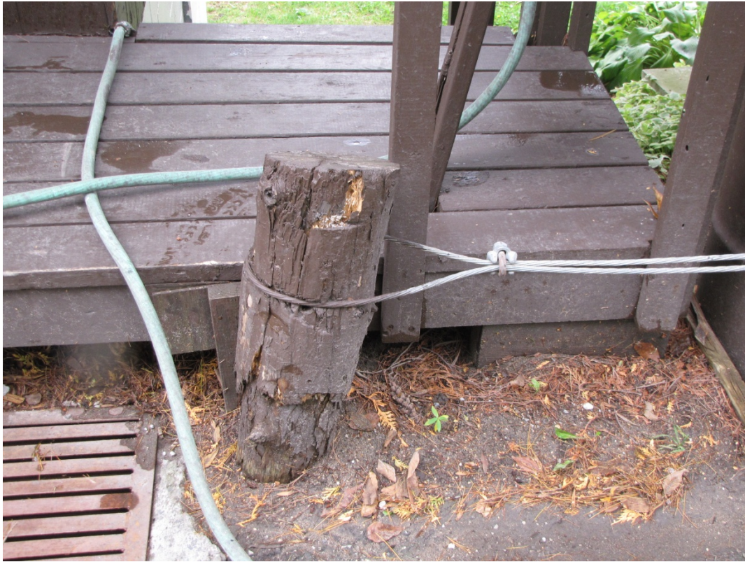
Photo S49: The first ten posts at the east end of the south-west guiderail are rotten (east post shown).
