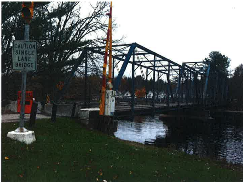
No.2: Overview of the Hamlet Bridge, looking west; the closest pier is the east pier which supports the west end of fixed bridge and east end of the swing bridge.
