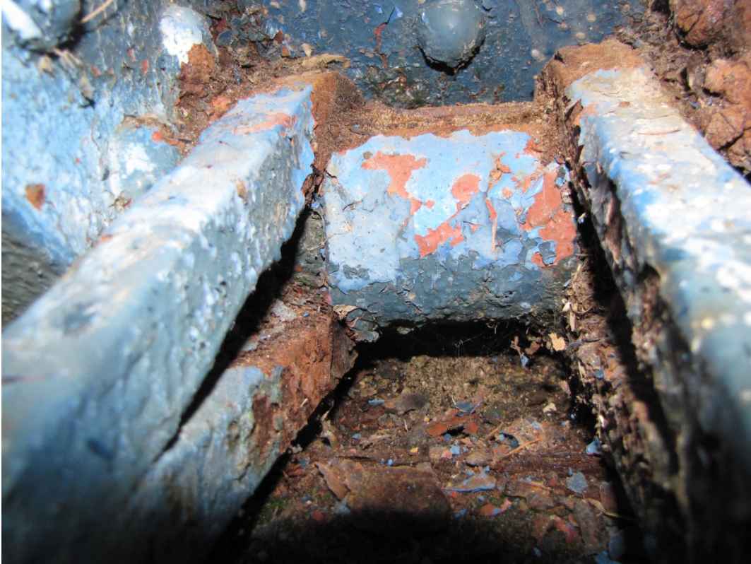
Photo F21: Severe corrosion and rust jacking of the north bottom chord I-bars at the west end of bridge.
