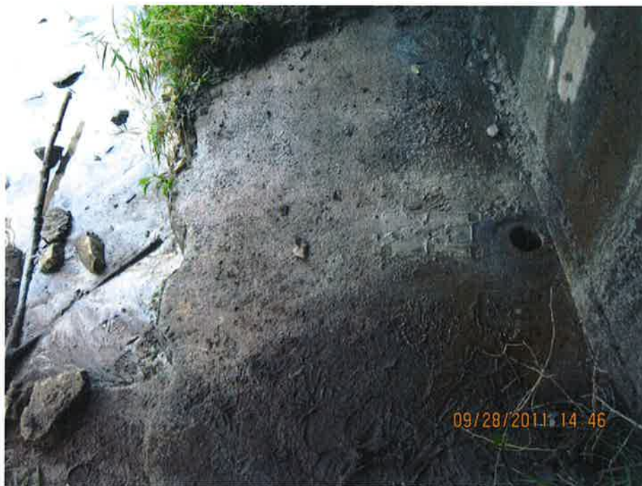
No.8: The concrete platform between the sheet piles and abutment wall; the core hole was terminated in the concrete due to refusal on steel rebar at a depth of about 0.5 m.
