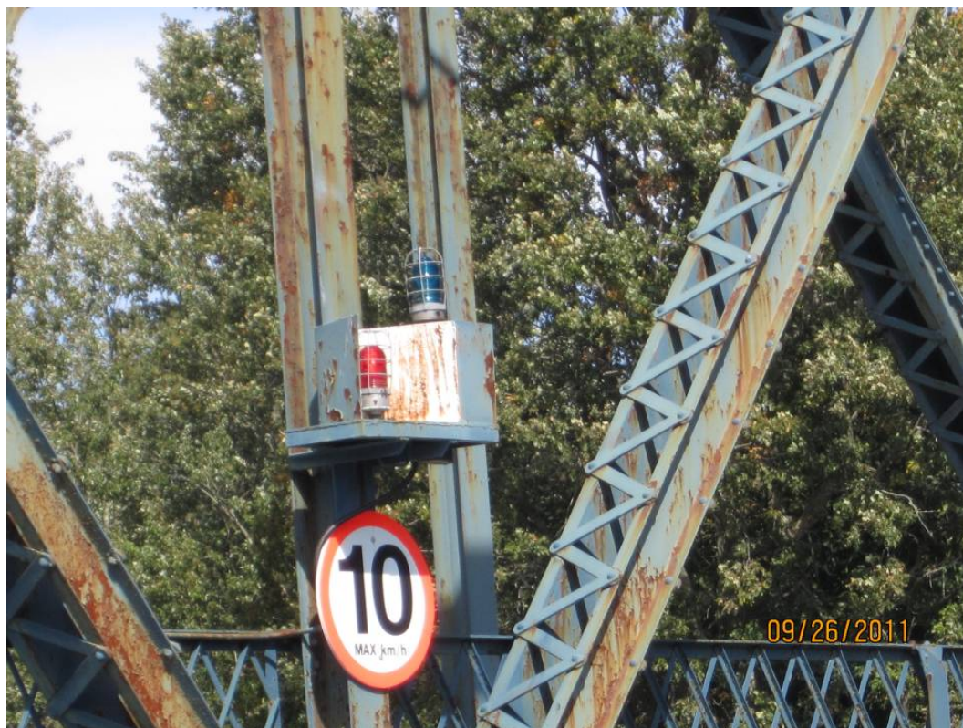
Photo E17: Span Navigation Lights.
