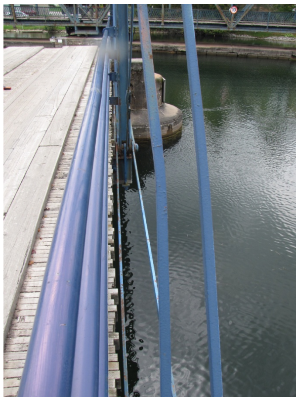
Photo F17: Inside member of U2N-L3N is bent.
