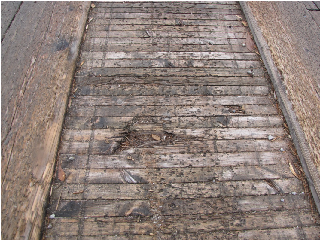
Photo S40: Central section of exposed deck between FB0 and FB1. Several deck members have areas of rotting. Note the typical small rot holes throughout and the abrasion on the edges of the inside wearing surface members.
