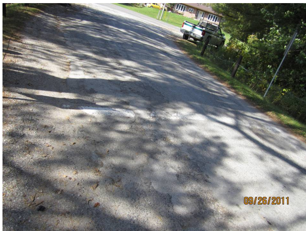
Photo E14: West Approach Stop Bar. Note the stop bar is heavily worn.
