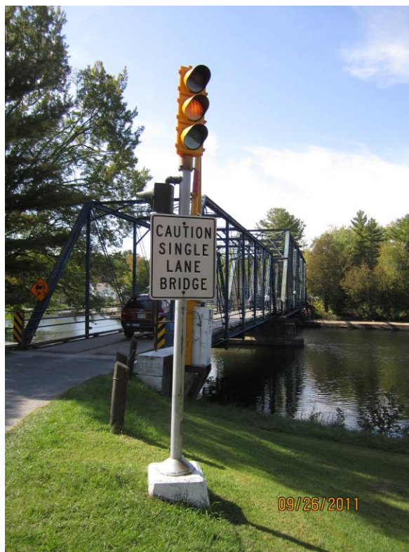
Photo E13: Typical Traffic Signal. Note the good condition of the pole and the signal heads. Also note the warning sign mounted on the signal pole.
