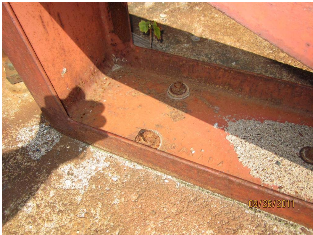
Photo M14: The east end of travel stop anchor bolts are in poor condition and exhibit evidence that the stop was impacted resulting in the anchors being slightly pulled out.
