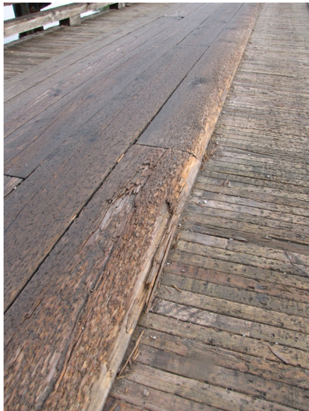
Photo S42: The edge of the inside wearing surface boards are typically rotten.
