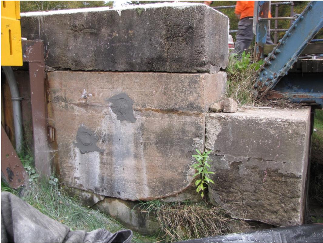
Photo F5: The north-east wingwall has wide gaps at the construction joints plus areas of spalling and disintegration.
