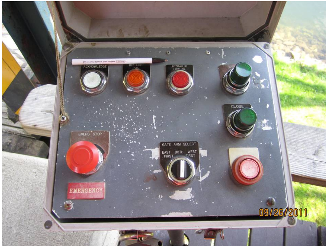
Photo E7: Bridge Operators Control Console. Note the two pushbutton controls for traffic control and bridge operation and the limited indication lights for status indication. Additionally, note the pushbutton at the lower right hand corner is not labelled.
