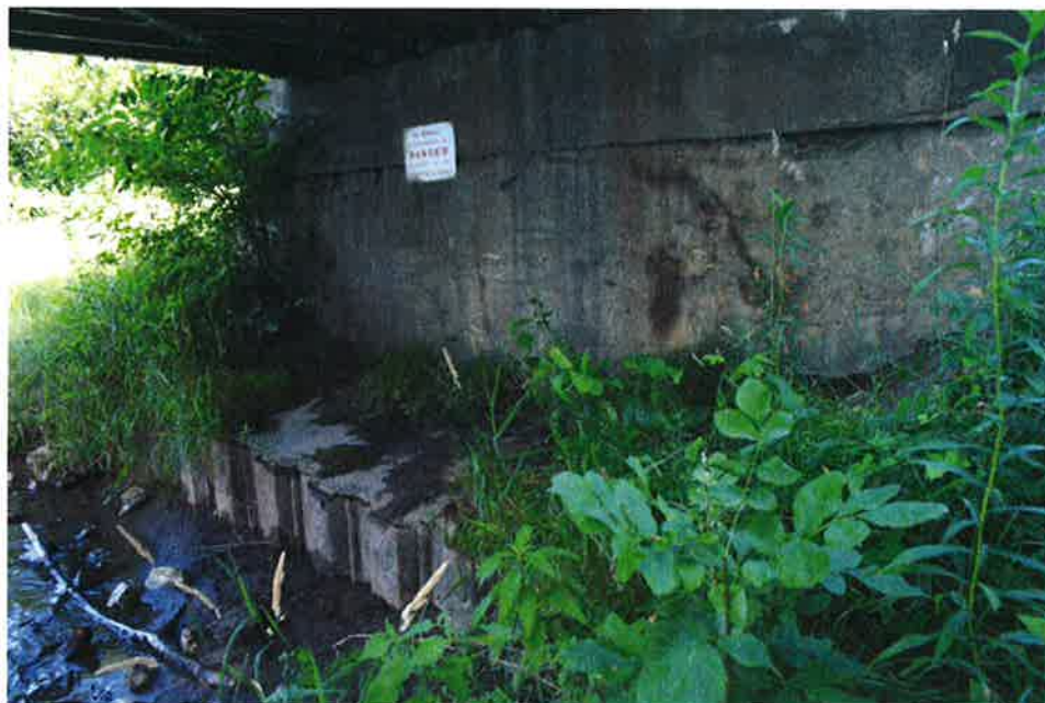
No.6: The north abutment concrete wall under the bridge; note the sheet pile wall installed for erosion protection; note the concrete platform behind the sheet pile walls.
