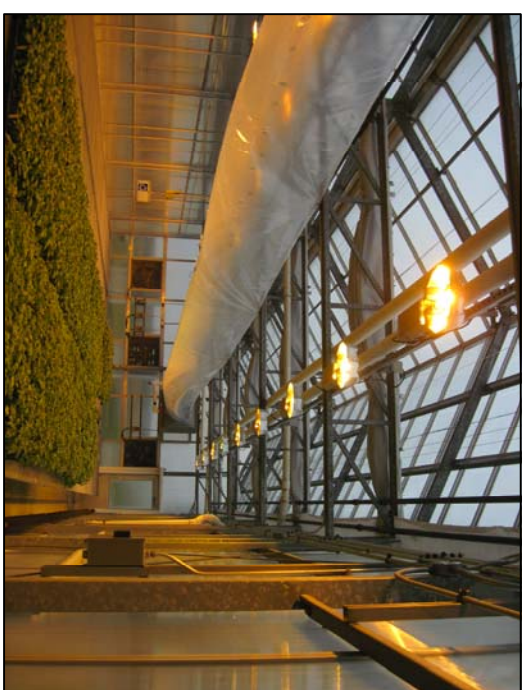
TYPICAL INTERIOR VIEW OF GREENHOUSES 2 AND 3 FACING SOUTH
