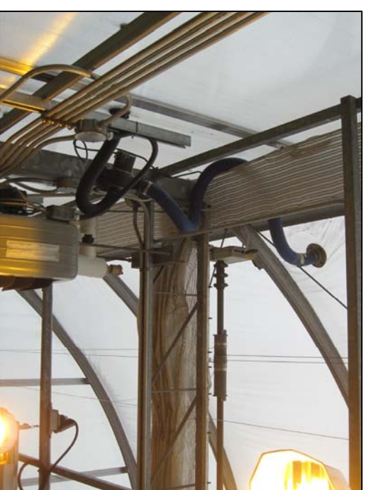
TYPICAL GREENHOUSE 2 AND 3 DRIVE MOTOR ASSEMBLY
