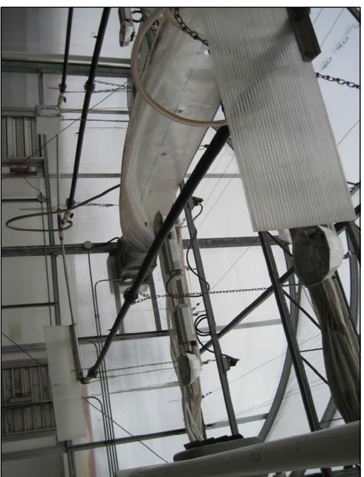
GREENHOUSE 6 INTERIOR VIEW FACING NORTH
