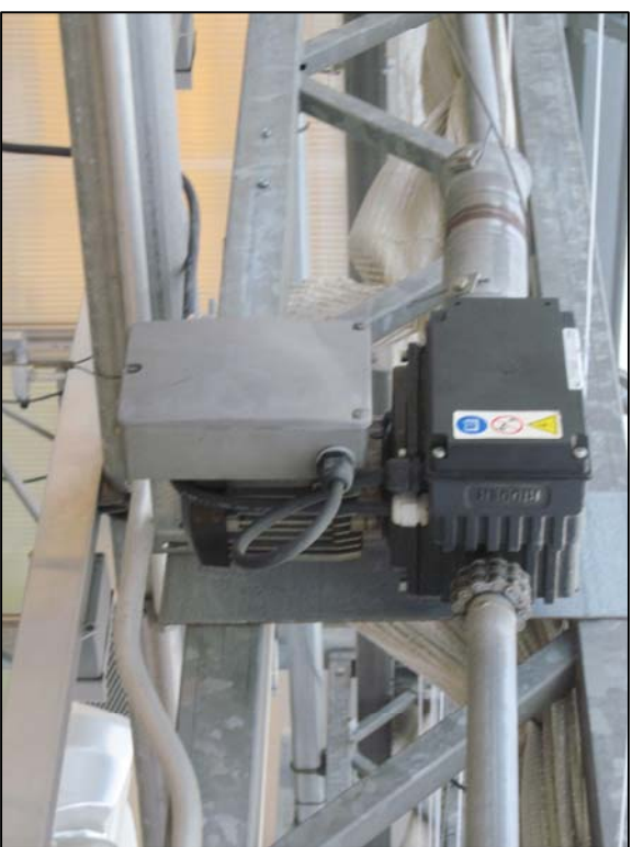
TYPICAL GREENHOUSE DRIVE MOTOR ASSEMBLY
