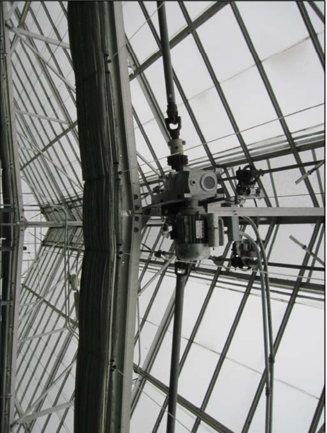
GREENHOUSE 1 DRIVE MOTOR ASSEMBLY
