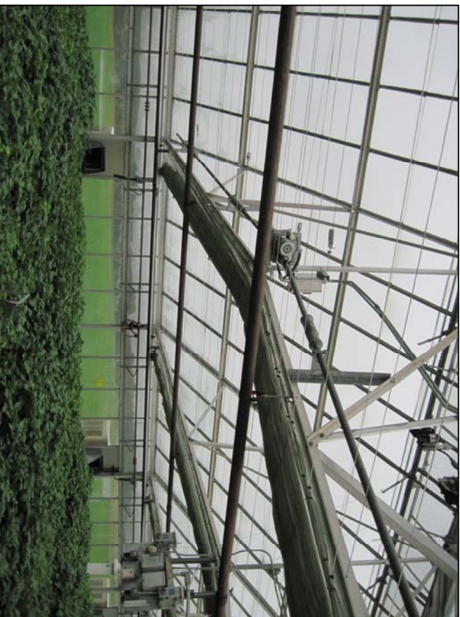
GREENHOUSE 1 DRIVE SHAFT ASSEMBLY
