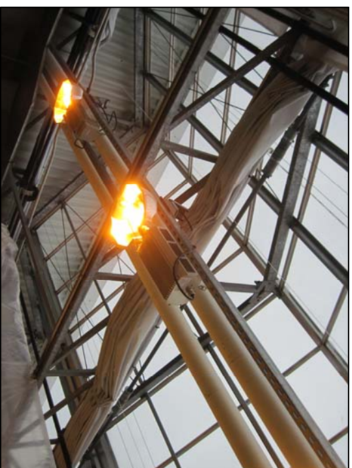
TYPICAL GREENHOUSE 2 AND 3 SHADE DRIVE SHAFT ASSEMBLY
