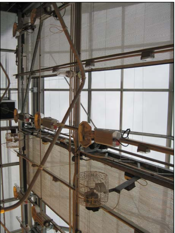
TYPICAL VIEW OF PARTIALLY DRAWN SHADE CURTAIN
