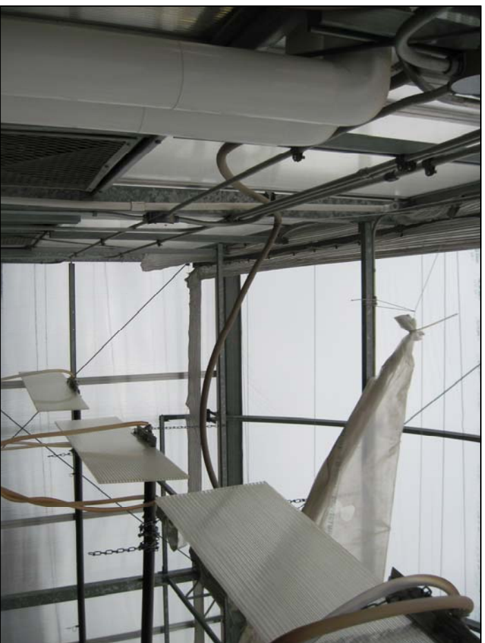
GREENHOUSE 6 INTERIOR VIEW FACING WEST
