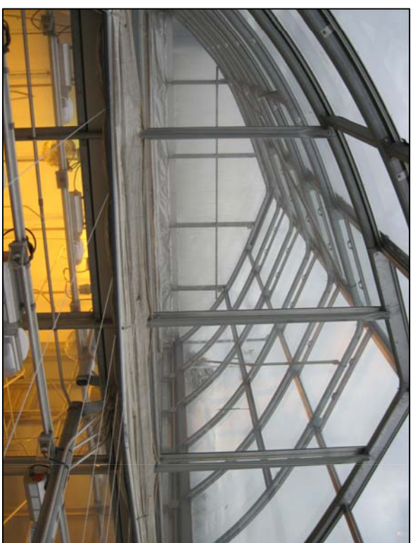
TYPICAL VIEW FROM CEILING SPACE
