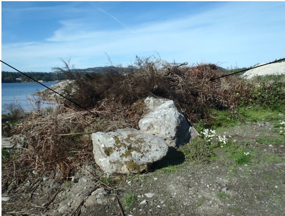
Photograph 7: View of pile of mixed brush for segregation and off-site disposal, and riprap for segregation and placed along the perimeter to restrict site access.
