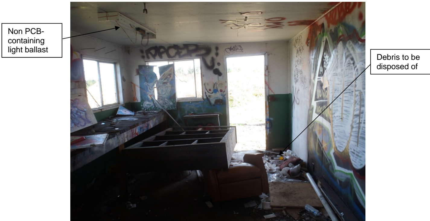
Photograph 4: View of the interior of the wooden shed.
