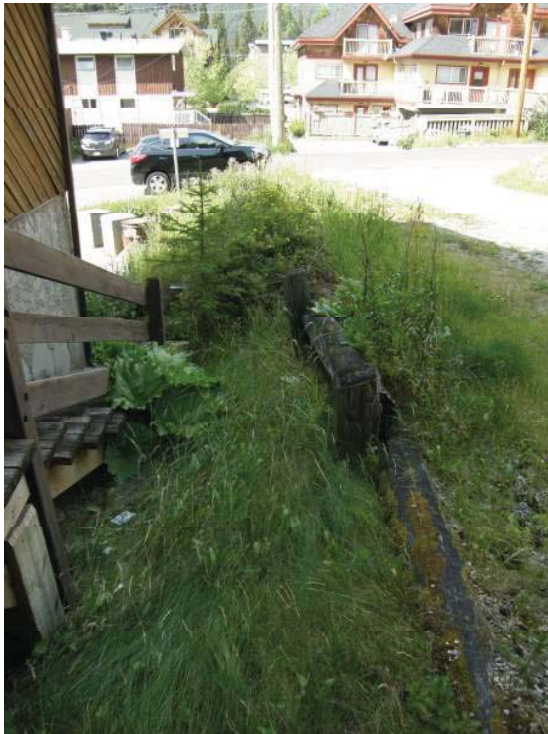
Figure 5: Timber retaining wall to remain in place as to not disturb the adjacent property.
