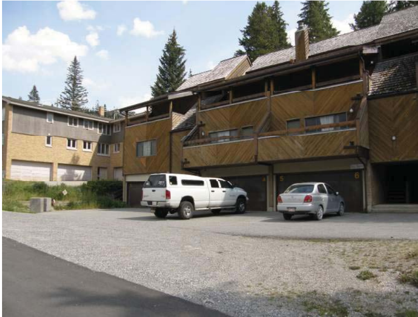
Figure 6: Asphalt surface to be removed and fine graded to allow for positive drainage away from the structure.
