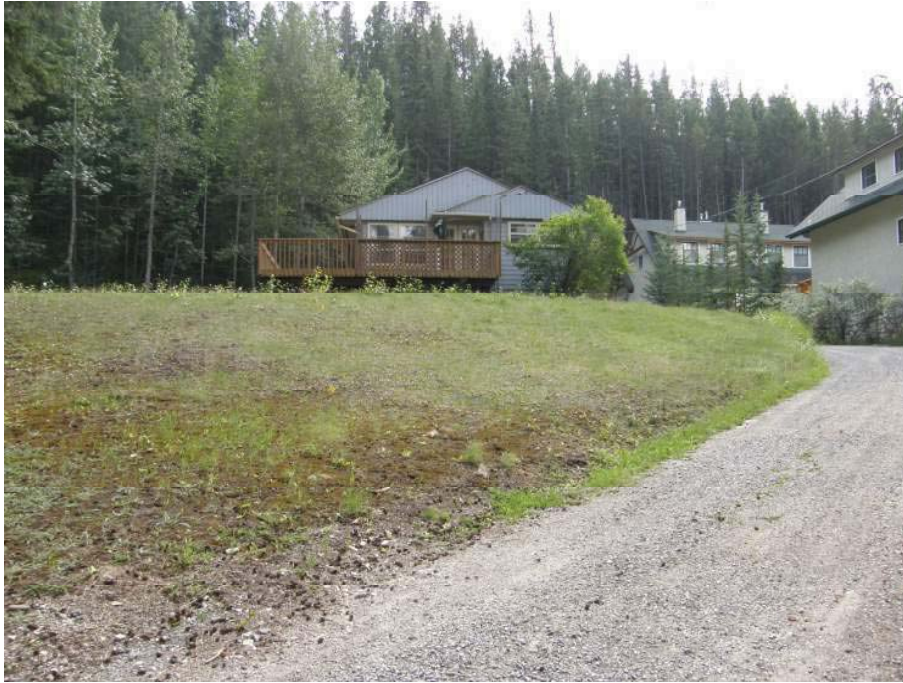
Figure 3: Grassed landscape hill that is to be cut down and re-contoured to generate fill for backfilling building footprint of house, garage and tenplex.
