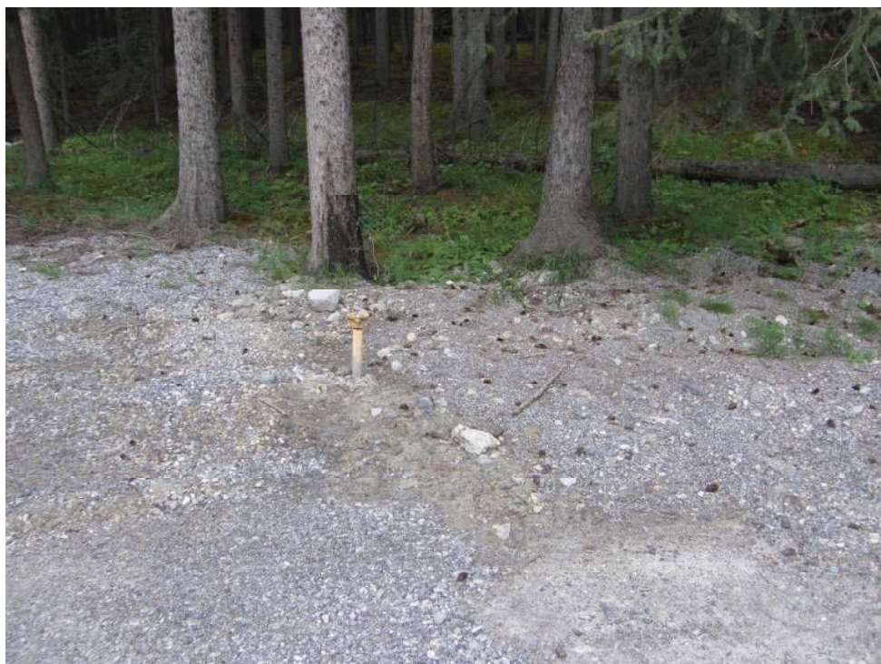
Figure 4: 151 Cave Ave curbstop and water service to be decommissioned and removed.
