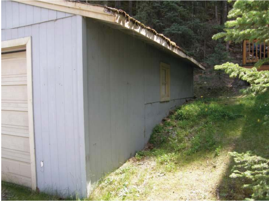
Figure 1: Slope to be backfilled and compacted once garage embedded in slope is removed.
