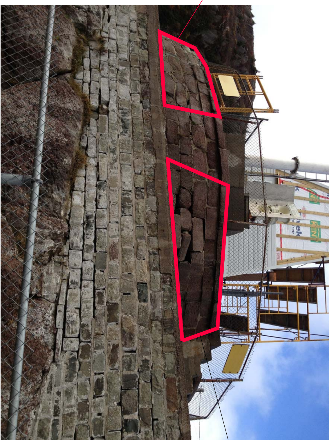
PHOTO 8-MASONRY RETAINING WALLS-EAST ELEVATION
