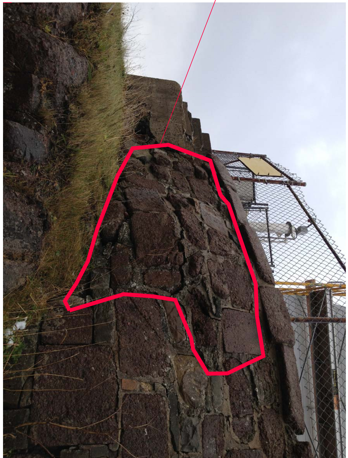
PHOTO 5-CIRCULAR MASONRY RETAINING WALL
