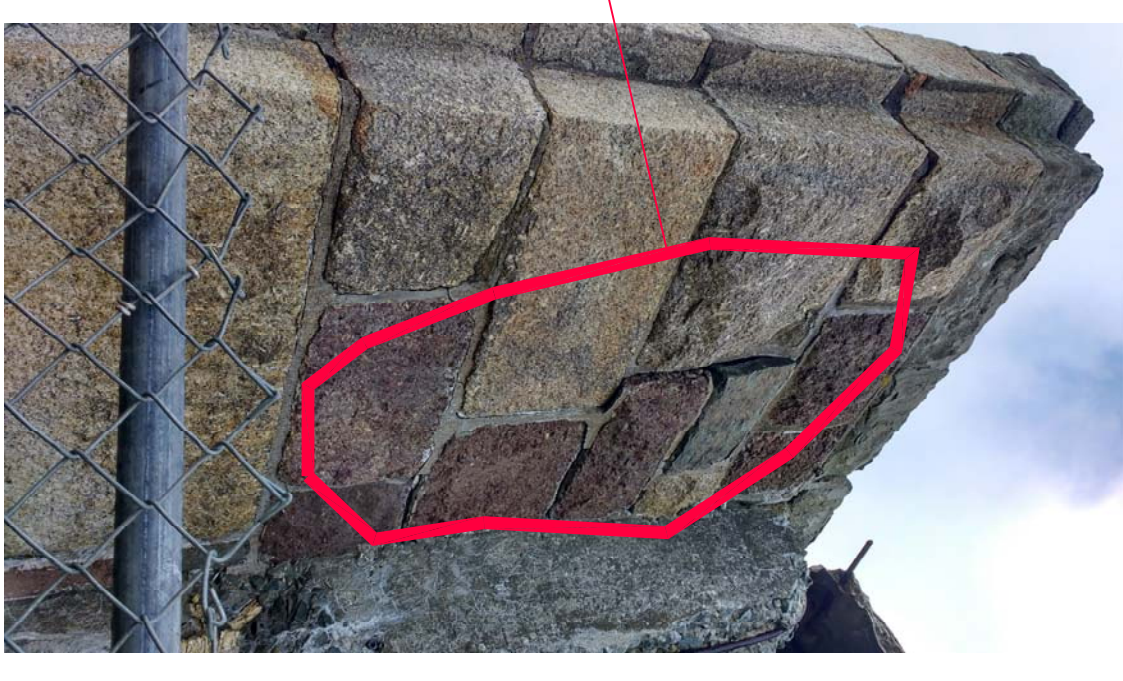
PHOTO 20-CRACKS AND WALL BULGE
