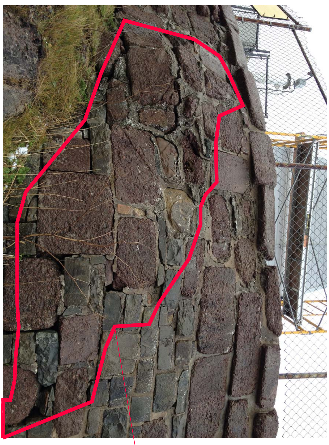
PHOTO 2-CIRCULAR MASONRY RETAINING WALL
