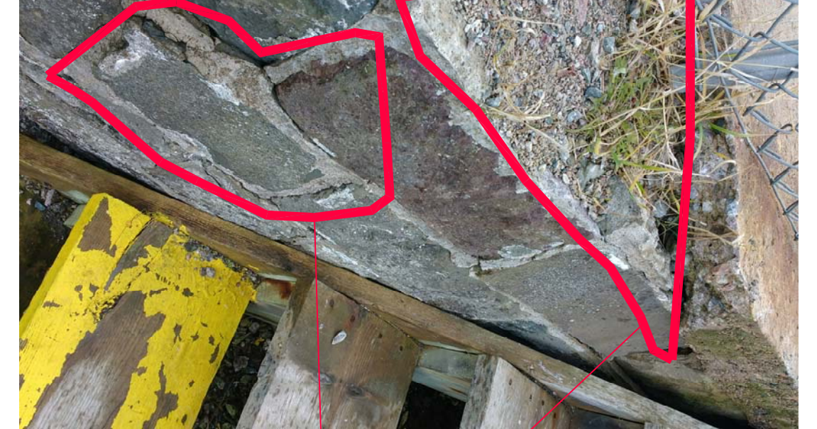
PHOTO 13-CONCRETE CAP MISSING
