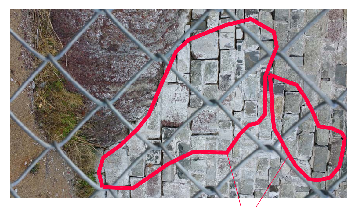
PHOTO 20-CRACKS AND WALL BULGE
