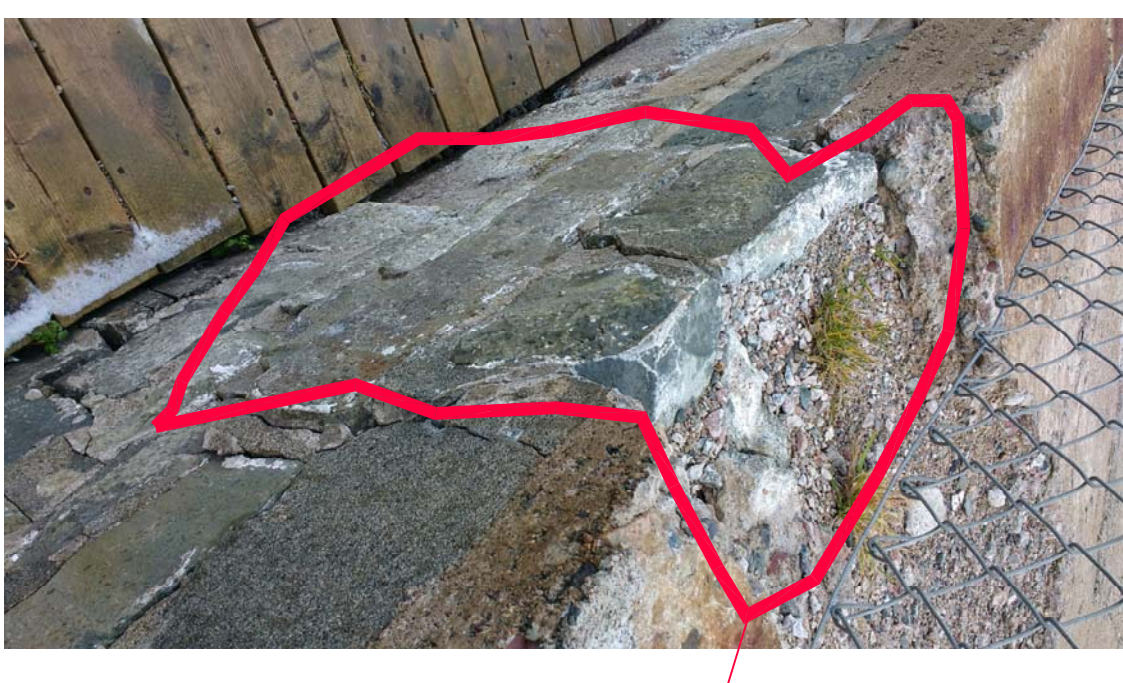
PHOTO 15-MASONRY WALL BULGE AND CONCRETE CAP LOSE
