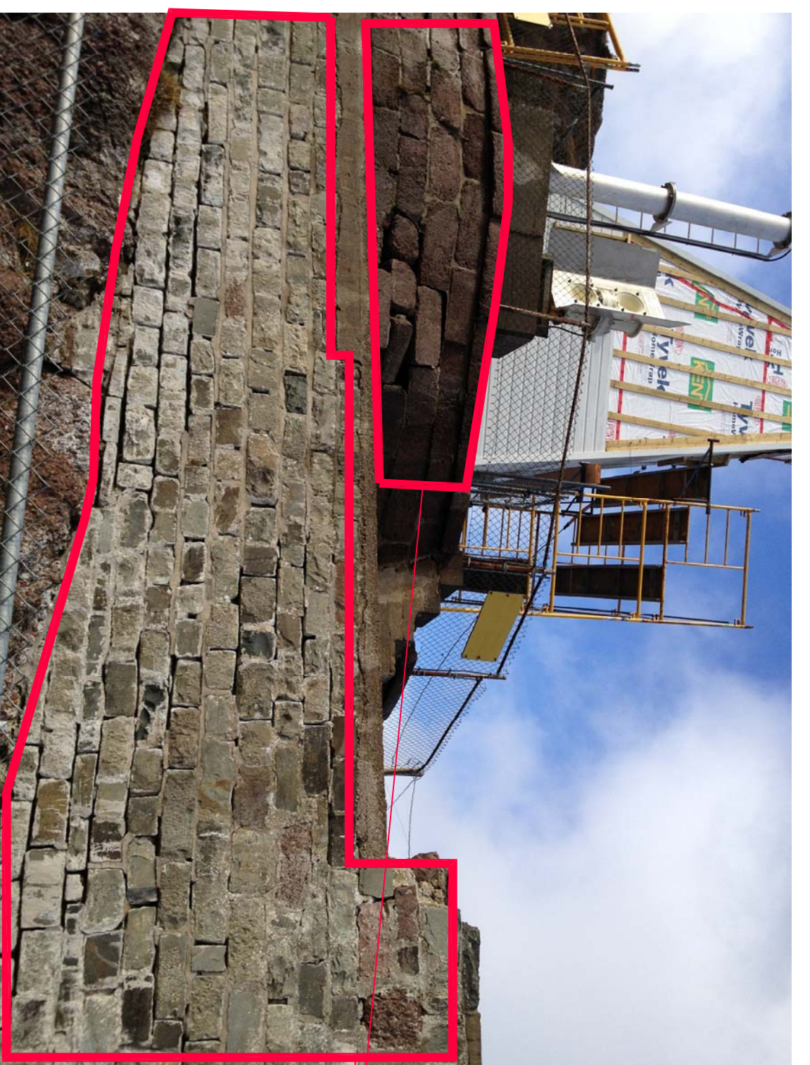
PHOTO 9-MASONRY RETAINING WALLS-EAST ELEVATION
