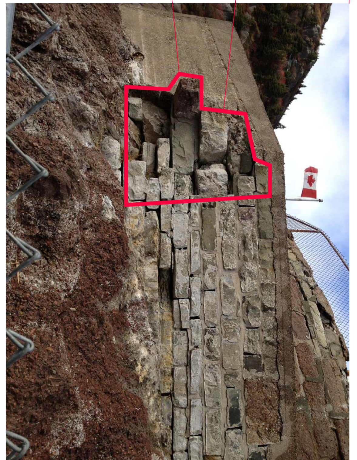
PHOTO 10-CORNER OF MASONRY WALL AND CONCRETE RETAINING WALL-SOUTH ELEVATION
