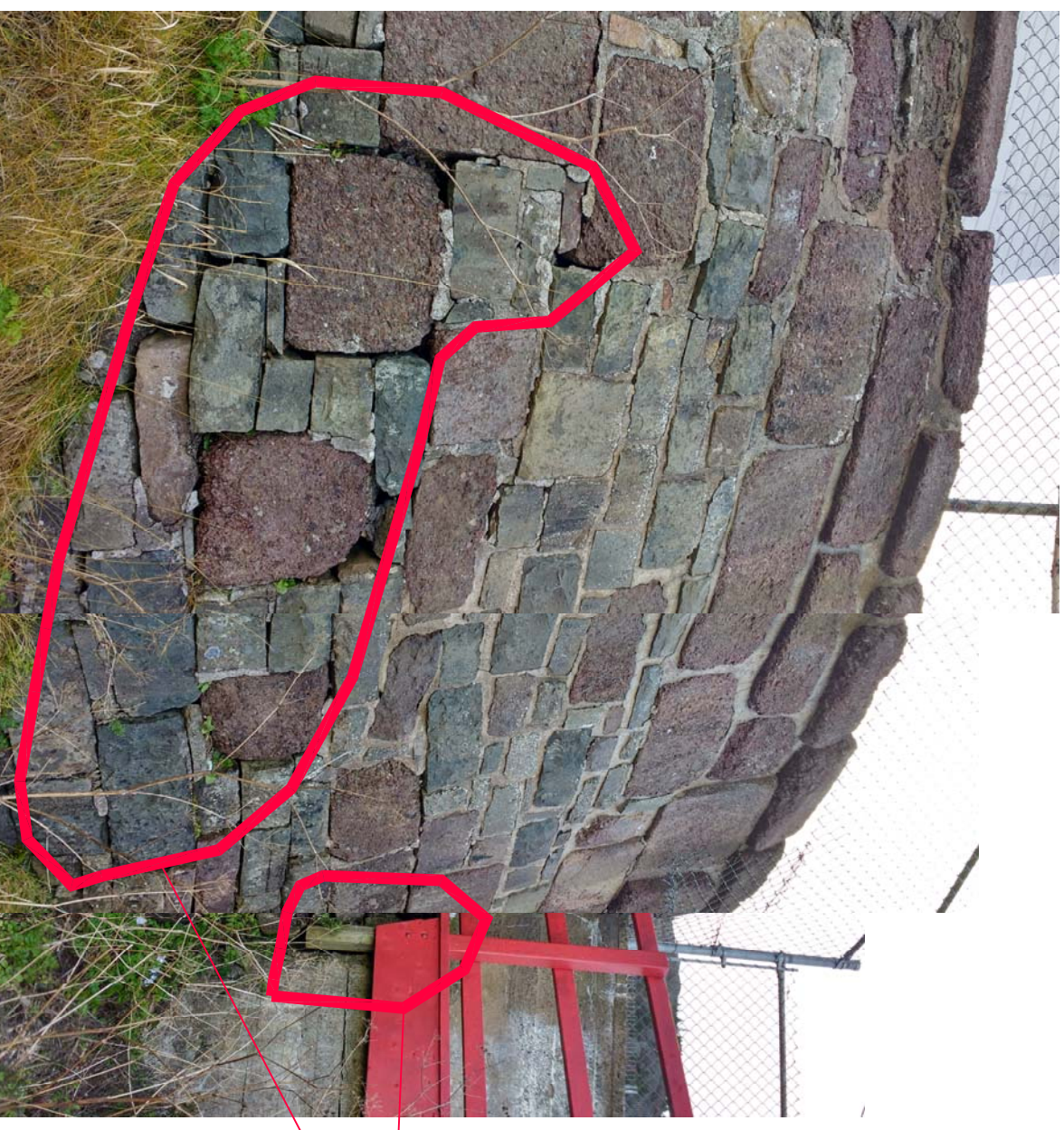
PHOTO 15-MASONRY WALL BULGE AND CONCRETE CAP LOSE
