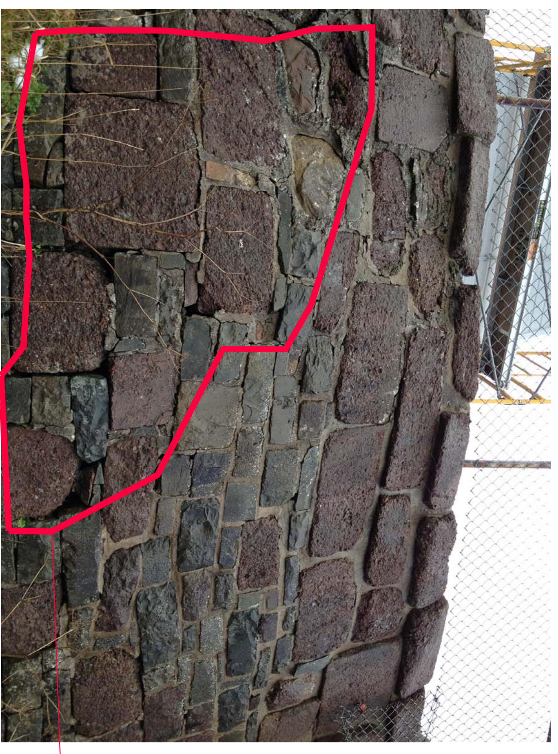
PHOTO 3-CIRCULAR MASONRY RETAINING WALL
