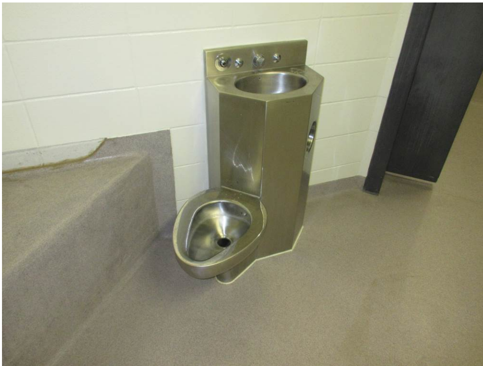
Photo 2 - Typical toilet to be removed and replaced
