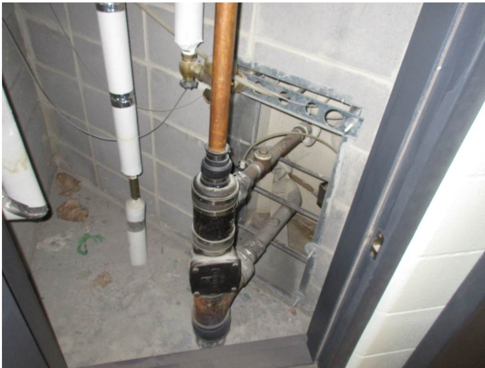
Photo 4 - Typical rear of toilet
