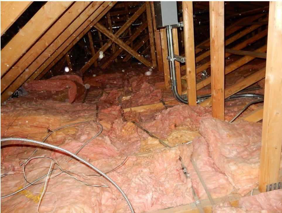
Photo 14 - Existing Attic Insulation
