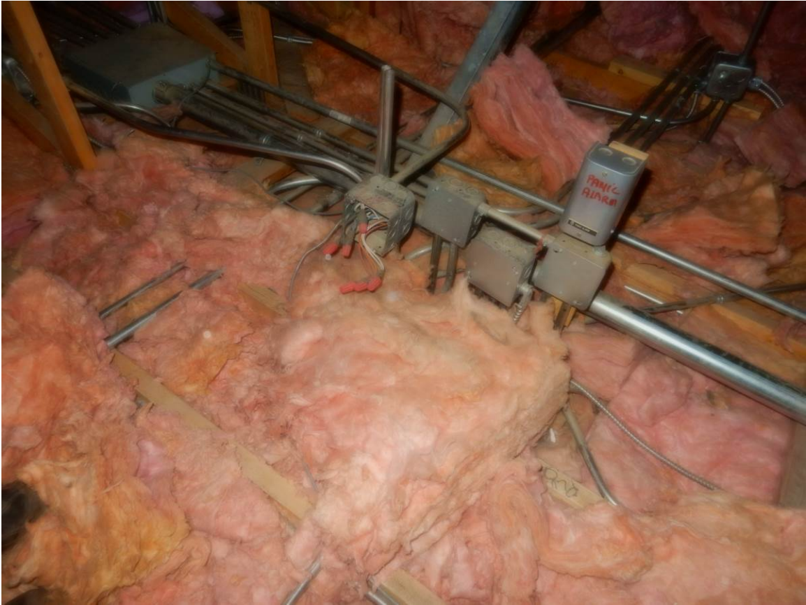
Photo 15 - Existing Electrical Box
