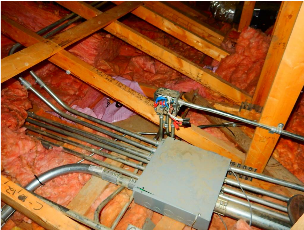
Photo 16 - Existing Electrical Box
