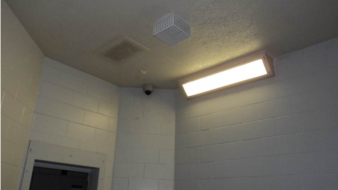
Photo 3 - Typical Existing Ceiling Light, Fire Alarm Cage and Camera
