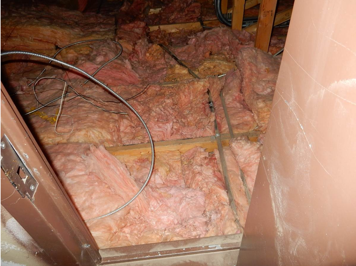
Photo 13 - Existing Attic Insulation
