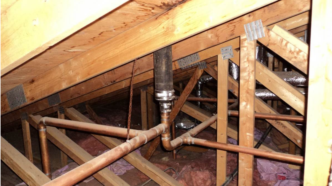
Photo 9 - Existing Plumbing Venting – To be Insulated
