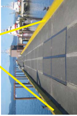
Typical Painting along surface and interior of Bull Rail. (Yellow)
