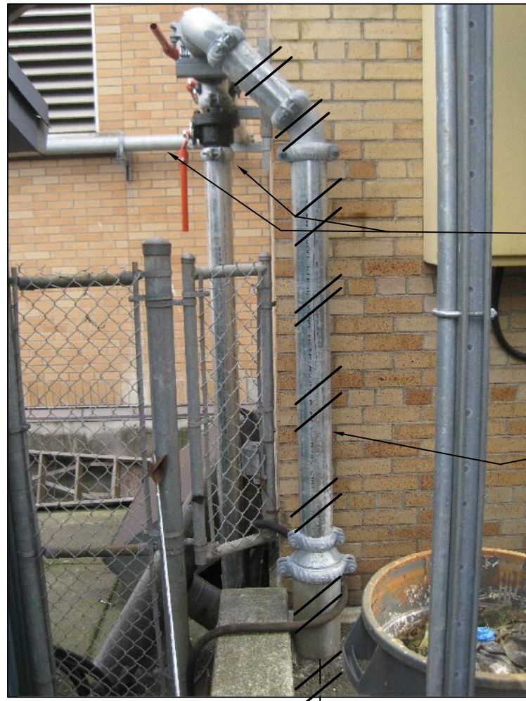
EXISTING COMPRESSED AIR STANDPIPE N.T.S.
