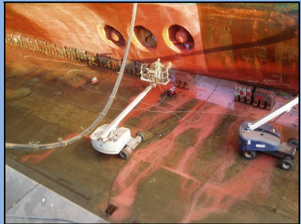
Antifoulant contaminated wash water entering the trench drain sump wells on dock bottom.
