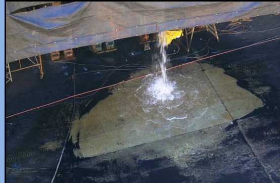
Sweep waste grit under the vessel to prevent it from being washed down the drain.
