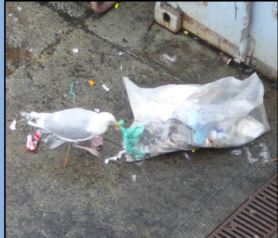
Leaving garbage around the work site attracts wildlife such as seagulls, racoons, and rats.
