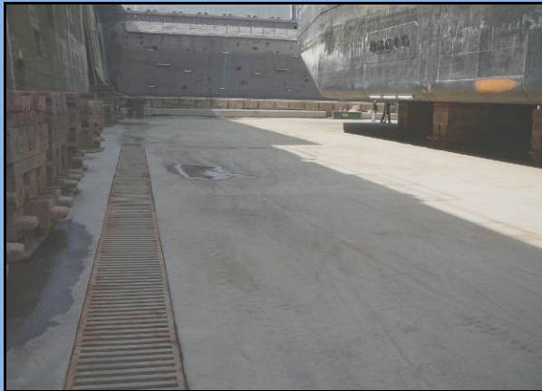
Example of a dock floor that would pass inspection.
