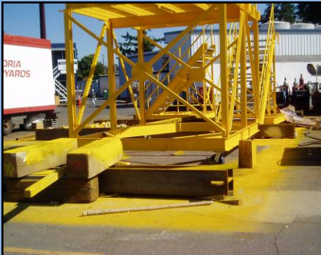
Ensure tarps are in place to prevent overspray impacting the surrounding work area.
