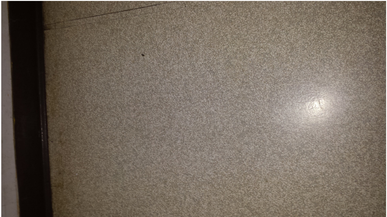
Photo 1 – ACM Sheet Vinyl Flooring with Stone Pattern and Paper Backing.
