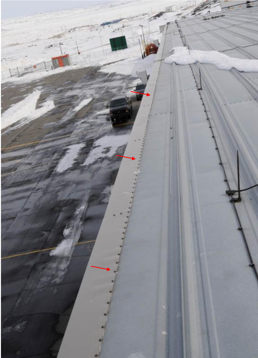
Photo 5: Photo at the eve of the roof deck along the east elevation of the building, viewing towards the south end of the roof deck. Joint between metal roof panel and sheet metal flashing to be repaired along the entire length of the east and west elevations.
