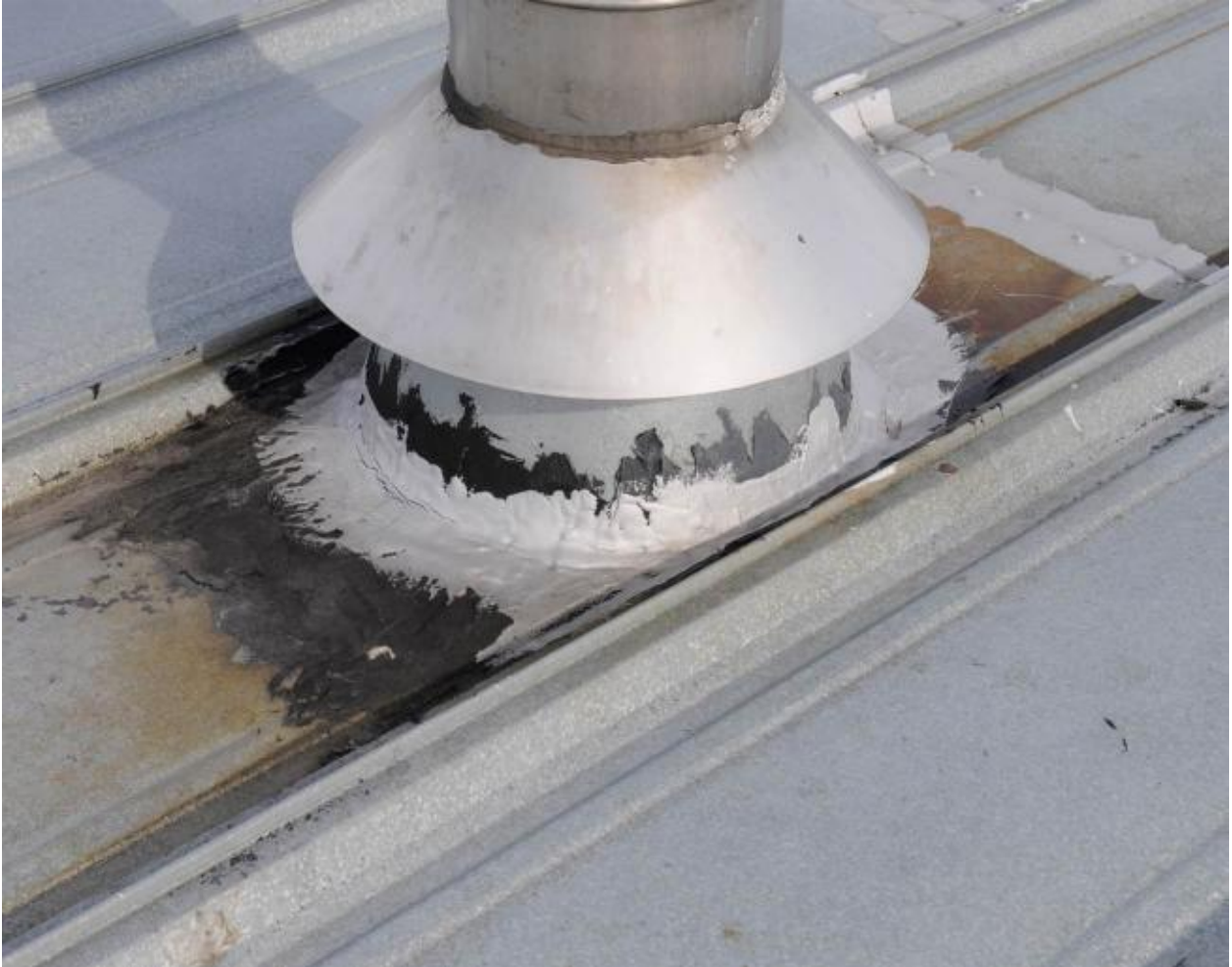
Photo 14: Typical metallic paint and asphalt mastic applied at the base of an exhaust stack. All asphalt and metallic paint material to be removed prior to installation of new bituminous membrane flashings.
