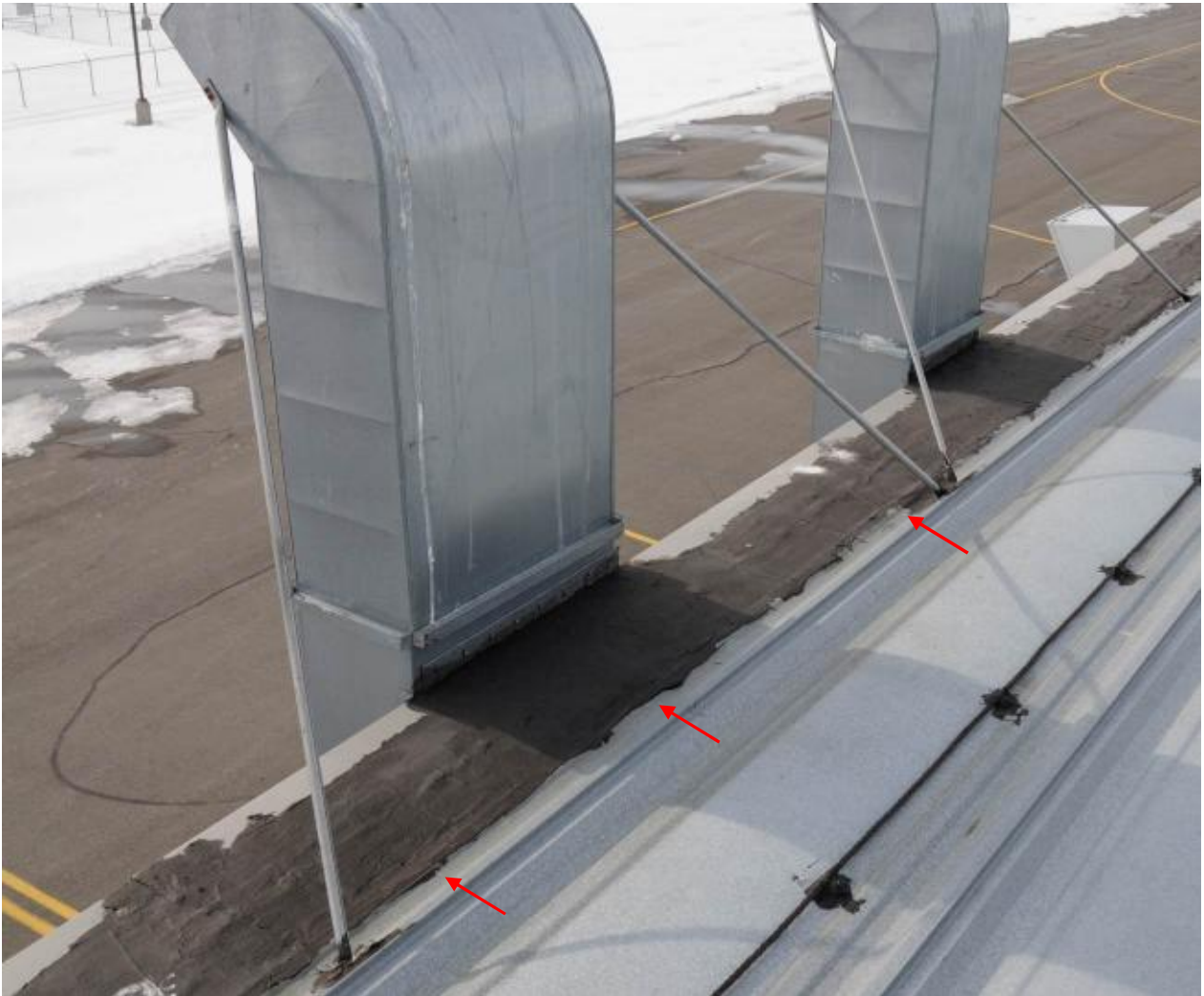
Photo 6: Typical asphalt mastic application at the interface between the sheet metal flashings along the eave of the roof system and metal roof panels on the east and west elevations. Photo taken along west elevation. All asphalt material to be removed prior to installation of new micro-sealant tape material along the joint between the metal pan and the sheet metal flashings along the east and west elevations.
