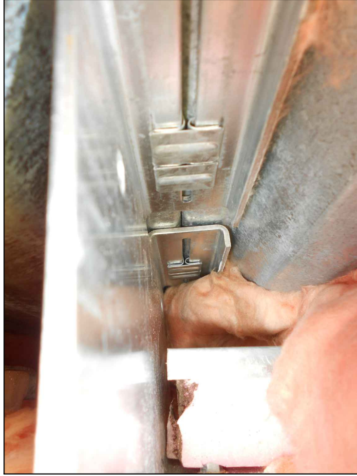
PHOTO_14: VIEW OF EXISTING PANEL CUT FROM THE UNDERSIDE OF THE ROOF SYSTEM
