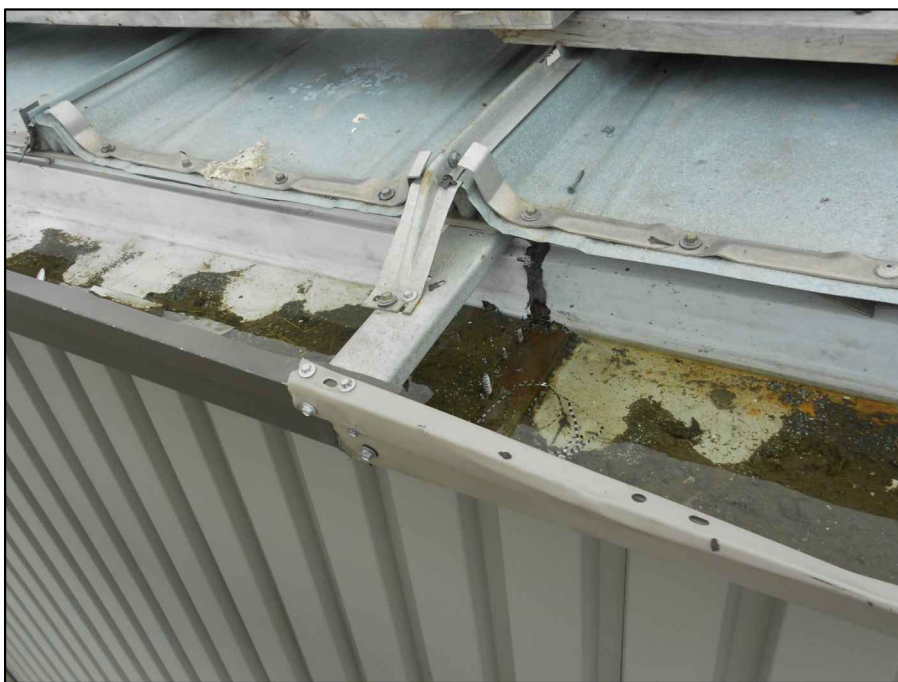
PHOTO_12: TYPICAL RAIN GUTTER SUPPORT BRACKET, NOTE DAMAGE AT TOP OF STANDING SEAM
