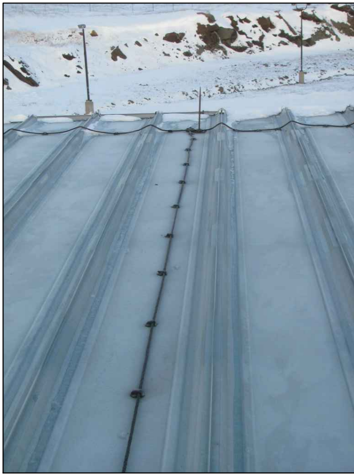
PHOTO_11: TYPICAL LIGHTNING ARREST SYSTEM
