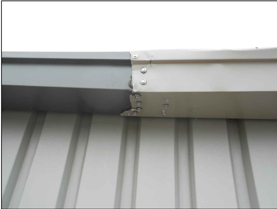
PHOTO_15: VIEW OF DAMAGED GUTTER TEMPORARY REPAIR
