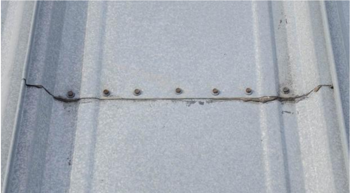
Photo 9: Typical head / end lap seam in the metal roof system.
