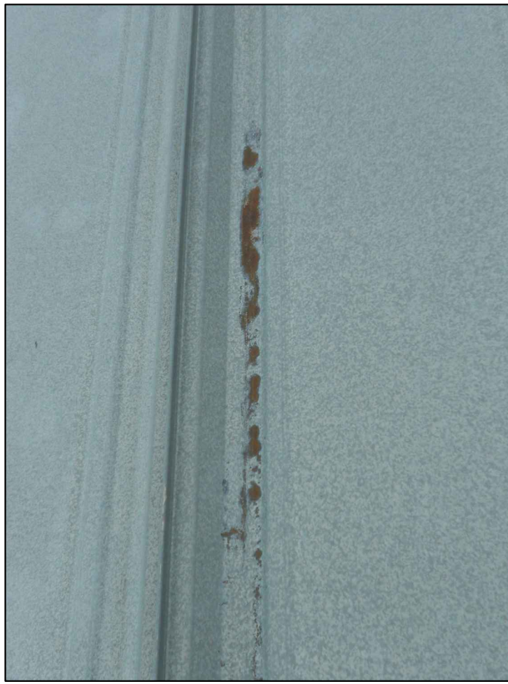
PHOTO_13: TYPICAL ROOF DECK CORROSION
