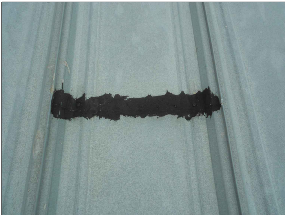
PHOTO_5: TYPICAL END LAP WITH ASPHALT MASTIC
