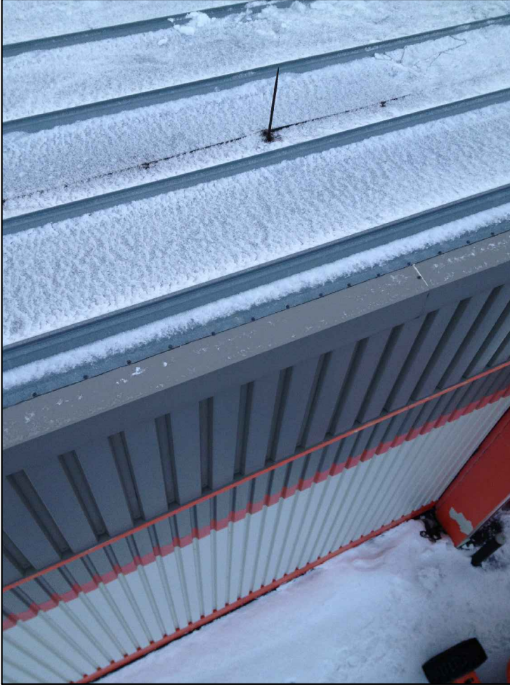
PHOTO_16: TYPICAL ROOF INSTALLATION AT (SIDE) PERIMETER OF ROOF DECK. SEE 3/R1.
