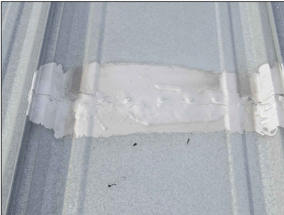
PHOTO_4: TYPICAL END LAP WITH ALUMINUM PAINT
