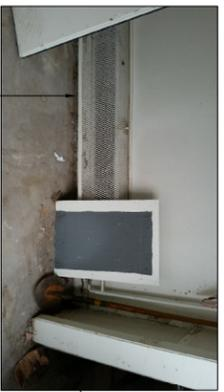
REMOVE AND REPLACE EXISTING ENTRANCE HOT WATER HEATER. RE-CONNECT PIPING AS REQUIRED TO NEW HEATER.
