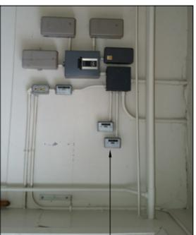
REMOVE ALL EXISTING ELECTRICAL AND ASSOCIATED EQUIPMENT BACK TO MAIN PANEL AND TERMINATE. WALL TO BE PATCH/REPAIRED/PAINITED TO COLOUR SELECTION BY OWNER.
