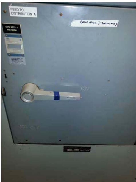
Existing disconnect feeding Distribution A
