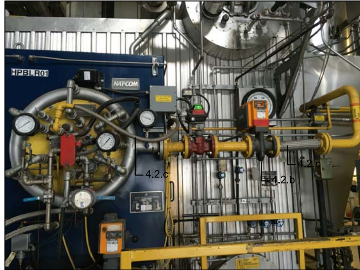
6 MOB BOILER#1 MISCELLANEOUS GAS TRAIN REPLACEMENTS SPECIFICATION 23 00 00, ARTICLE 4.2.b & 4.2.c
