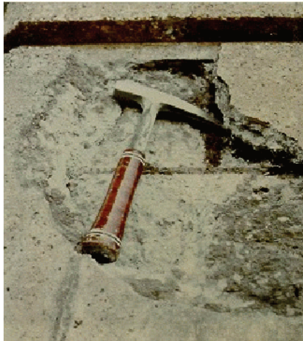
Figure 2.2.6(b) Severe Localized Spalling
