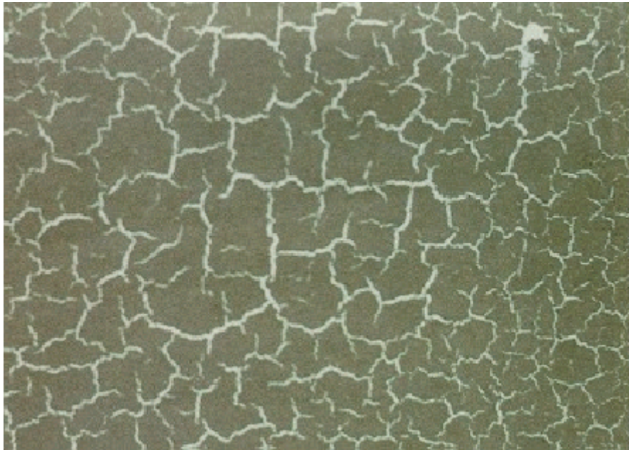
Figure 2.8.1(c) Alligatoring (typical mud crack pattern)
