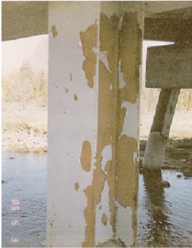
Figure 2.8.2(c) Intercoat Delamination
