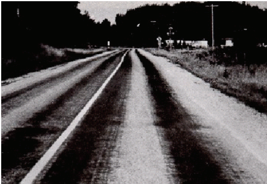
Figure 2.7.8 Slippery Surface
