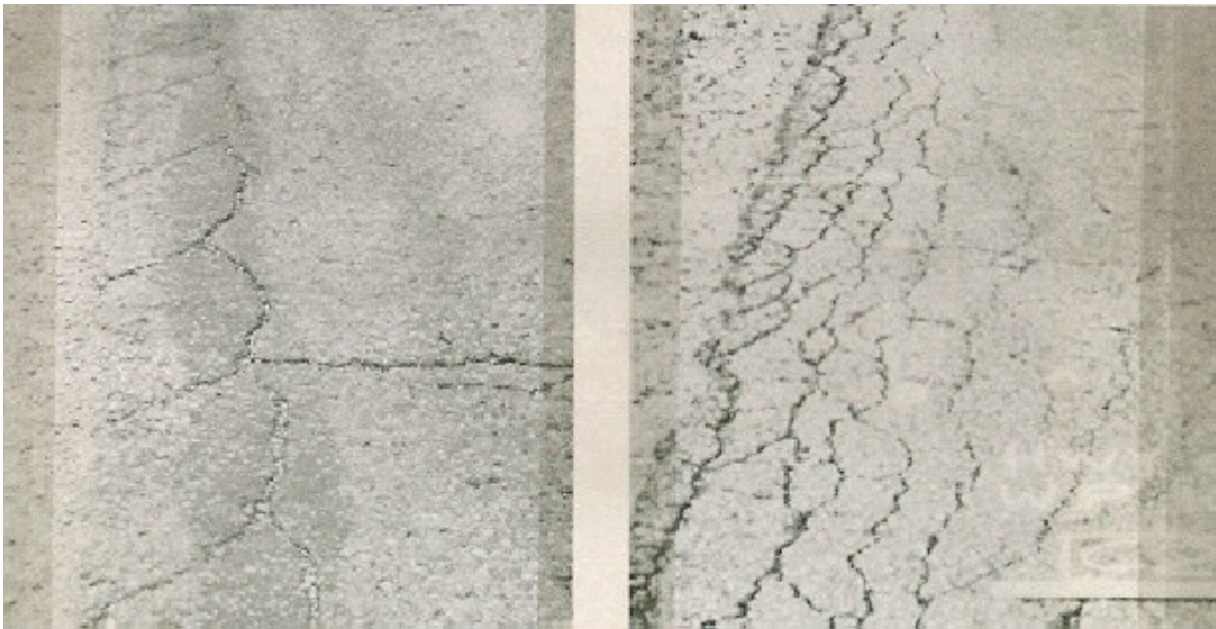
Figure 2.7.1(e) Medium Progressive Edge Cracks
