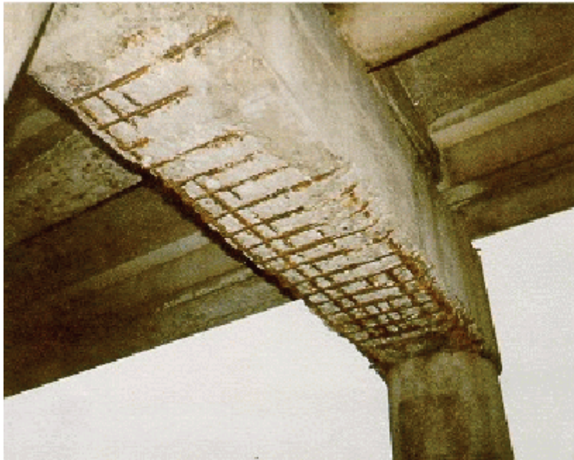
Figure 2.2.6(a) Very Severe Spalling in a Concrete Pier Cap due to Corrosion of Reinforcement
