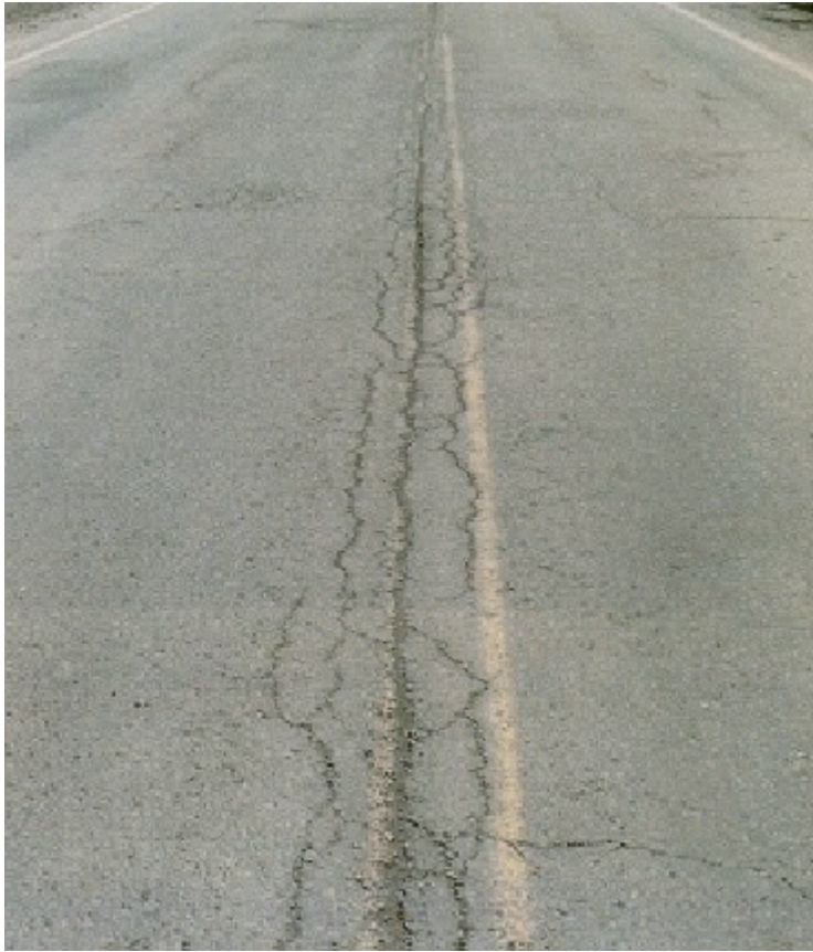
Figure 2.7.1(a) Medium Longitudinal Crack
