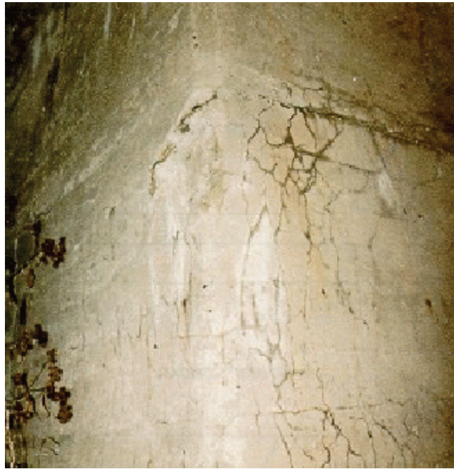
Figure 2.2.7(c) Medium Pattern Cracks in an Abutment
