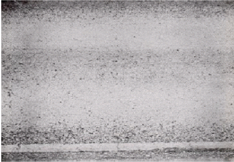
Figure 2.7.7 Severe Flushing
