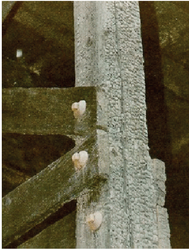
Figure 2.4.6(a) Medium Fire Damage on Wood
