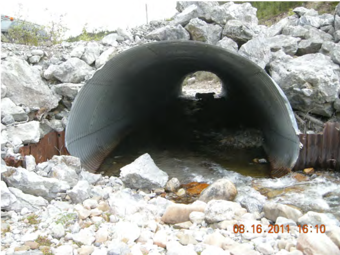
P04 - South Barrel - Inlet and East Embankment
