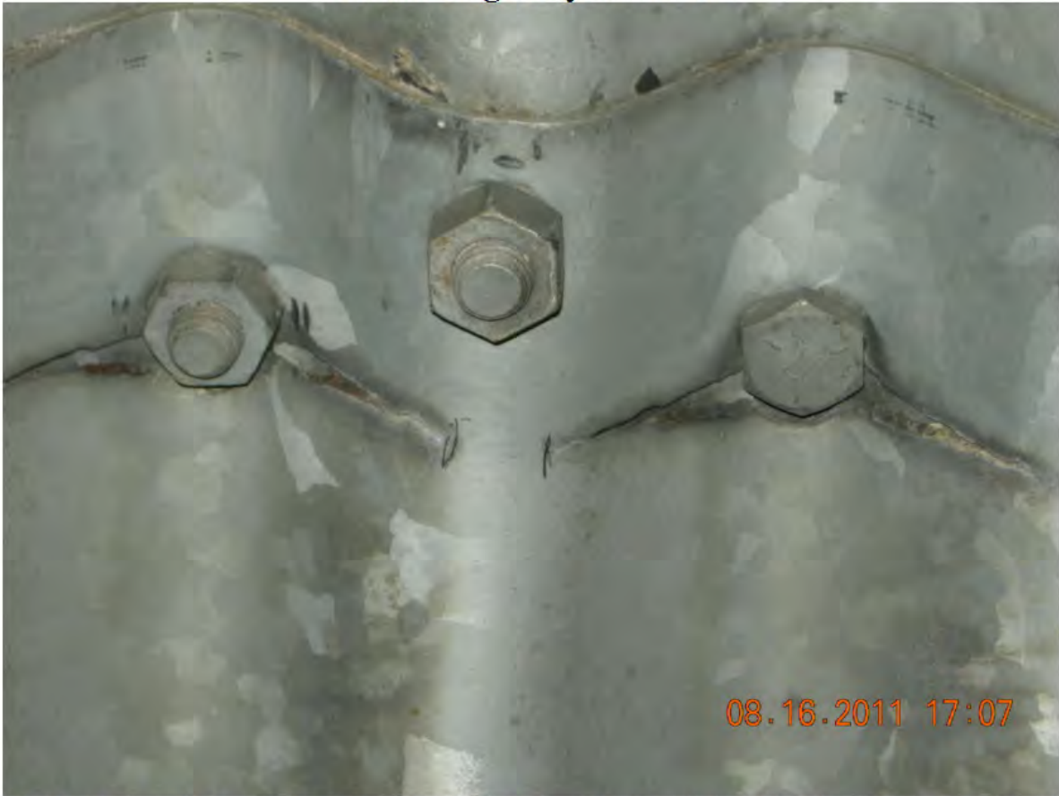
P17 - North Barrel - Longitudinal Cracking in Both Barrels - Ring 4 @ 4:30 - 23 mm Remaining Section
