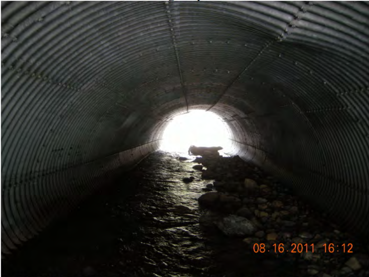
P07 - South Barrel - Looking Towards Outlet - Most Flow on South Side - Debris on North Side
