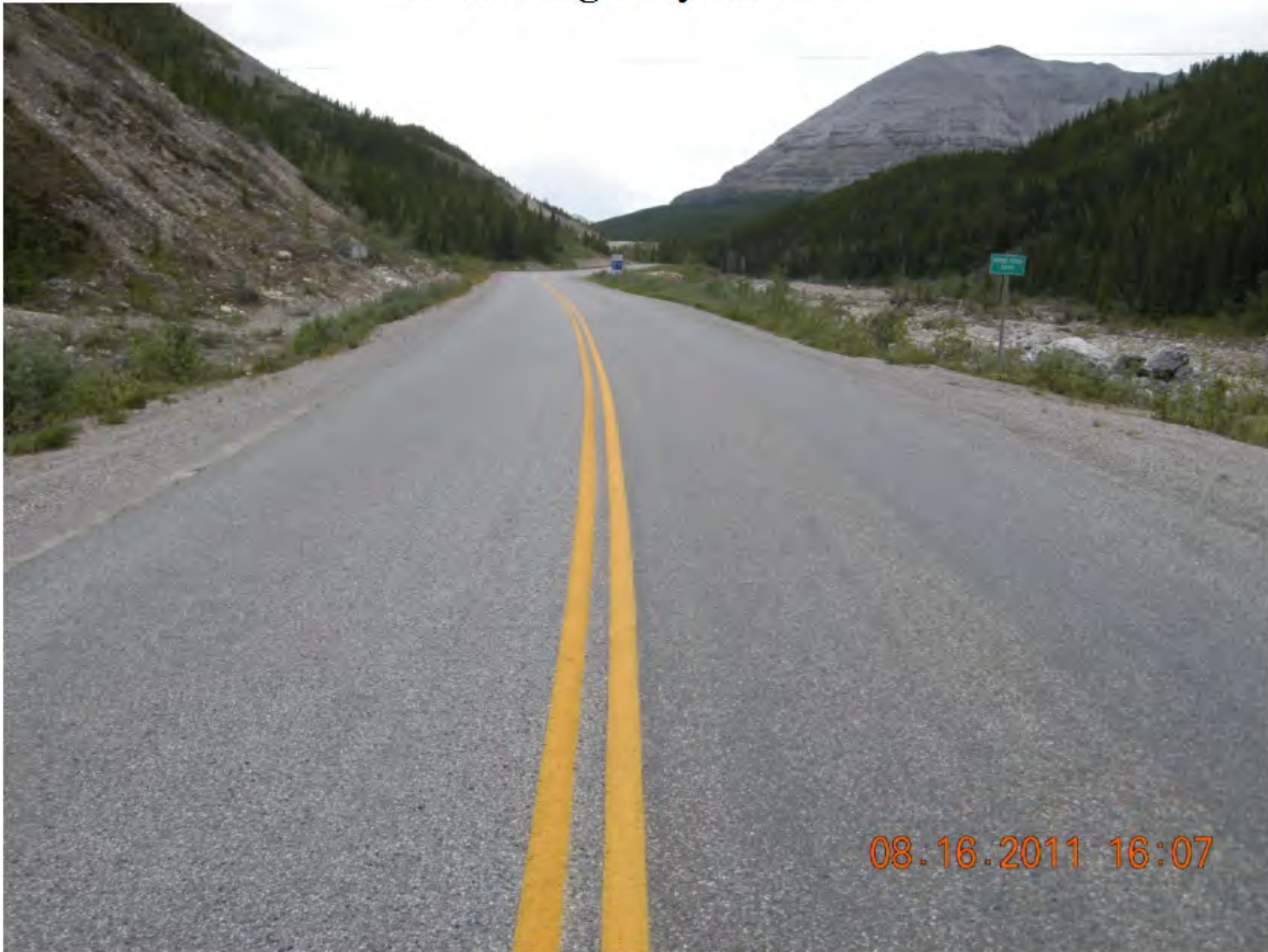
P01 - Roadway Looking North
