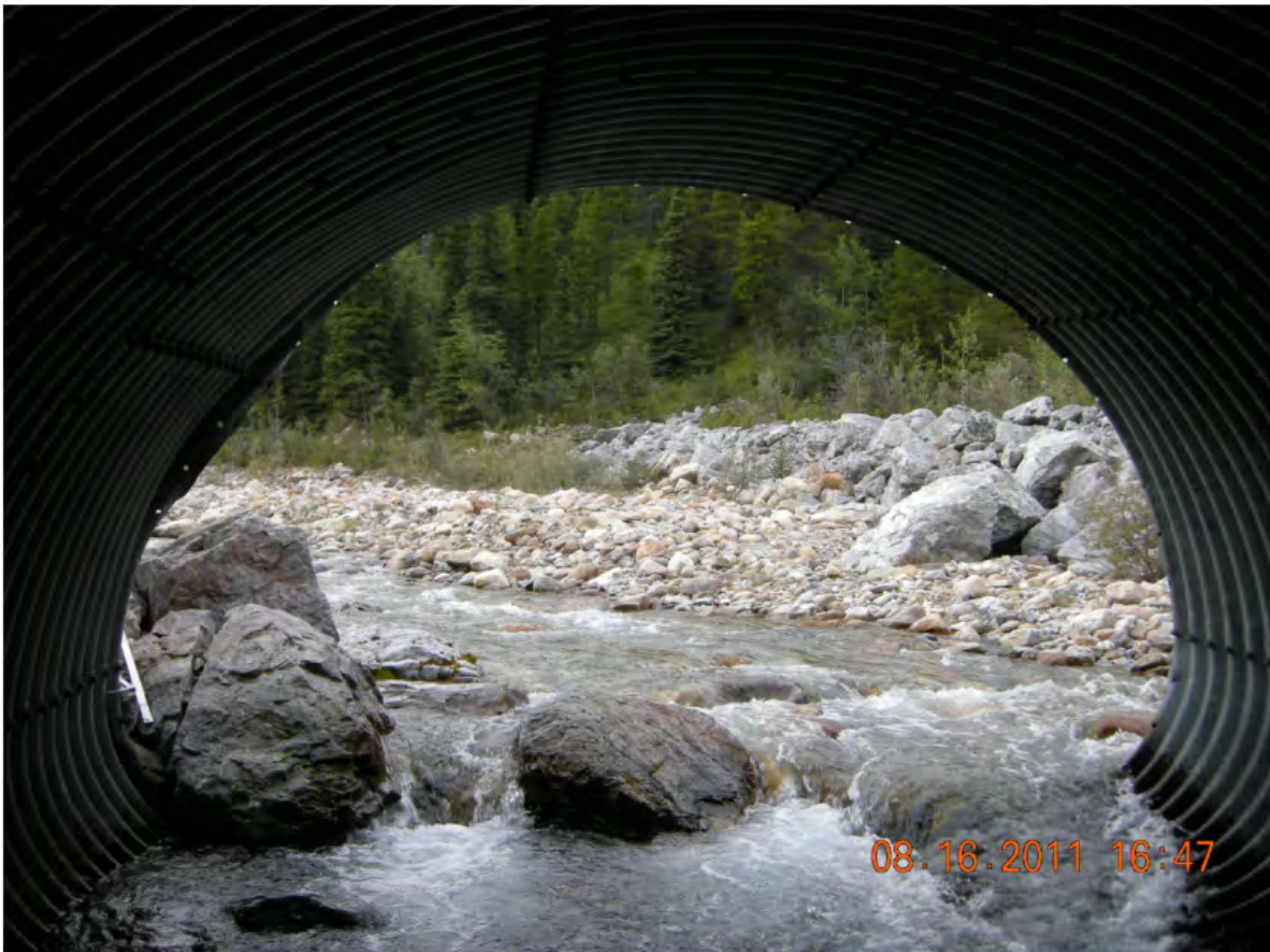
P12 - North Barrel - Inlet Watercourse - Large Riprap in Watercourse
