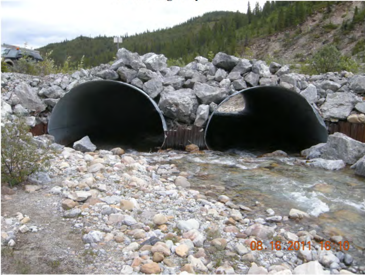
P03 - Inlets and East Embankment
