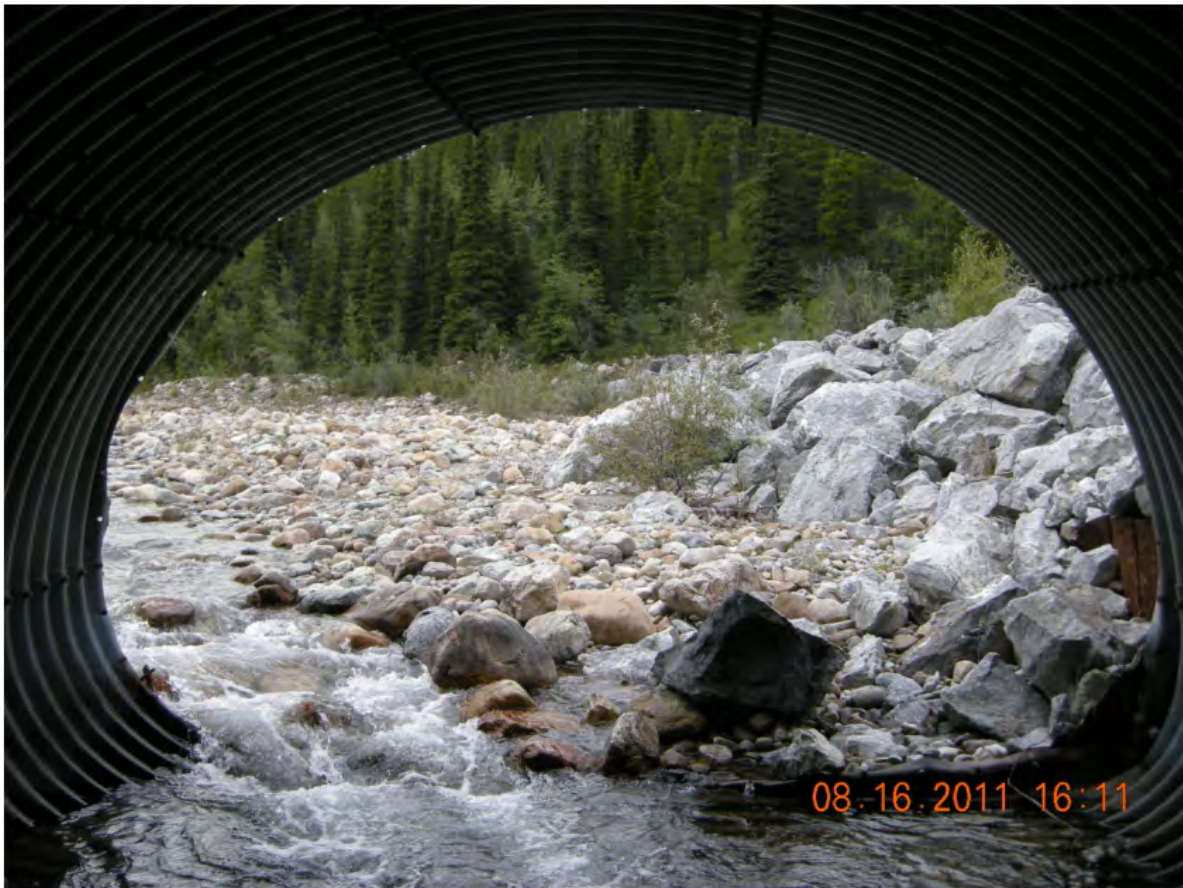
P06 - South Barrel - Inlet Watercourse to North of Inlet
