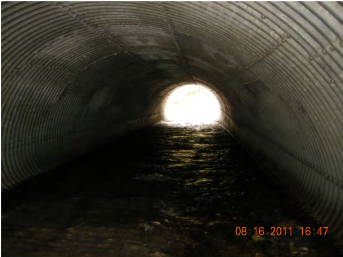
P14 - North Barrel - Looking Towards Outlet
