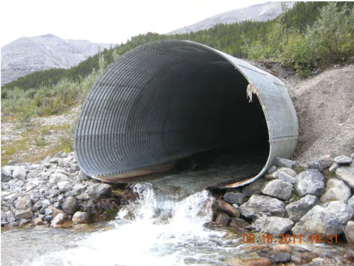
P18 - North Barrel - Outlet - Floor has Drooped Down ~400 mm in Both Barrels
