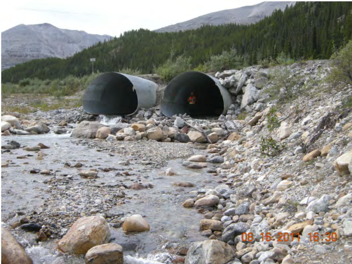
P20 - Outlets and West Embankment
