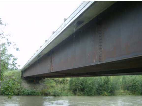
Figure 5: Exterior of Box Girder.
