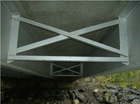
Figure 10: Intermediate Bracing.
