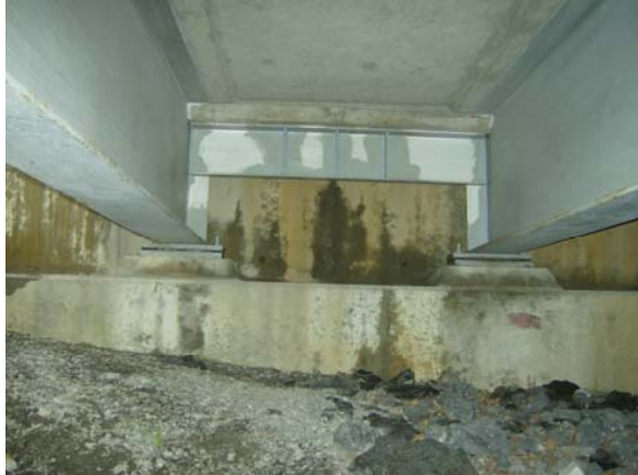
Figure 11: End Bracing.
