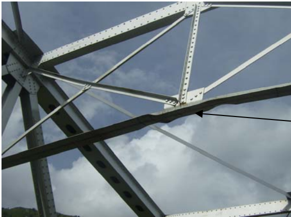
Figure 17: Typical Intermediate Sway Frame Lateral Bracing.
