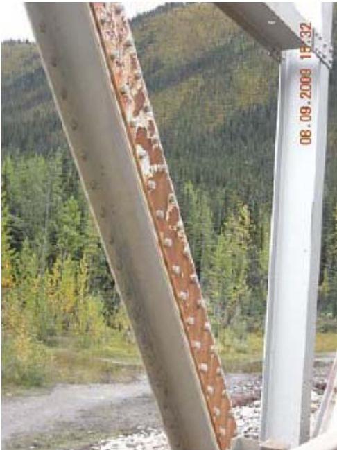
Figure 14: Previously Strengthened Diagonal Compression Truss Member.
