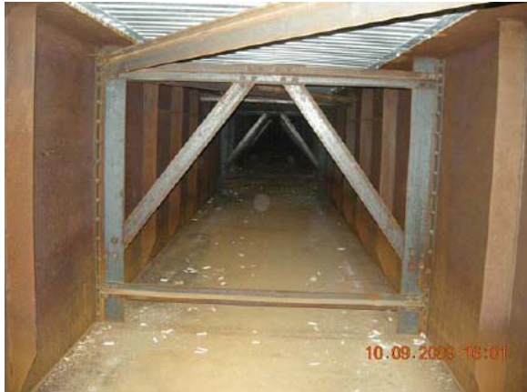
Figure 12: Typical Diaphragm Inside of Box Girder.
