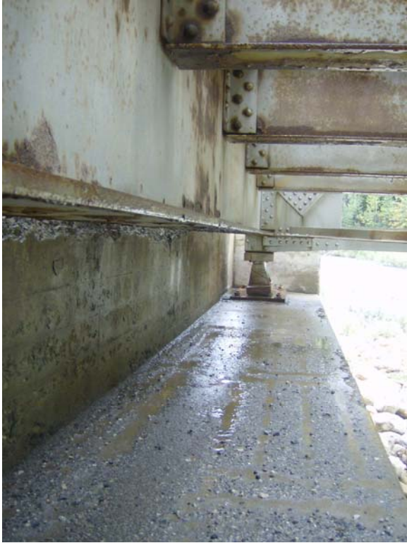
Figure 7: Truss Bearing.
