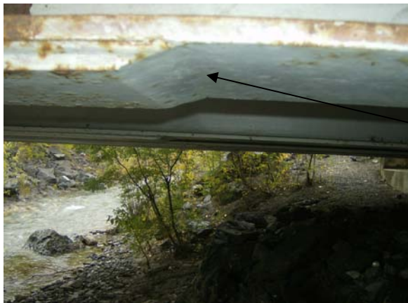
Figure 6: Plates Welded to Girder Bottom Flanges.
