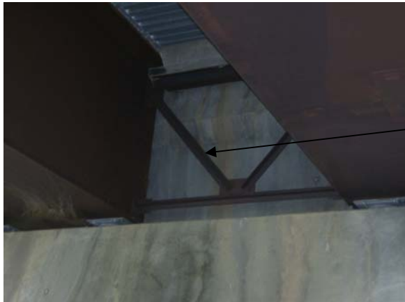
Figure 11: North End Bracing.
