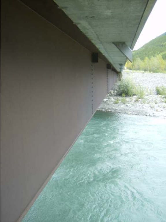
Figure 5: Exterior of Box Girder.
