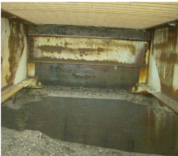
Figure 24: Jackspan End Bracing.
