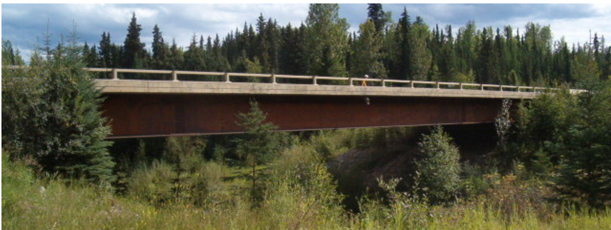
Figure 1: Steamboat Creek Bridge Photo.
