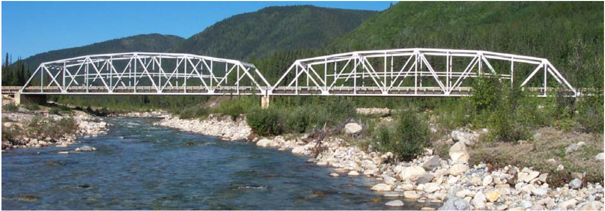
Figure 1: Tetsa River Bridge #1 Photo.
