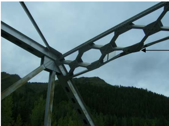
Figure 16: Typical End Portal Lateral Bracing.
