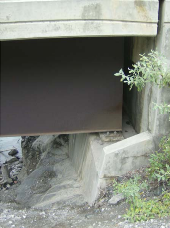
Figure 6: Box Girder Bearing.
