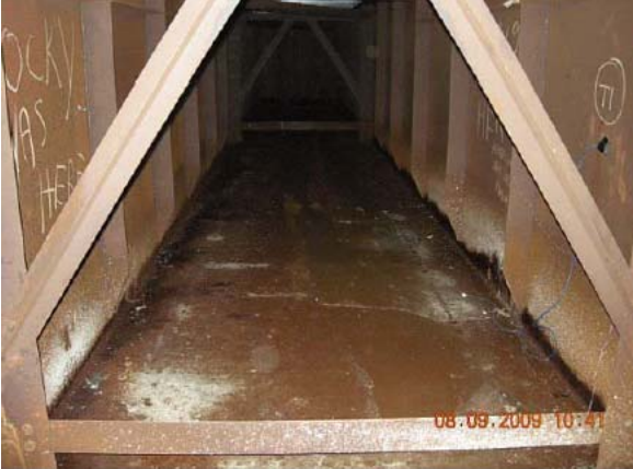
Figure 10: Typical Diaphragm Inside of Box Girder.
