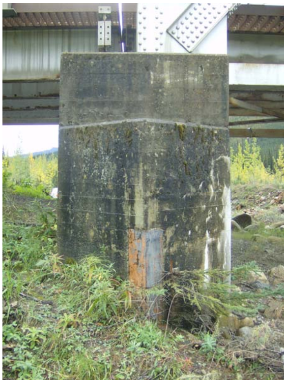
Figure 22: Jackspan to Truss-Span Pier.
