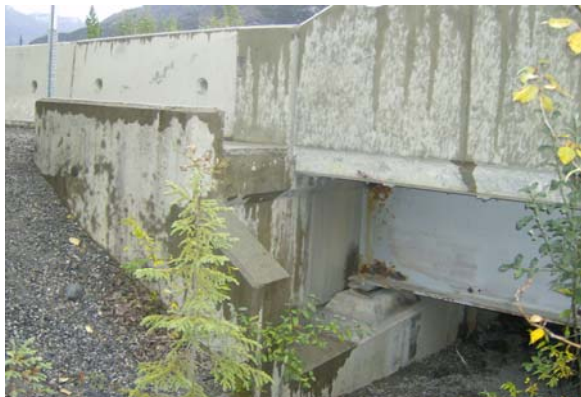
Figure 7: Abutment and Wingwall.
