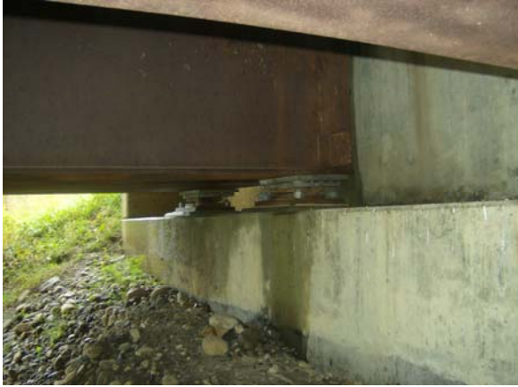
Figure 7: Box Girder Bearing.
