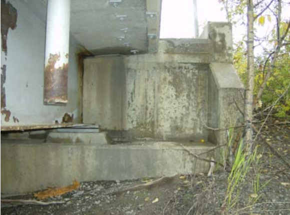
Figure 8: Exterior Girder Bearing.
