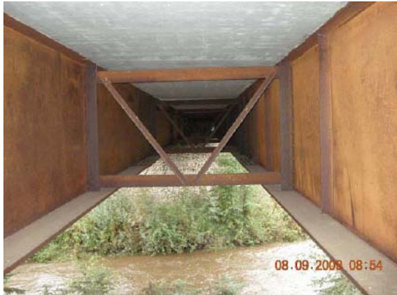
Figure 9: Intermediate Bracing.
