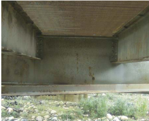
Figure 9: Stringer to Floor Beam Connections.
