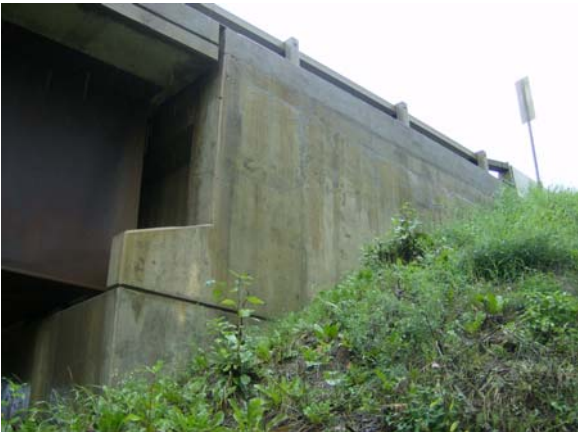
Figure 6: Abutment and Wingwall.
