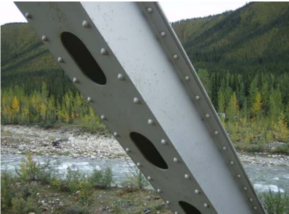
Figure 13: Top Chord Truss Member.
