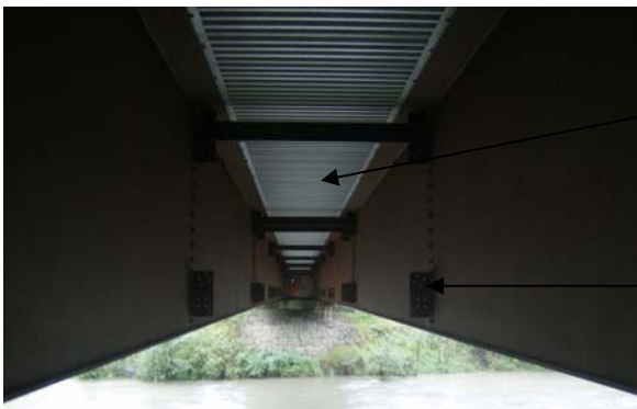
Figure 7: Box Girder Bearing.
