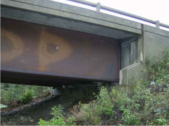
Figure 7: Exterior Girder Bearing.
