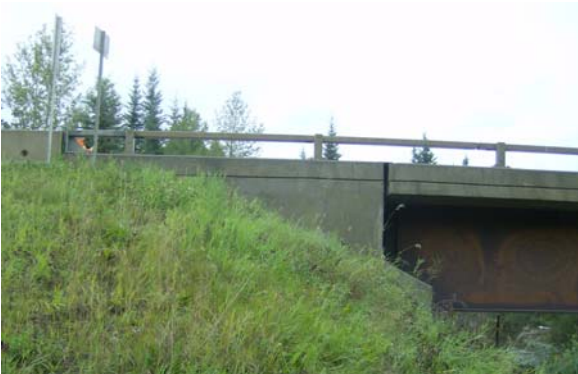
Figure 6: Abutment and Wingwall.
