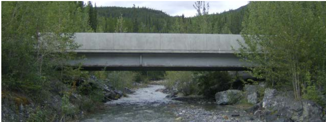
Figure 1: Petersen Creek Bridge Photo.
