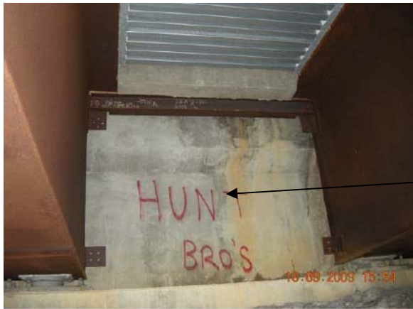
Figure 10: South End Bracing.
