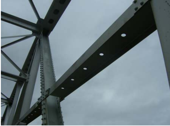
Figure 15: Vertical and Diagonal Truss Member Horizontal Bracing.
