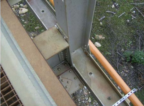
Figure 12: Bottom Chord and Vertical Truss Members.
