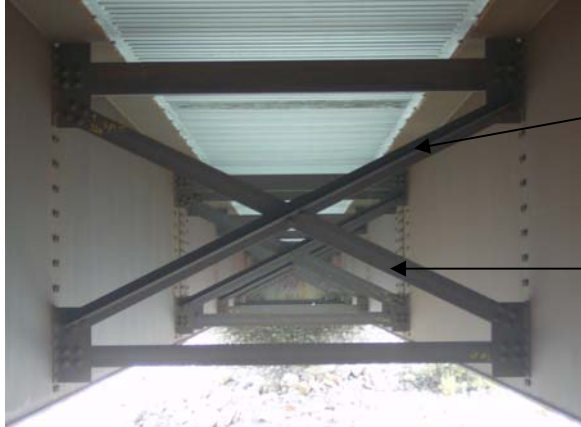
Figure 9: Intermediate Bracing.
