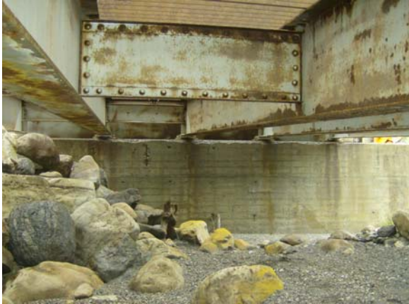
Figure 23: Jackspan Girder Lines and Intermediate Bracing.
