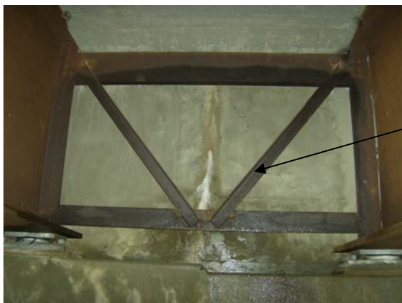
Figure 10: End Bracing.
