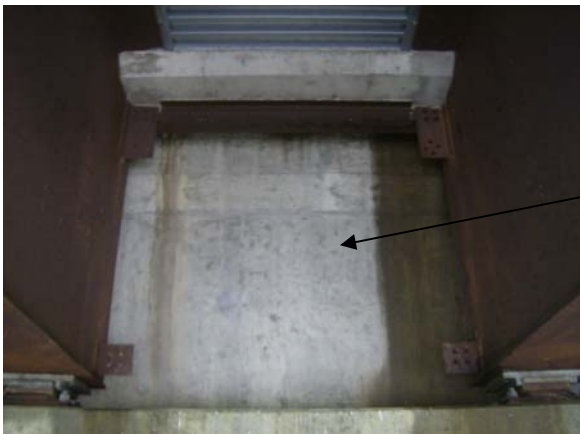
Figure 9: End Bracing.
