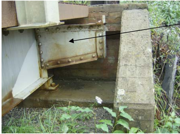
Figure 21: Exterior Jackspan Girder Bearing.
