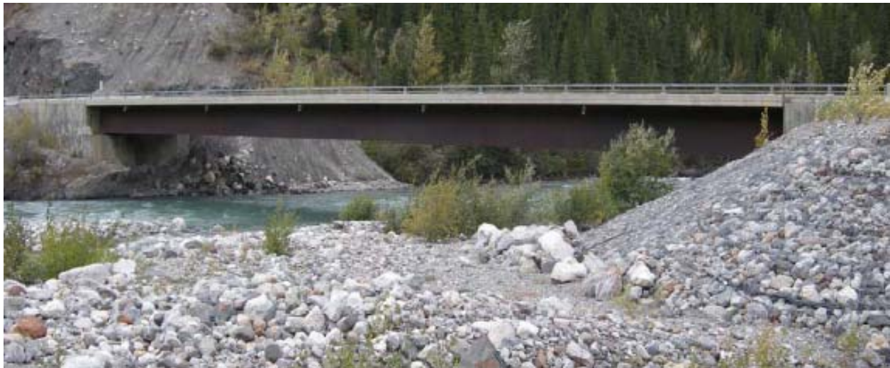
Figure 1: Toad River Bridge Photo.
