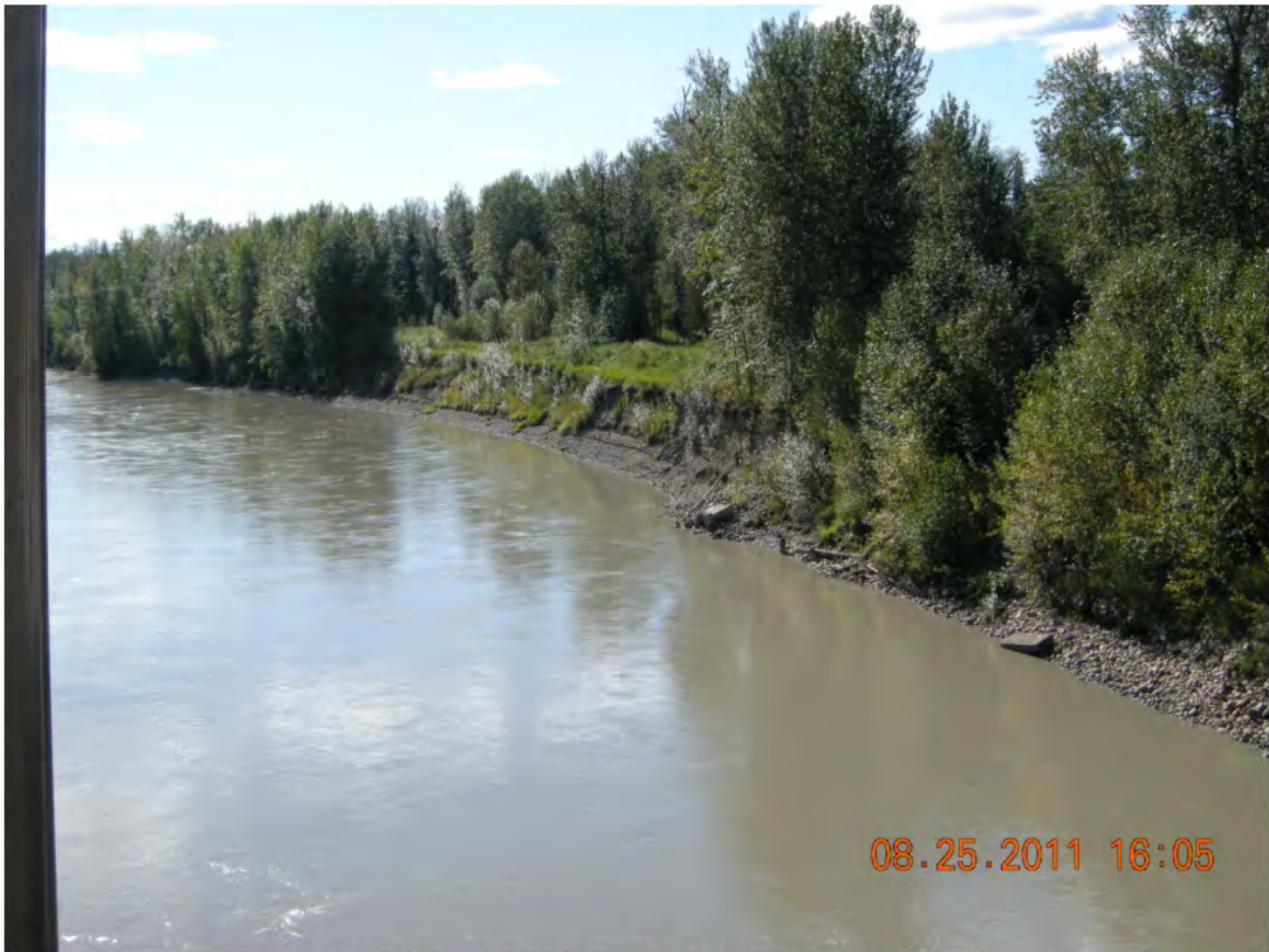
P06 - Erosion Upstream on the NW River Embankment
