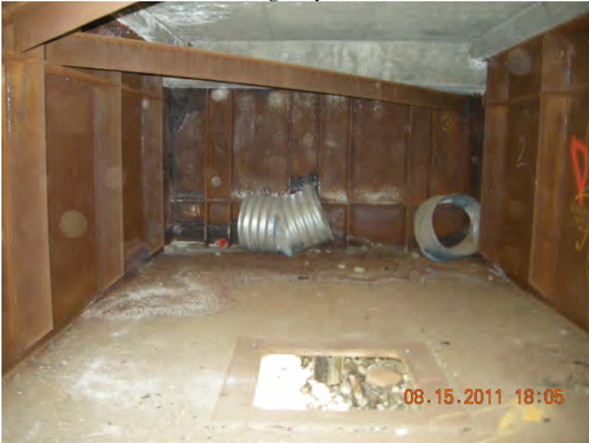
P55 - West Girder - Span 5 - North End
