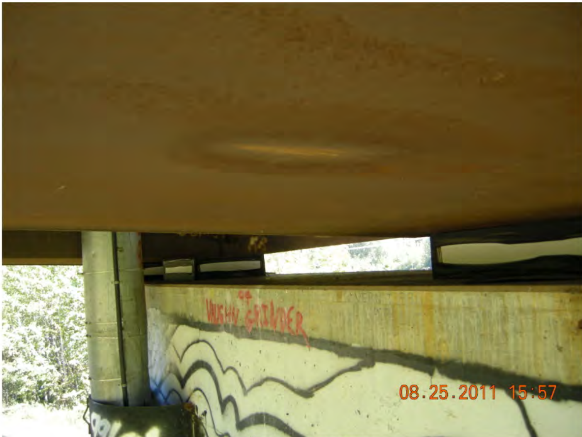
P74 - Pier 4 - Bearing Seat
