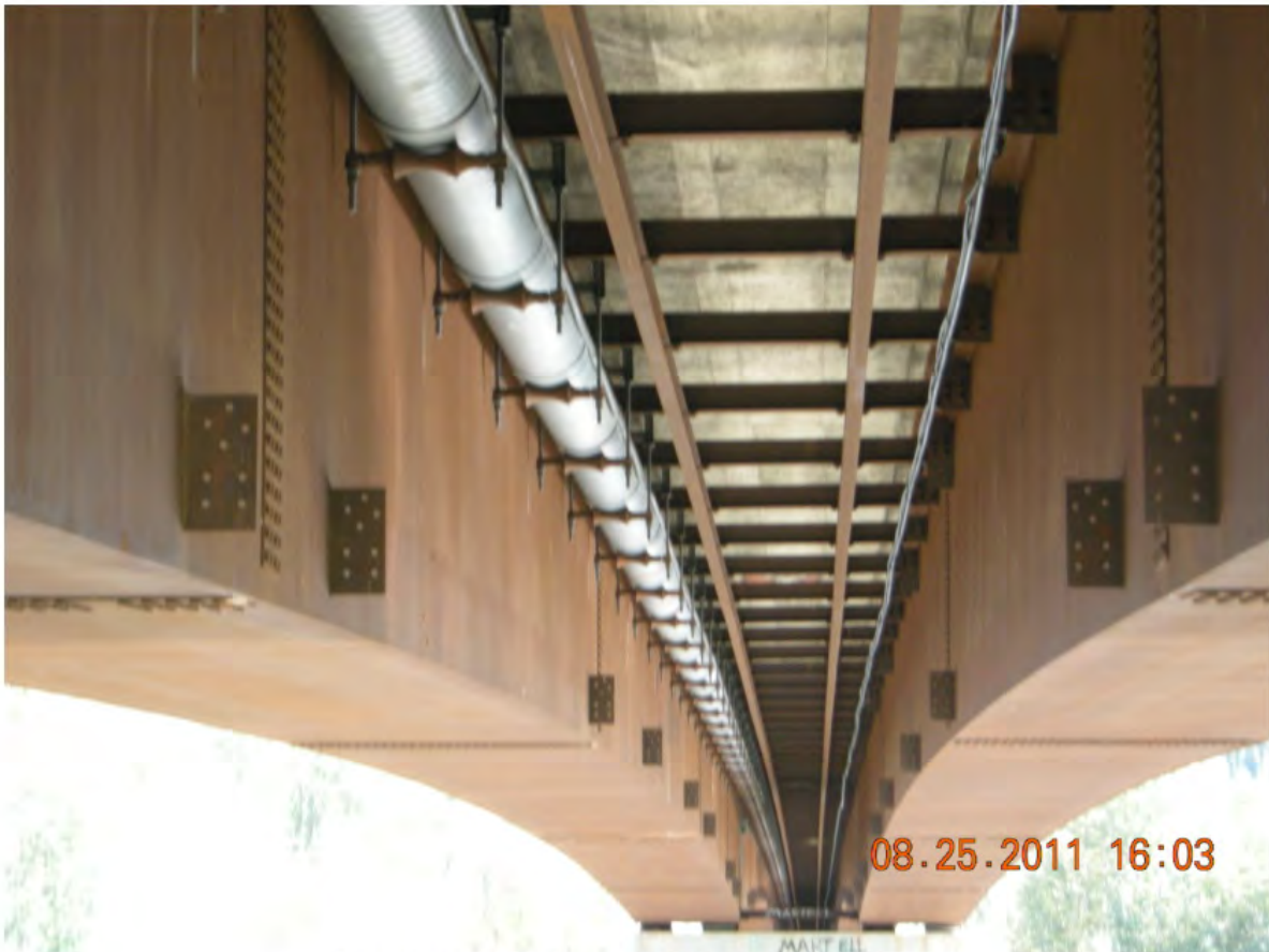
P34 - Span 4 Girders and Soffit - Looking South
