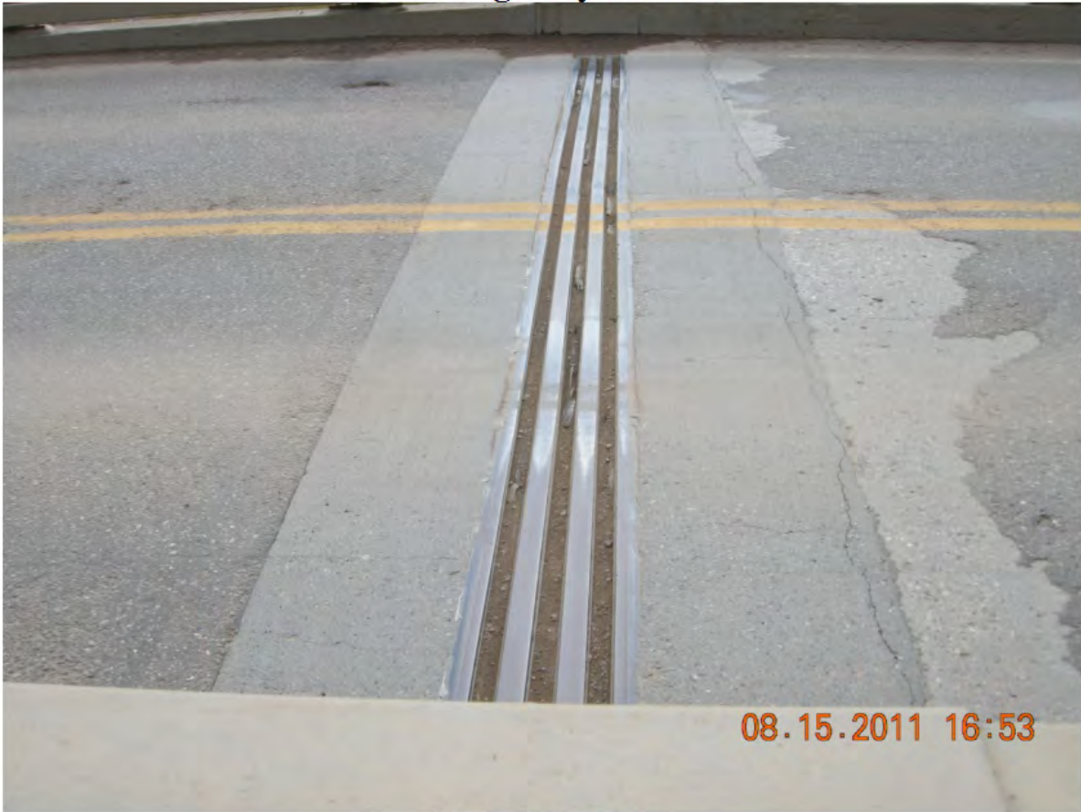
P13 - North Deck Joint
