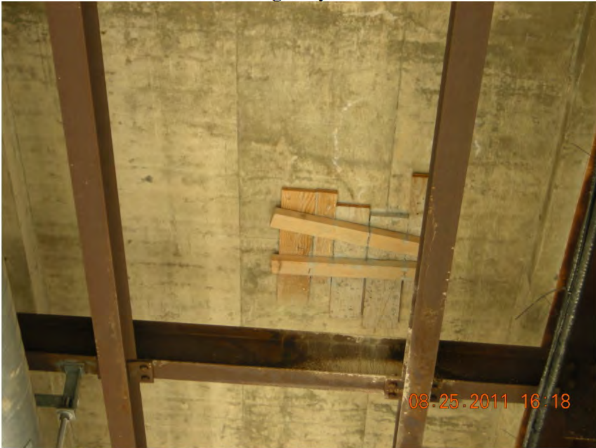
P31 - Span 3 - Soffit Patch near Midspan - Timber Formwork Still in Place
