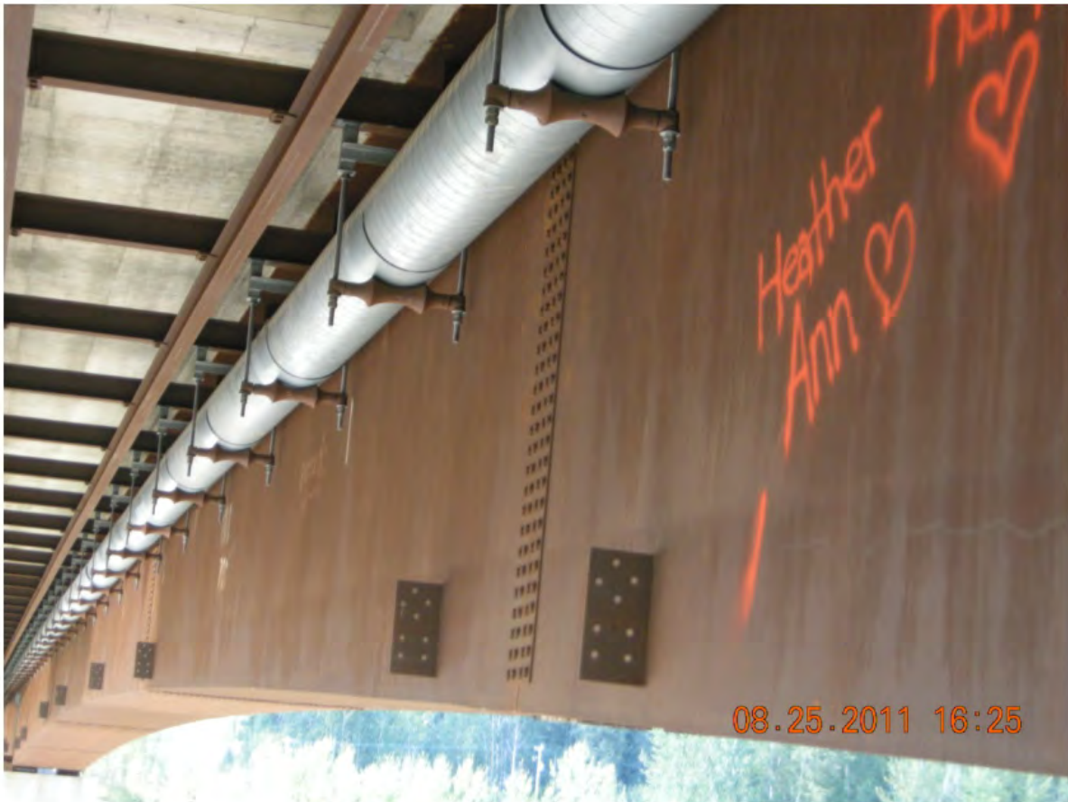
P26 - Span 2 - East Girder - Looking North
