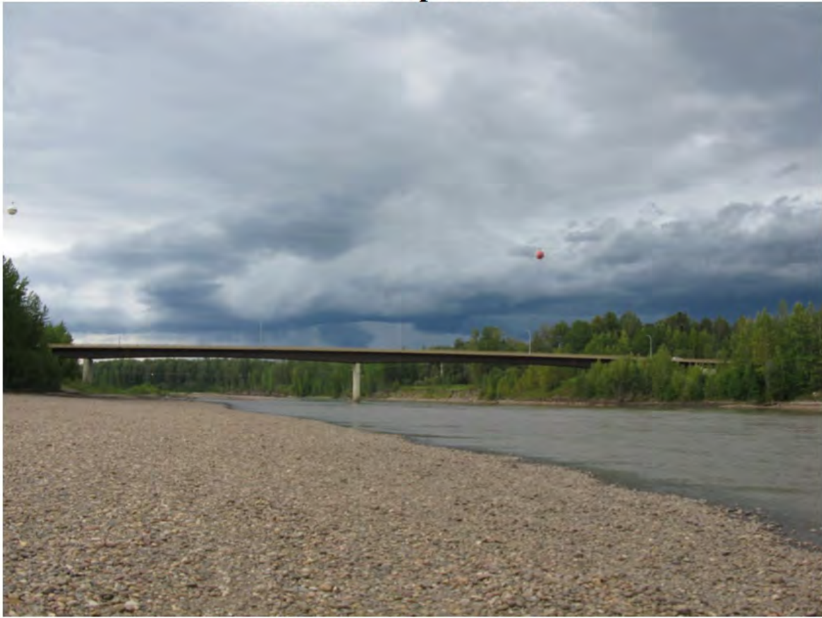
UW01 - Overall view looking US
