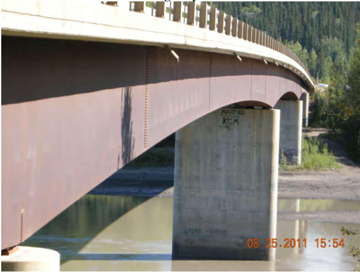
P05 - West Side - Looking South
