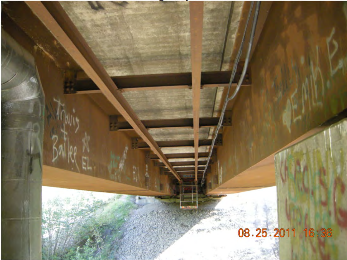
P25 - Span 1 and South Abutment
