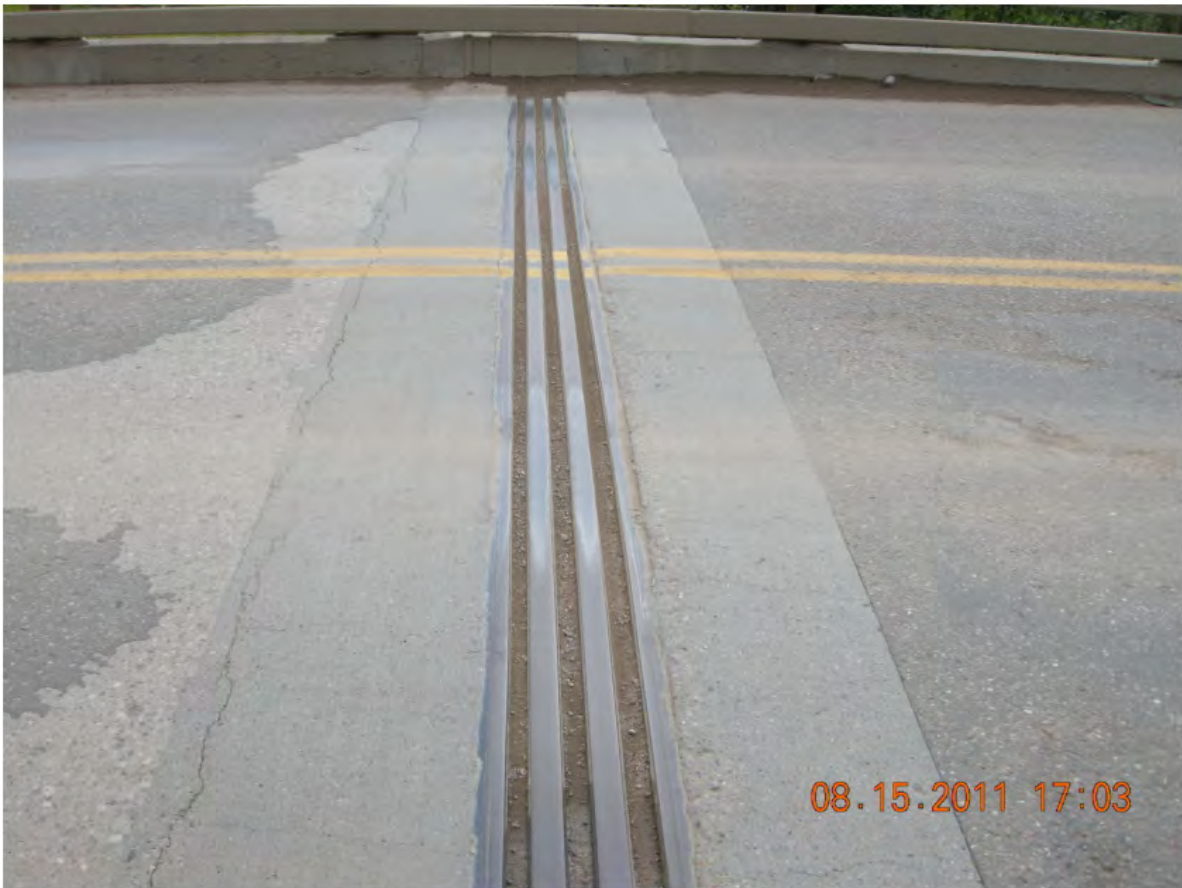
P12 - South Expansion Joint - Looking West
