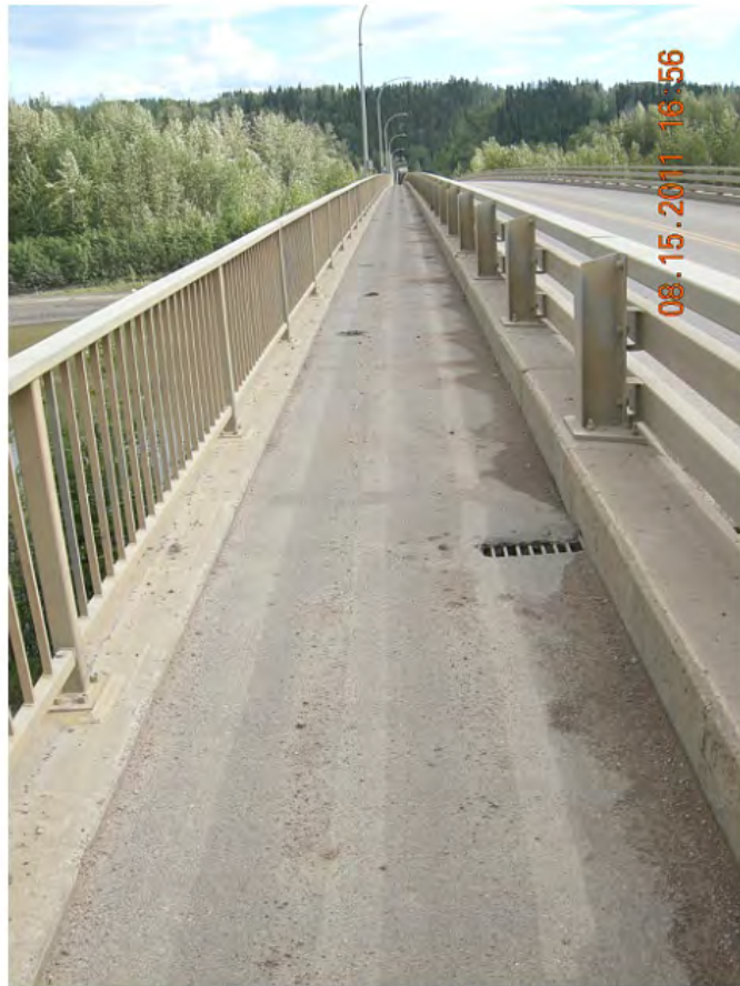
P10 - Sidewalk on East Side of Bridge
