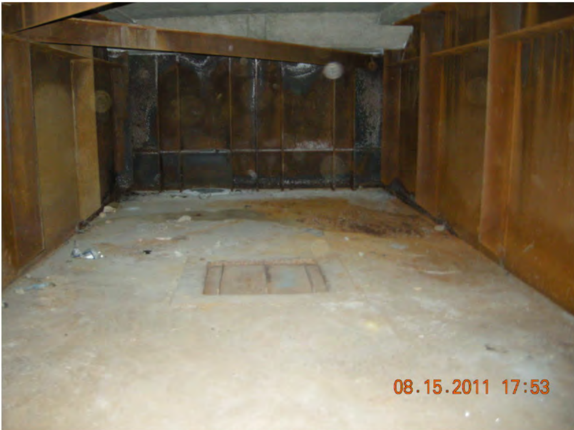
P40 - East Girder - Span 1 - South End
