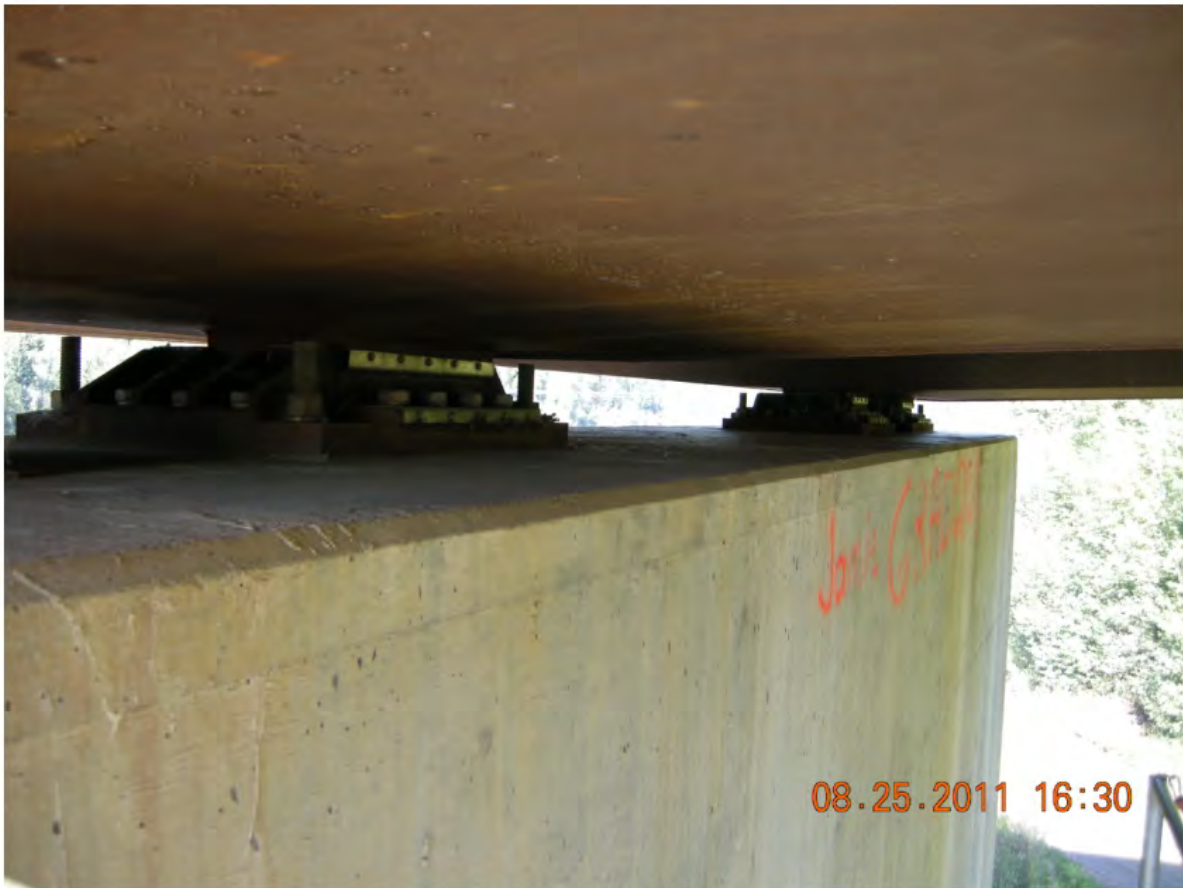
P68 - Pier 2 Bearings - All Uncladded
