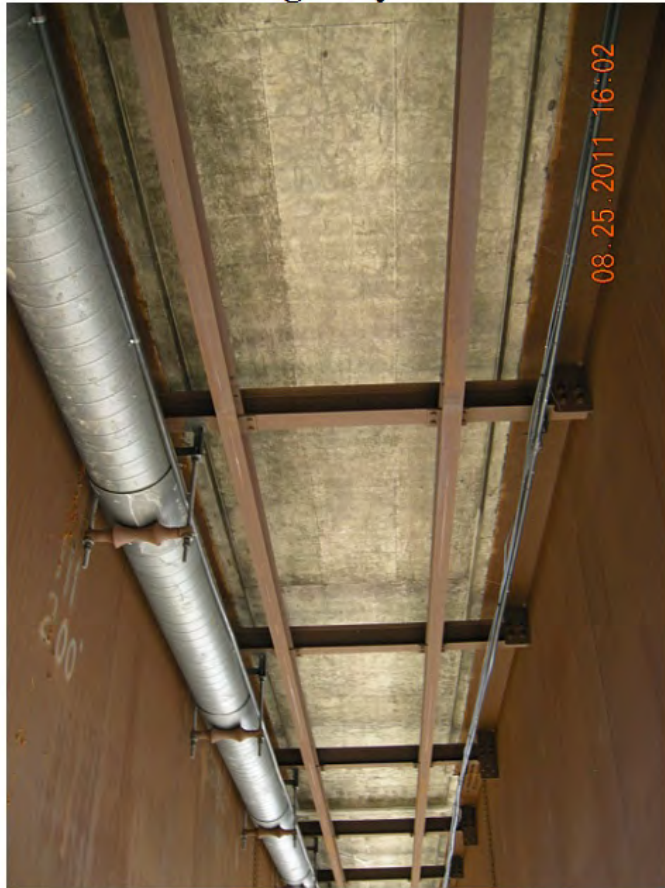
P35 - Span 4 Soffit - Utilities on Both Girders
