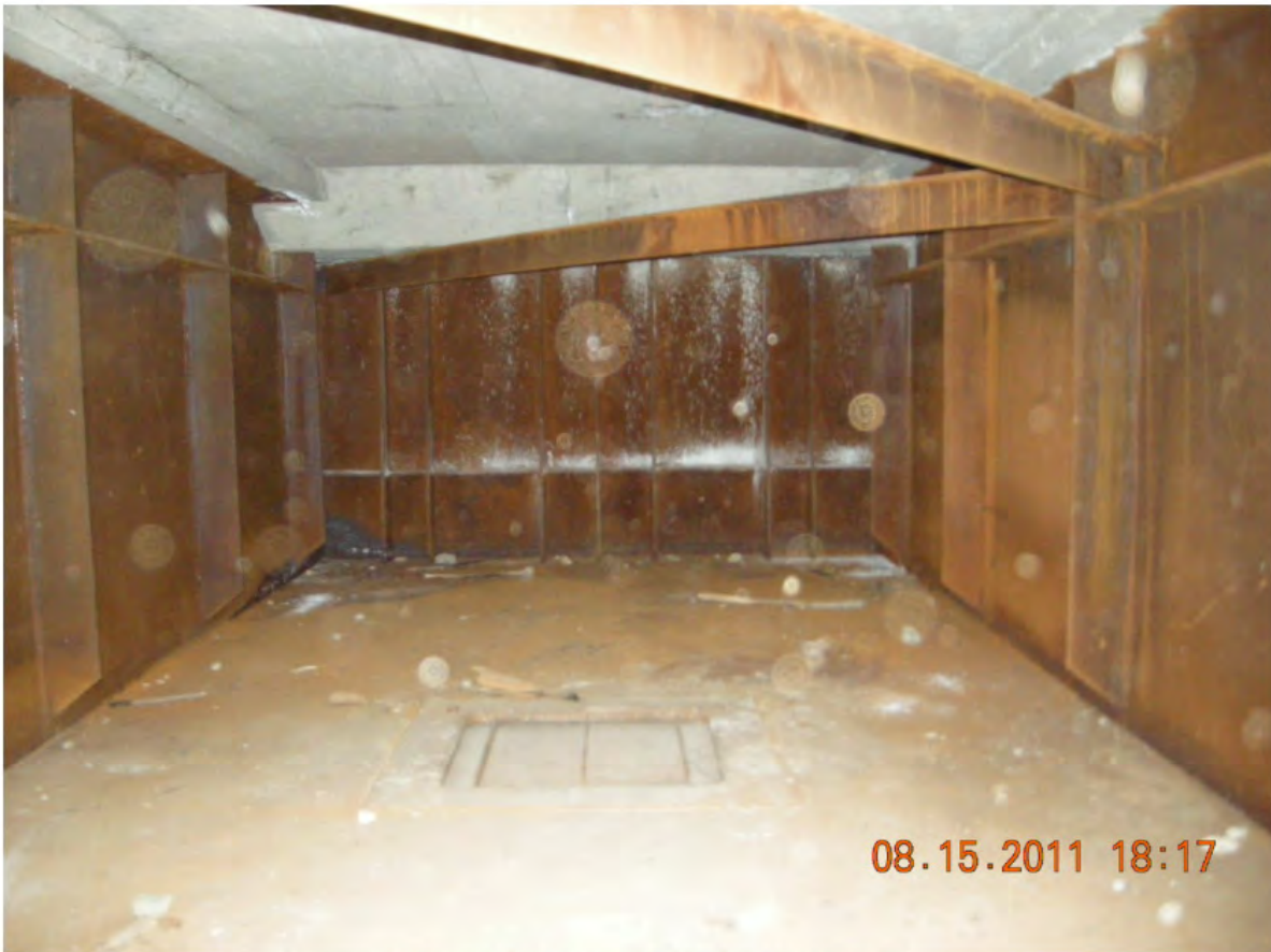
P50 - West Girder - Span 1 - South End
