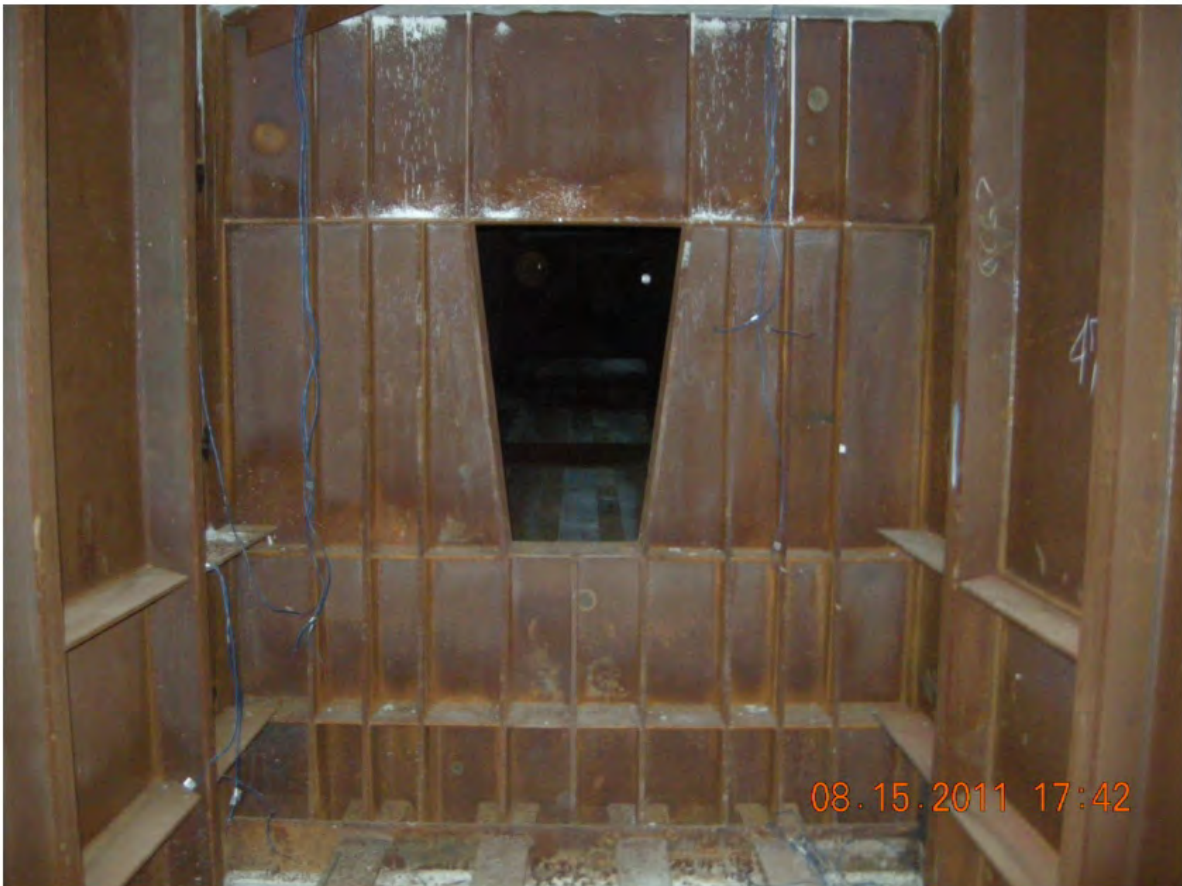
P46 - East Girder - Pier 4 Diaphragm
