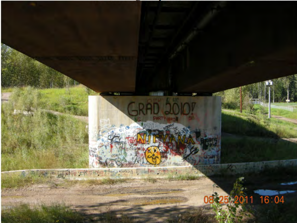
P73 - Pier 4 - South Side
