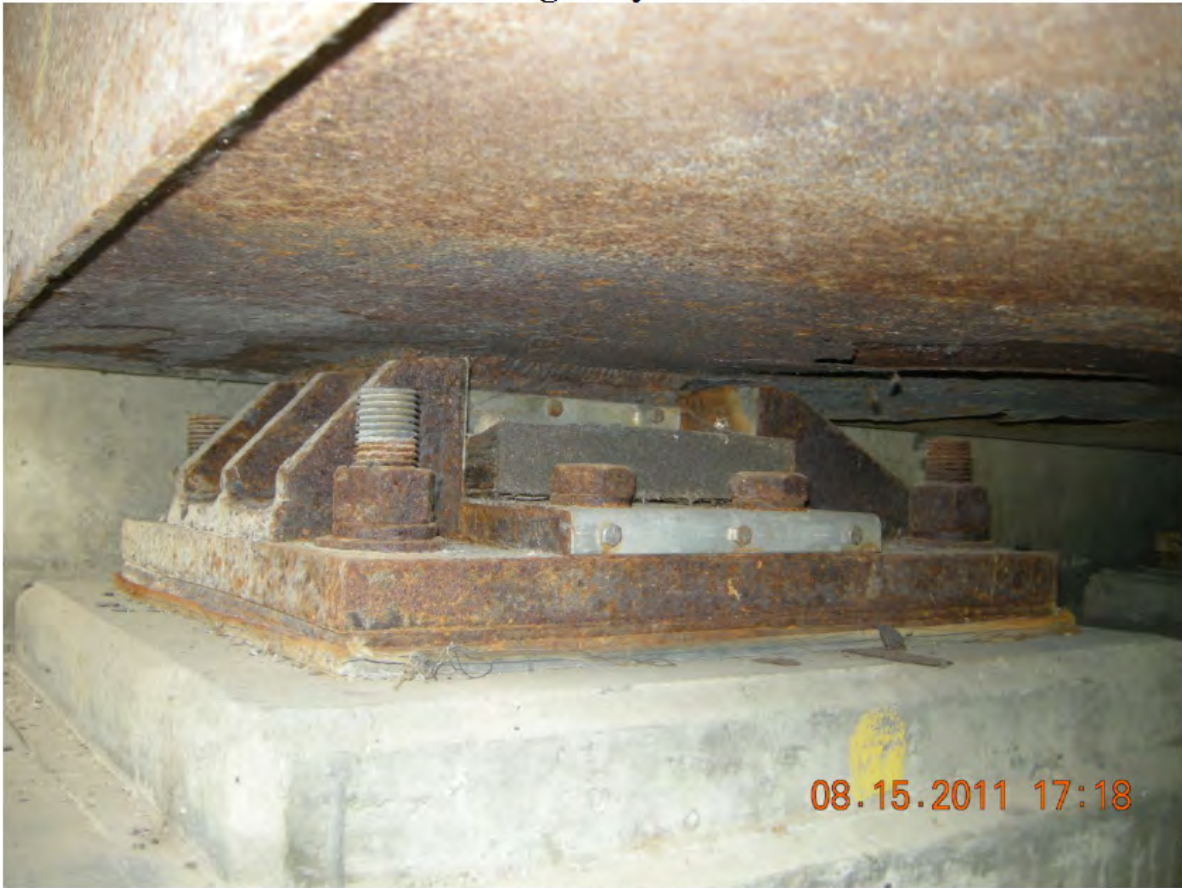
P59 - South Abutment - East Girder - East Expansion Bearing
