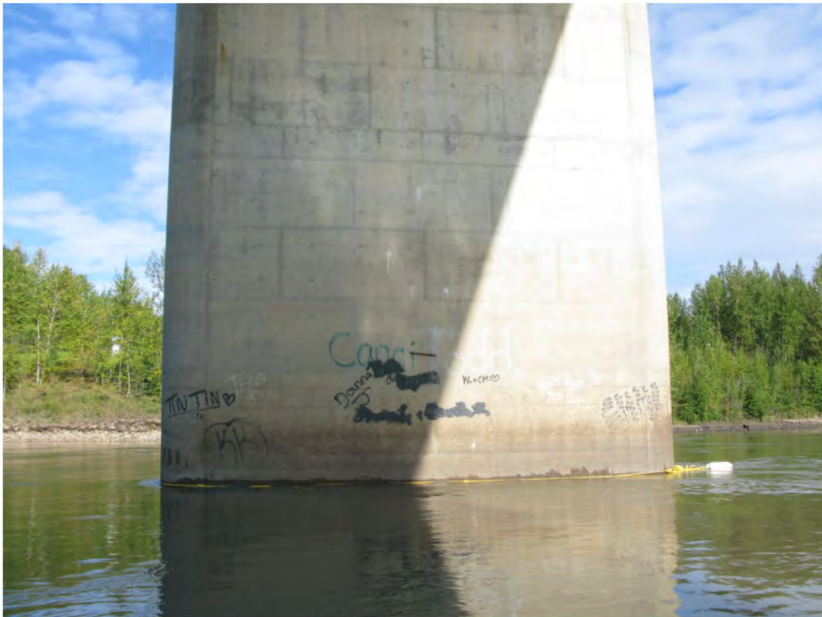
UW08 - Pier 3 LC face 2
