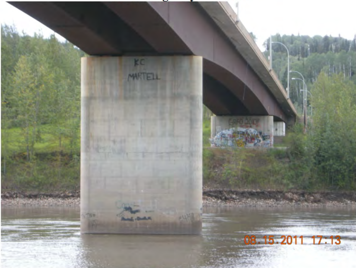
P69 - Pier 3 - South Face
