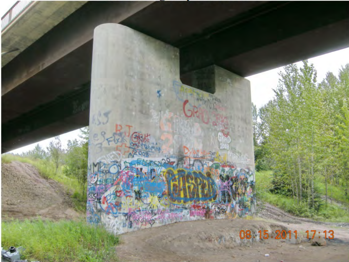
P61 - Pier 1 - North Face
