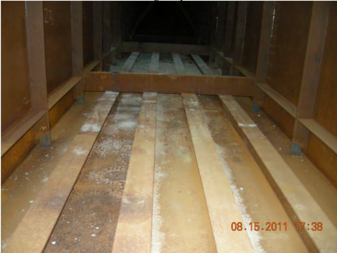
P47 - East Girder - Span 5 - Bottom Flange Stiffeners
