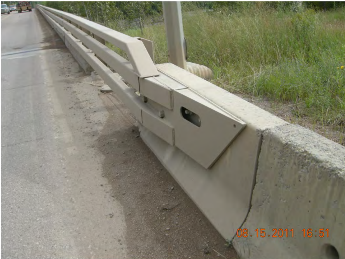
P22 - NW Bridge Railing - Concrete Approach Barrier Transition
