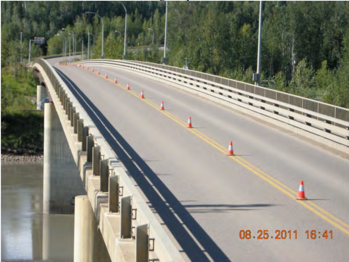
P09 - Overall Deck - Looking North
