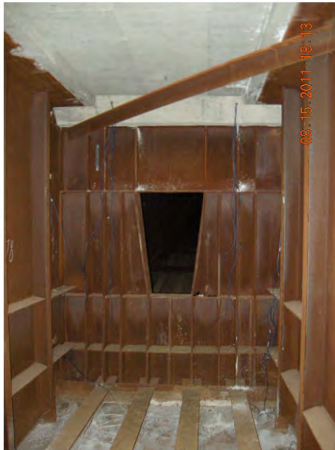
P52 - West Girder - Pier 2 Diaphragm
