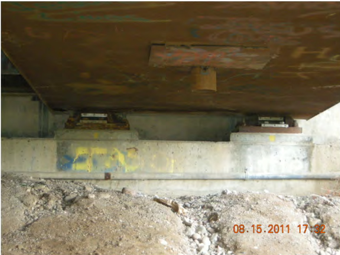
P78 - North Abutment - East Girder Bearings have Cladding Removed
