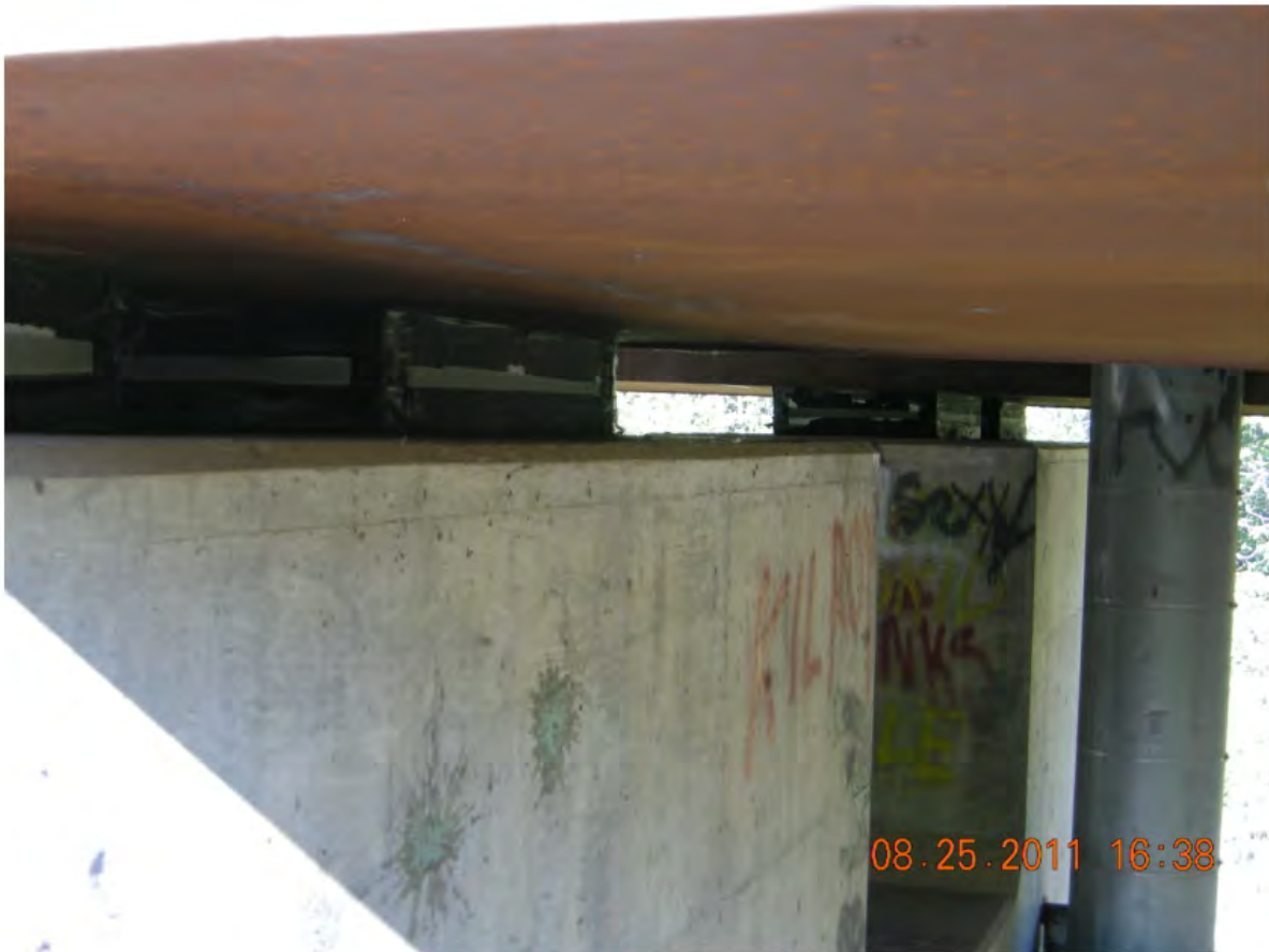
P62 - Pier 1 - Bearings and Seat
