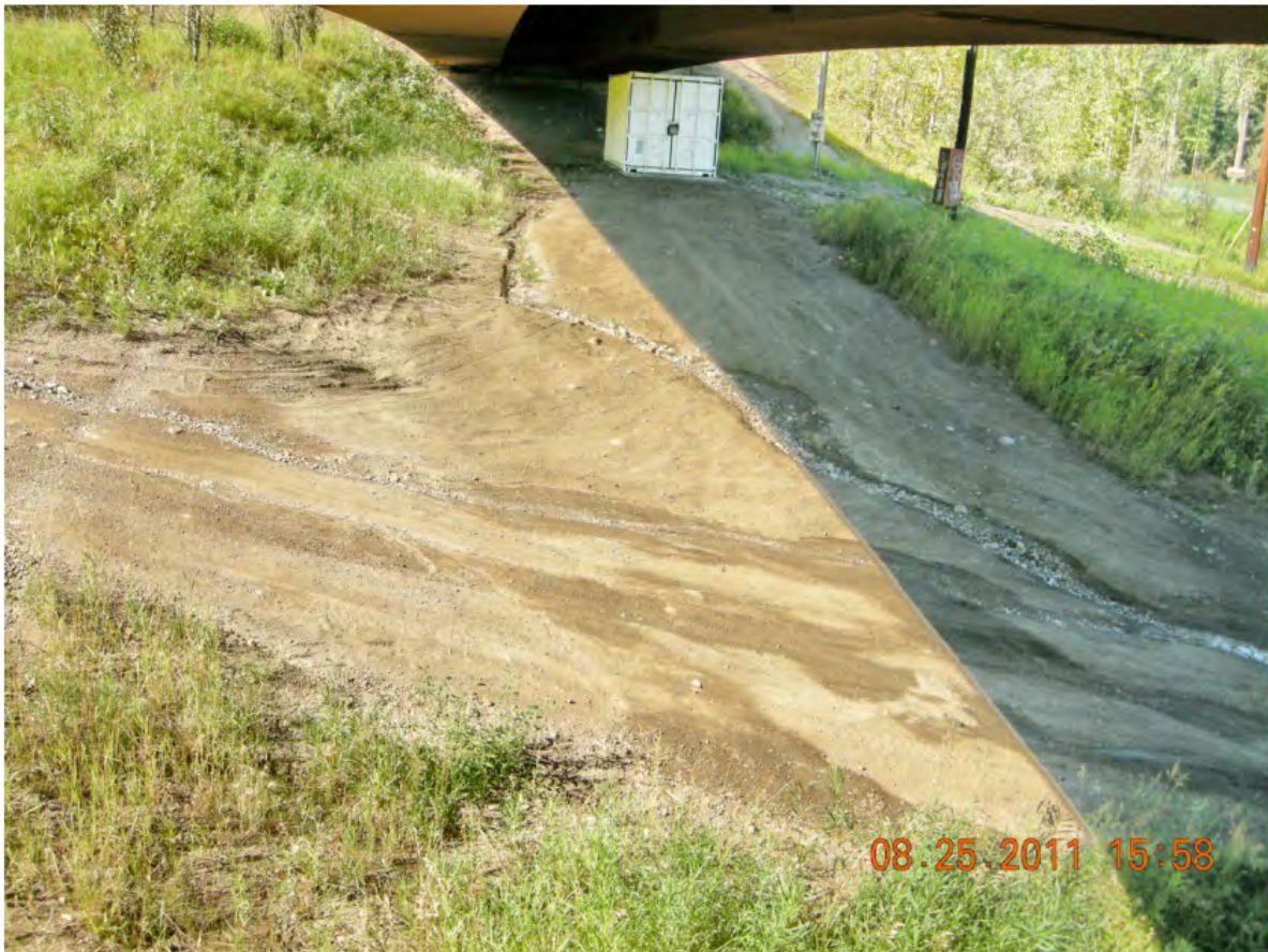
P76 - North Abutment and Embankment
