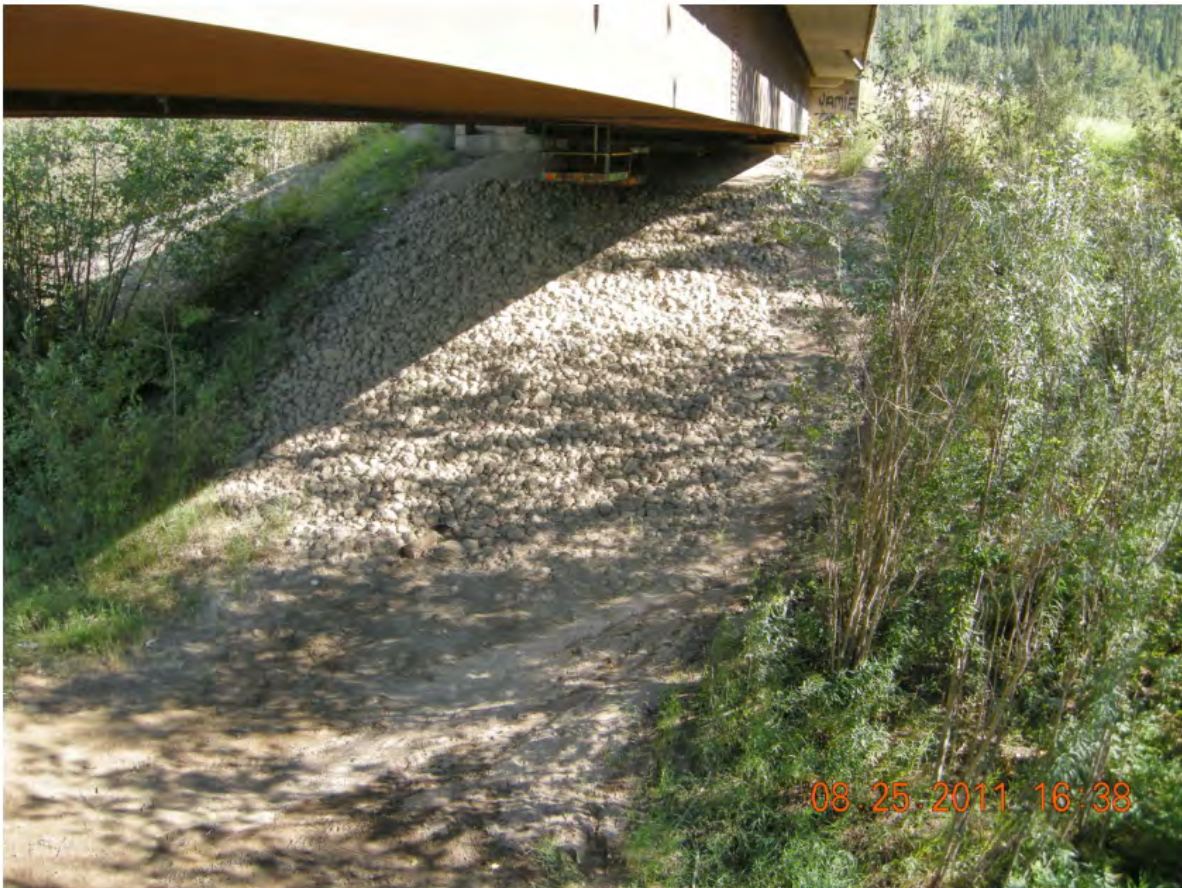
P56 - South Abutment and Embankment - Gabion Slope Protection
