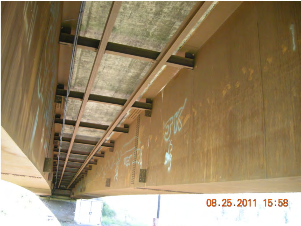
P38 - Span 5 Girders - Looking North
