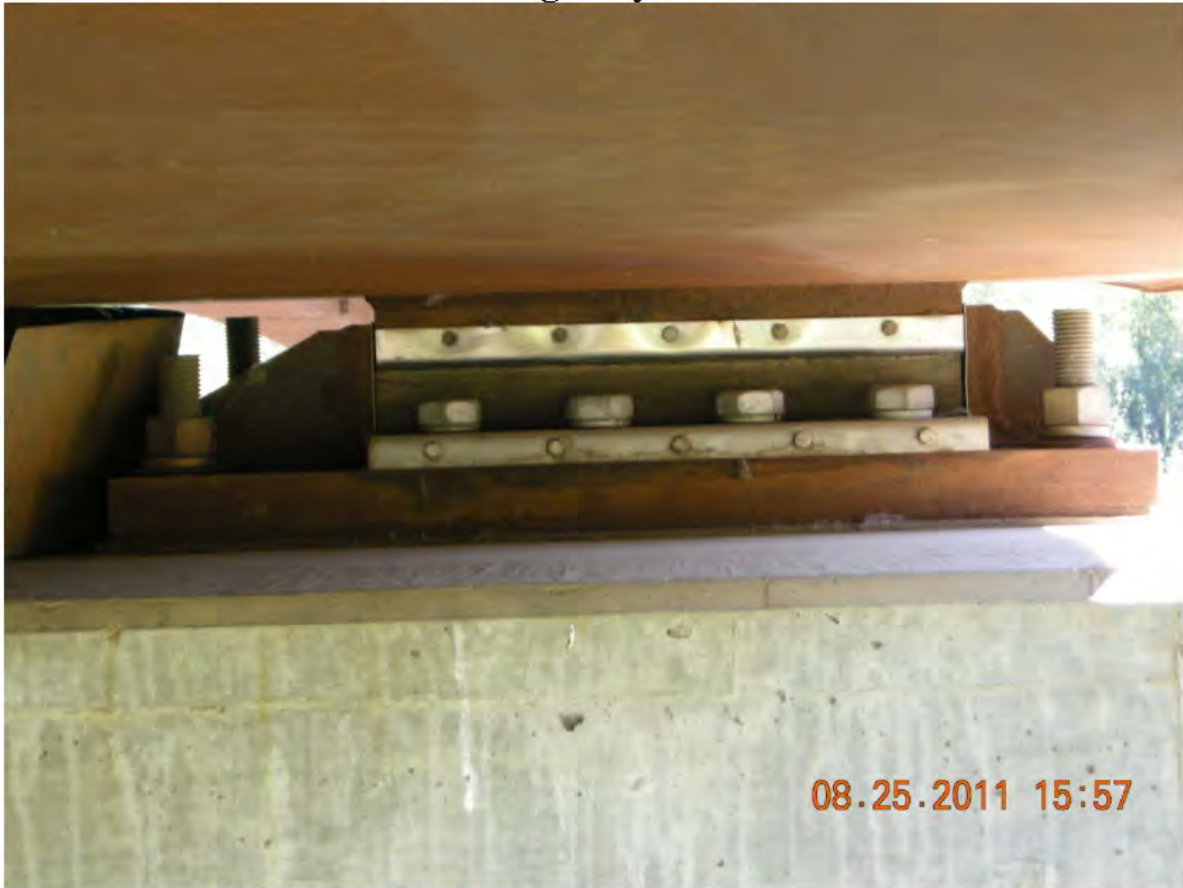
P75 - Pier 4 - 1 Bearing Exposed below West Girder
