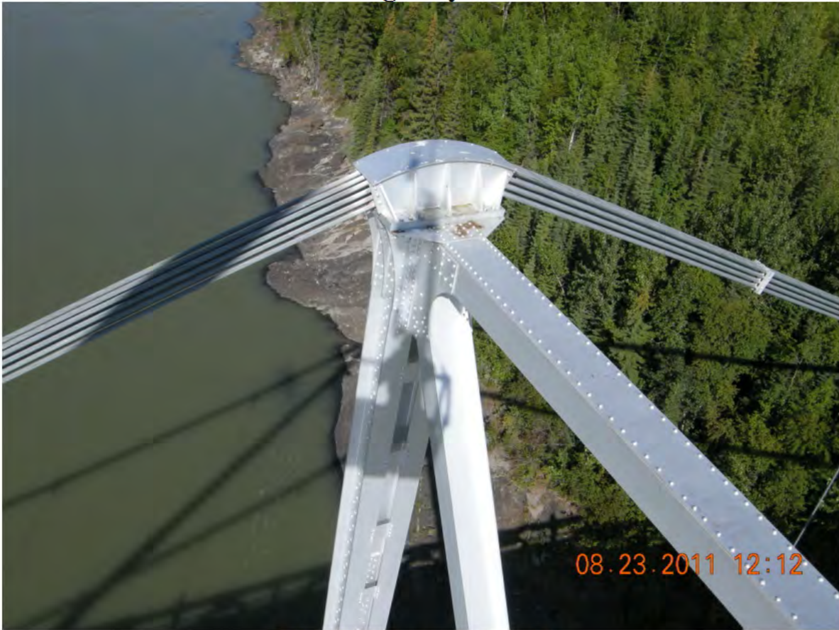
P111 - North Tower - West Saddle
