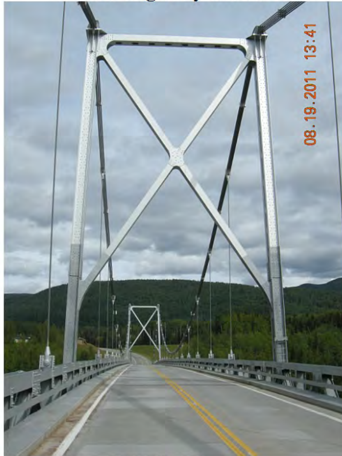
P101 - South Tower
