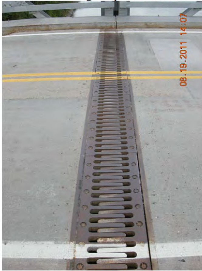
P11 - South Tower - Finger Joint
