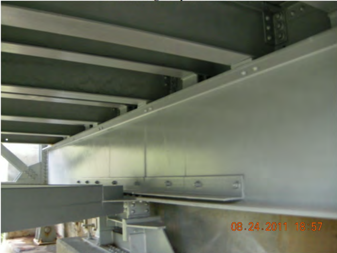
P25 - Span 1 - Floorbeam L12 at South Abutment
