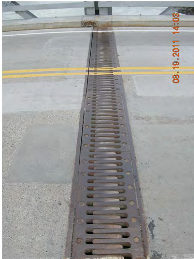
P12 - North Tower - Finger Joint
