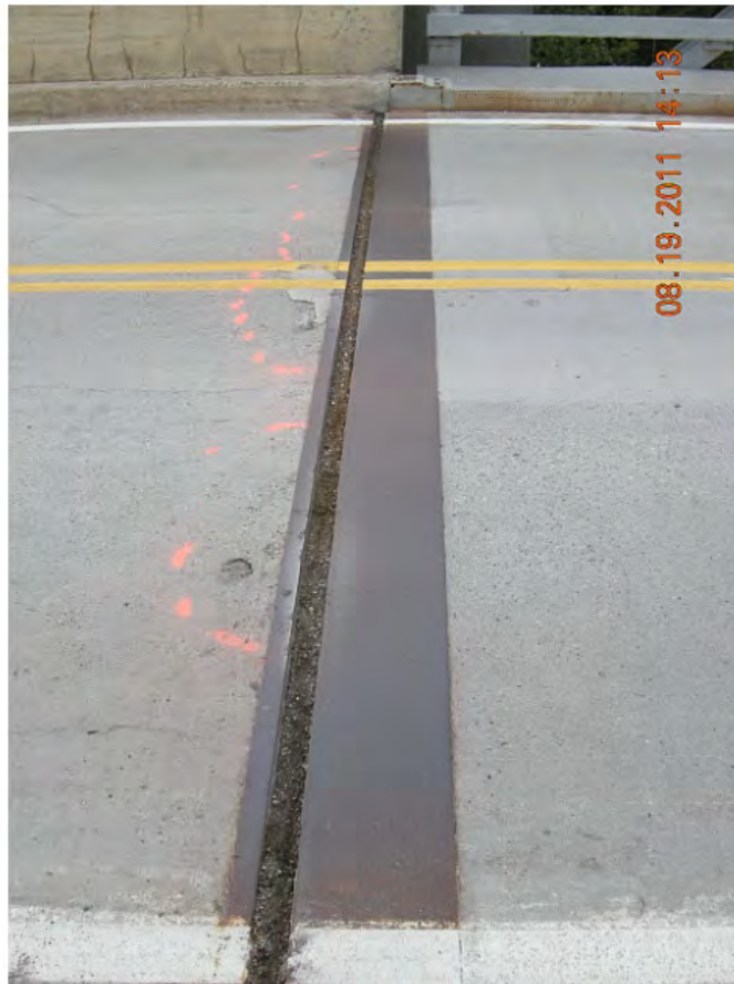
P10 - South Abutment - Expansion Joint
