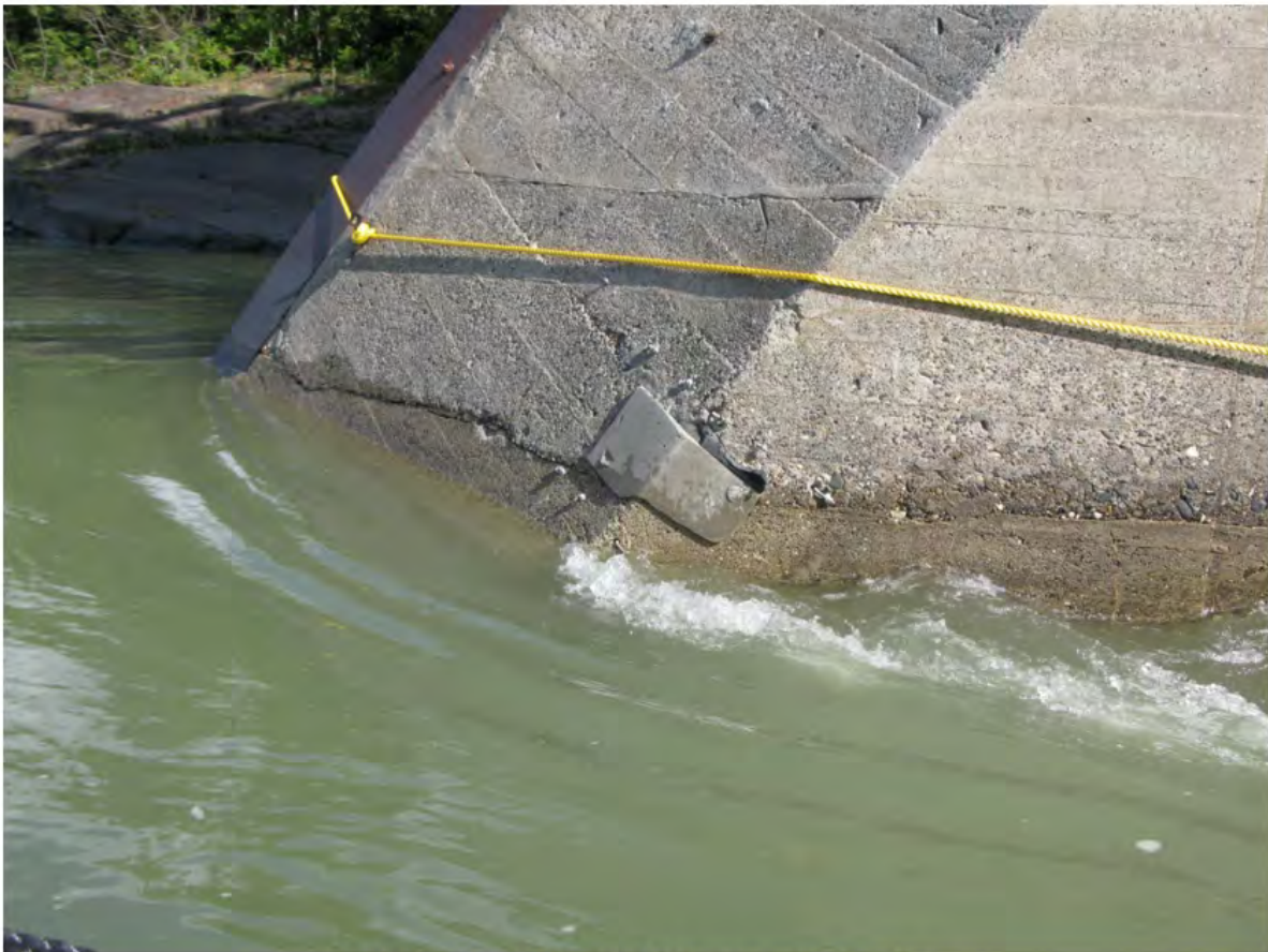
UW18 - Pier 2 US nose LC face repair on nose
