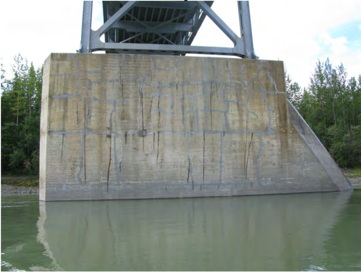
UW03 - Pier 1 HC face 2
