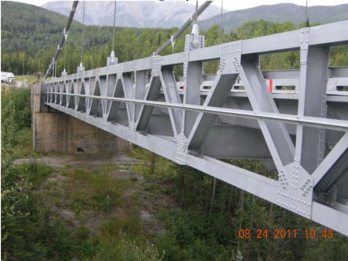
P23 - Span 1 - East Deck Truss - Looking South
