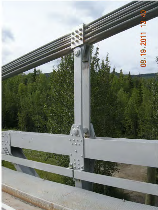
P50 - Span 1 - Hanger 2S West
