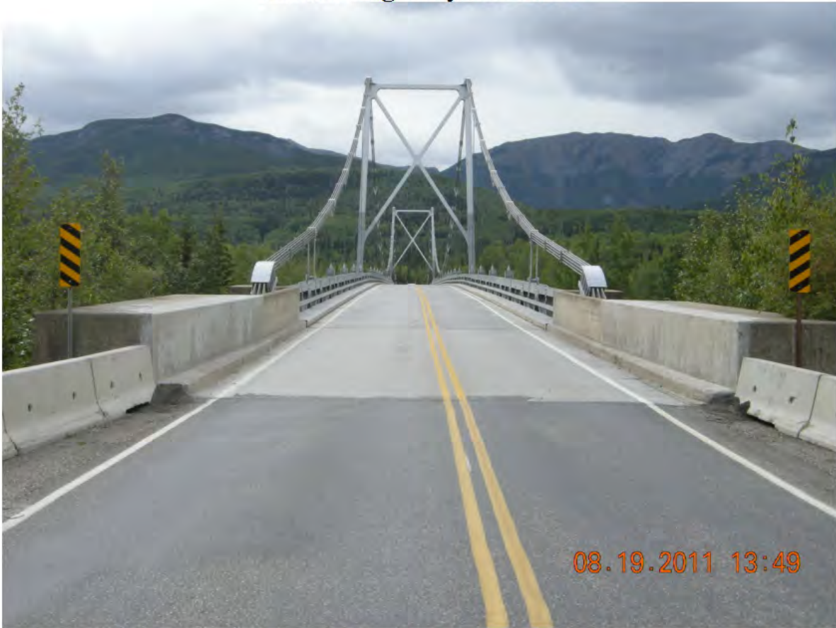
P17 - North Approach - Abutment Barriers have Tapers Installed Since 2009 Inspection - Similar at South Abutment
