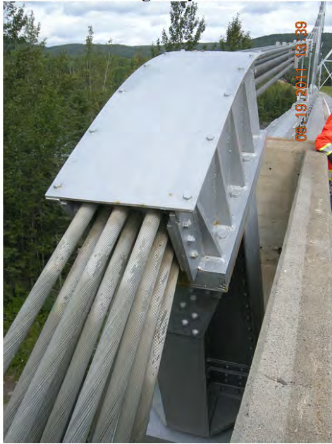
P95 - South Abutment - SW Cable Saddle
