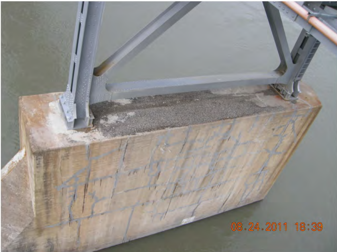
P98 - South Pier = South Face
