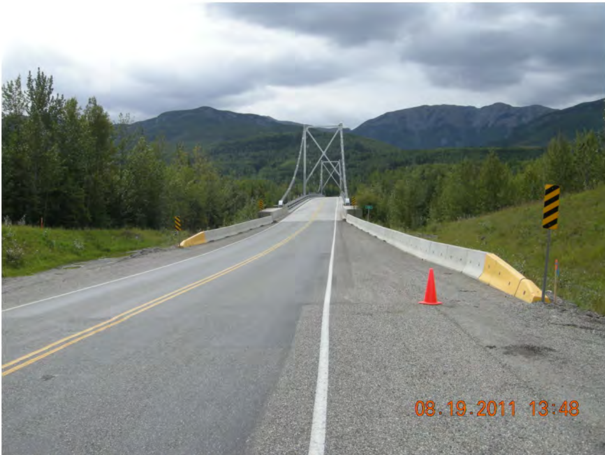
P02 - North Approach - Looking South - All 4 Delineators and River Name Sign in Place
