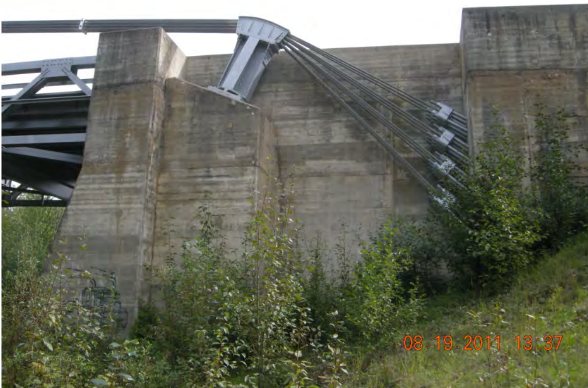
P90 - South Abutment - SW Cable Saddle and Anchorage
