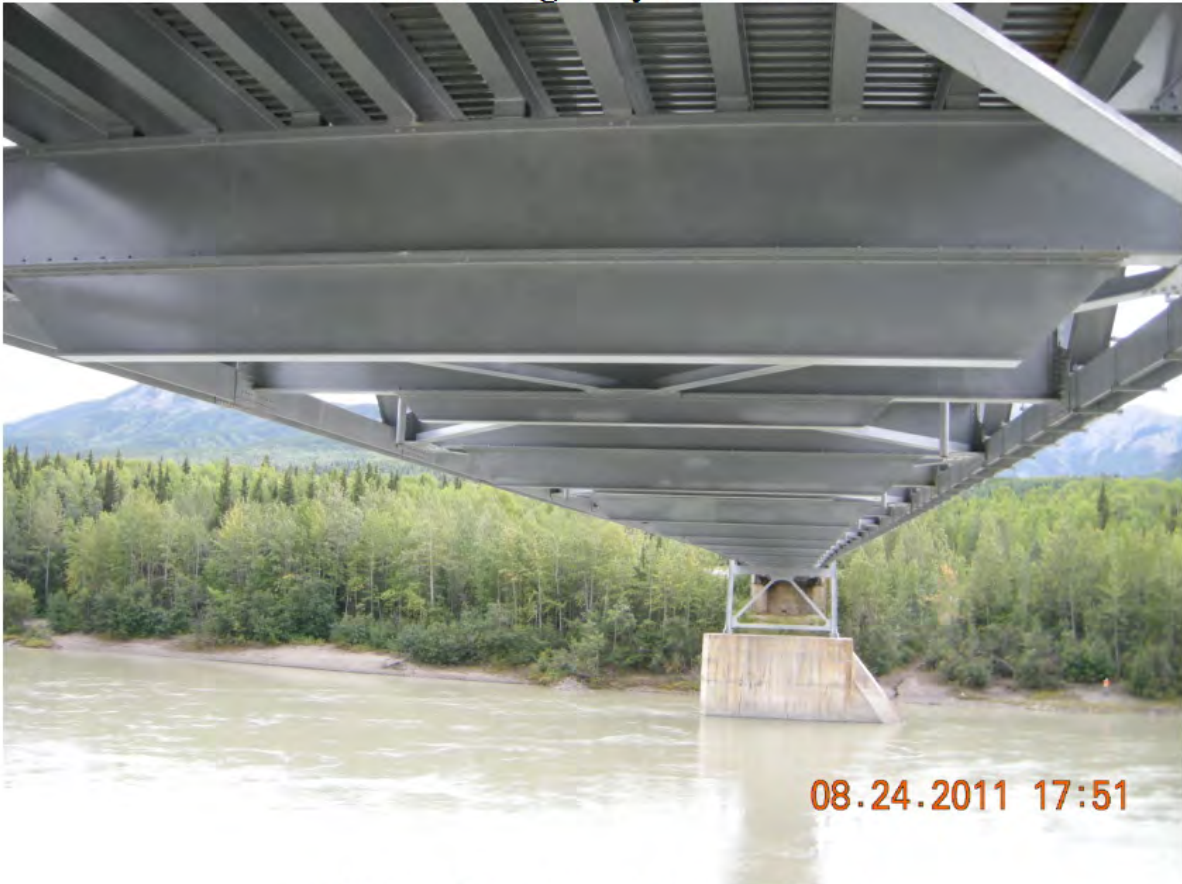
P33 - Span 2 - Floorbeam L15 - Looking South
