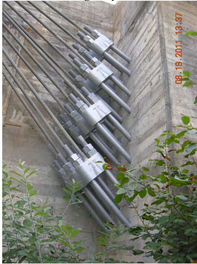
P91 - South Abutment - SW Cable Anchorage
