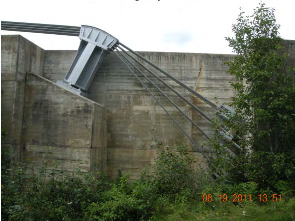
P113 - North Abutment - NE Cable Saddle and Anchorage
