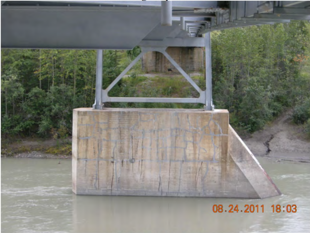
P99 - South Pier - North Face
