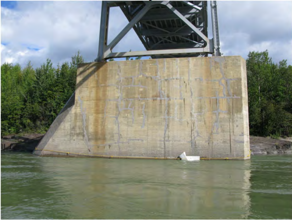
UW19 - Pier 2 LC face genera 2
