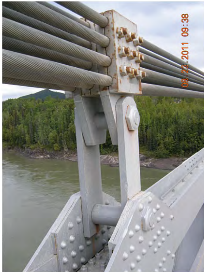
P66 - Span 2 - West 26 Hanger
