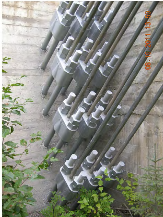
P114 - North Abutment - NW Cable Anchorage
