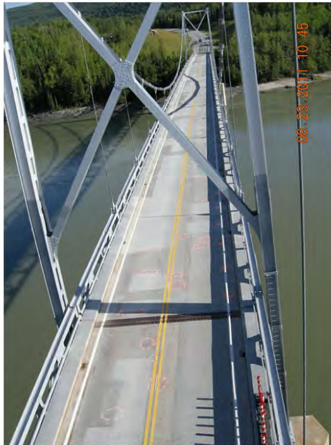
P08 - Overall Deck - Looking North
