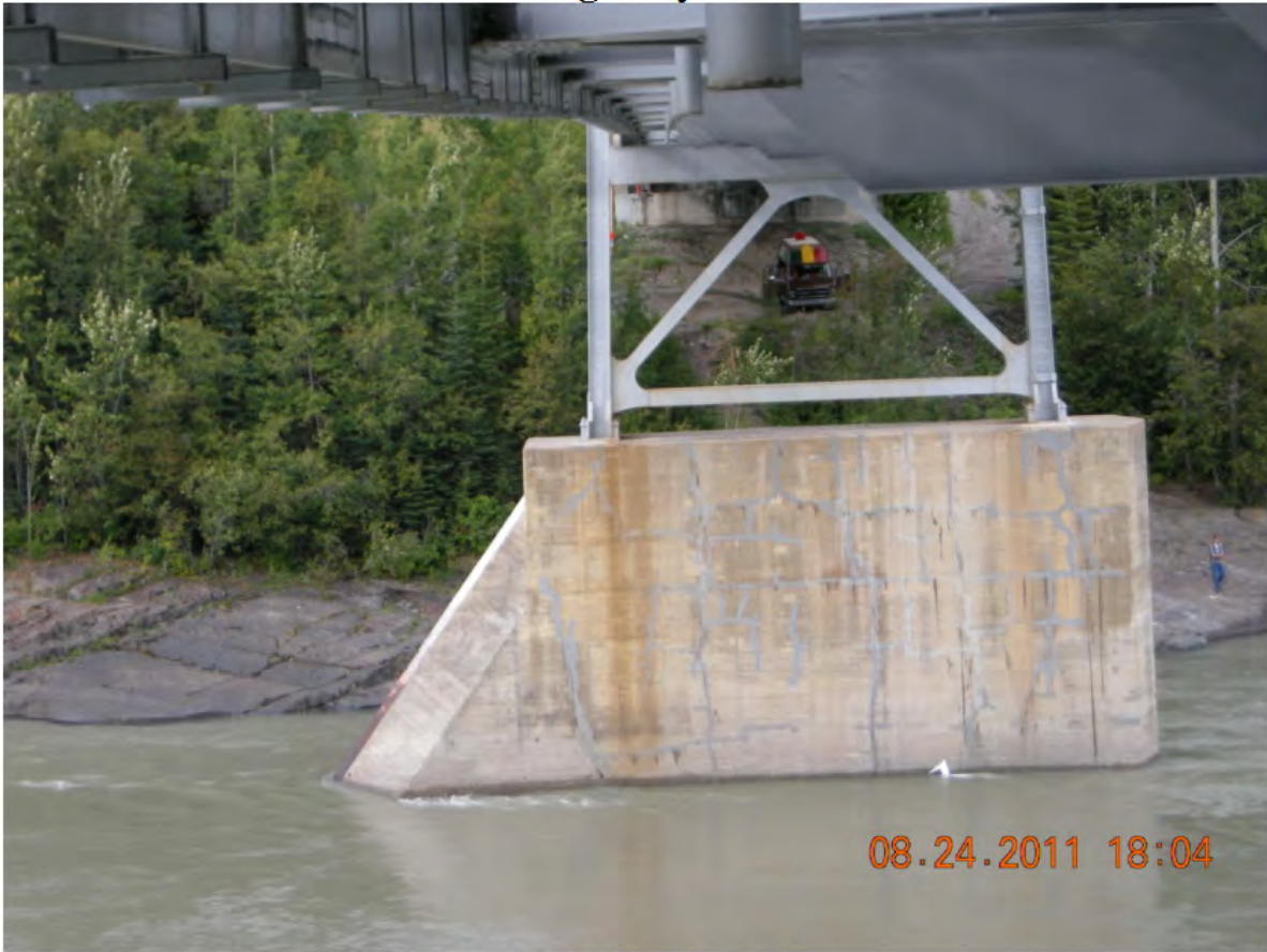
P105 - North Pier - South Face
