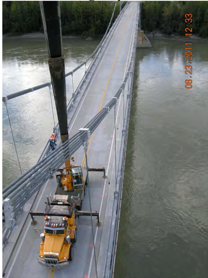
P61 - Span 2 - West Cables - Looking South from North Tower
