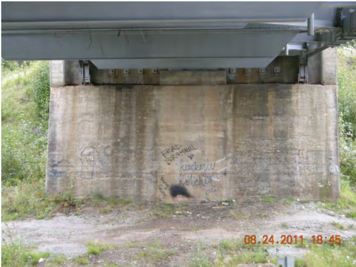
P92 - South Abutment
