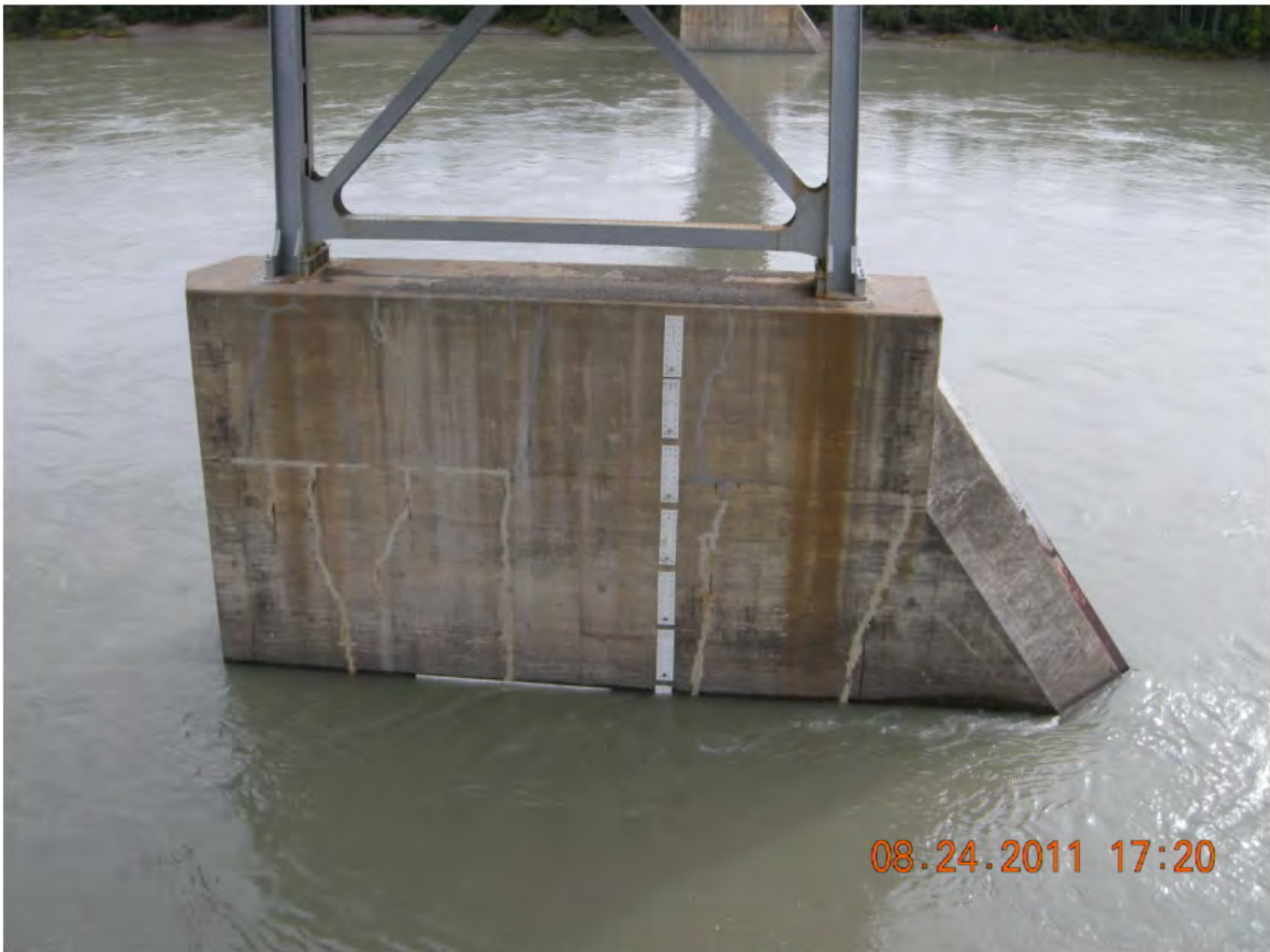
P106 - North Pier - North Face
