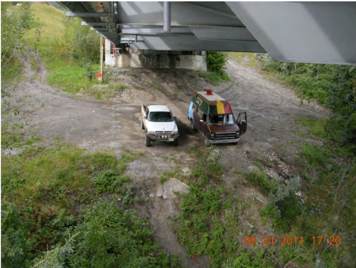
P112 - North Abutment and Embankment
