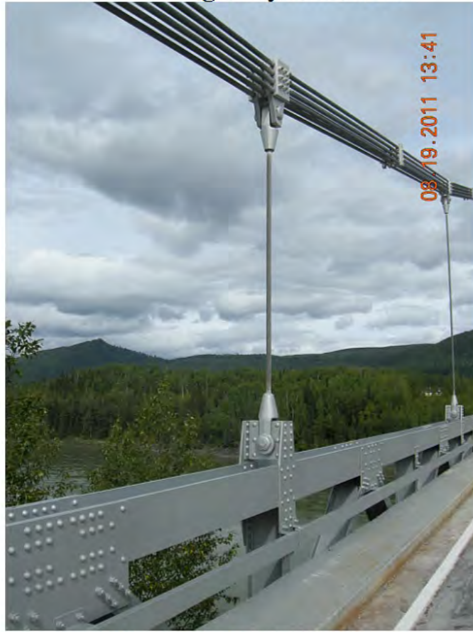
P51 - Span 2 - Hanger 16S West
