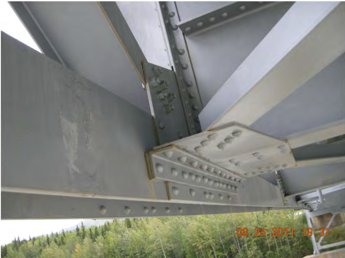
P34 - Span 2 - East Truss - Typical Truss - Floorbeam Connection
