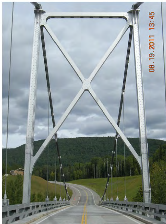
P110 - North Tower - Looking North
