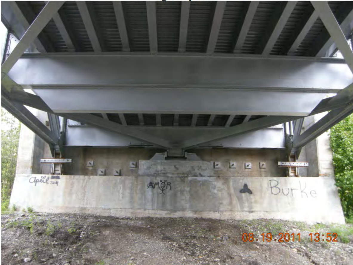
P115 - North Abutment Wall and Bearing Seat
