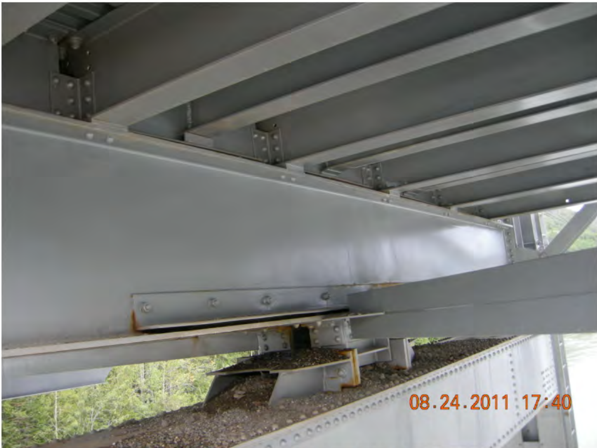
P42 - Span 2 - Floorbeam L28 below North Finger Joint
