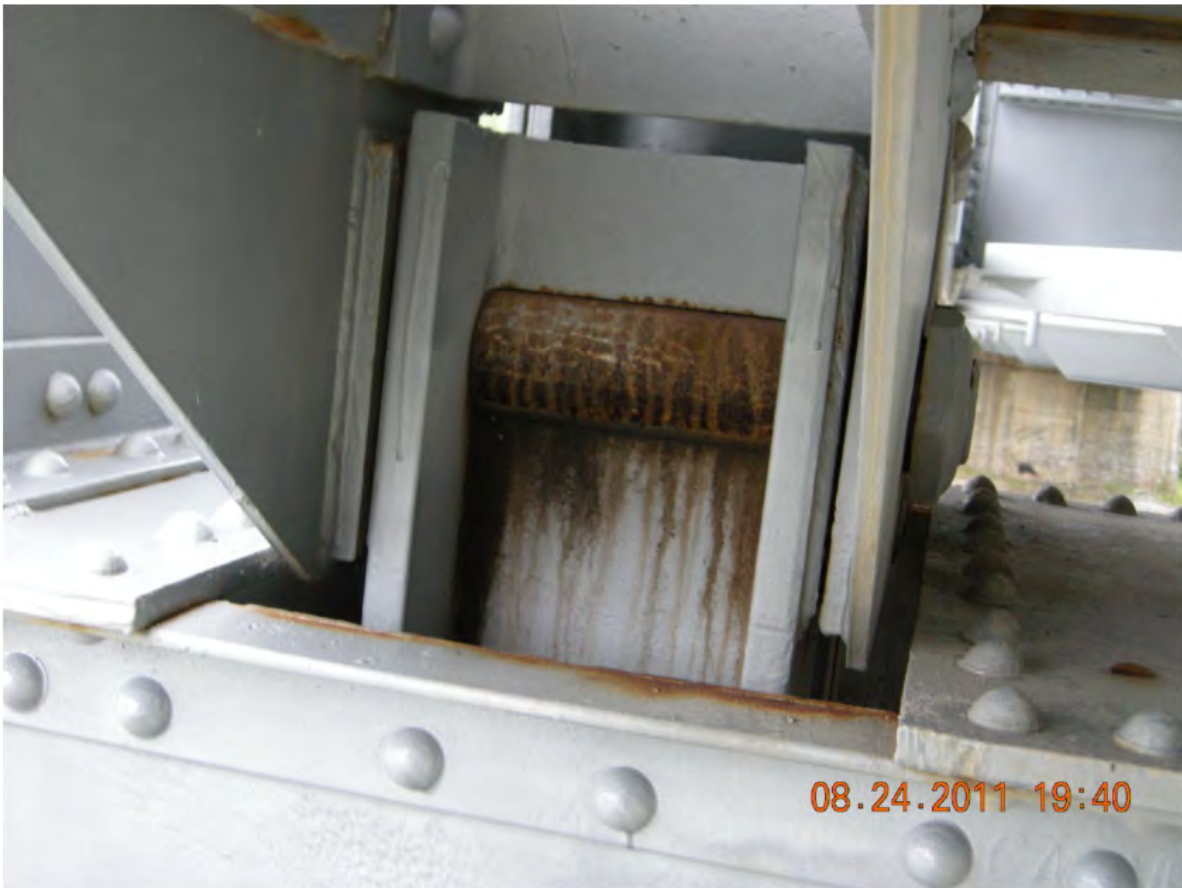
P100 - South Pier - East Bearing Pins
