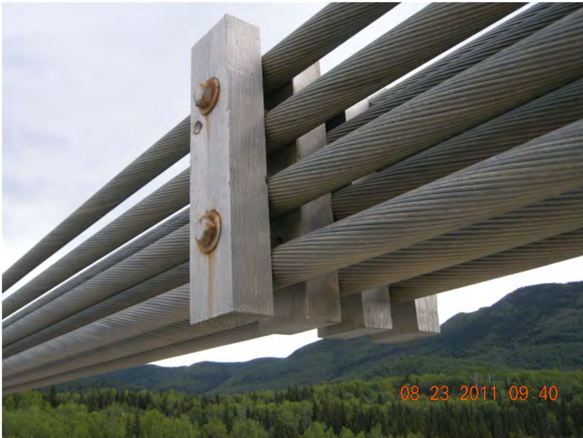
P62 - Timber Cable Spacer - Typical between all Hangers
