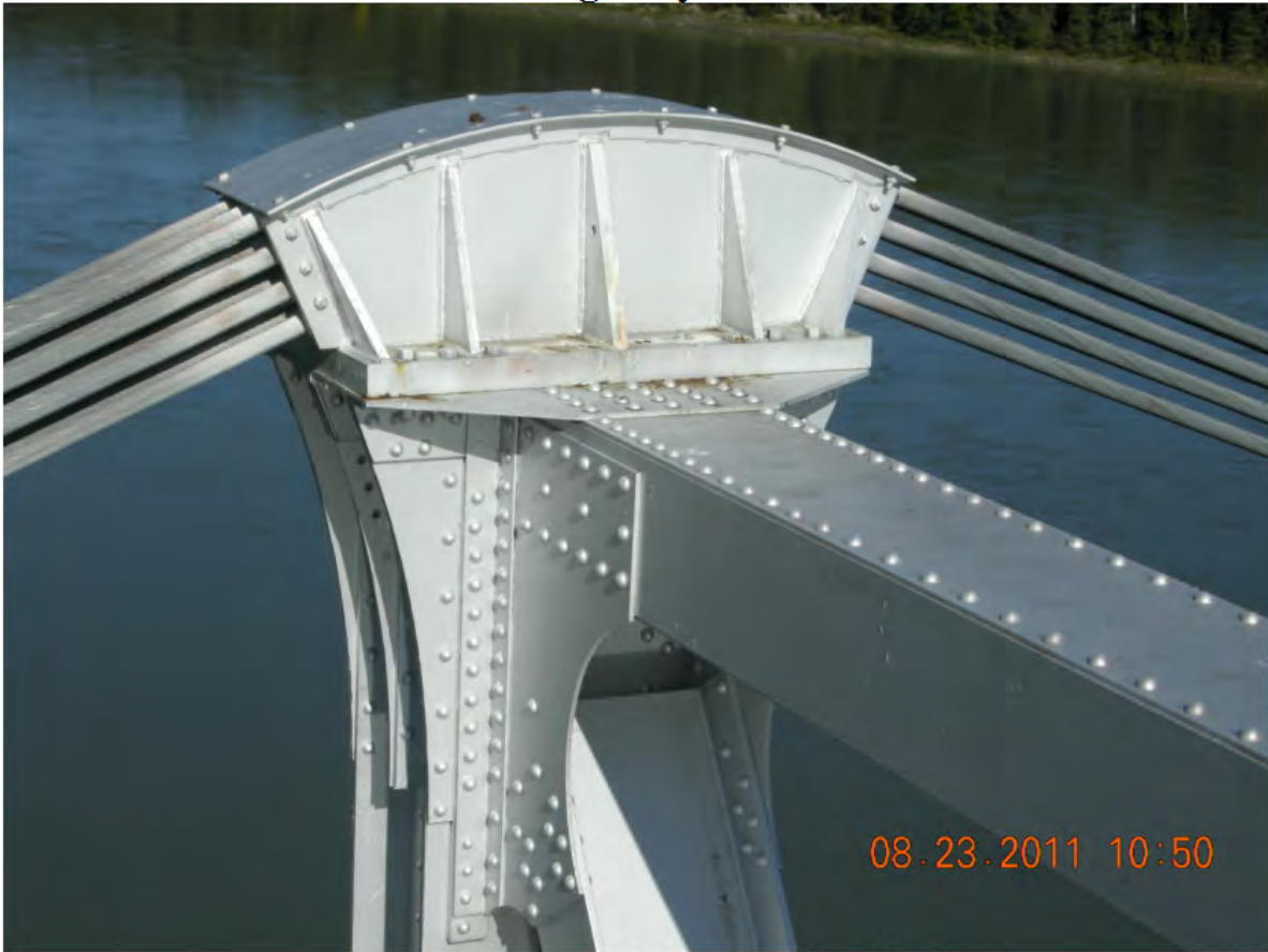
P103 - South Tower - Saddle for West Cables
