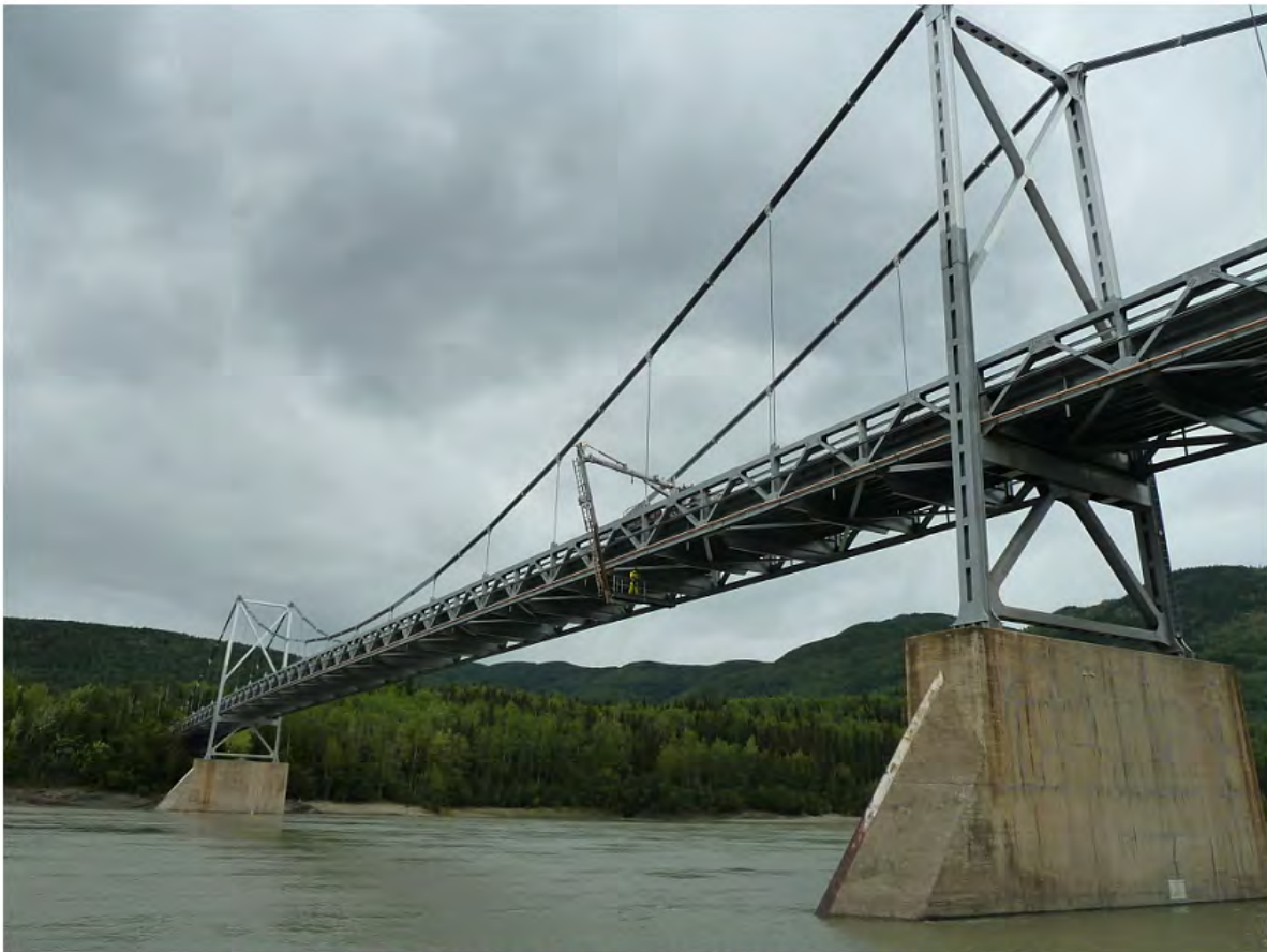
P06 - Inspection of Stiffening Trusses and Floor System by Snooper
