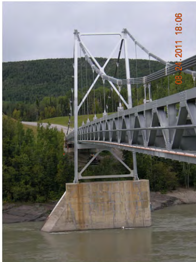
P104 - Deck Truss - Looking North from Midspan
