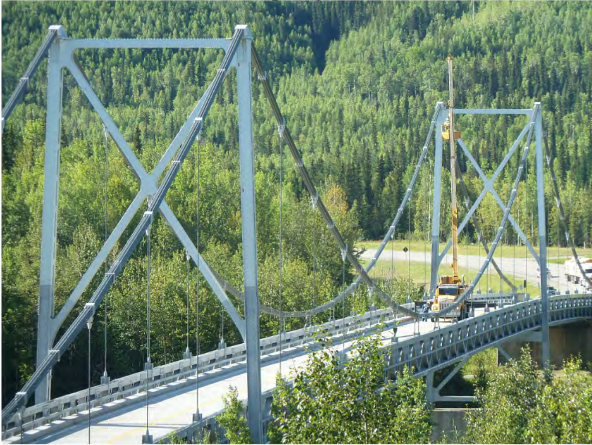
P07 - Inspection of Suspension Cables by Crane
