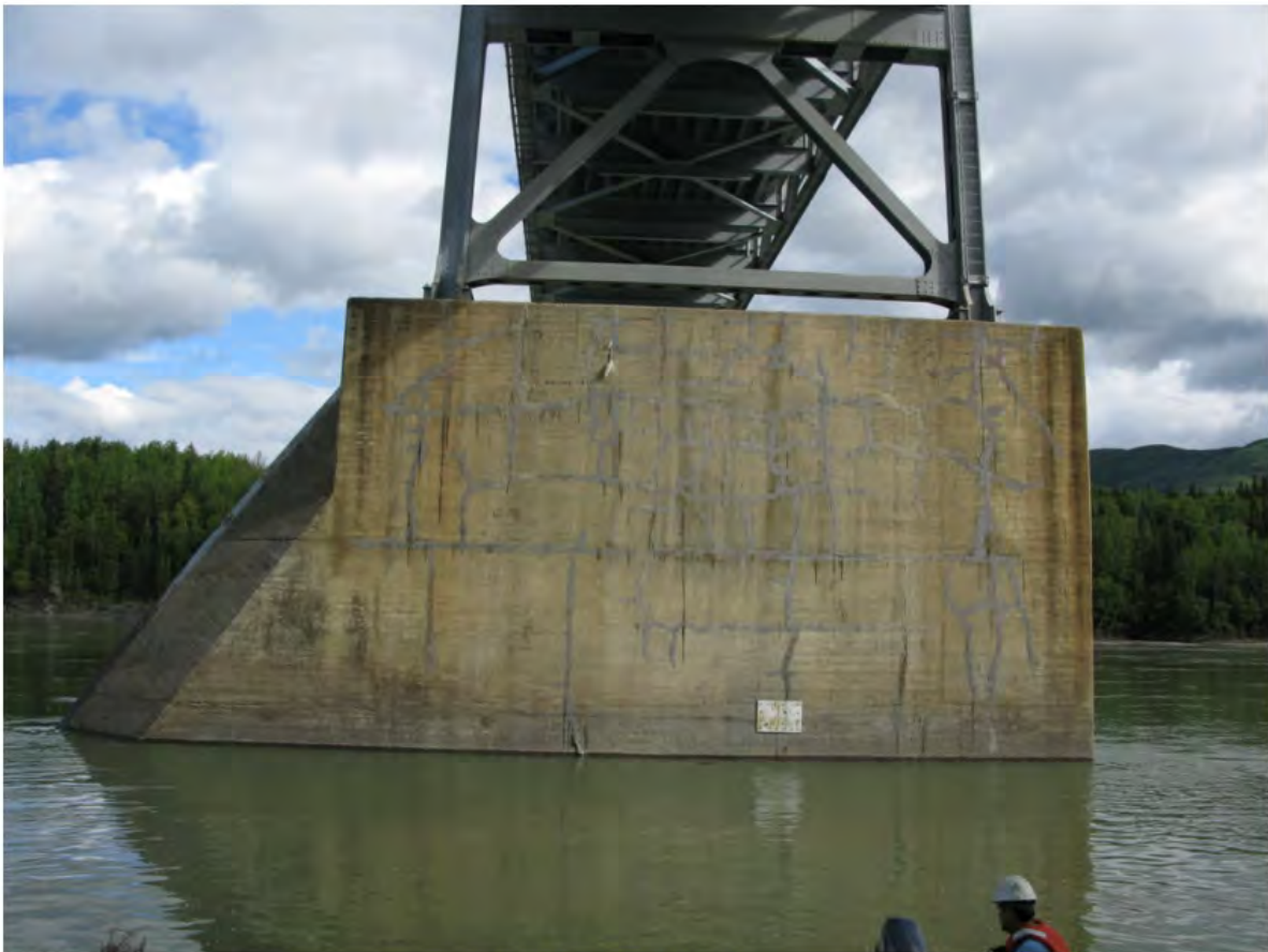
UW08 - Pier 1 LC face
