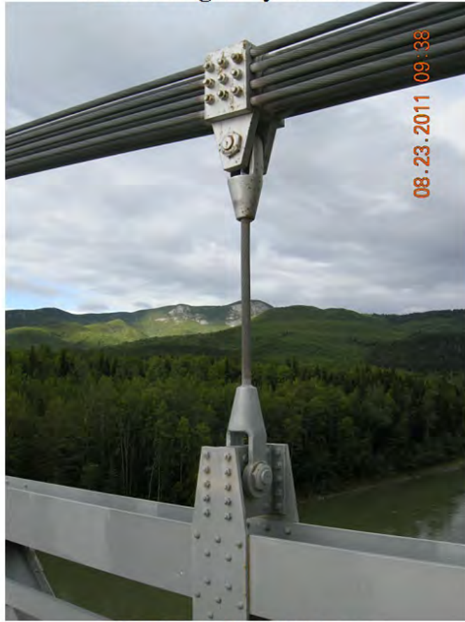
P65 - Span 2 - West 22S Hanger
