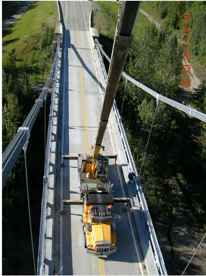
P49 - Crane Setup at Bridge Centreline for Cable Inspections
