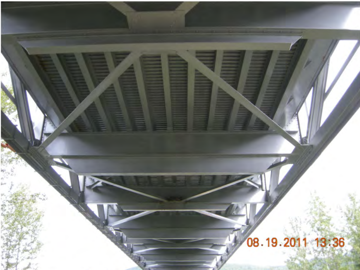
P24 - Span 1 Soffit and Floor System - Looking North
