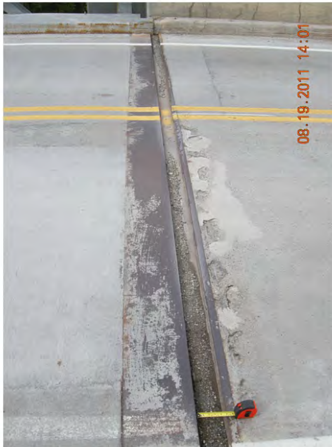
P14 - North Abutment - Expansion Joint
