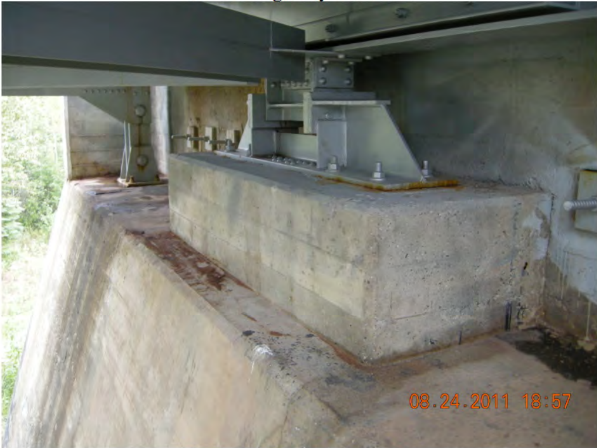
P93 - South Abutment - Lateral Bracing
