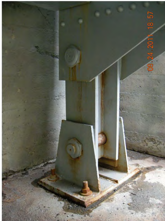
P94 - South Abutment - West Bearing Anchor and Pins
