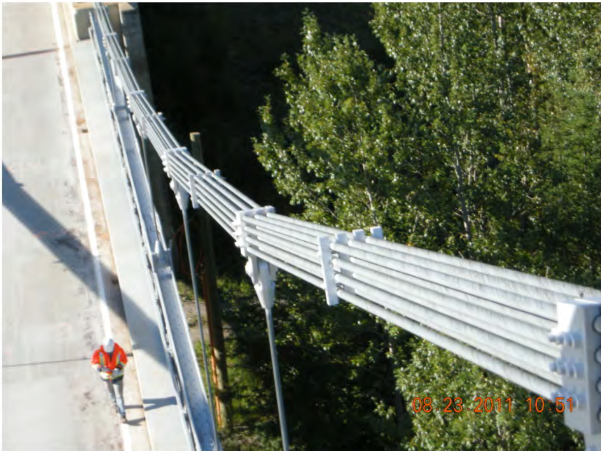
P52 - Span 1 - West Cables
