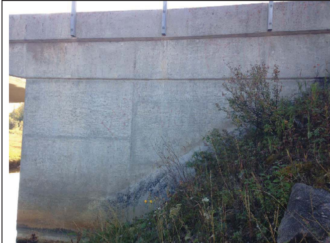
View of southwest wingwall showing loss of fill material, typical all four corners
