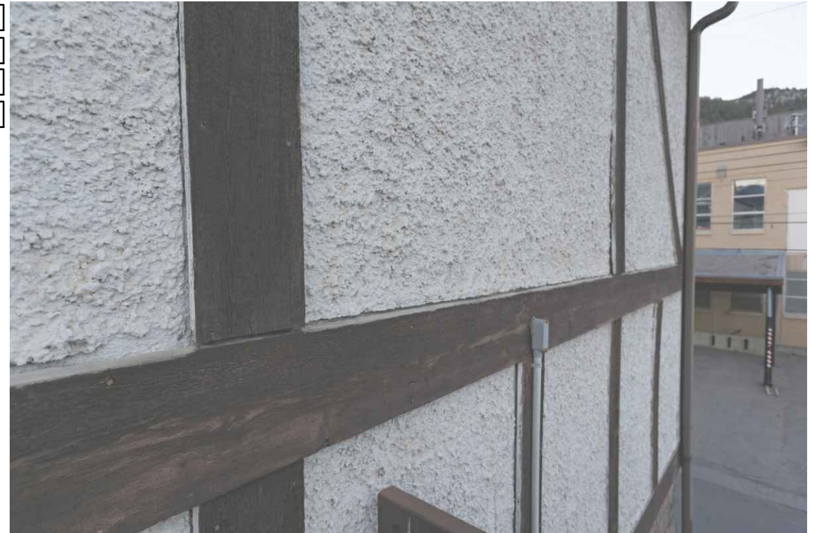
5 | HALF TIMBER/ STUCCO DETAIL – TYP.
