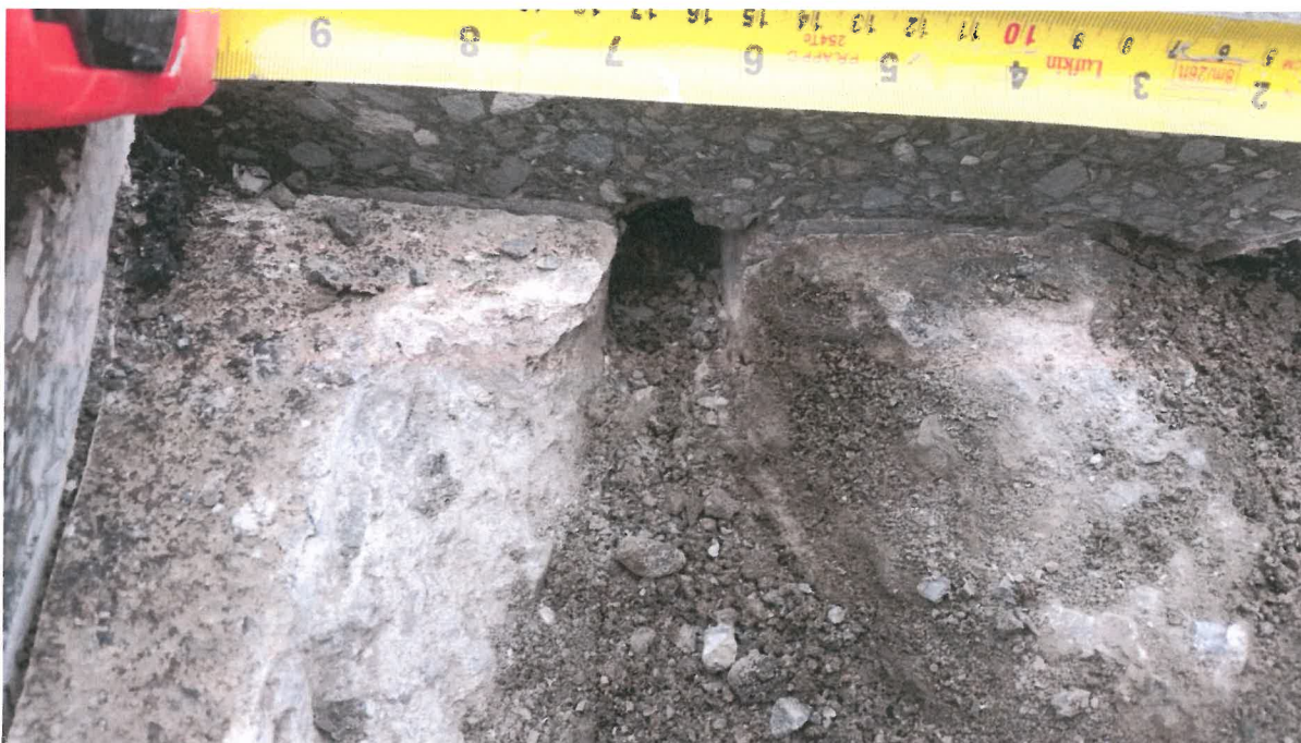
Figure 5 – East Expansion Joint
