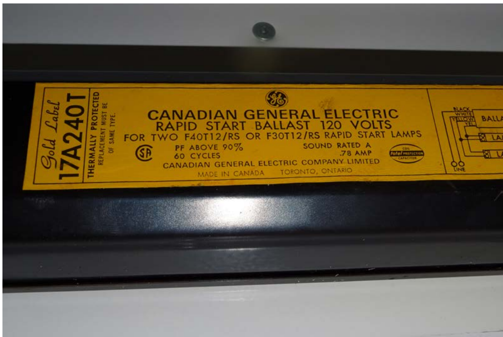
PHOTO 9: Showing suspected PCB-containing fluorescent lamp ballast in the lighthouse.
