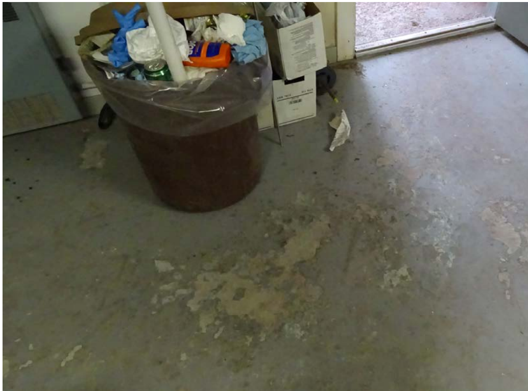
PHOTO 1: Showing gray paint over pale green paint on base level mechanical room floor (PS-CSIL-01).
