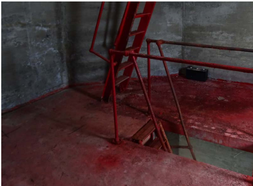
PHOTO 3: Showing red paint on concrete floors on all levels (PS-CSIL-03).
