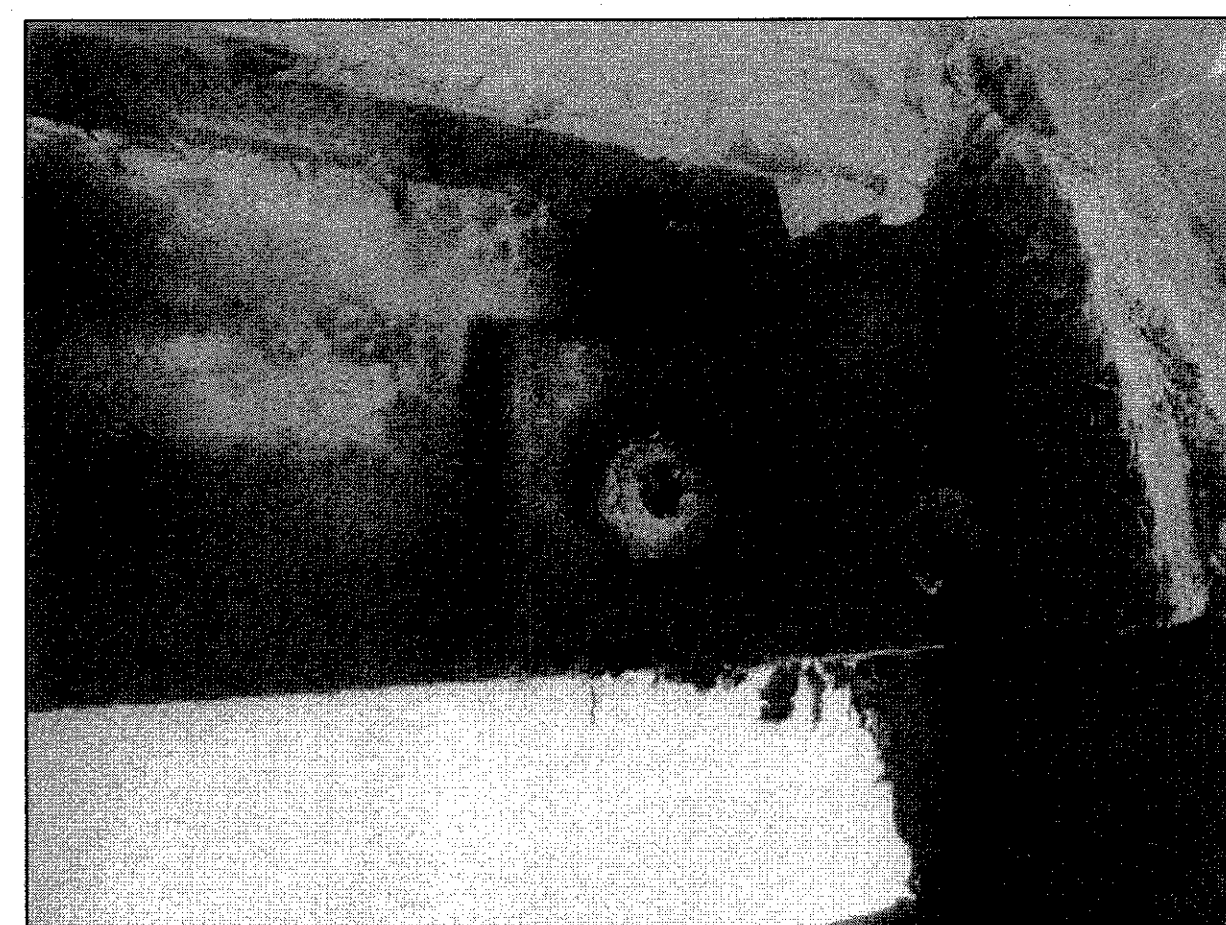
IMAGE 02: BRACKET AT TOP OF LADDERS 1, 2 & 3 TO BE REPLACED. REFER TO DETAIL 2/Ab500
