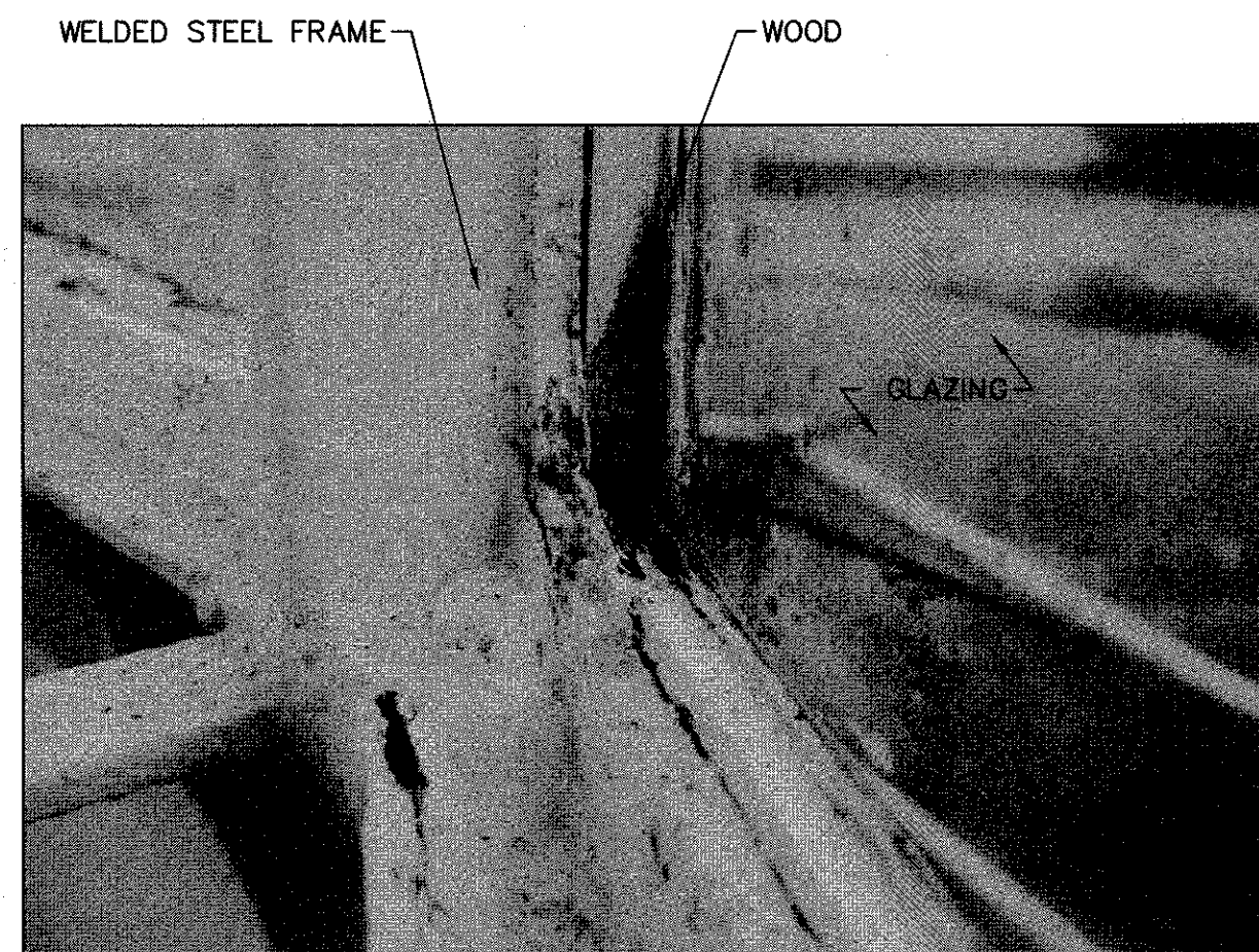
IMAGE 05: DETAIL VIEW OF LANTERN WINDOW ASSEMBLY (INTERIOR). REFER TO DETAIL 4/Ab501
