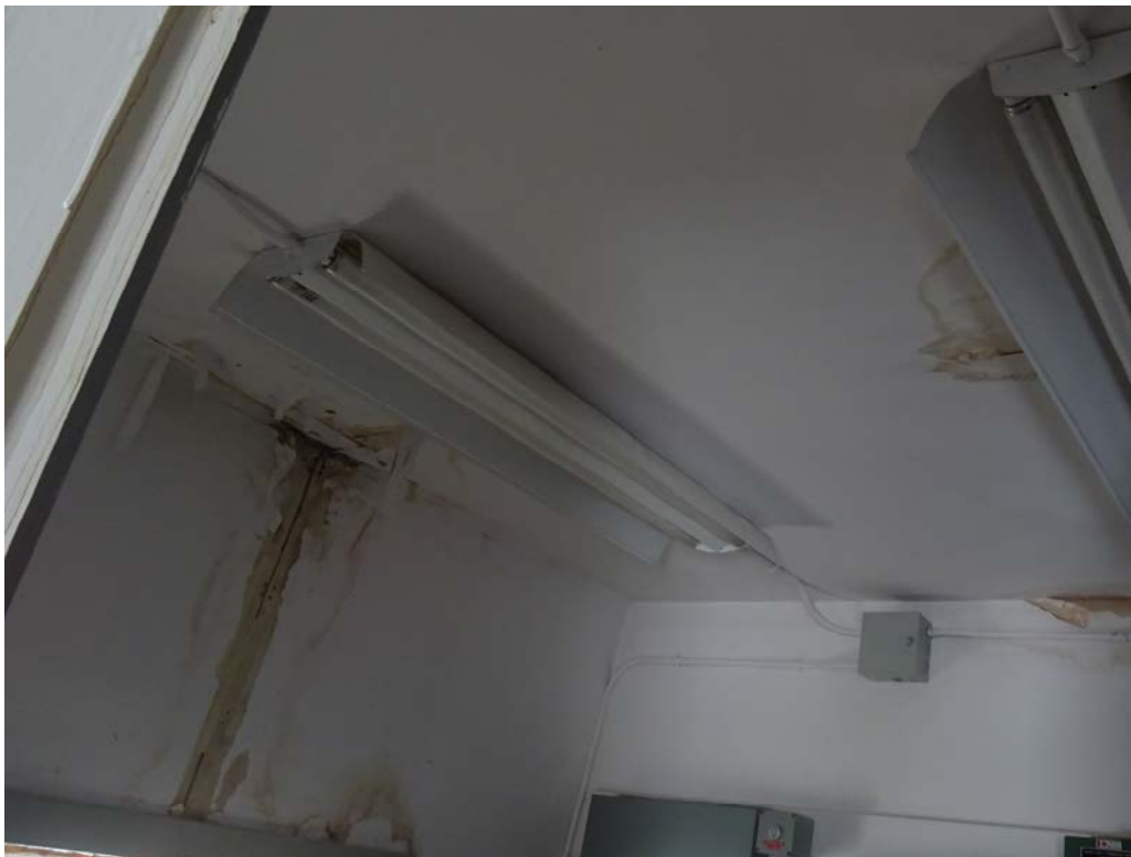
PHOTO 5: Showing white paint on drywall in 2 nd level operations room (PS-CSIL-05). Also showing light fixtures housing suspected PCB-containing lamp ballasts.
