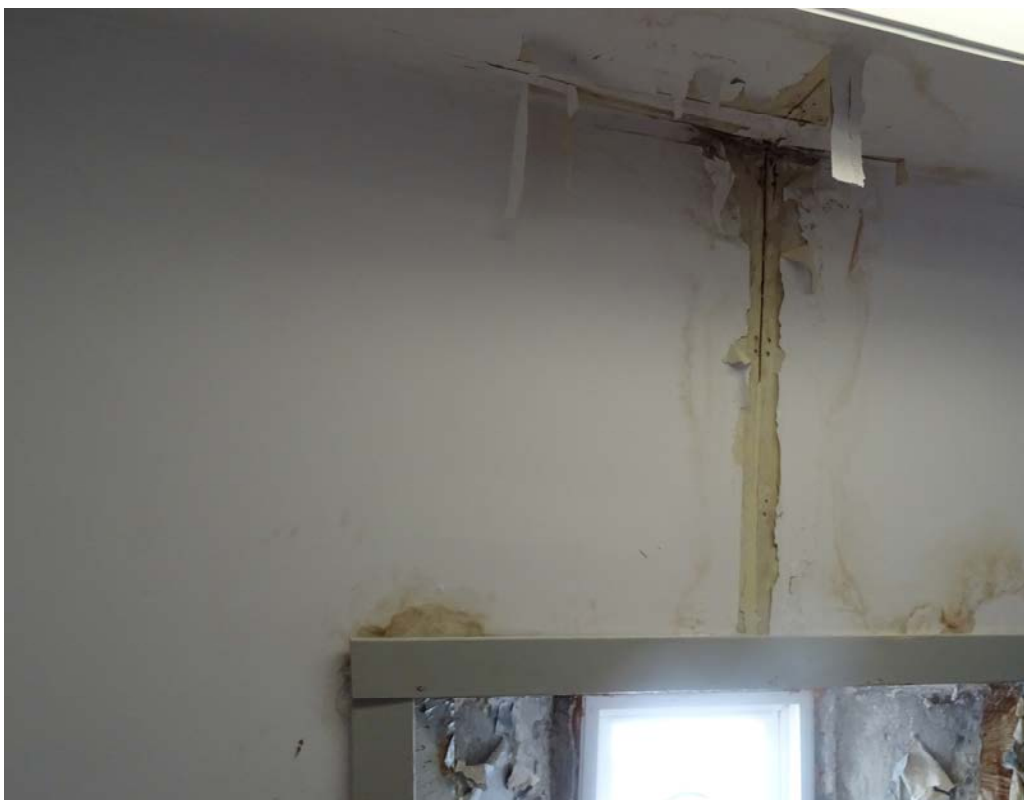
PHOTO 8: Showing the asbestos-containing drywall joint compound in poor condition in the 2 nd level operations room (BS-CSIL-03A).
