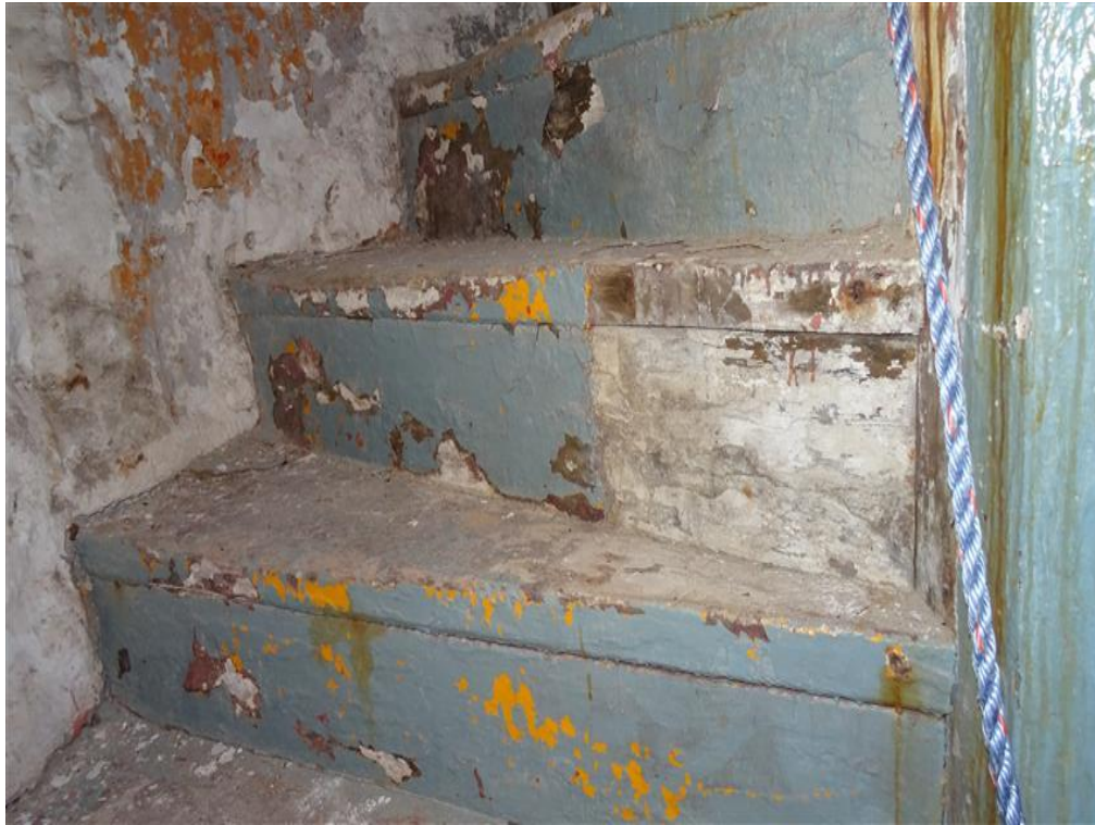
PHOTO 3: Showing grey paint over yellow and brown paint on interior wood stairs (PS-SIL-06).
