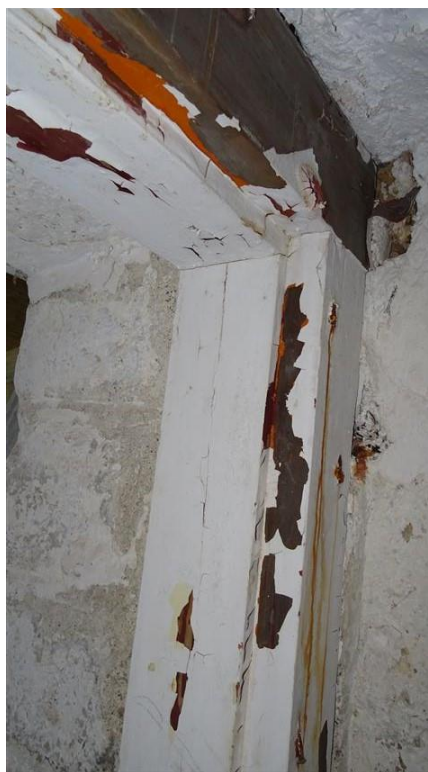
PHOTO 2: Showing white paint over red, cream and brown paint on interior wood trim (PS-SIL-05).
