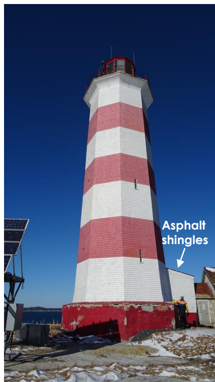
PHOTO 1: Showing exterior white (PS-SIL-01) and red (PS-SIL-03) paint on wood shakes, as well as the red paint on concrete base (PS-SIL-02). Arrow pointing at location of asbestos containing asphalt roof shingles (BS-SIL-02A).
