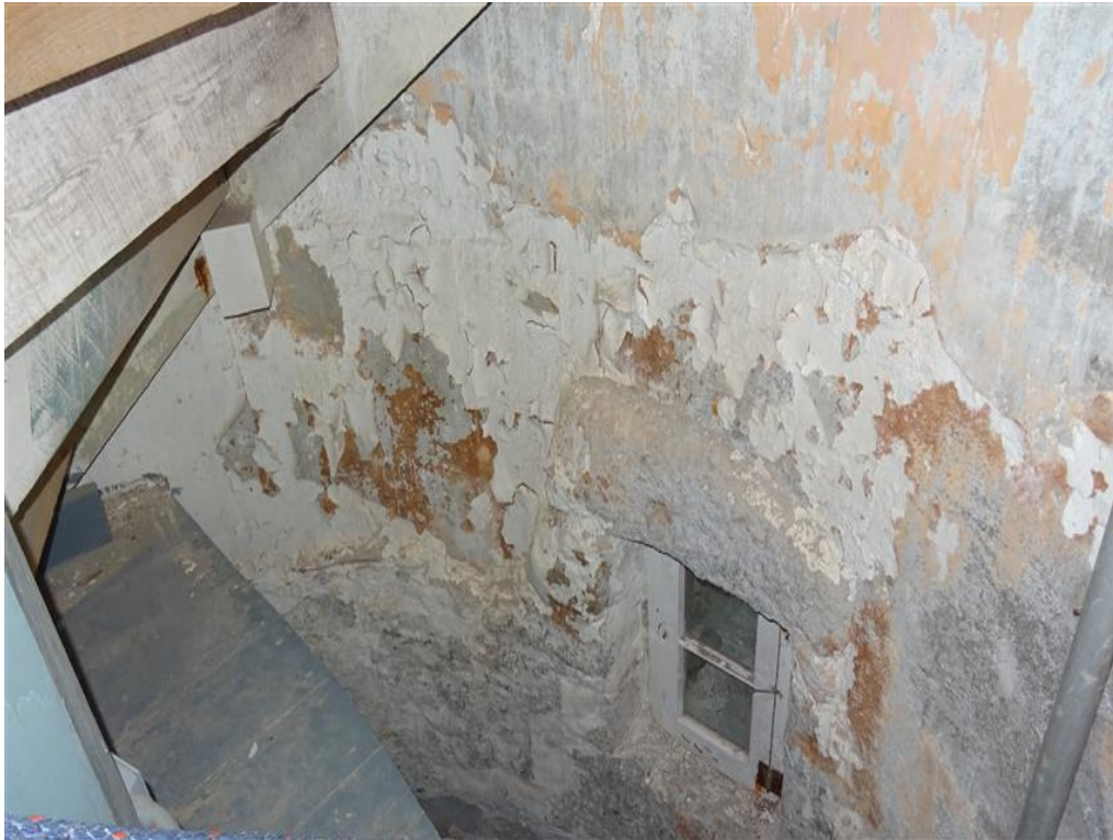
PHOTO 5: Example of white paint over cream paint on interior concrete walls (PS-SIL-07).
