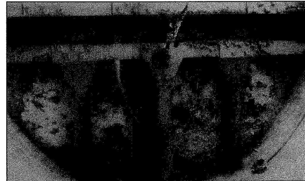
IMAGE 06 - UNDERSIDE OF GALLERY LEVEL FLOOR FRAMING, TO BE PREPARED, PRIMED AND PAINTED
