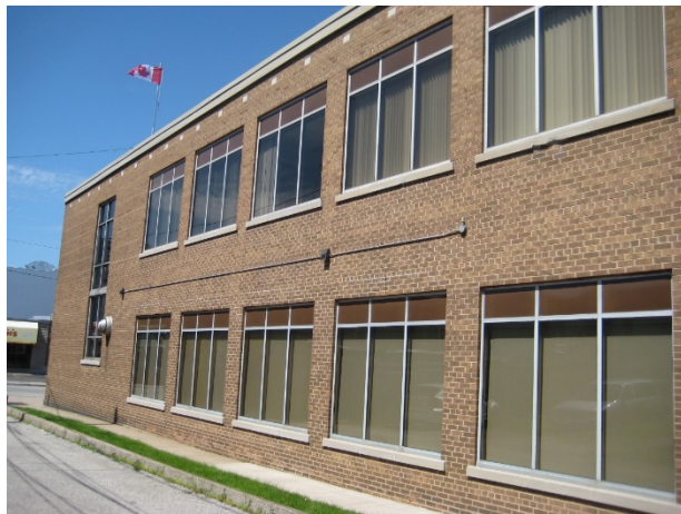
Figure 8 Exterior Windows (Photo: DIALOG 07-15-15)
