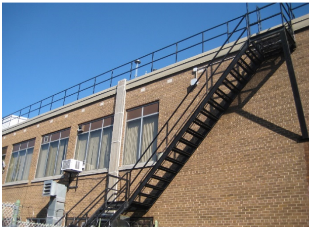
Figure 18 Roof Access Stair (Photo: DIALOG 07-15-15)
