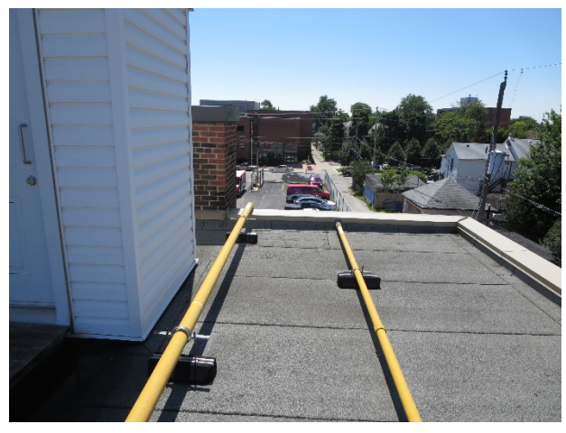
Figure 15 Typical Roof Curb/Parapet (Photo: DIALOG 07-15-15)
