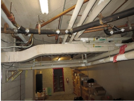
Figure 22 Basement Concrete Structure (Photo: DIALOG 07-15-15)
