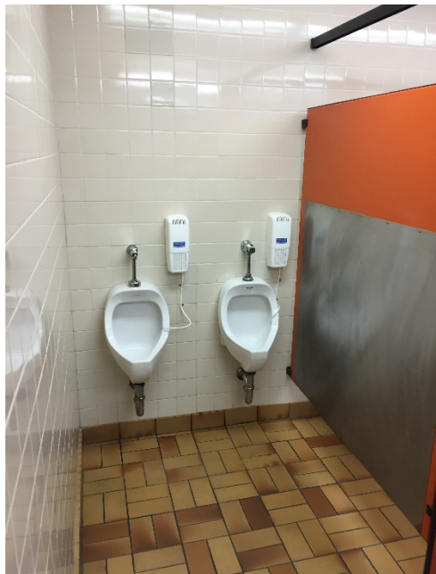
M-Figure 3 Existing Urinals
