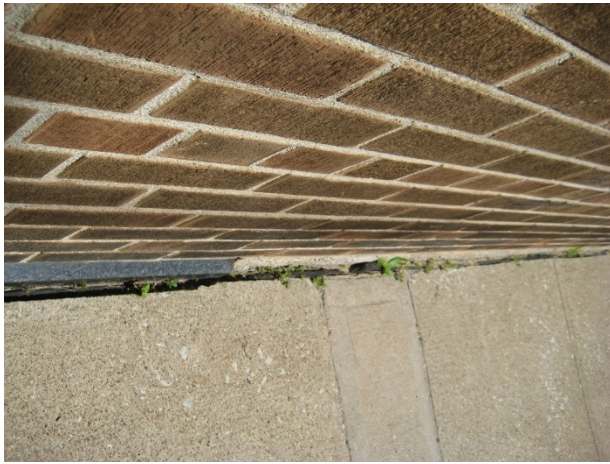
Figure 16 Foundation/Sidewalk (Photo: DIALOG 07-15-15)
