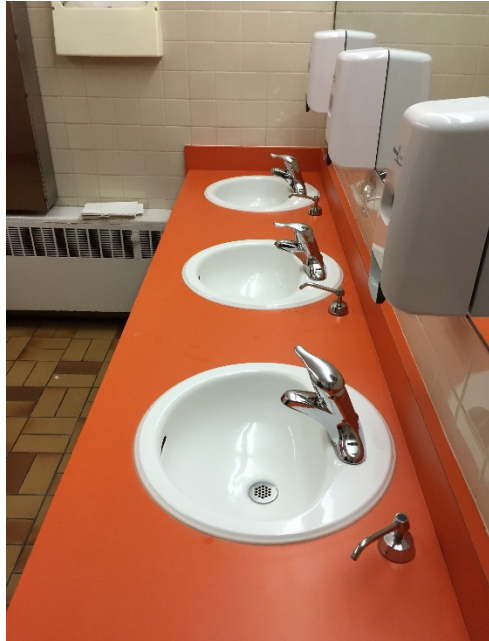
M-Figure 1 Existing Lavatories
