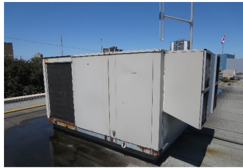
M-Figure 6 Existing Rooftop Units
