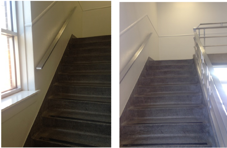
Figure 28 A & B – N-E Stair Handrails. (Photo DIALOG 07-15-15)
