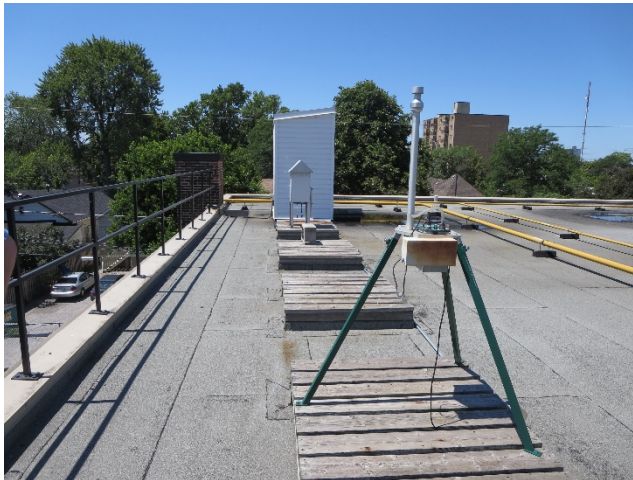
Figure 14 Guardrail on South Elevation (Photo: DIALOG 07-15-15)
