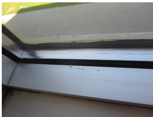
Figure 9 Window Glazing Units (Photo: DIALOG 07-15-15)
