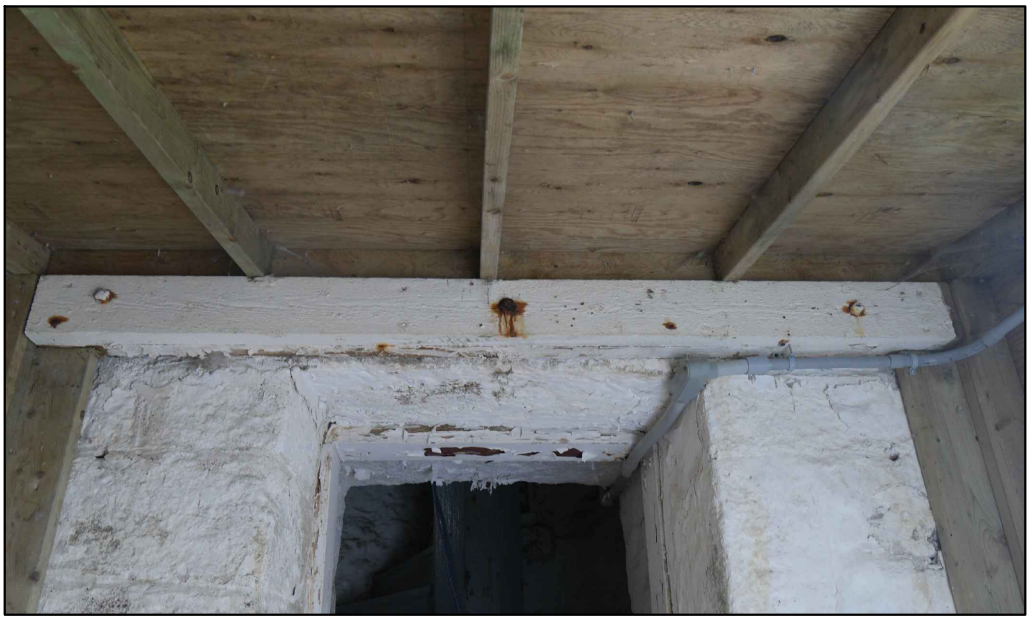
IMAGE 08 – INTERIOR MASONRY WALL AND WOOD LINTEL TO BE PAINTED
