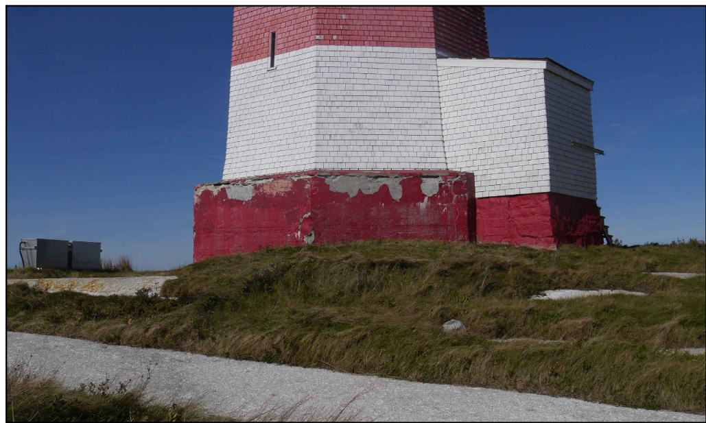
IMAGE 01 – CONCRETE BASE TO BE REBUILT, REFER TO STRUCTURAL
