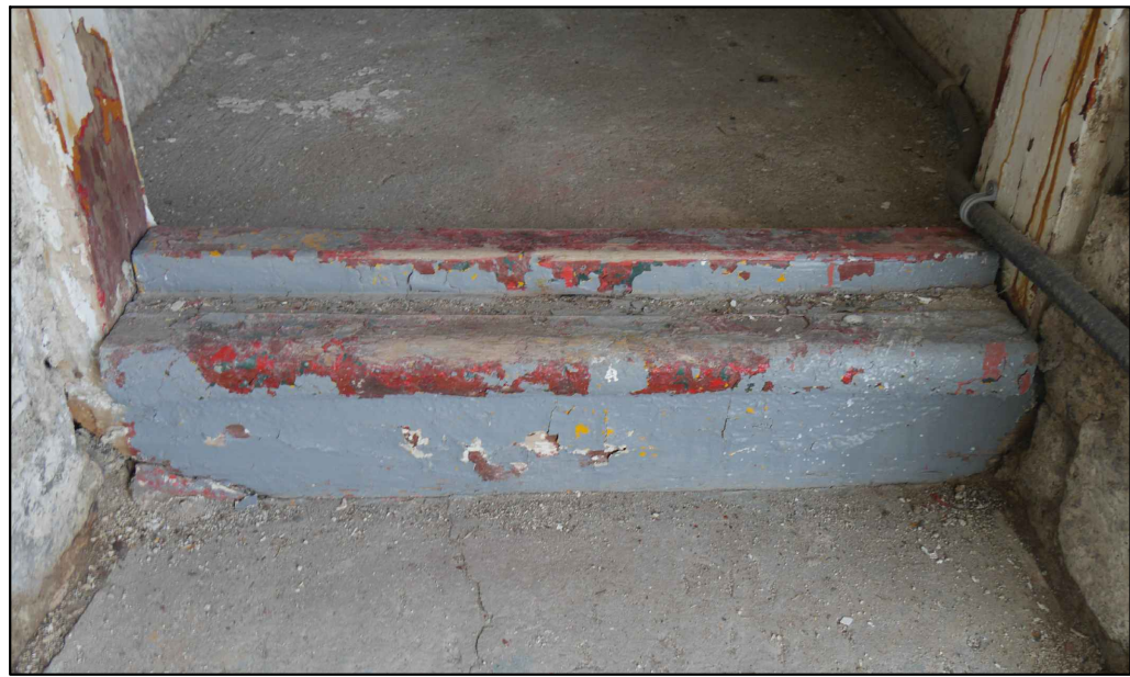
IMAGE 04 – INTERIOR STEPS AT ENTRY LEVEL TO BE RE-NAILED AND PAINTED
