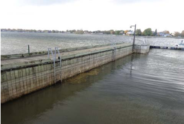
Figure 3 Quai fixe, Quai B
