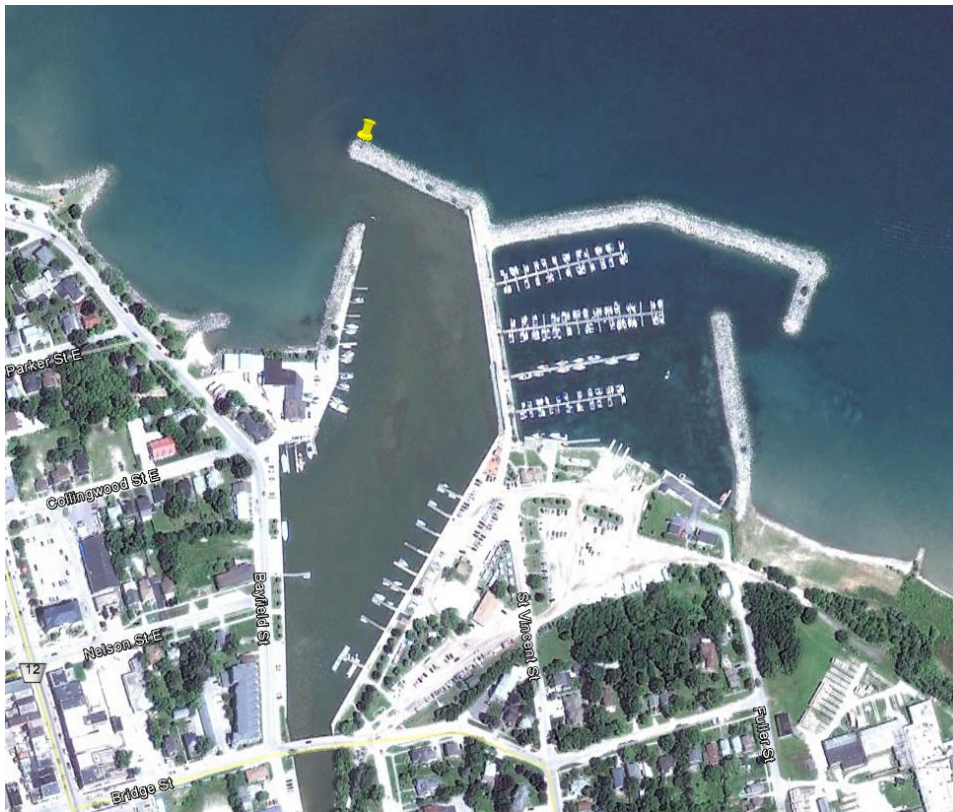
Figures 3 and 4: Project Site Location – Meaford, ON
