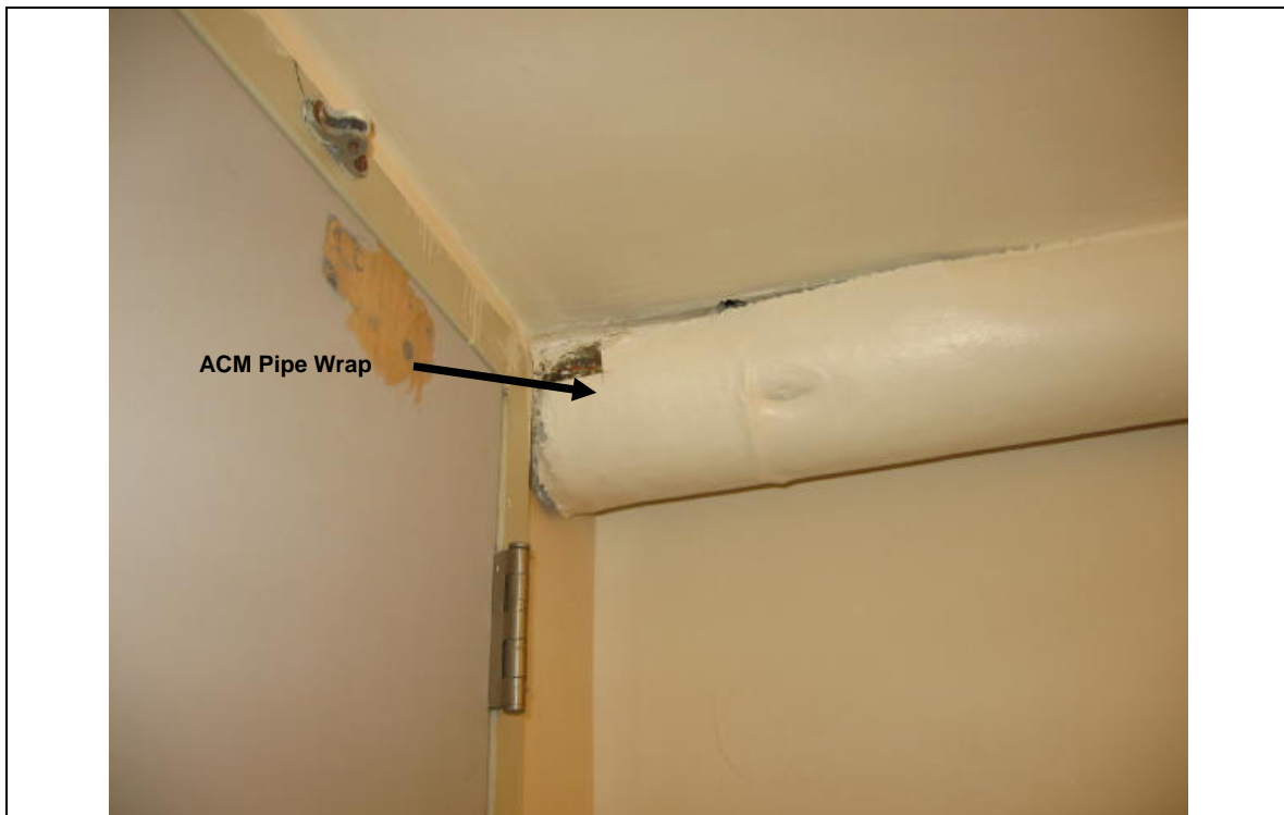
Photograph 3: ACM pipe wrap insulation, corrugated paper-type, Room No. SB-7. (Sample No. ACM 14)
