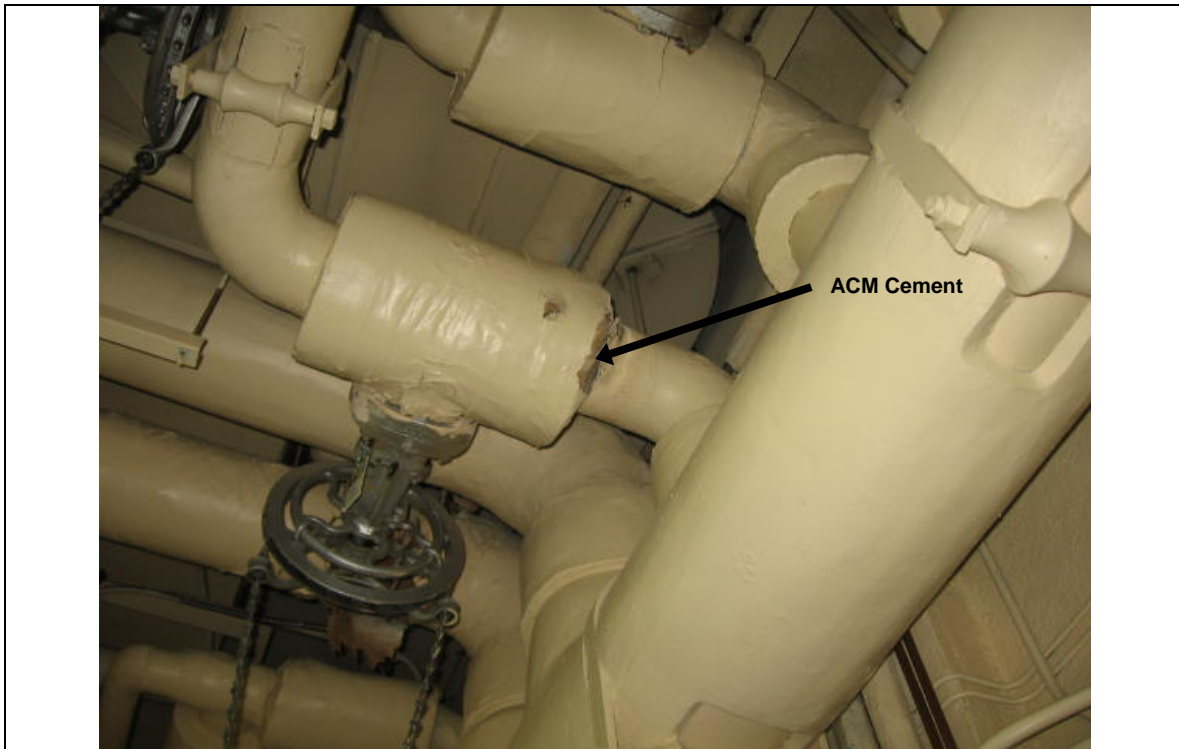
Photograph 11: ACM cement on end of fiberglass-insulated pipe valve. Room No. SB-1 (Sample No. ACM 38)
