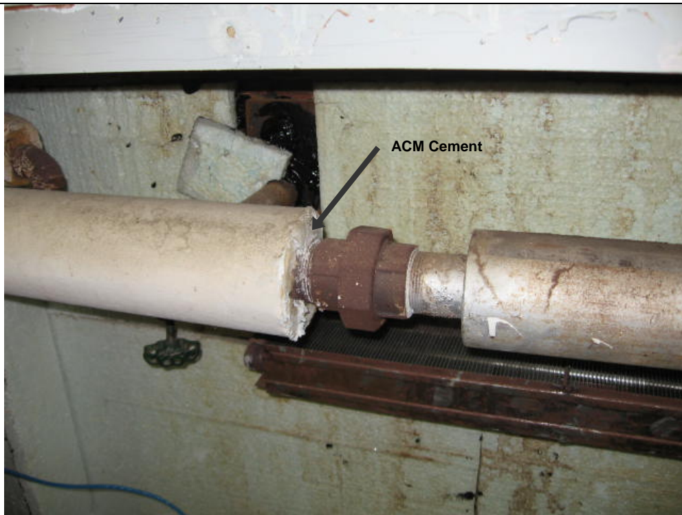
Photograph 9: ACM cement on end of fiberglass pipe wrap in Room No. 1-10 (Sample No. ACM 30).
