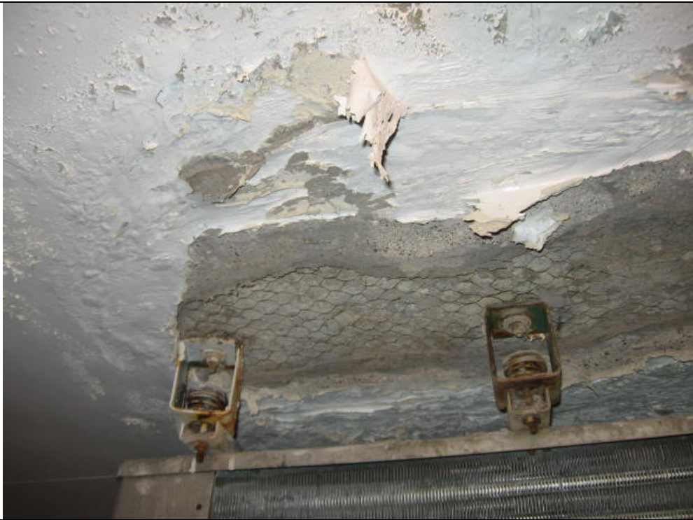
Photograph 15: Damaged plaster ceiling in Room No. B-21 (Freezer Room). (Sample No. ACM 47). Note that although analysis of this material showed no asbestos was detected, material should be treated as asbestos based on positive results of similar samples and non-homogeneous nature of material.
