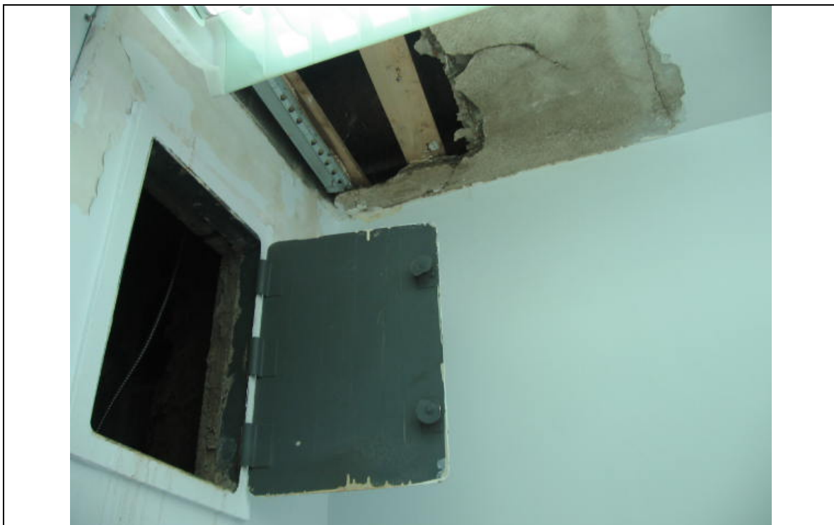
Photograph 12: Damaged ACM plaster ceiling, Room No. 1-16.
