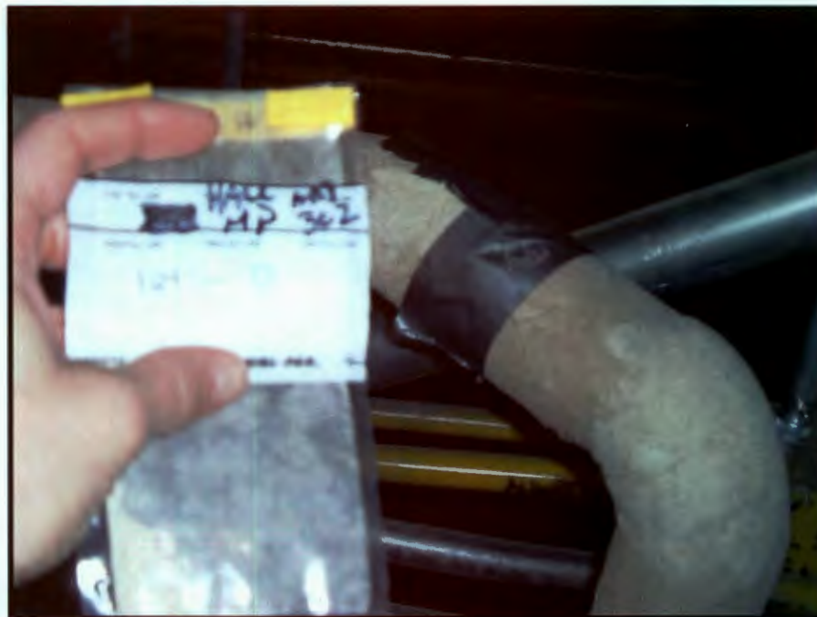
Photograph 52: Sample 124-32-53, Third Floor / Mudding on Pipe Elbow
