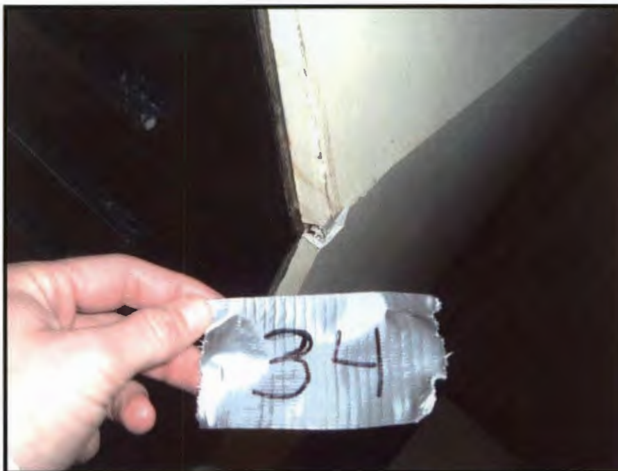
Photograph 33: Sample 124-B8-34, Ceiling Material under Stair, First Landing up from Basement / Drywall Joint Compound
