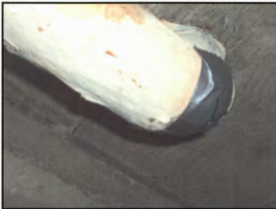
Photograph 10: Sample 124-B7-10, Above Ceiling Tile, Smaller White-Coloured Pipe / Mudding on Pipe Elbow
