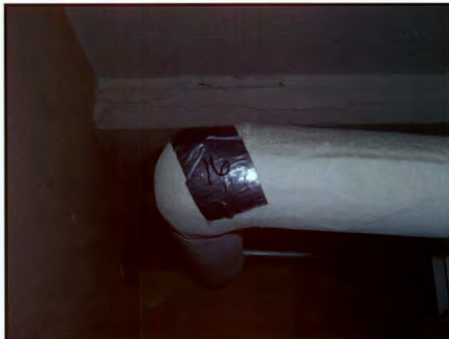
Photograph 16: Sample 124-B5-16, Hot Water Return Line (Smaller) / Pipe Elbow Mudding
