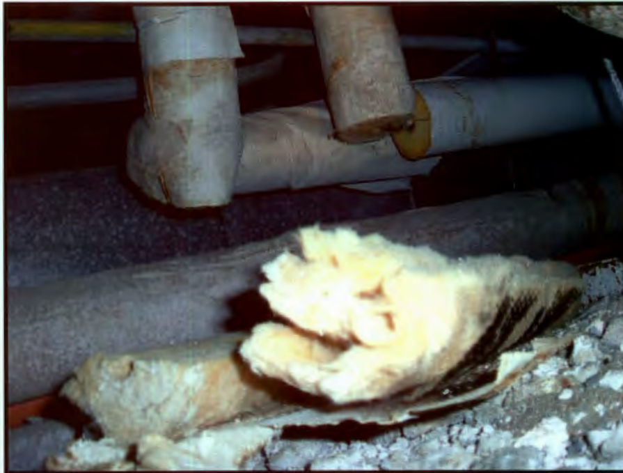
Photograph 31: Sample 124-129-32, First Floor Ceiling Space / Mudding on Pipe Elbow
