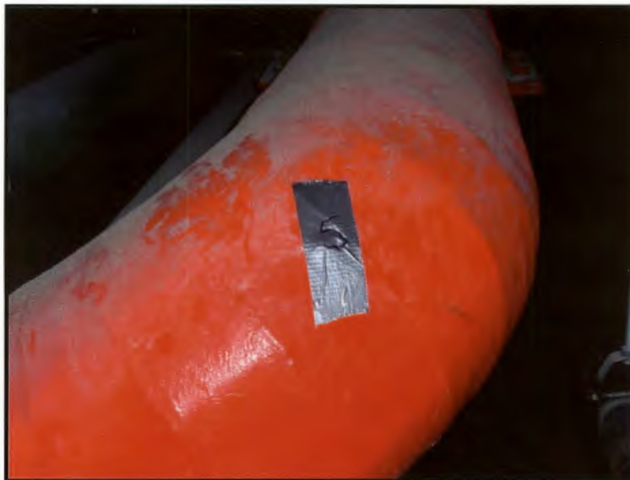
Photograph 5: Sample 124-B1-5, Orange Pipe, High Pressure Steam / Mudding on Pipe Elbow
