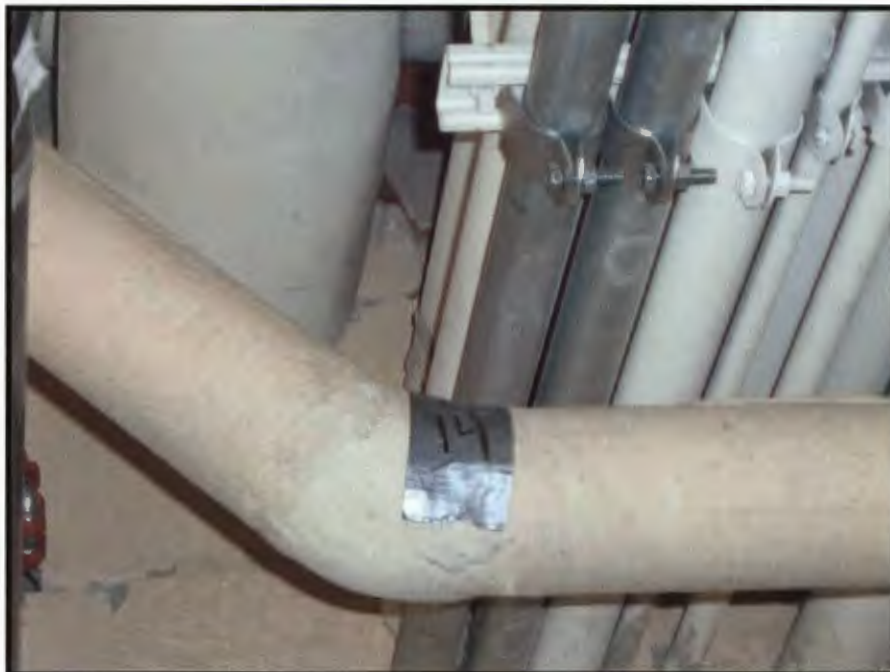
Photograph 14: Sample 124-B4-14, Hot Water Heating Return Pipe / Mudding on Pipe Elbow
