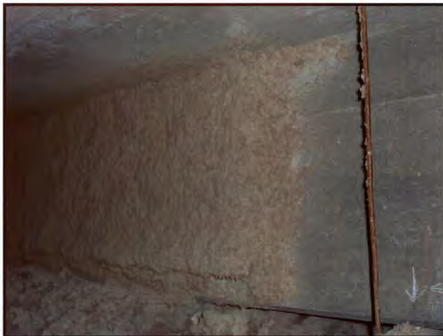
Photograph 3: Sample 124-B1-3 / Spray-Applied Insulation
