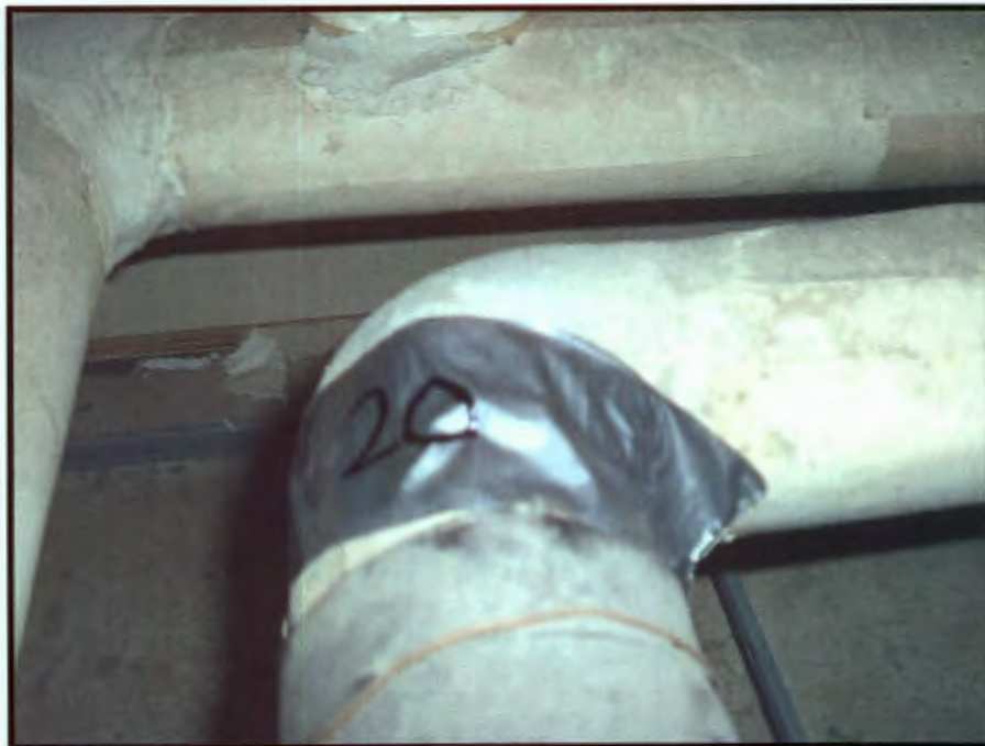
Photograph 19: Sample 124-11-20, Hot Water Heating Return / Mudding on Pipe Elbow
