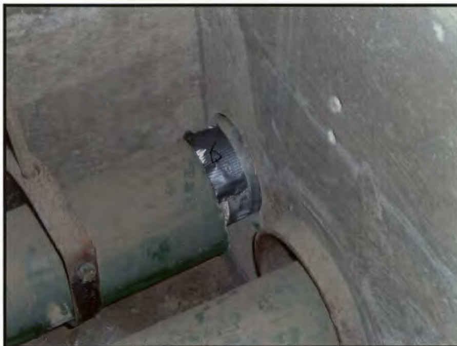
Photograph 6: Sample 124-B1-6, Green Pipe, High Pressure Condensate / Mudding on Straight Run
