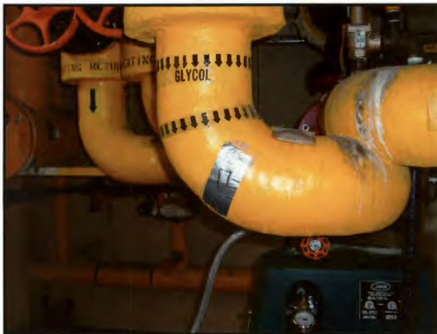
Photograph 17: Sample 124-B6-17, Hot Water Heating Return (Yellow Pipe) / Mudding on Pipe Elbow
