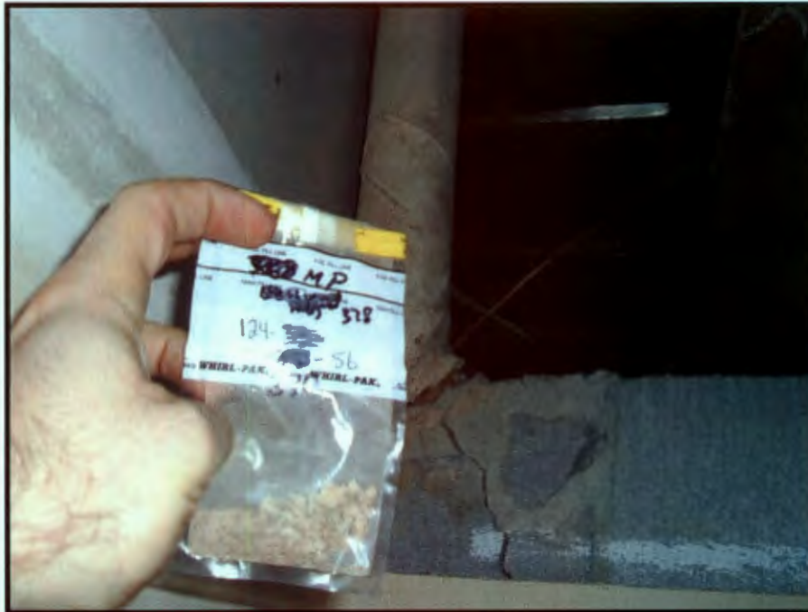
Photograph 55: Sample 124-370-56, Third Floor Storage Room / Mudding on Pipe Elbow
