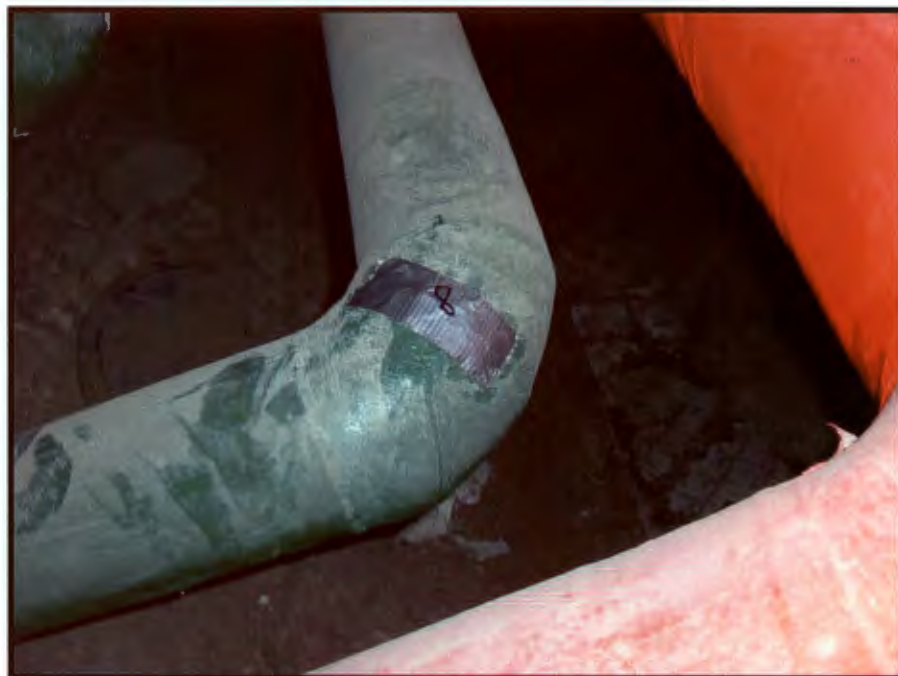
Photograph 8: Sample 124-B1-8, Green Pipe, Condensate Return / Mudding on Pipe Elbow
