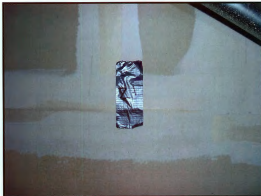
Photograph 20: Sample 124-11-21, from Ceiling Space / Drywall Joint Compound
