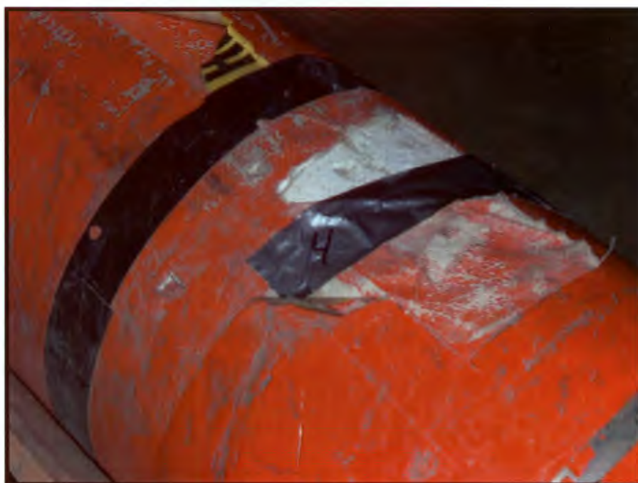
Photograph 4: Sample 124-B1-4, Orange Pipe, High Pressure Steam / Mudding on Straight Run
