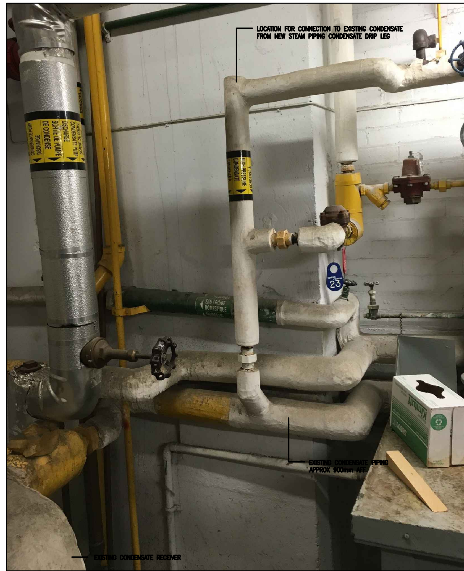
1 MISCELLANEOUS PIPING NEAR CONDENSATE RECEIVER M06 NTS
