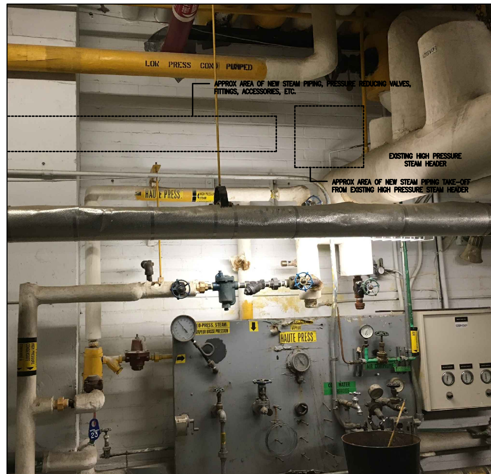
4 HIGH PRESSURE STEAM HEADER M06 NTS
