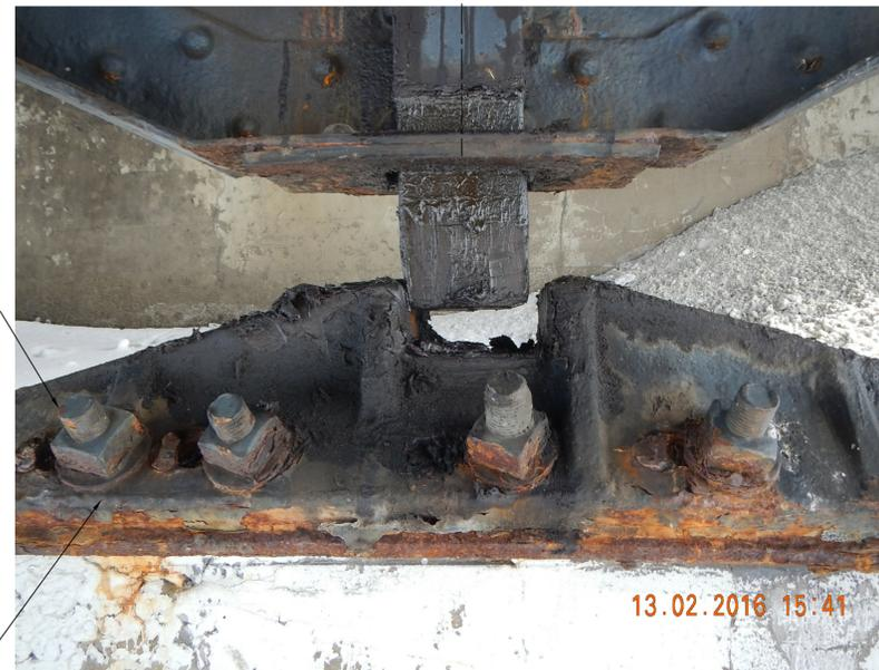
REMOVE AND SALVAGE EXISTING END LATCH RECEIVER FOR RE-USE. CLEAN END LATCH RECEIVER AND APPLY TWO COATS OF ZINC RICH PAINT PRIOR TO REINSTALLATION.
