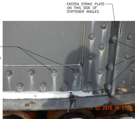
REMOVE THESE TWO (2) RIVETS. FASTEN CONNECTION ANGLE AT THIS LOCATION WITH TWO (2) M22 BOLTS.
