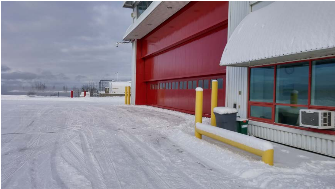
Figure 4: Hangar doors, and buried concrete apron
