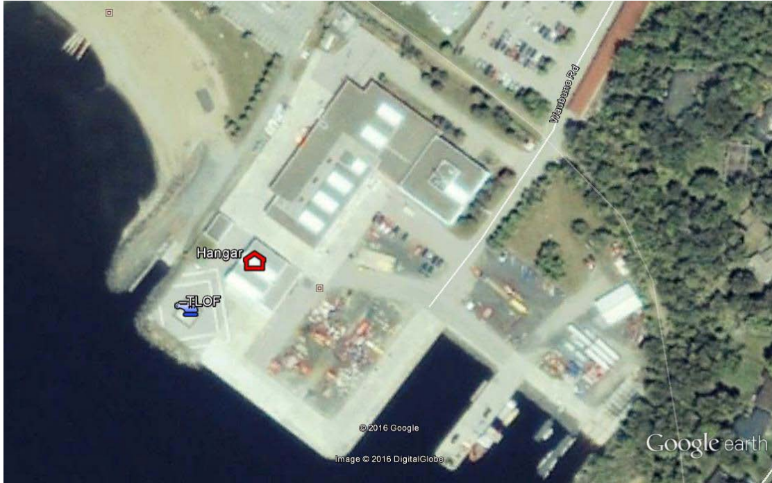
Figure 3: Hangar and TLOF are at CCG Base Parry Sound
