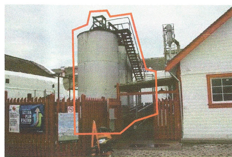
4B TWO EXISTING FISH OIL TANKS, RELATED PIPING, VALVES AND STAIR HANDRAILS.
