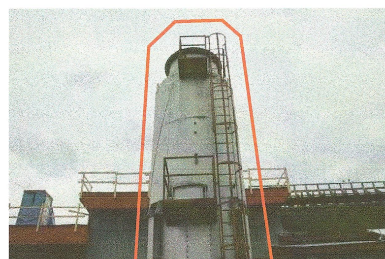
9A EXISTING "STINKEROO" TANK AND RELATED LADDER AND PLATFORMS
