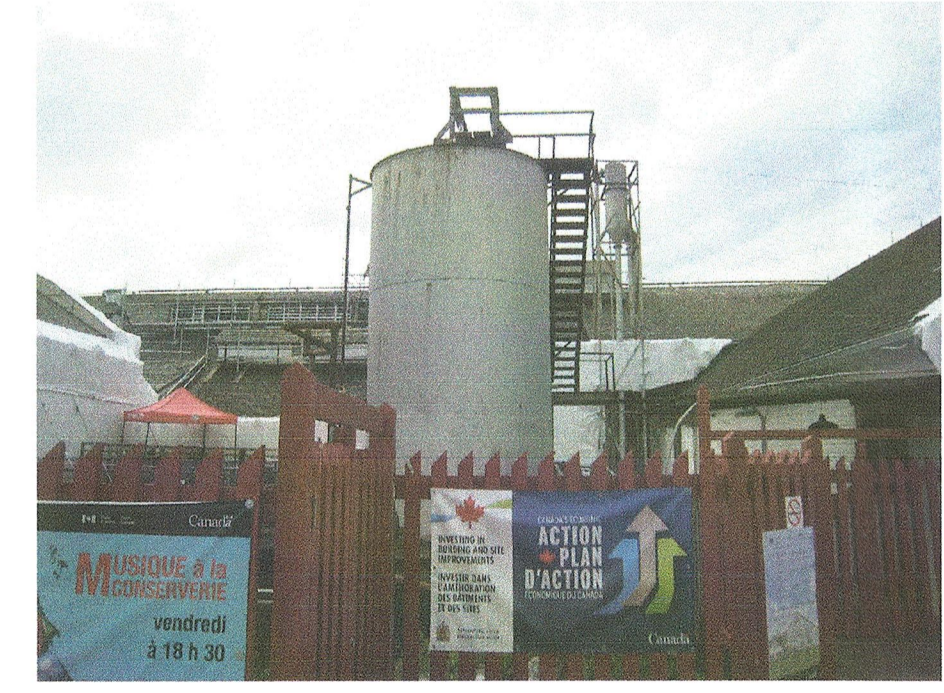
FISH OIL TANKS - 6
