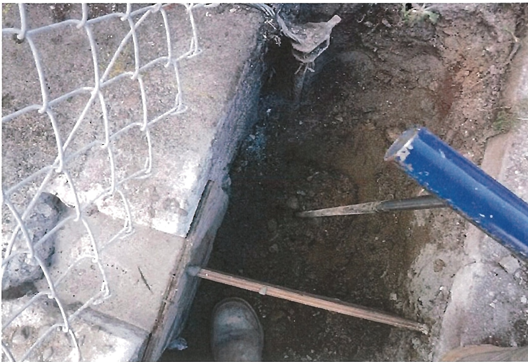
Photo # 8: Subgrade Soil (Dyke FILL) exposed in test pit
