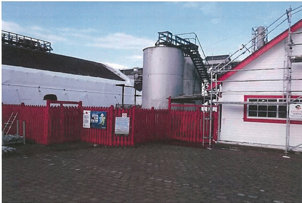
Photo # 5: Fish Oil Tanks ( 2 nos.) Artifact on pile deck
