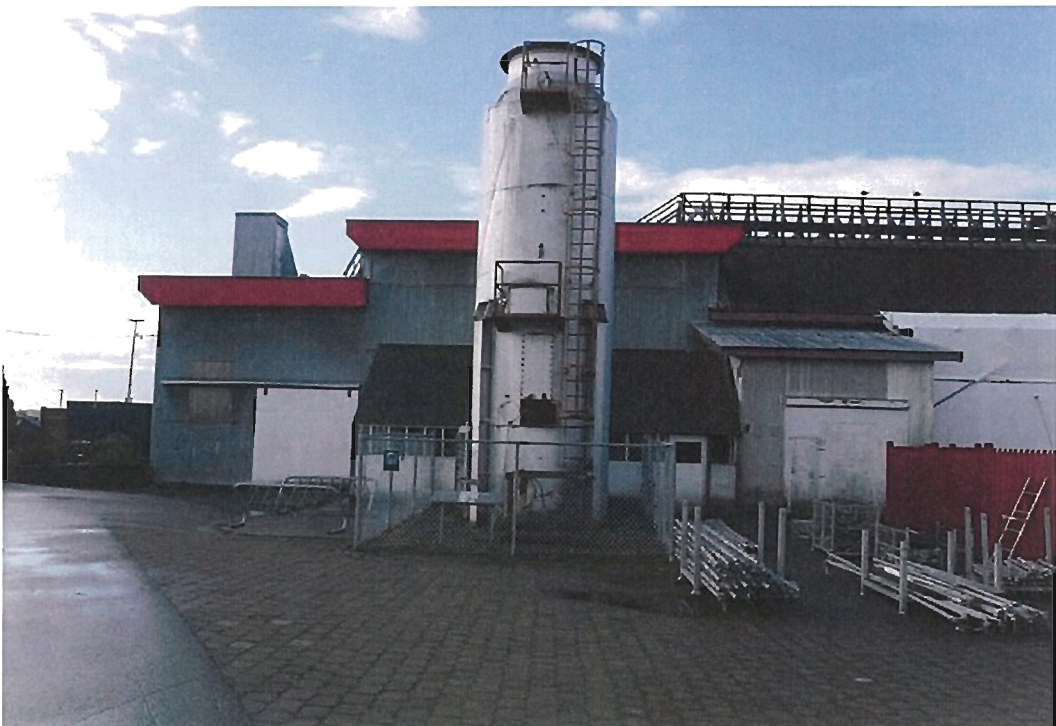
Photo # 4: Stinkeroo Tank Artifact on crown of old dyke
