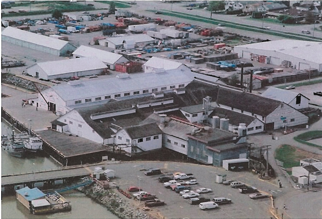
Photo # 3: Present Cannery Site, showing a new dyke in adjacent to Site
