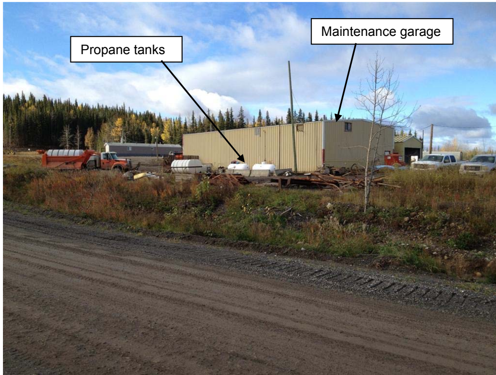
Photograph 3: East side of maintenance garage and equipment, looking southwest.
