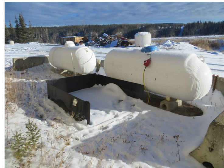
EXISTING PROPANE TANKS TO BE RELOCATED
