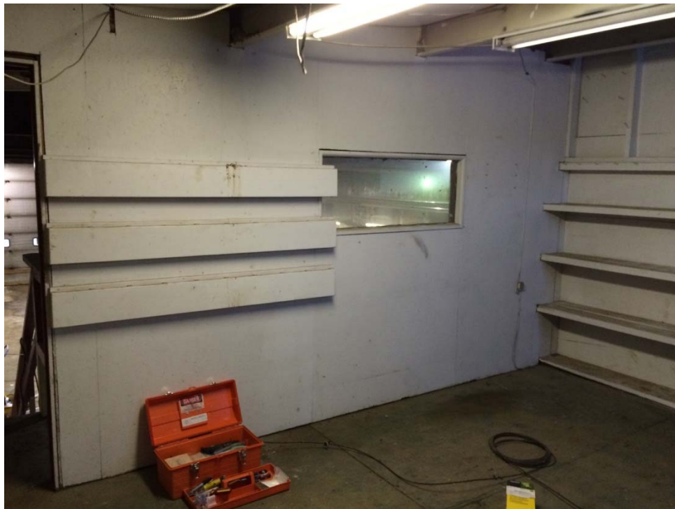
Photograph 4: Sample P2 – Maintenance Garage – Lead-containing green floor paint within the upper mezzanine area collected to the right of the orange toolbox.
