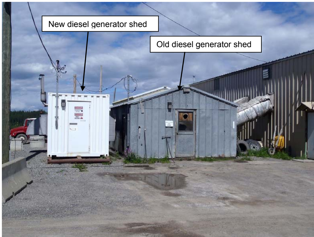
Photograph 2: New generator shed and old generator shed to the west of the maintenance garage, looking northeast.
