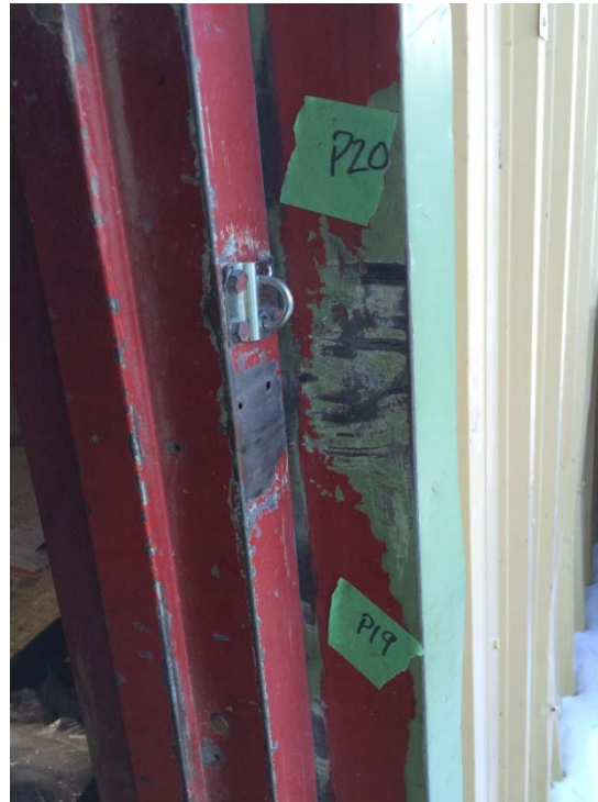
Photograph 7: Samples P19 and P20 – Maintenance Garage – Lead-containing red (P19) and green (P20) paints on the man-door entrance.
