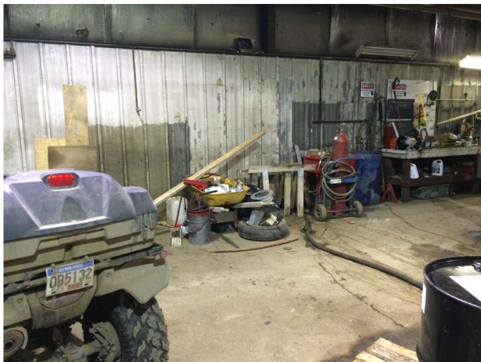
Photograph 6: Samples P21 and 22 – Maintenance Garage – Lead-containing white (peeling) and off-white paints on the interior walls.
