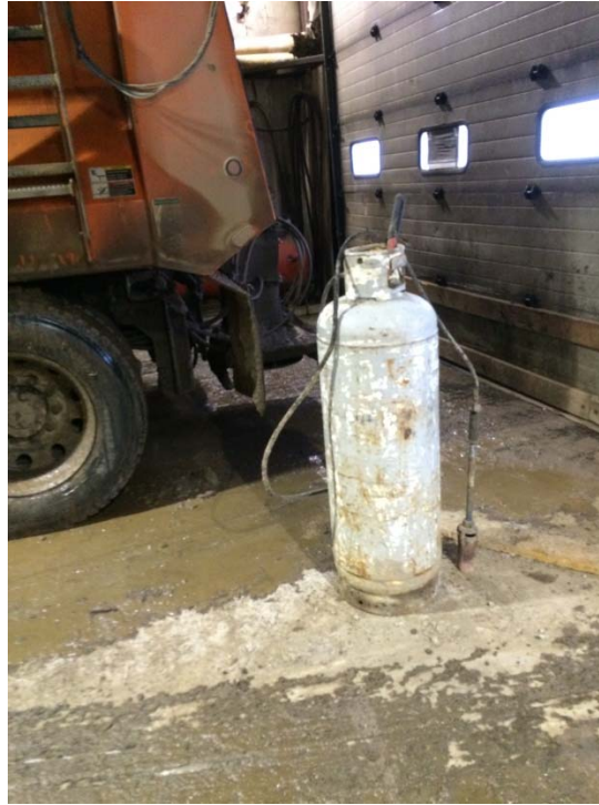
Photograph 21: Maintenance Garage – propane cylinder in the vehicle parking area.
