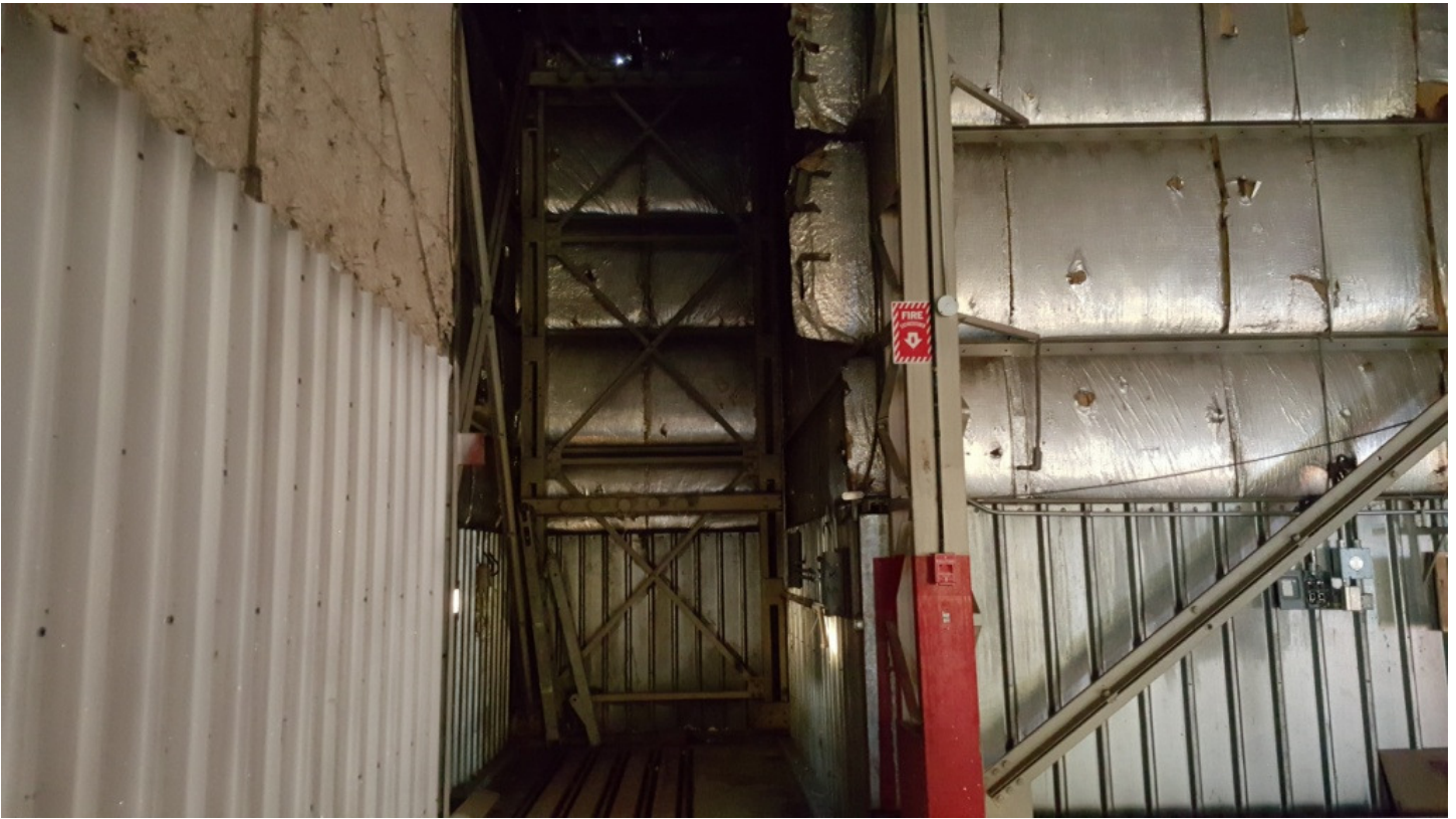
Photo 12. Interior Elevation Showing Column Spacing and Height at Hangar Door Storage Area.
