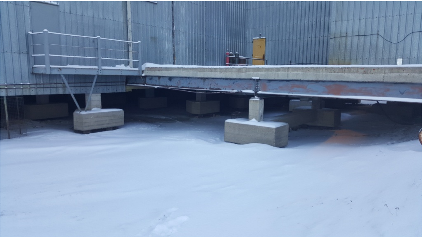
Photo 33. Photo Showing Building Footings
