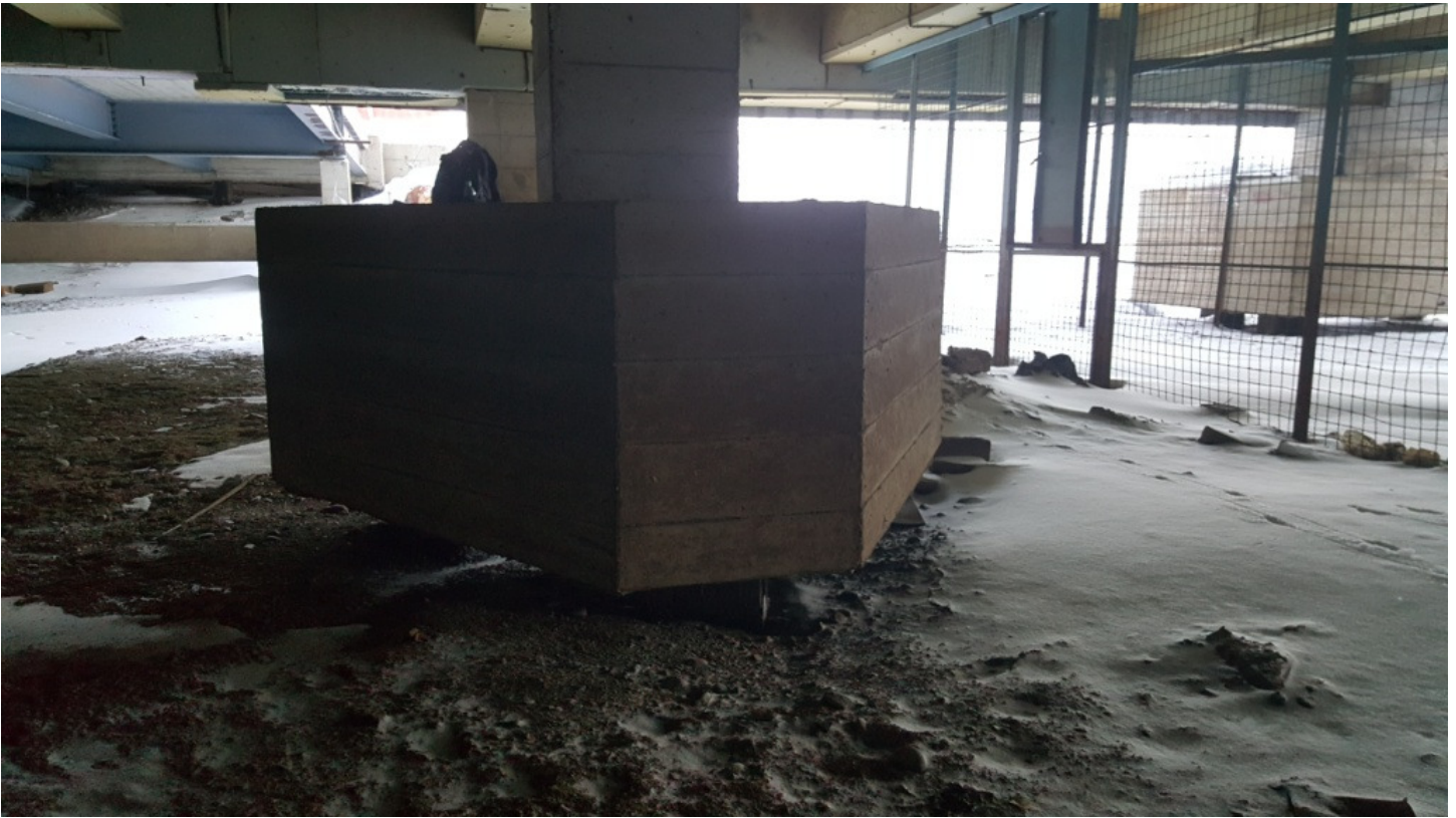
Photo 38. Detail Photo of Building Footing.
