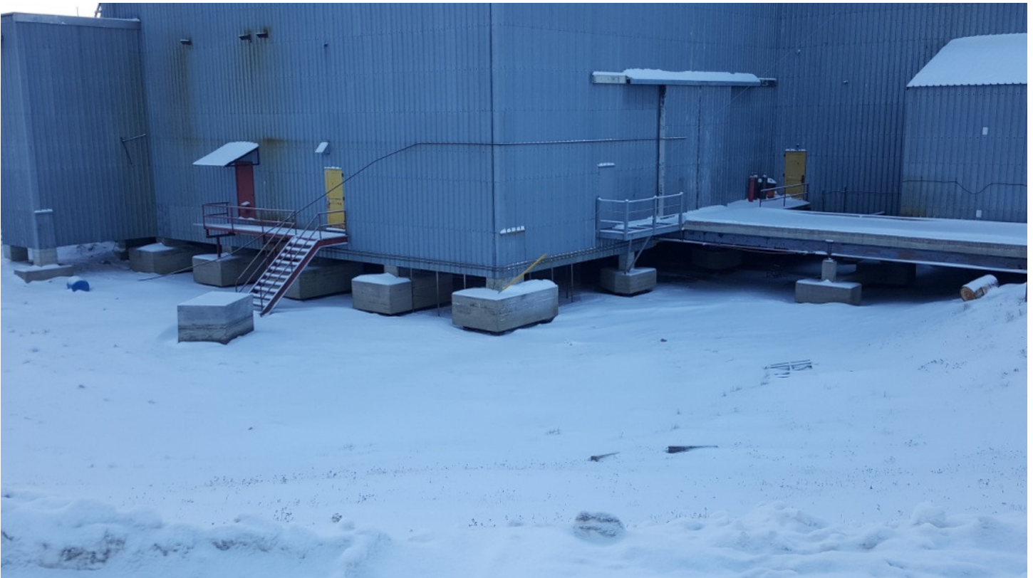
Photo 23. Photo Showing Building Footings
