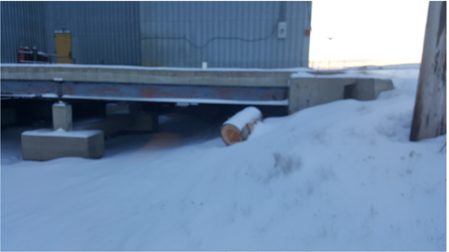
Photo 32. Photo Showing Building Footings
