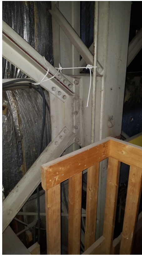
Photo 20. Column Connection Detail above office area.
