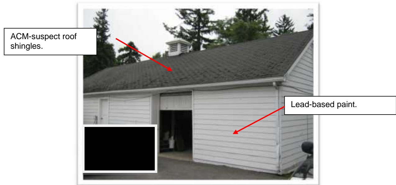
Photo 1: Exterior view of the Storage Shed. The exterior white paint has been tested and confirmed to be lead-based. The asphaltic roofing materials are ACM-suspect.
