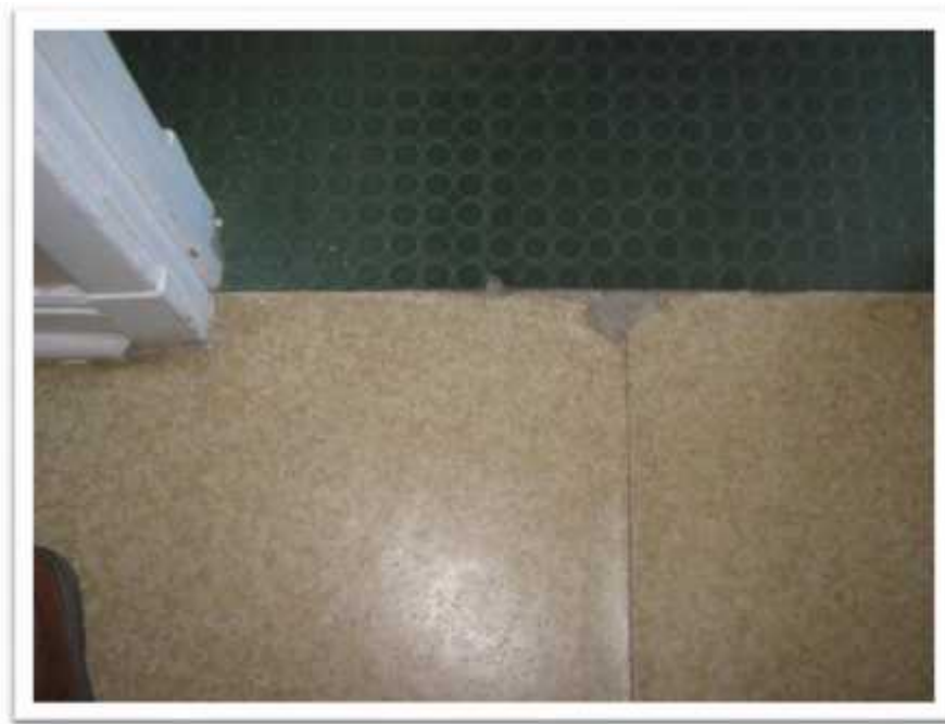
Photo 11: Brown vinyl sheet flooring sampled in the ground floor rear office does not contain asbestos (Samples 243867-08A-C).
