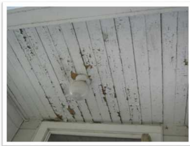
Photo 20: Exterior white porch paint at front entrance contains 200,000 ppm lead (Sample 243867-LP-02).
