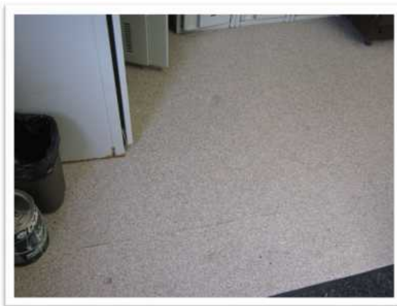
Photo 4: Vinyl sheet flooring in Survey Location #7 has been tested (Samples 94189-04A-C) and confirmed to contain no asbestos.
