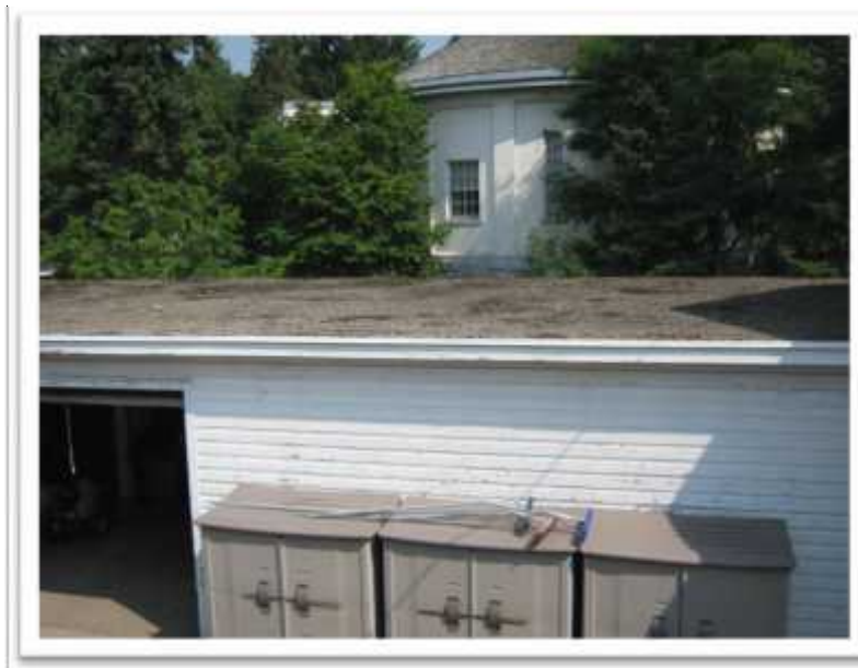
Photo 3: Roof of the Storage Garage. The asphalt materials are a suspected non-friable ACM.
