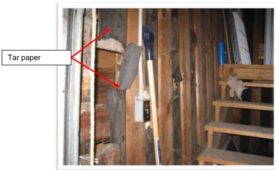
Photo 4: Tar paper has been tested and does not contain asbestos.
