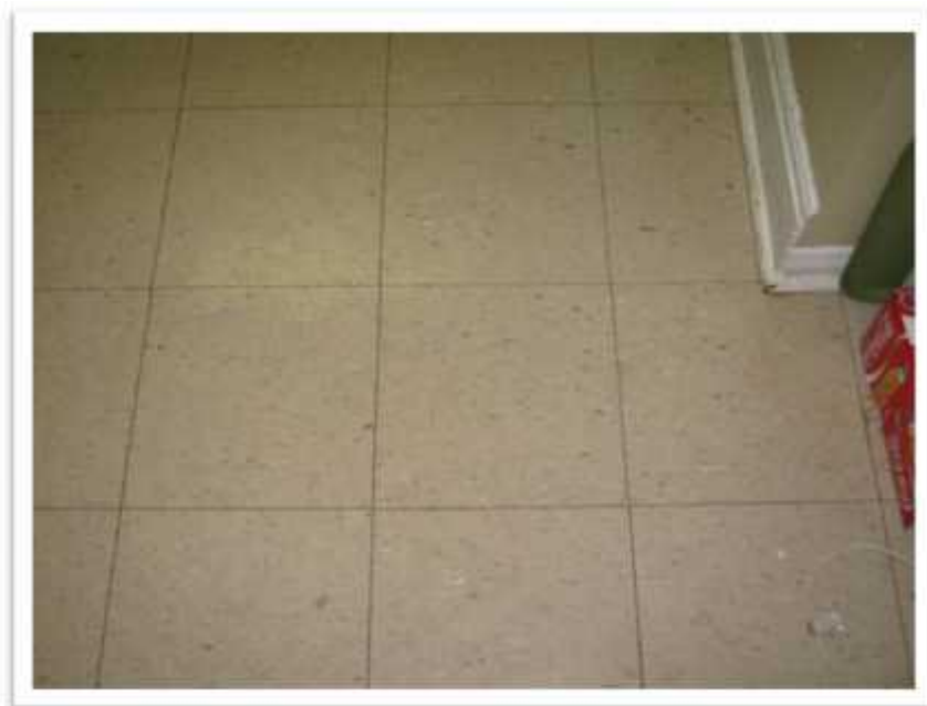
Photo 12: Brown 12" x 12" vinyl tile flooring sampled in the ground floor rear common area does not contain asbestos (Samples 243867-09A-C).
