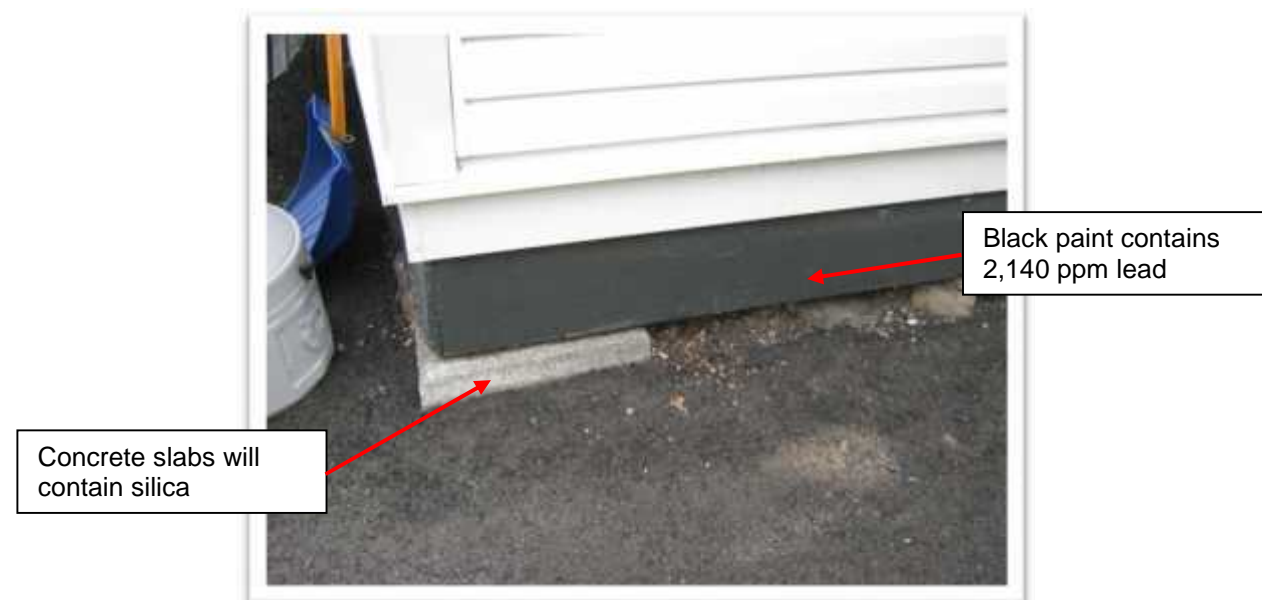
Photo 5: The exterior black paint (Sample 94189-LP-03) on the wood skirts at the base of the building's exterior contains 2,140 ppm lead. This is classified as a lead-based paint. The concrete corner slabs will contain silica.
