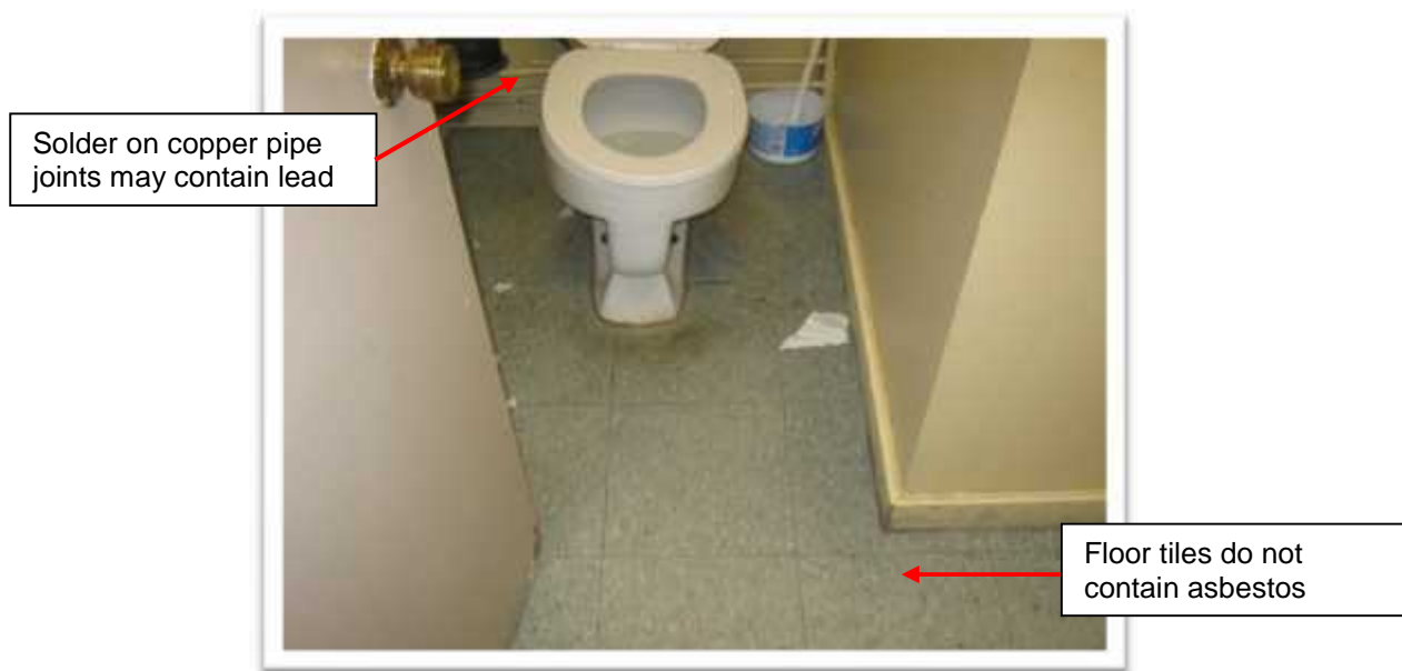
Photo 3: Vinyl floor tiles in Survey Location #5 (Bathroom) have been tested (Samples 94189-03A-C) and confirmed to contain no asbestos.
