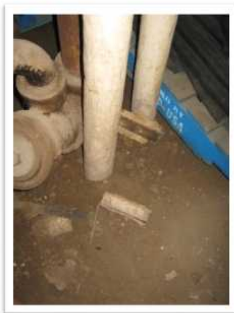
Photo 8: Layered cardboard wrap insulation (Sample 243867-05A) noted on pipes the basement storage/mechanical room contains 20% Chrysotile asbestos in the tar paper layer. Some debris (POOR condition) associated with this material was also noted on the ground in this area.
