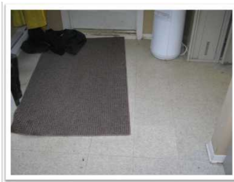
Photo 2: Vinyl floor tiles in Survey Location #3 have been tested (Samples 94189-01A-C) and confirmed to contain no asbestos.
