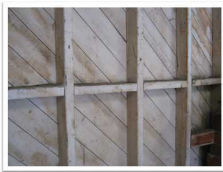
Photo 6: Interior beige paint (Sample 335846-LP-02) contains 4,170 ppm lead. This paint retains its bond with the wood substrate and is on GOOD condition. No remedial action is required.
