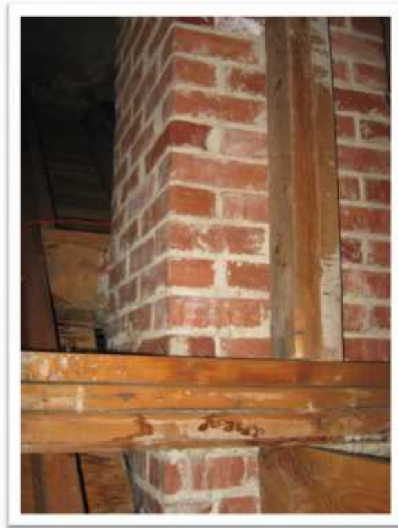
Photo 19: Chimney brick mortar sampled does not contain asbestos (Samples 243867-14A-C).
