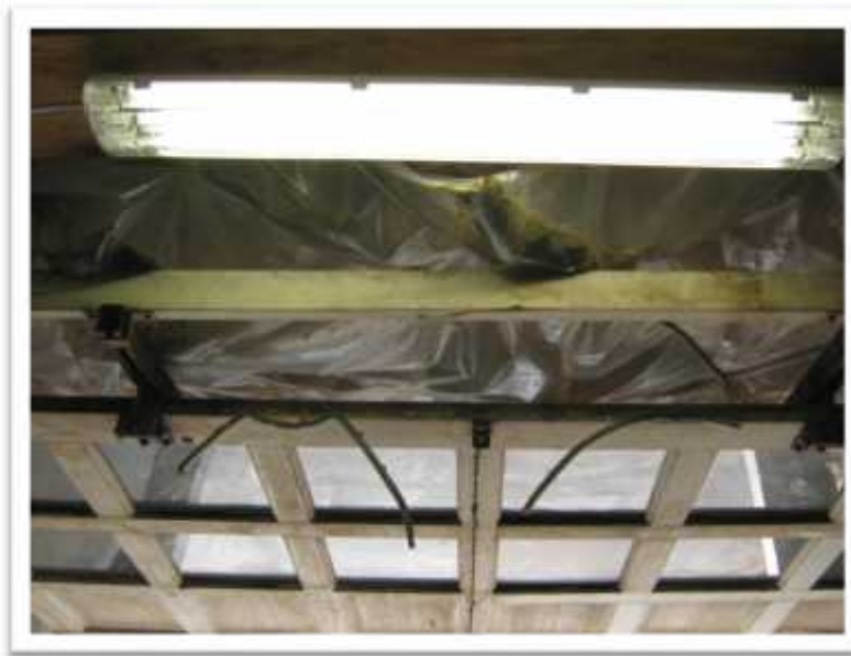
Photo 8: Mould impacted materials above the polyethylene sheeting suspended from the rafters. DST recommends Level II CCA mould remediation.
