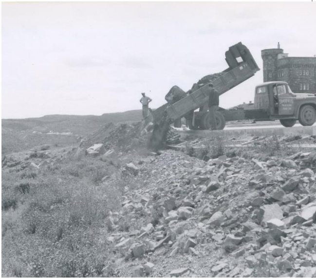
Figure 7. Dumping fill along edge of new parking lot for sidewalks, 1963.
