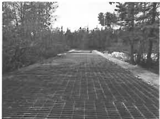
Picture No. 4: Fishway from Step in Fishway to Upstream End
