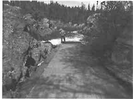
Picture No. 2: Fishway from Corner to Downstream
