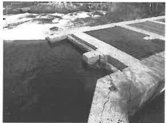
Picture No. 16: Upstream Entrance to Fishway
