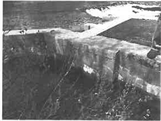
Picture No. 14: Upstream Wall to be repaired
