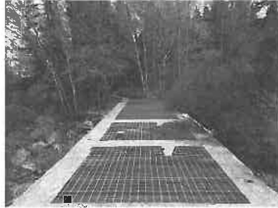
Picture No. 8: From Upstream End Looking to Corner Bend
