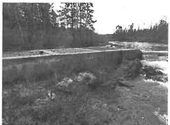
Picture No. 18: Upstream Section of Fishway
