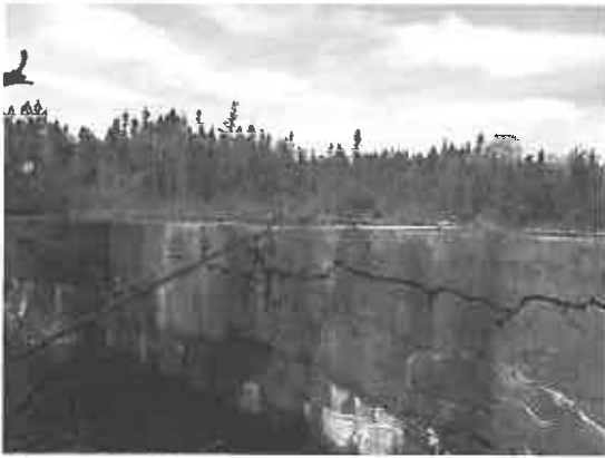
Picture No. 15: Upstream Wall to be Repaired
