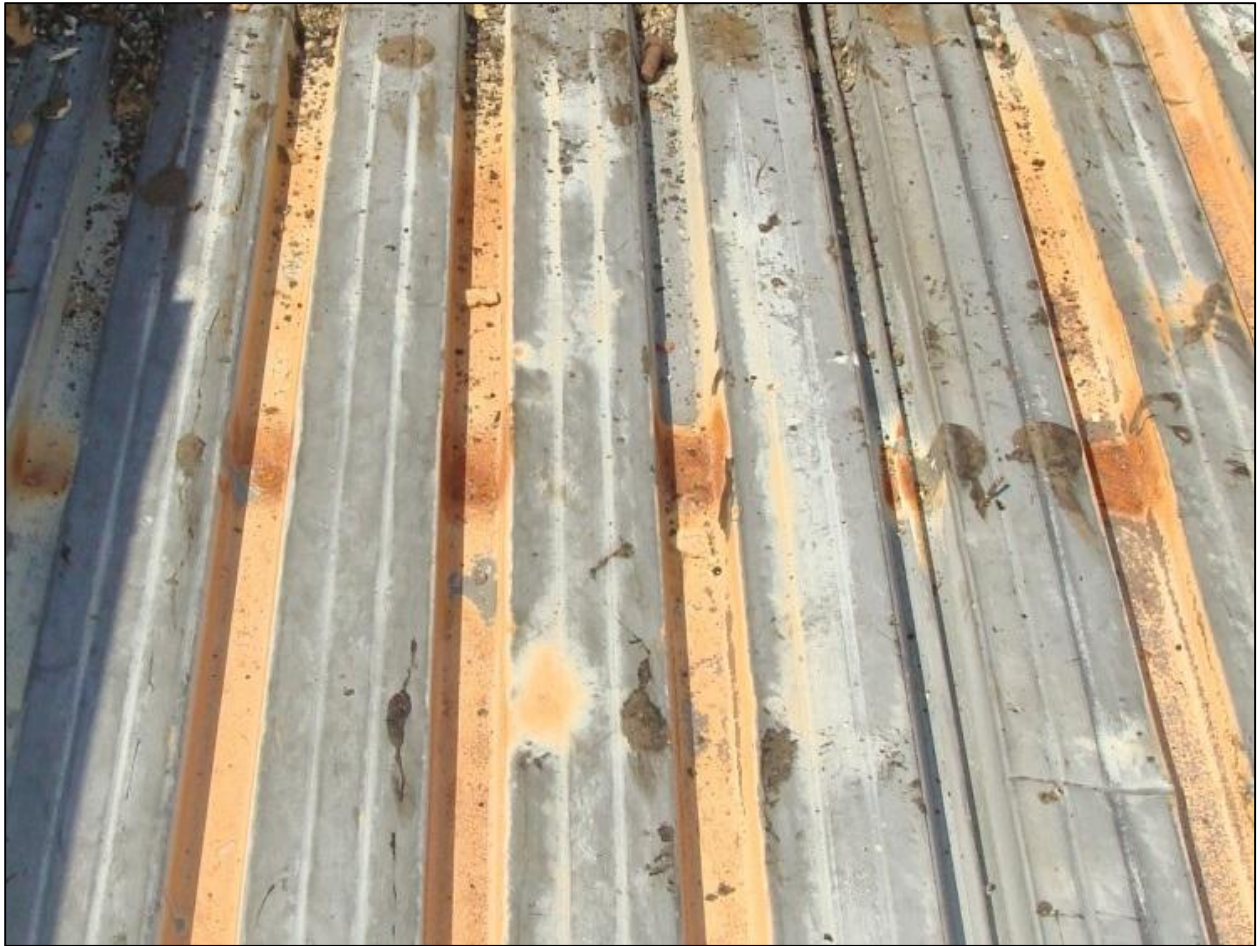
Photo of Level 2: Light to Moderate Corrosion
