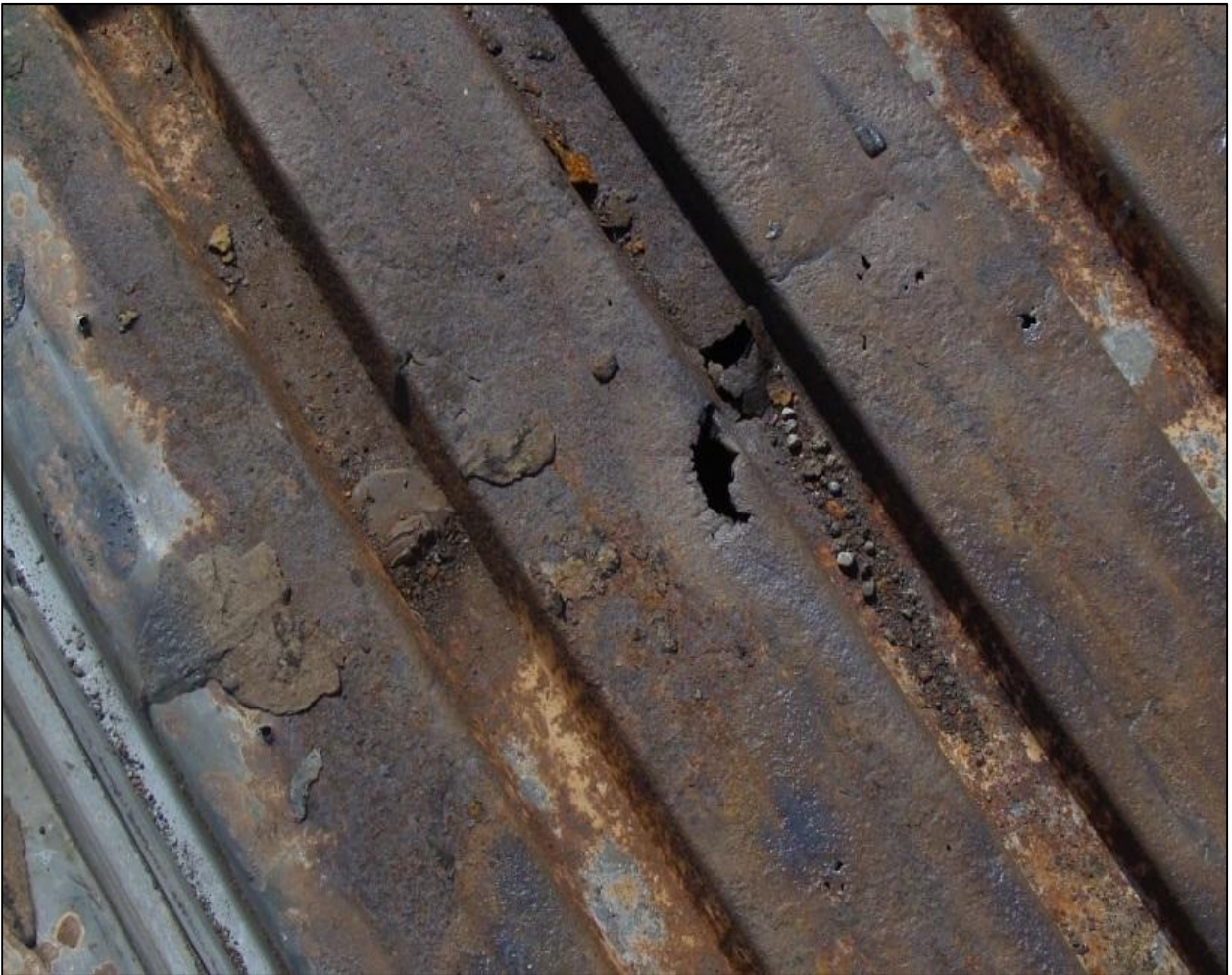
Photo of Level 4: Severe Corrosion With Holes
