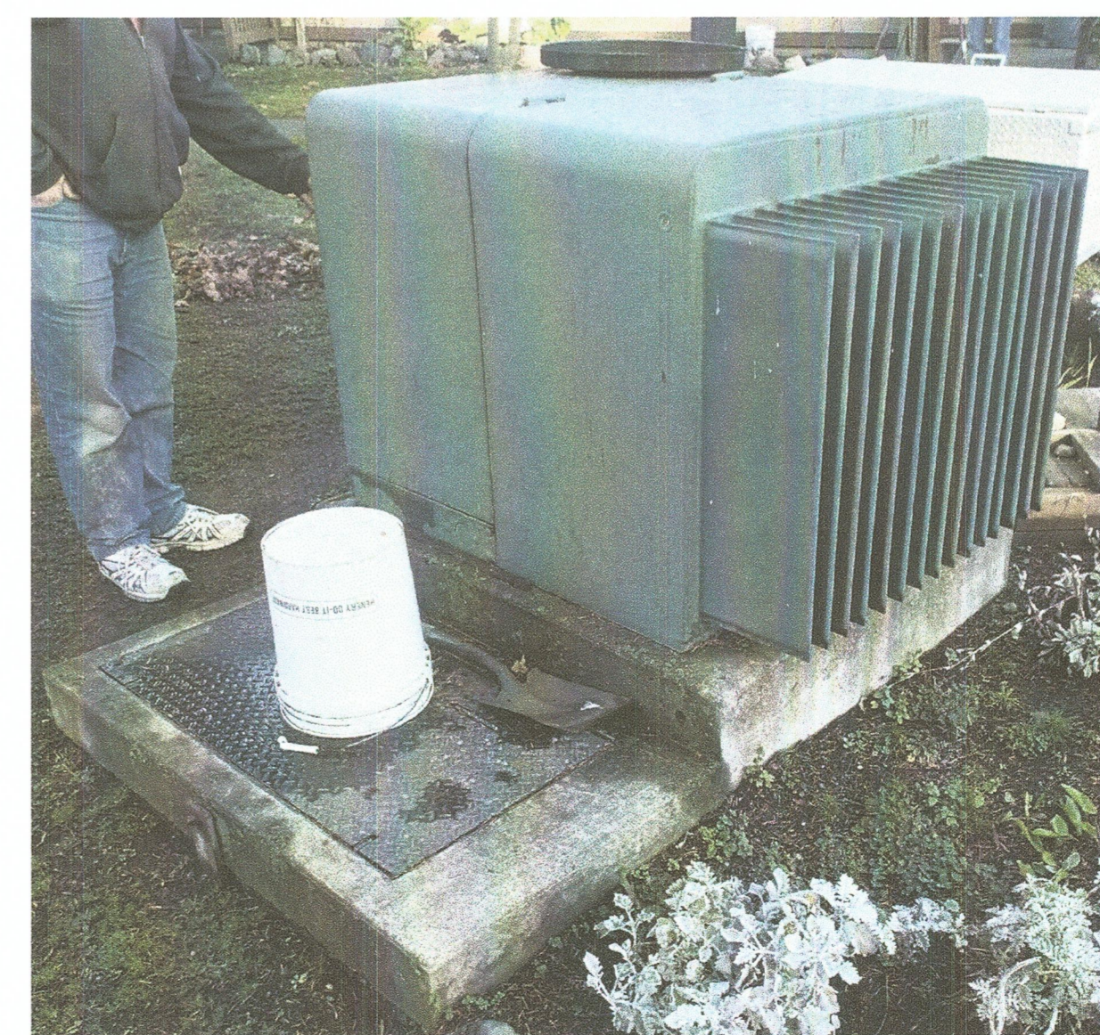
6 EXISTING PADMOUNT TRANSFORMER AND CONCRETE PAD N.T.S.
