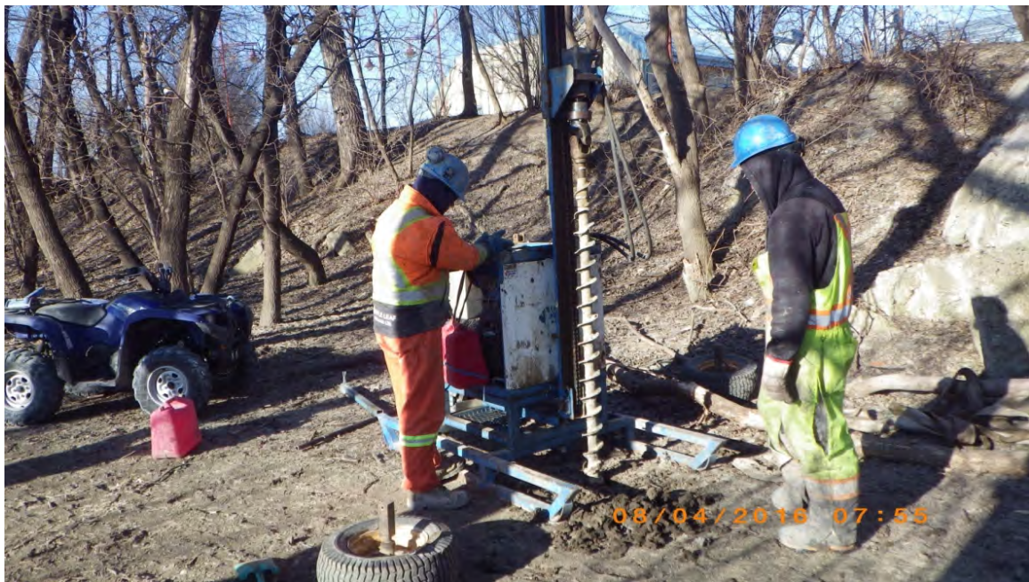
Figure 5. Monitoring soil disruption during geotechnical drilling operations.
