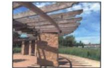
EXIST. 203x102 HSS BEAM TO BE SANDBLASTED & COATED TYP. REFER TO ARCHITECTURAL
