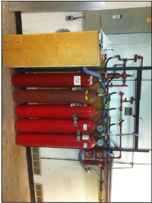
3 PRIMARY CARBON DIOXIDE SYSTEM ON 8th FLOOR
