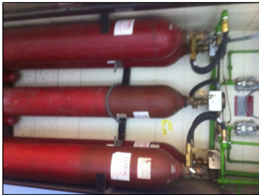
2 BACKUP CARBON DIOXIDE SYSTEM ON 7th FLOOR
